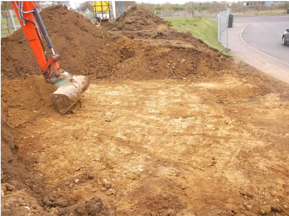
Northern part of site, soil stripping, looking south-east Fig 5
