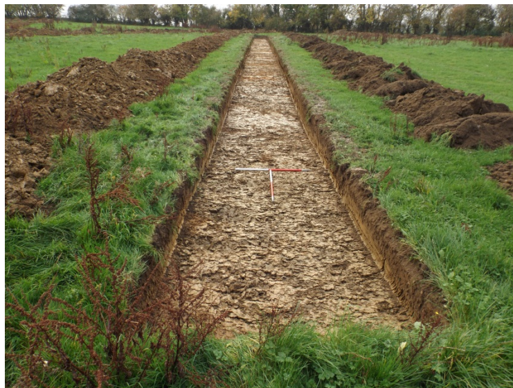
Trench 5, general view, looking south-west Fig 10
