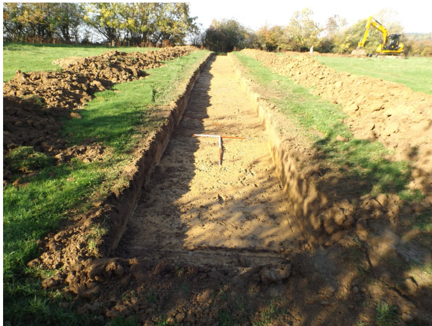
Trench 10, general view, looking north-west Fig 15
