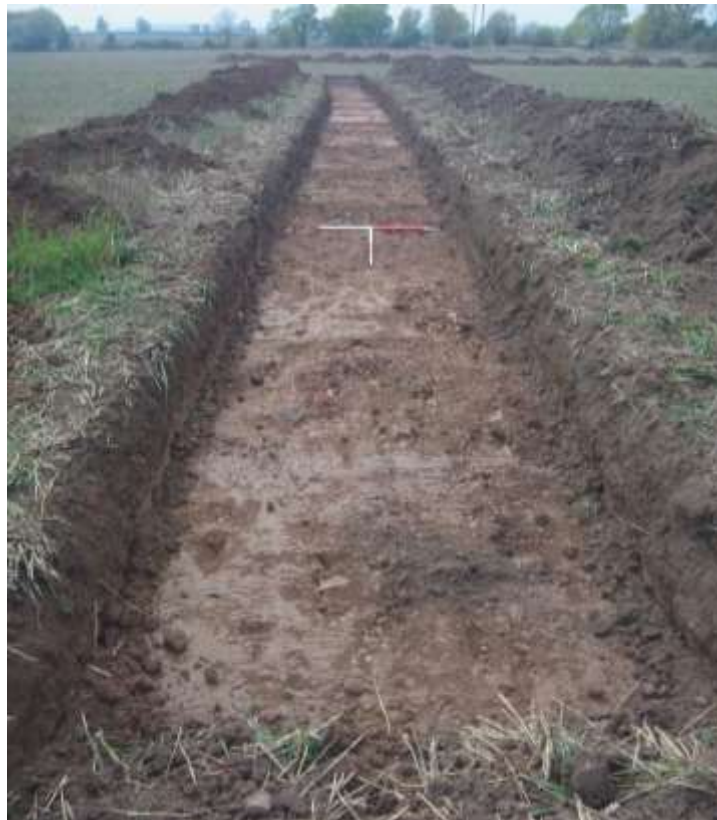
Trench 11, general view, looking south-west Fig 23
