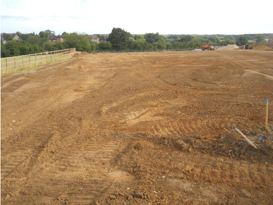
Disturbed ground prior to stripping, looking north-west Fig 5
