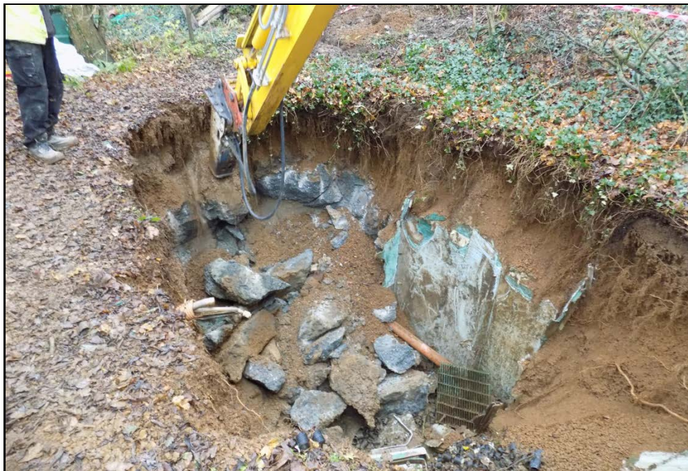
Removing the concrete footing, looking east Fig 2
