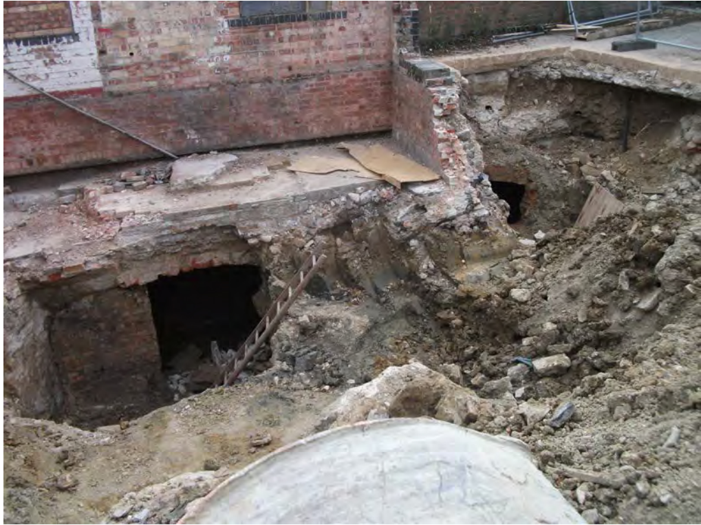
General view of the modern overburden and cellars Fig 3
