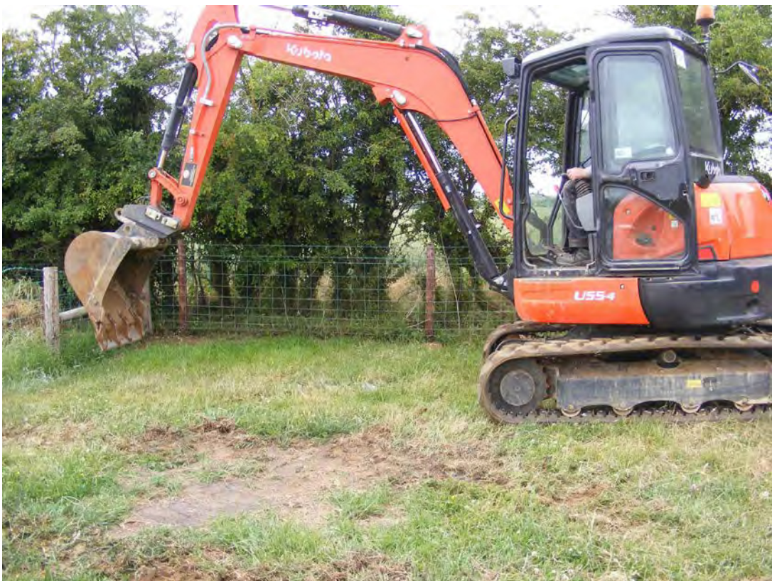
The groundworks in progress Fig 3
