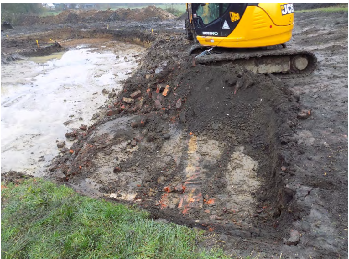
Modern brick footings, south-eastern corner of site, looking north Fig 8
