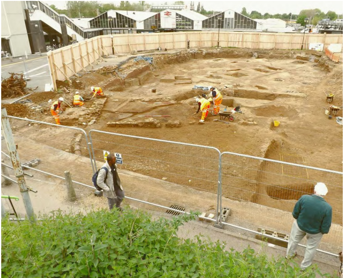
General view of site during excavation, looking north towards the now demolished station Fig 3
