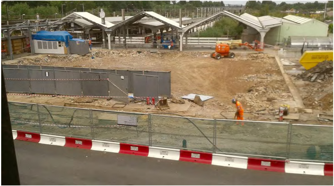
Watching brief during the demolition of the 20th-century station Fig 17
