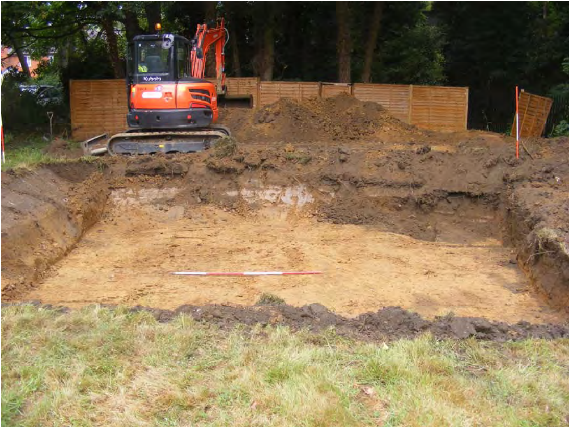
The house plot after soil removal, looking north Fig 5
