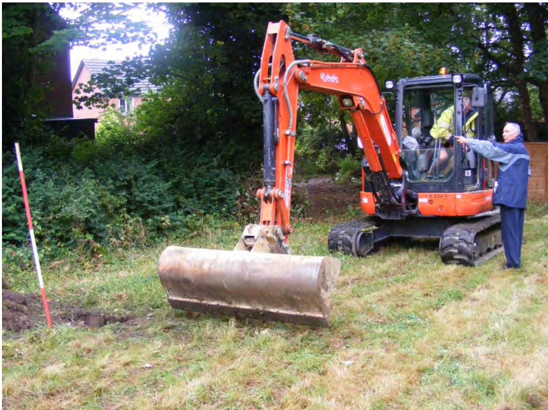
The groundworks in progress Fig 4
