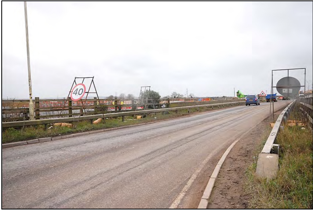
The deck of the Houghton Regis Bridge, looking west Fig 71
