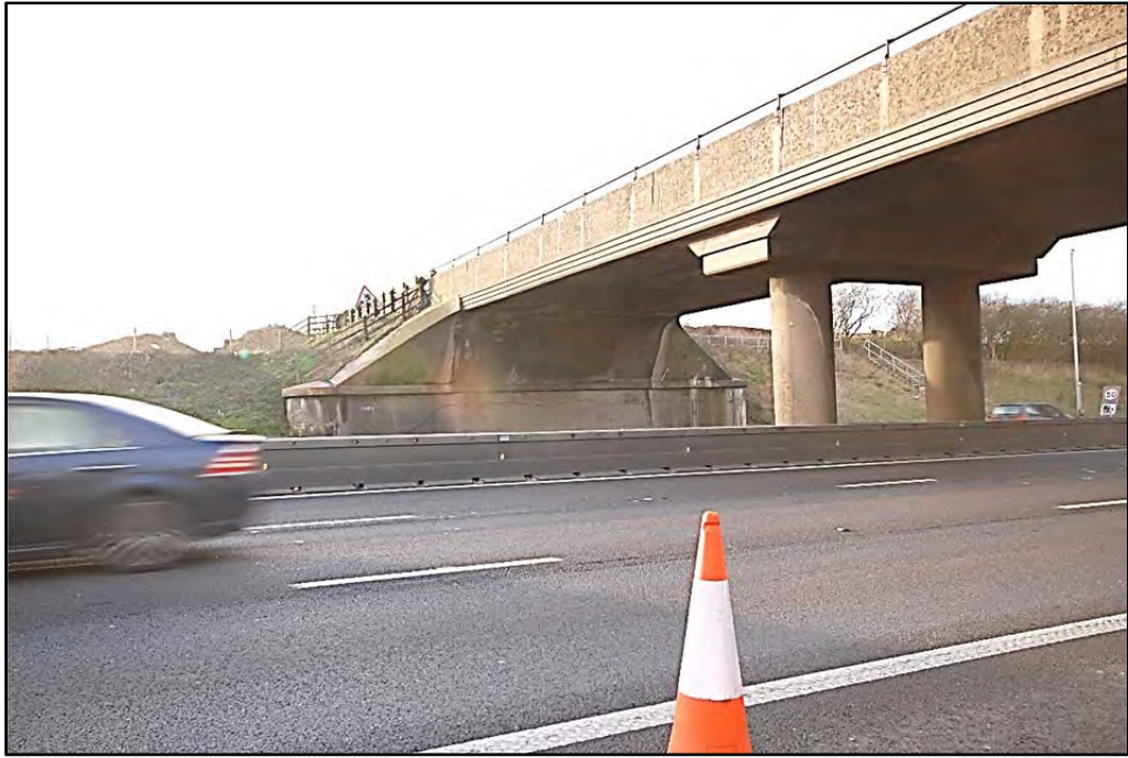
The west abutment wall with scrolls, looking west Fig 63
