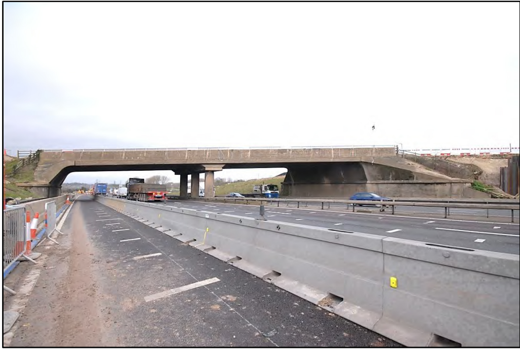
South elevation of Chalton Bridge, looking north Fig 19
