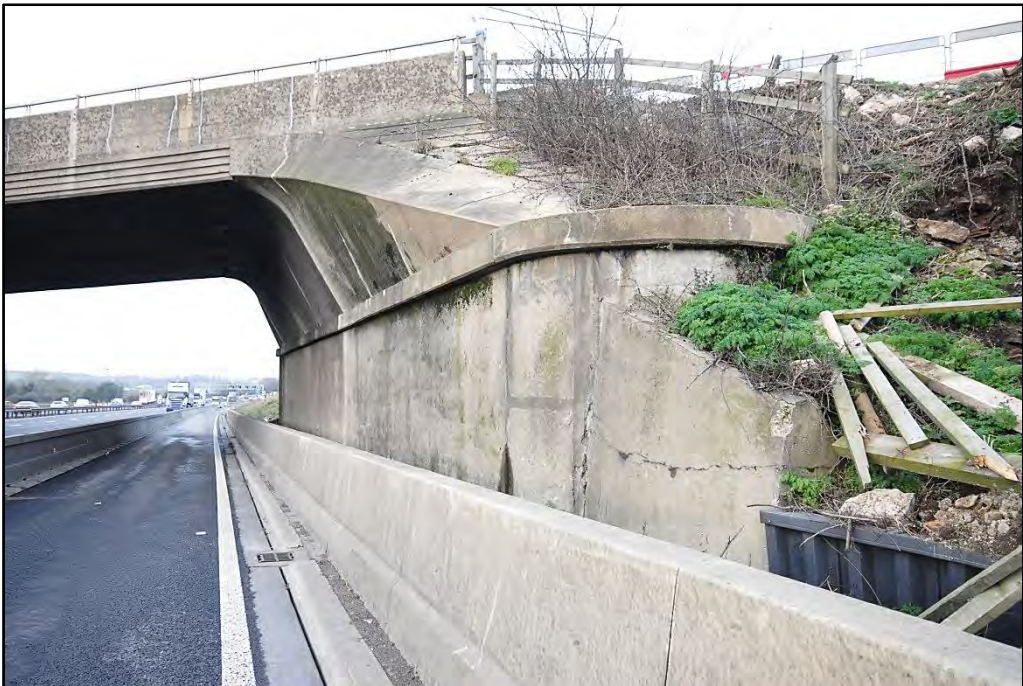
South-eastern scroll of northern bridge, looking north Fig 30
