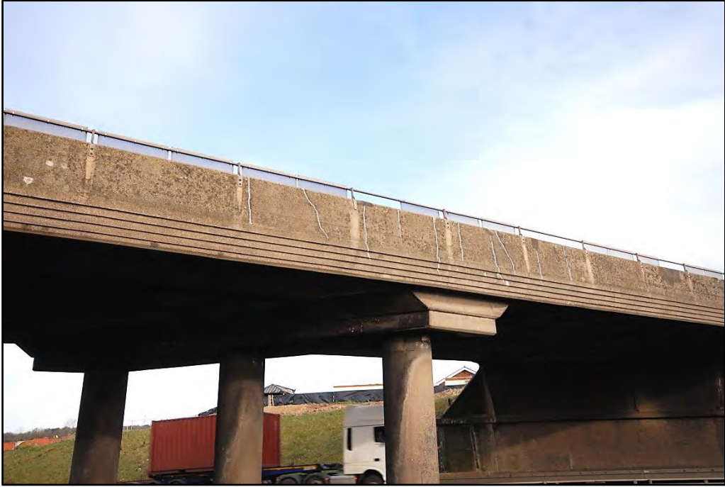
In-filled cracks/joints on the external south elevation of the parapet Fig 49
