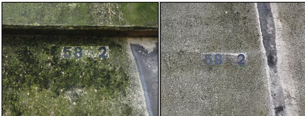
Bridge markings northbound and southbound Fig 16
