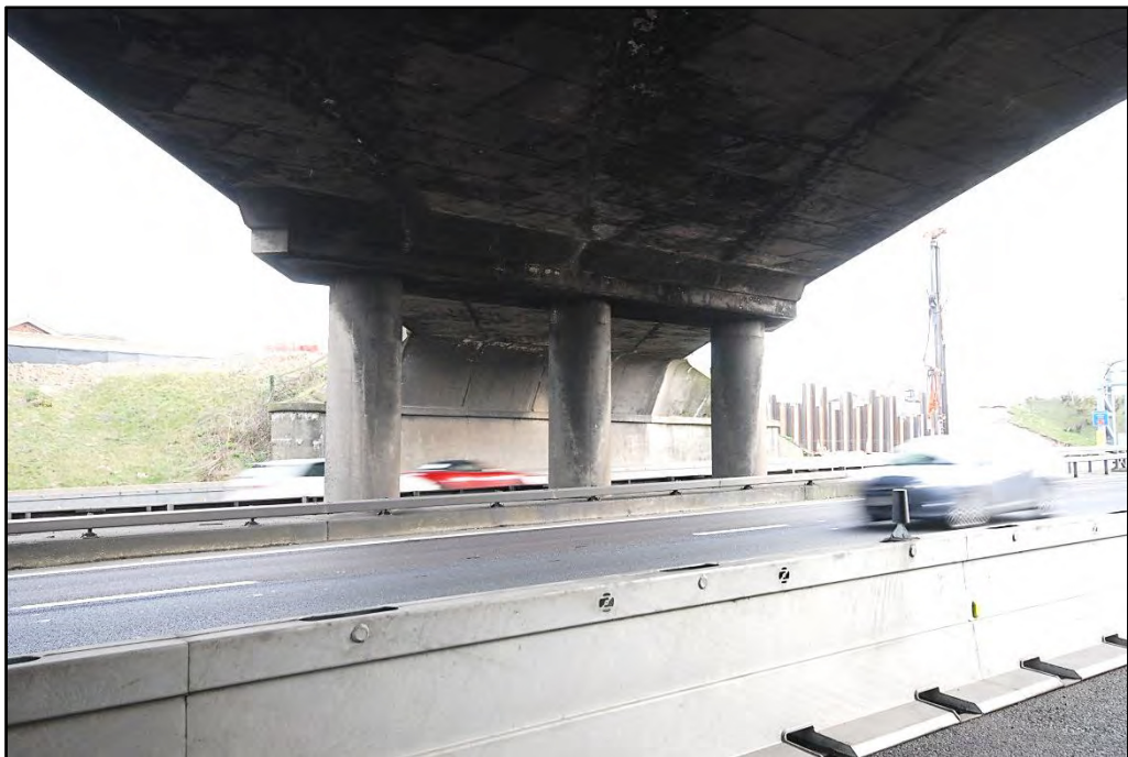
Central reservation and columns, looking south-east Fig 20
