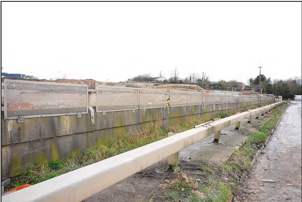
South side parapet guards, path and barrier, looking north-west Fig 37
