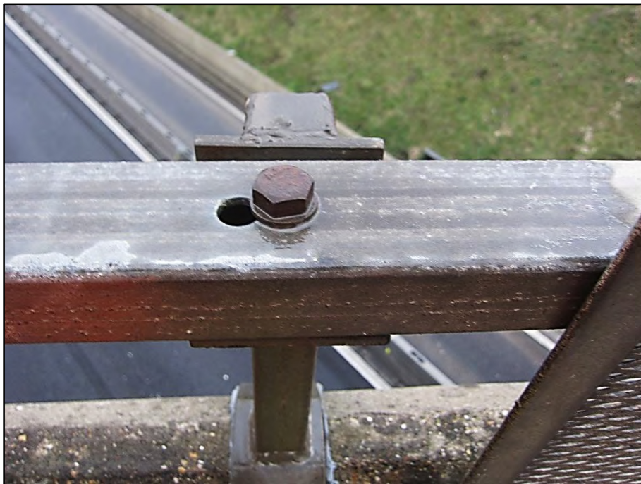
Bolt holes for the railing Fig 41
