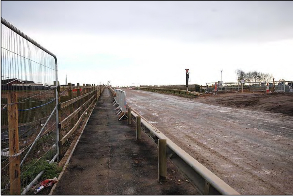
The deck of the Chalton Bridge, looking south-east Fig 36
