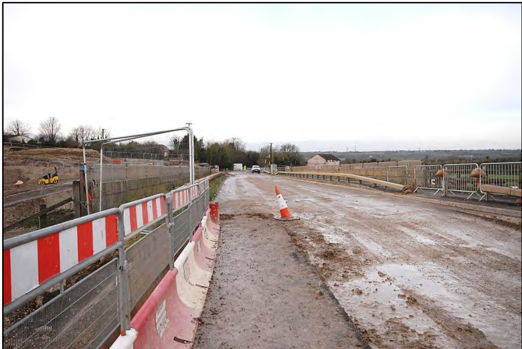
The deck of the Chalton Bridge, looking north-west Fig 35
