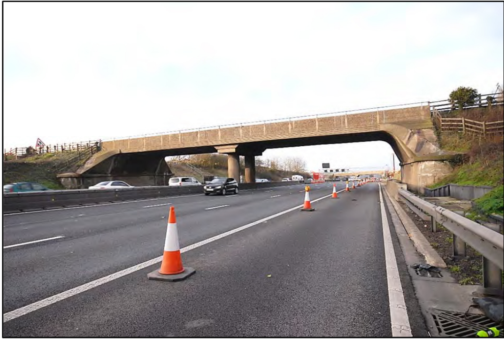
The south elevation, looking north-west Fig 59
