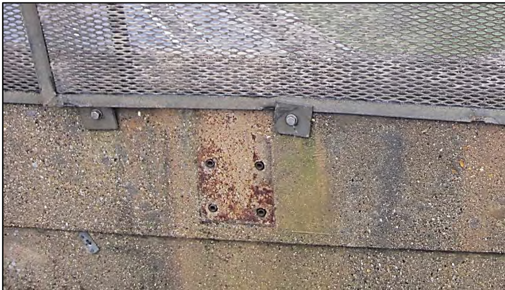
Close-up of bolt holes and cable fixings on north parapet Fig 45
