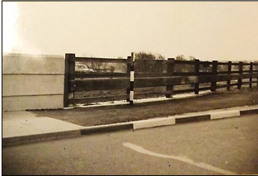
London – Yorkshire Motorway, Junction at Upper Heyford, Photograph No. 4 Fig 12
