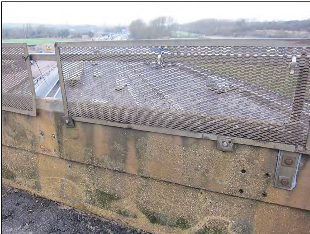
Bolt holes on north parapet, looking north-west Fig 43
