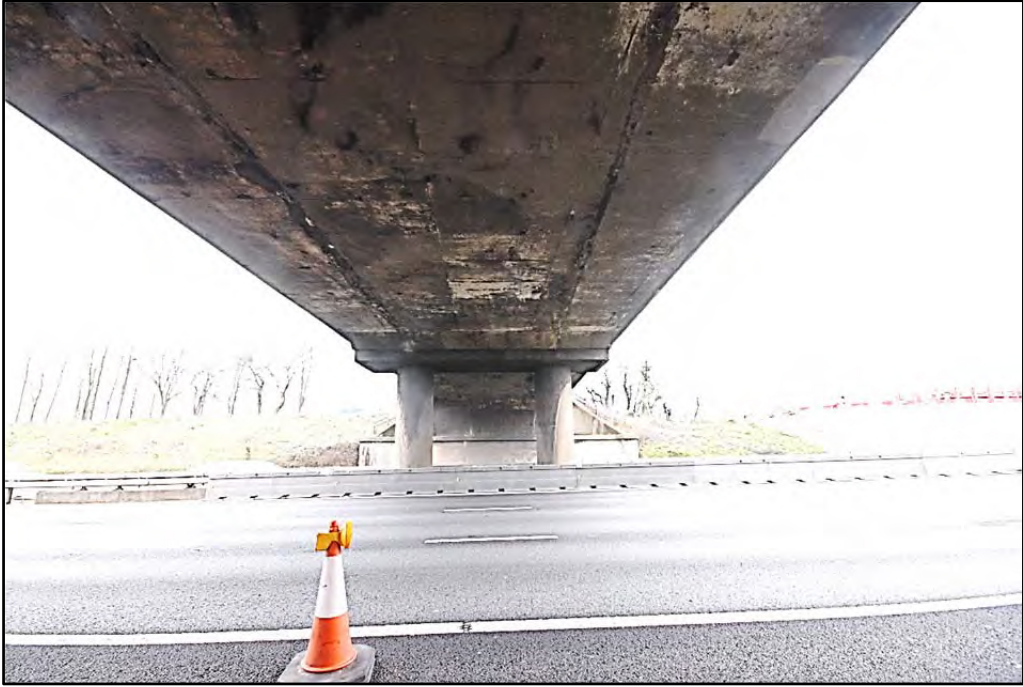
The central columns, looking north-east Fig 61
