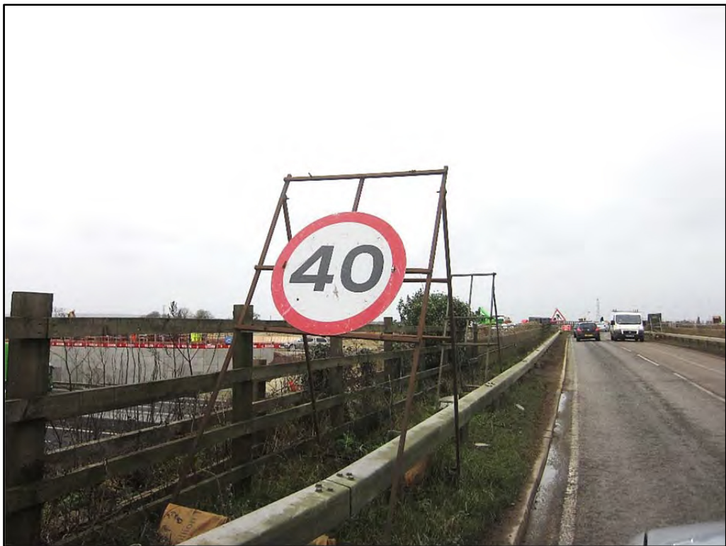
The deck of the Houghton Regis Bridge, looking west Fig 72
