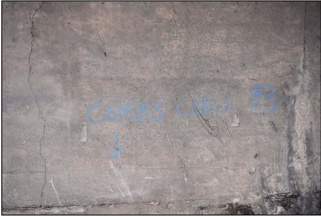
Comms cable 93 marking on southbound side Fig 55
