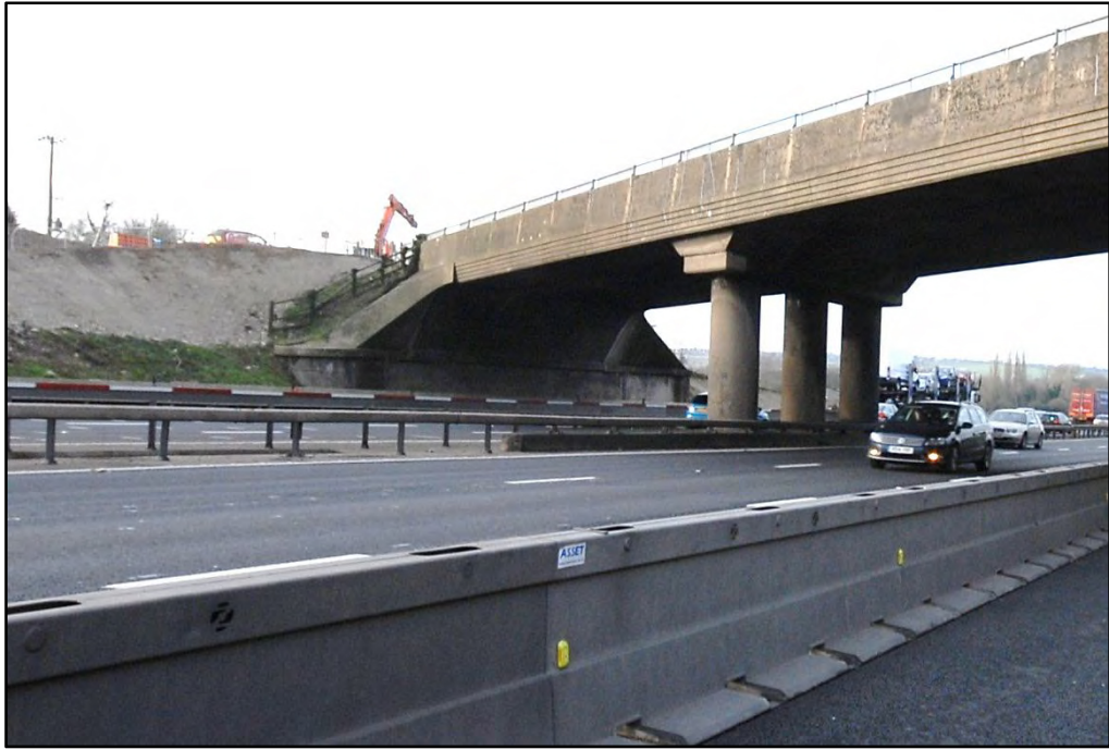
Scrolls and abutment wall with central columns, looking north-west Fig 23
