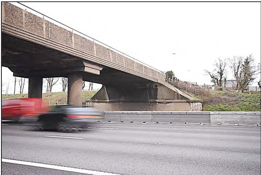
The east abutment wall with scrolls, looking north-east Fig 64
