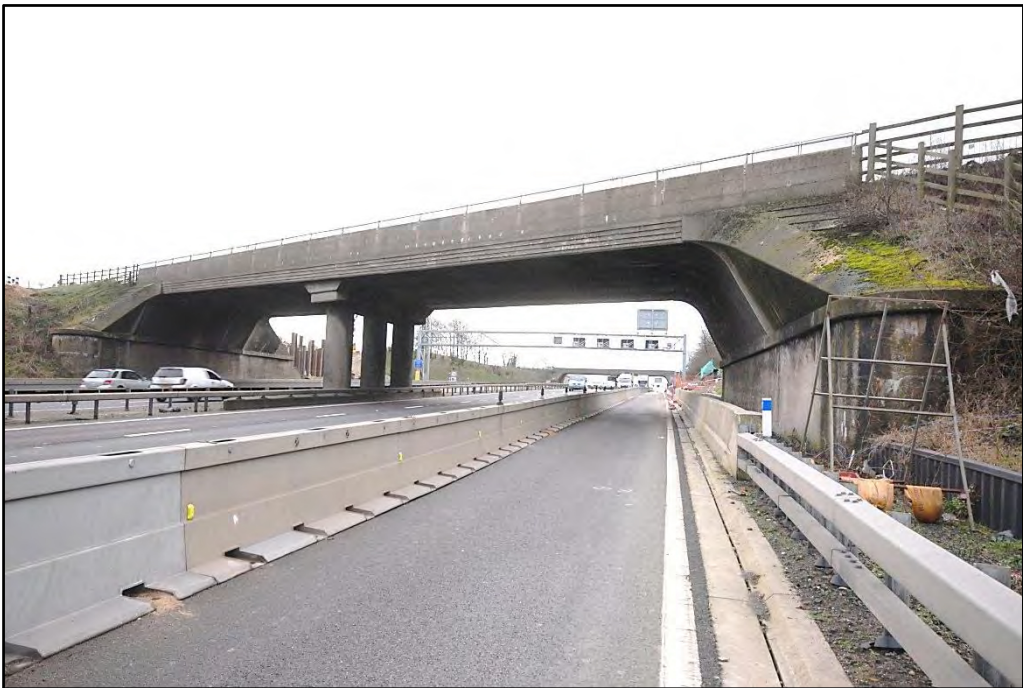
The north elevation of Chalton Bridge, looking south-east Fig 18
