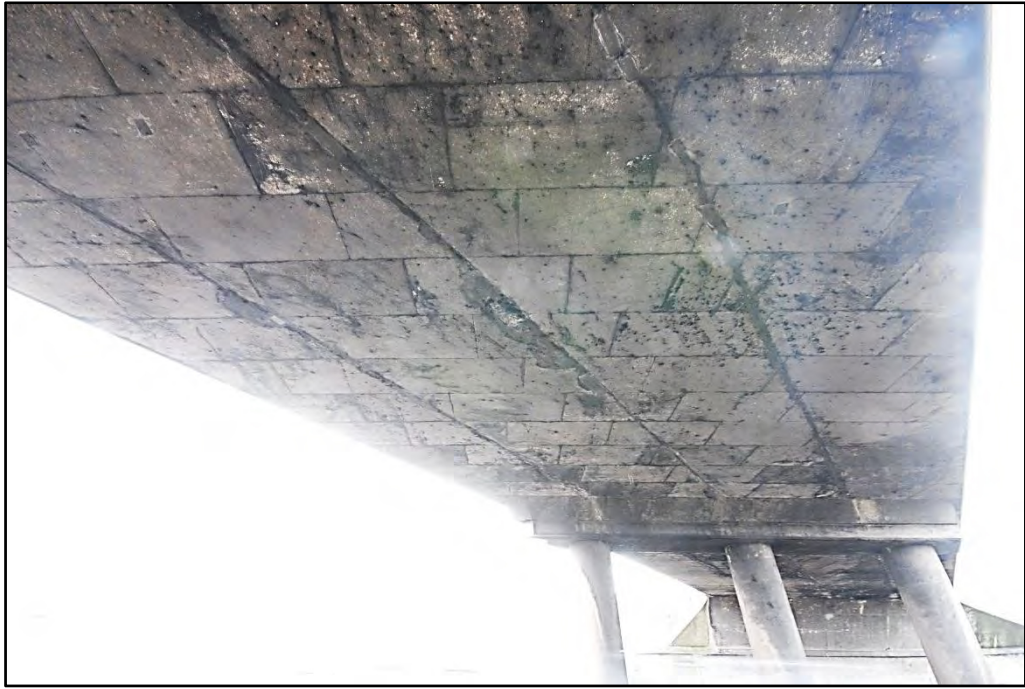
Underside of bridge with patching and columns, looking west Fig 21
