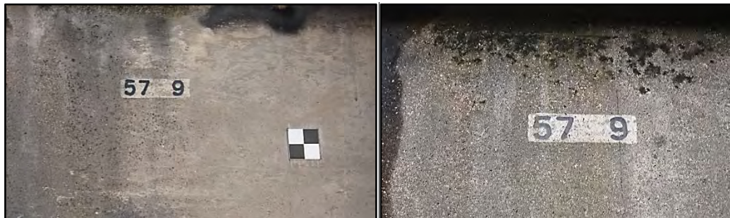
Bridge number and square southbound and number northbound Fig 56
