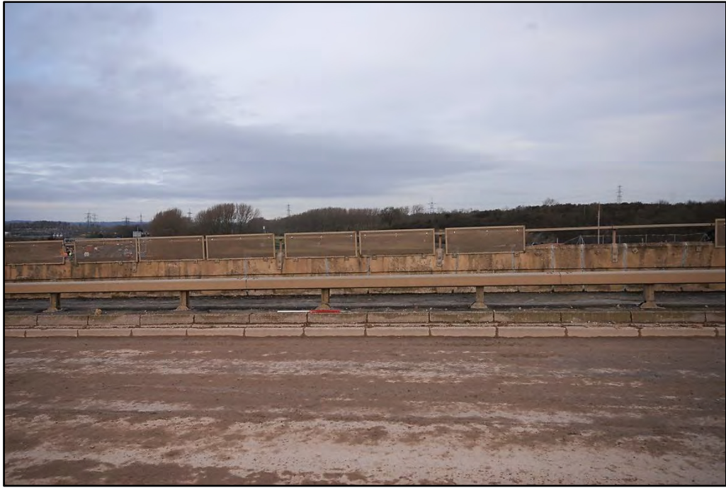
The road, pavements with barrier and north parapet, looking north-east Fig 38
