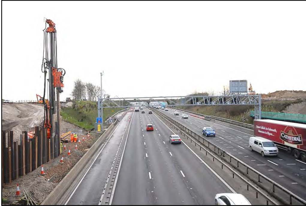
View of southern bridge from northern bridge, looking south Fig 57
