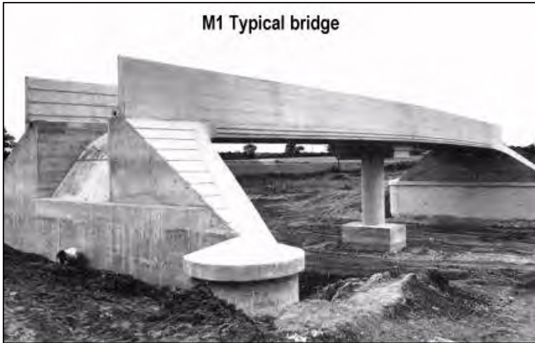
2-span bridge (The Motorway Archive) Fig 10
