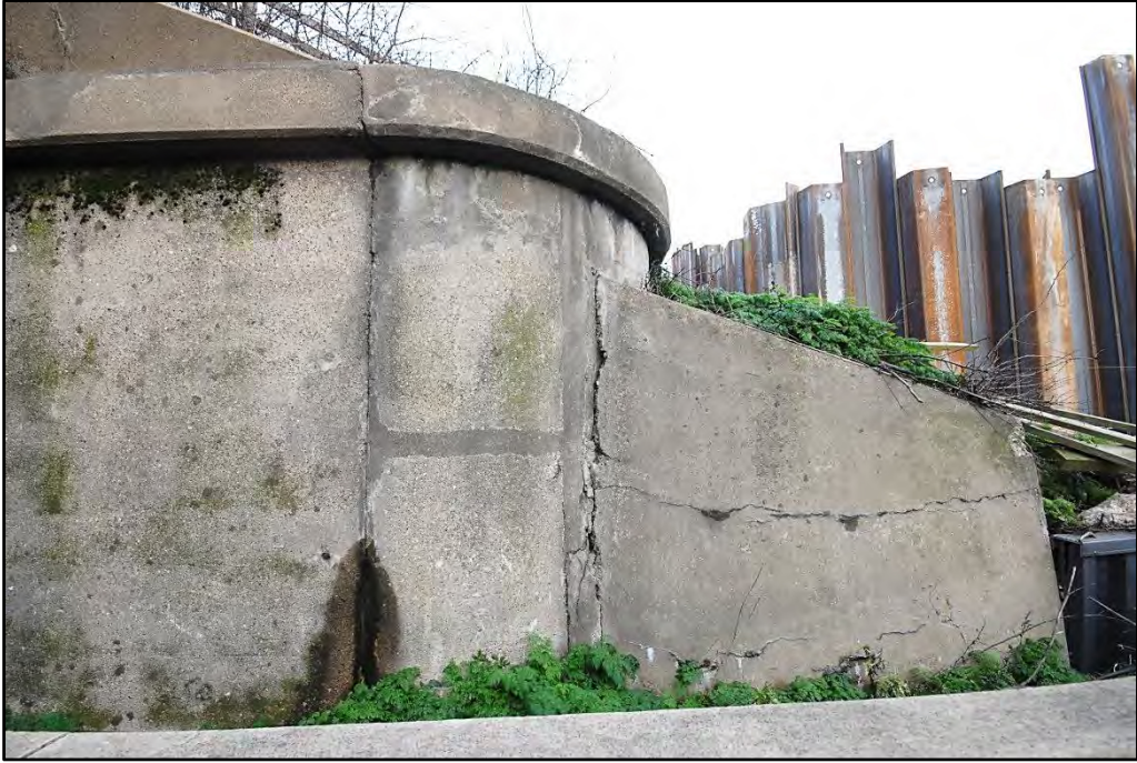
South-eastern scroll with sloping toe wall, looking east Fig 31
