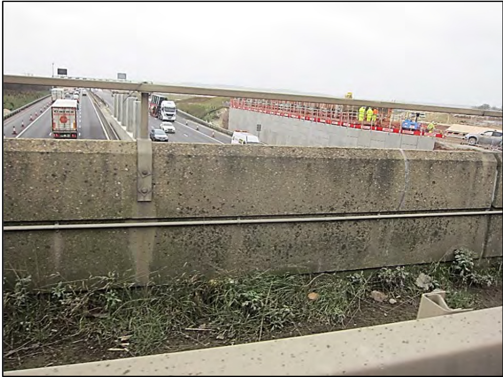
The parapet on the south side Fig 73
