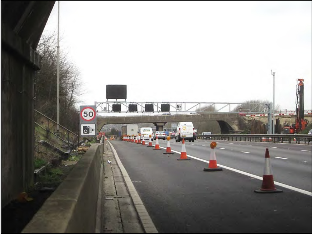
The Chalton Bridge from under the Houghton Regis Bridge, looking north-west Fig 17
