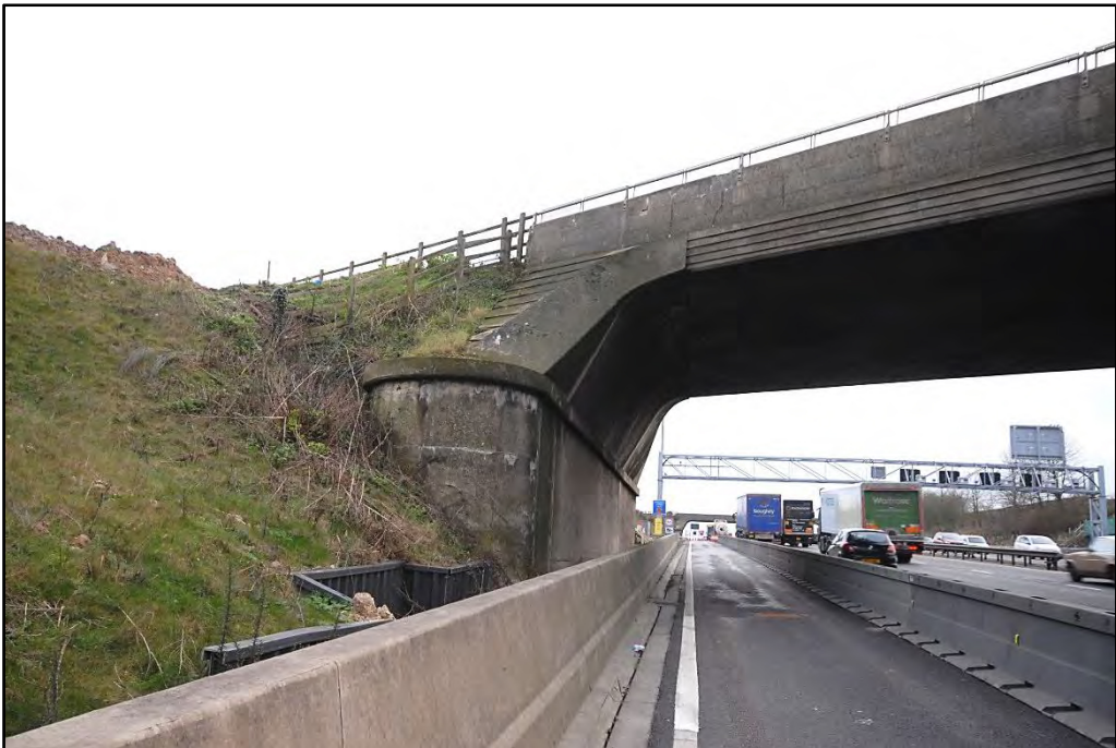
North-eastern scroll of northern bridge, looking south Fig 26
