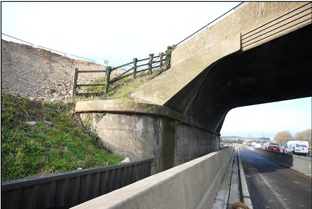
South-western scroll of northern bridge, looking north-west Fig 28
