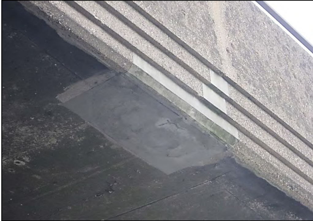
Repair on underside of deck on south elevation Fig 76
