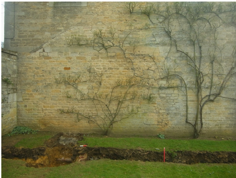
Building scar upon Deene Hall, the left scale locating wall [205] and the right scale indicates wall [206] Fig 6
