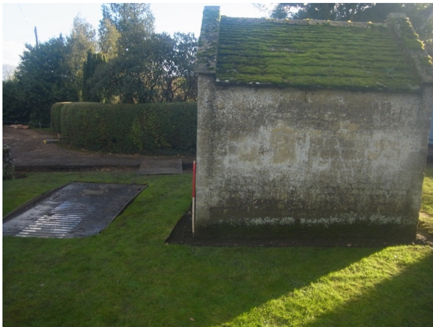
Weigh station house and platform Fig 12
