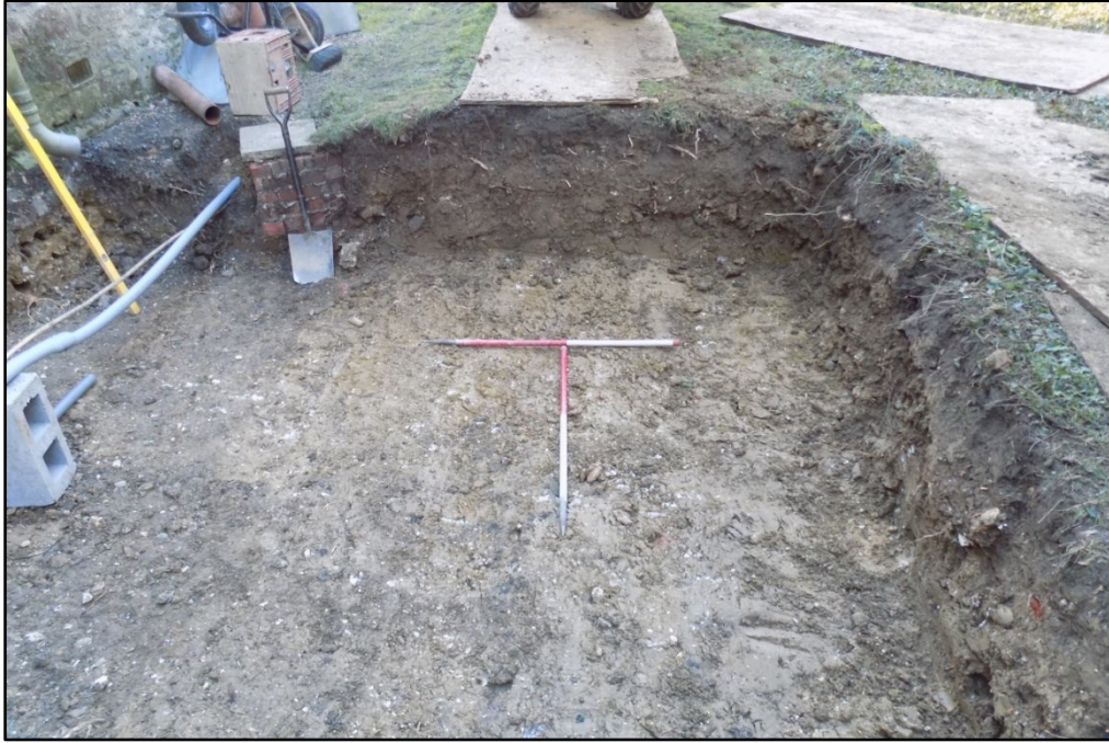
Trench 1, fully excavated, looking west Fig 21
