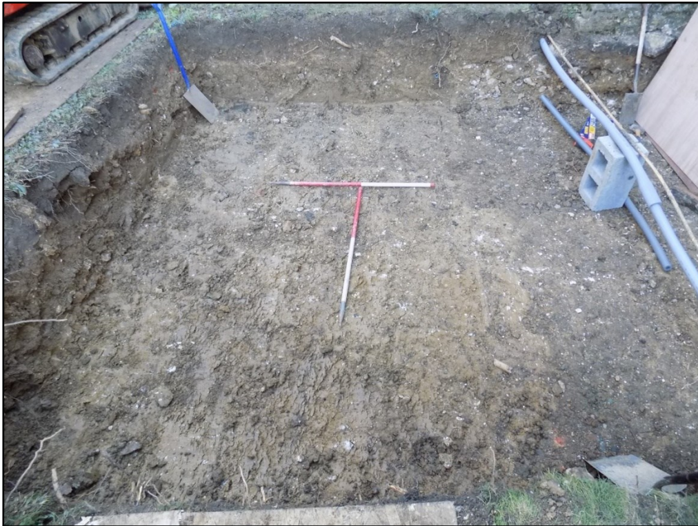
Trench 1, fully excavated, looking east Fig 22
