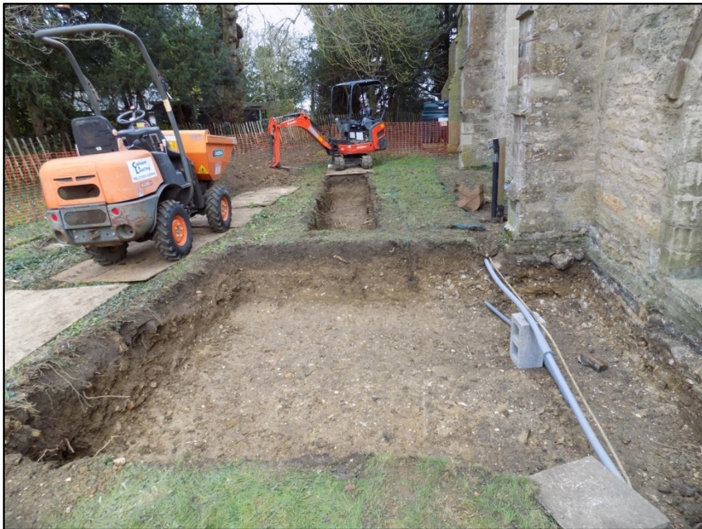
Trench 1 and Trench 2 (background), looking east Fig 24
