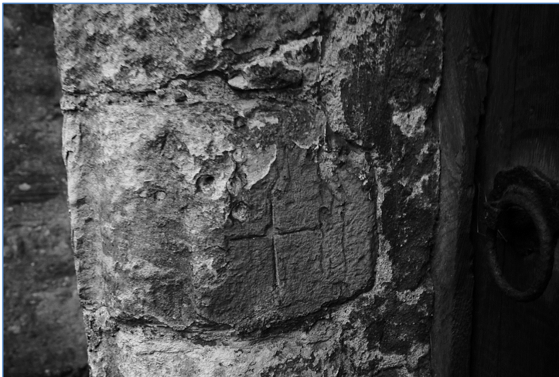
Carved + on the inside of the door jamb Fig 18
