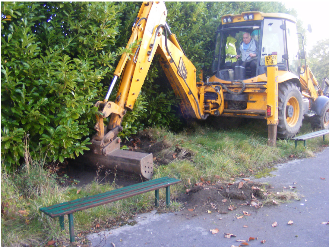
The groundworks in progress Fig 4
