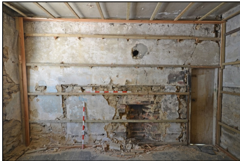
Room 3, looking east, showing brick fireplace Fig 174
