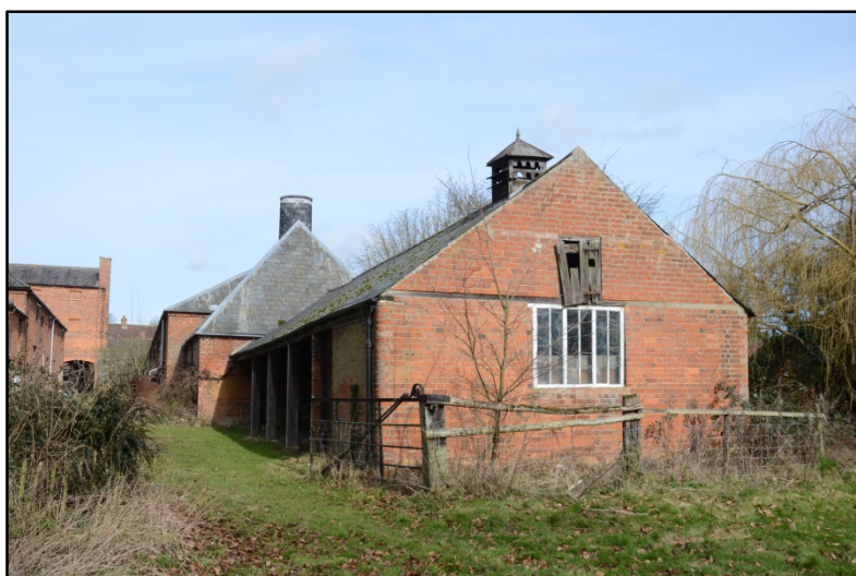
The Cart Shed and Blacksmith's Workshop, looking north-east Fig 153
