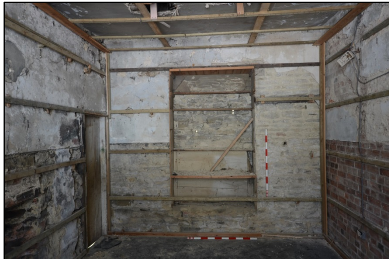
Former cupboard in the south wall of Room 3 Fig 176
