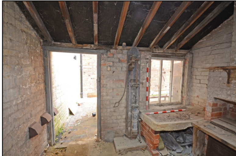
The workshop, looking north-east, showing pump and stone sink Fig 77
