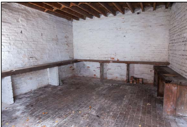
The Carriage House, looking west (©RichardPrimrose2015) Fig 94
