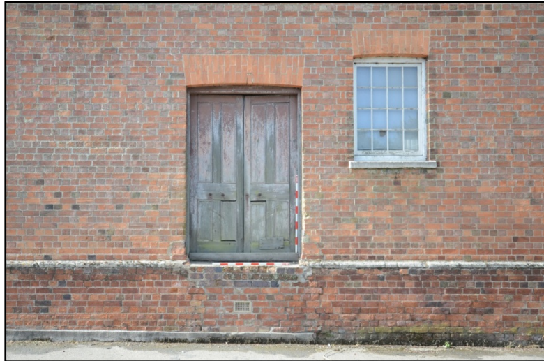
Elevated loading door to brewing floor Fig 11
