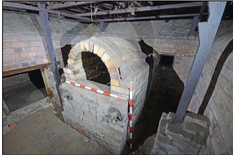
The kiln interior, looking north-west Fig 143
