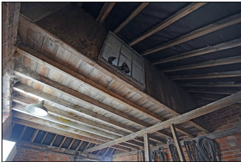
The platform over the Blacksmith's Workshop Fig 159
