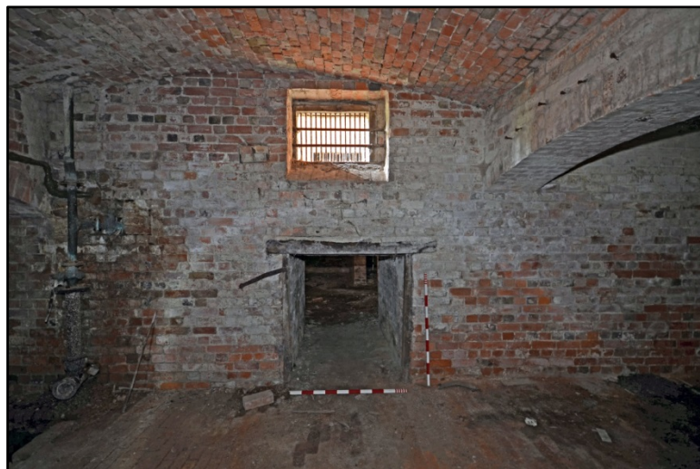
Crawl space to adjacent cellar Fig 33
