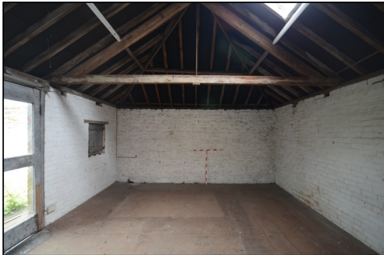
The Brewhouse, looking south Fig 66
