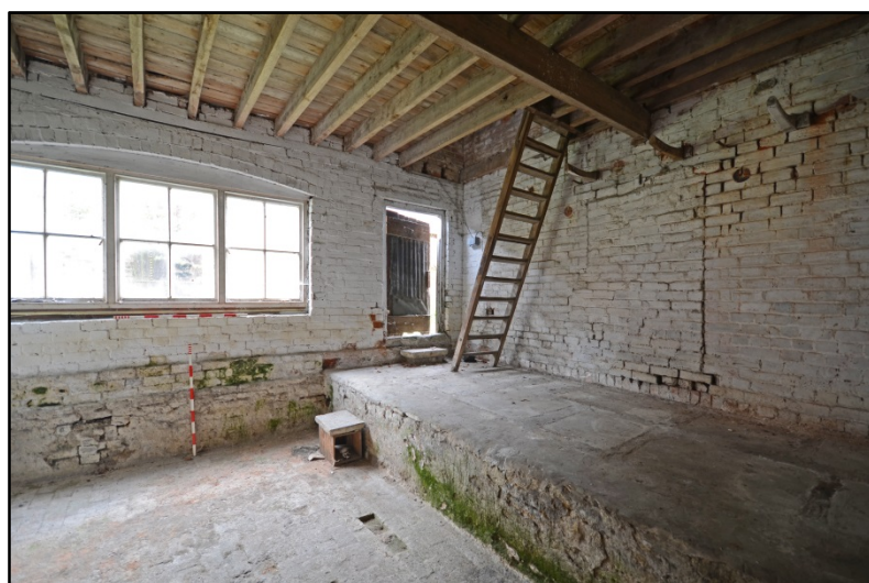
Outhouse 2, looking south-east Fig 103
