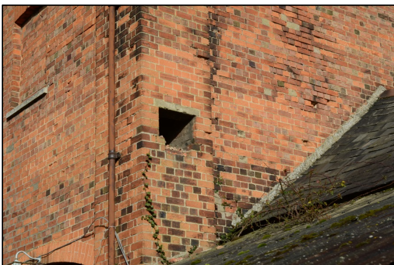
Opening to the firebox, with scar of tank to the right Fig 16
