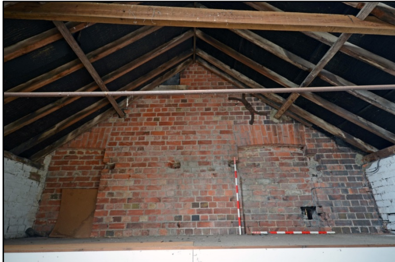
Blocked windows above the covered passage Fig 65
