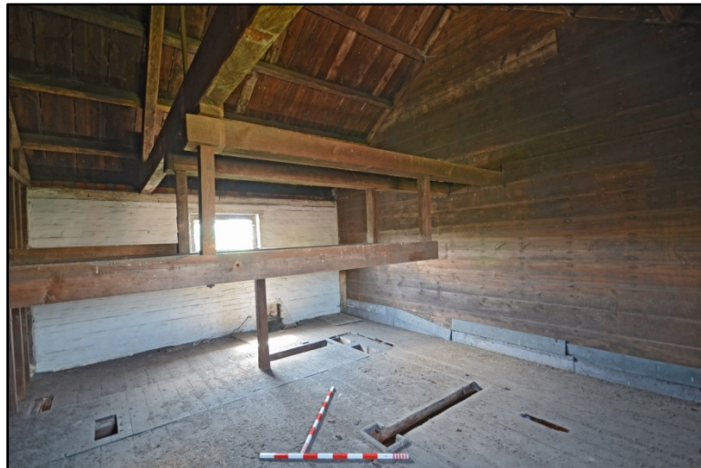
Room S1, looking south-west Fig 52
