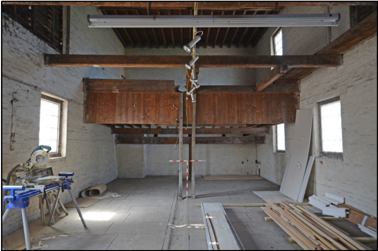
Brewery, ground floor, looking west Fig 23
