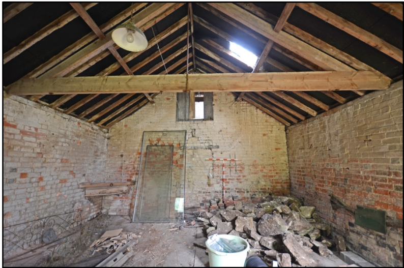
Stable 4, looking north Fig 114
