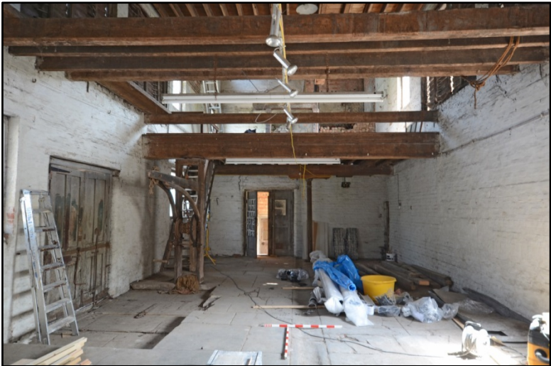
The ground floor, looking east Fig 24
