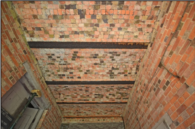
Carriage arch roof, showing supports for the firebox Fig 20
