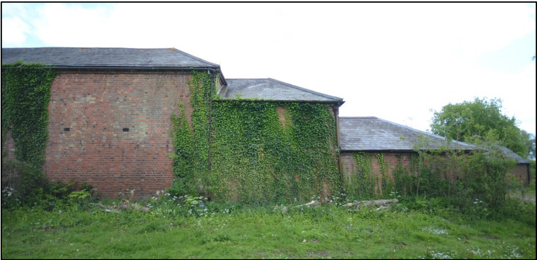
The southern extent of the west elevation of the Stables Fig 90
