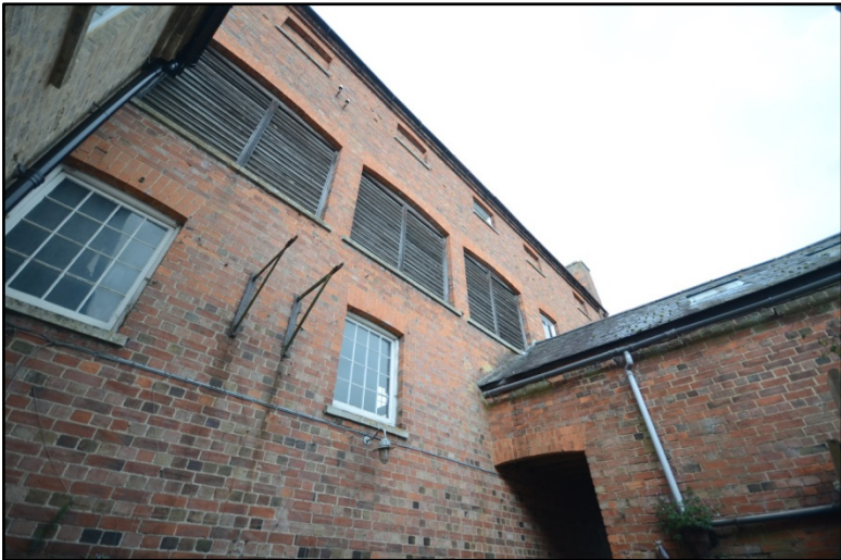
The south elevation viewed from the rear courtyard Fig 18
