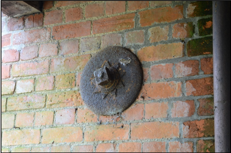
Detail of tie plate Fig 150
