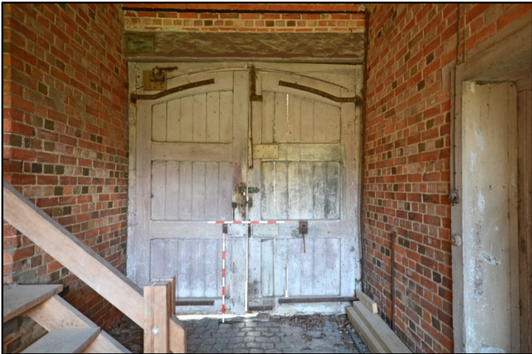
Interior face of carriage arch door Fig 21
