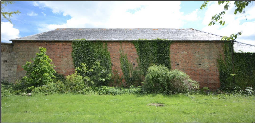
The west elevation of the Stables Fig 91
