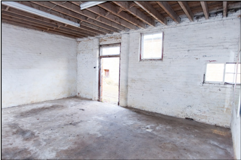
Stable 2, looking north-east Fig 98
