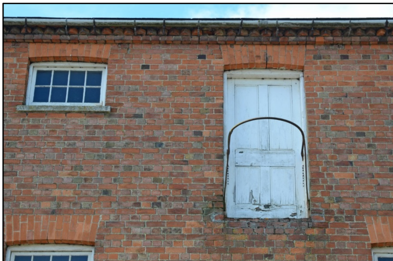
The second floor loading door Fig 14
