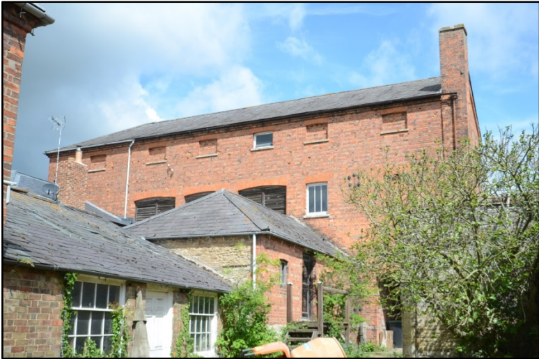
The south elevation of the Brewery Fig 17
