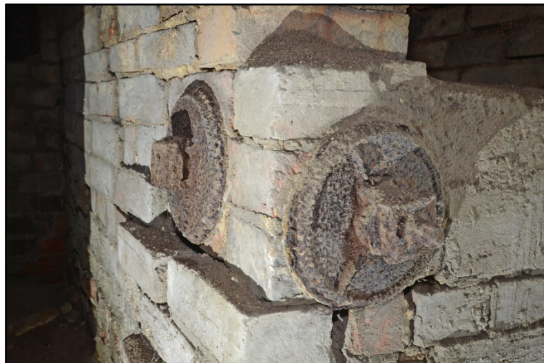
Detail of tie plates Fig 145
