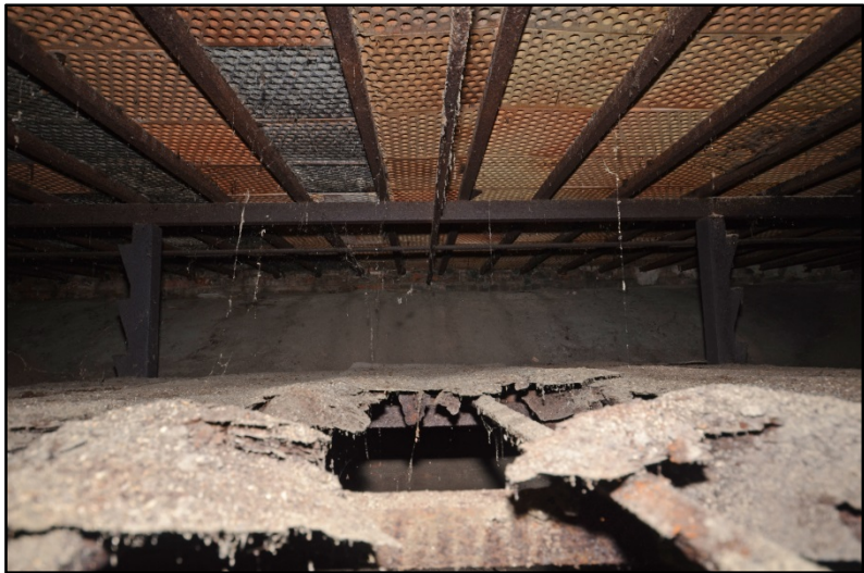
The underside of the drying floor Fig 147
