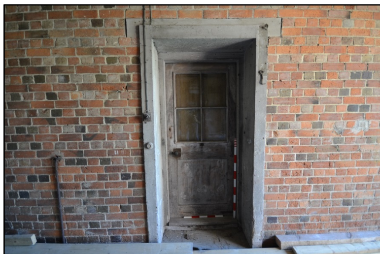
External view of the west wall of Room 3 Fig 178
