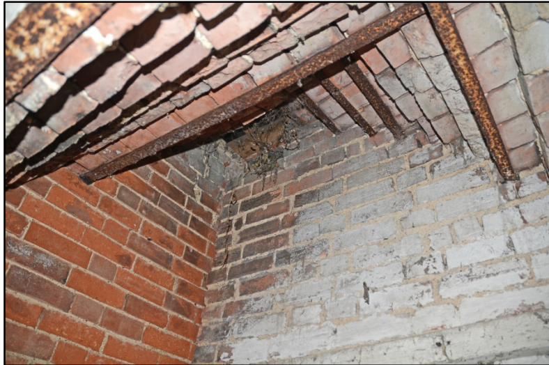
Interior view of the forge chimney Fig 158
