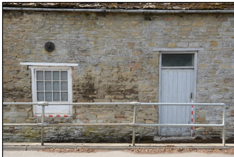
Detail of fenestration with tie plate Fig 162
