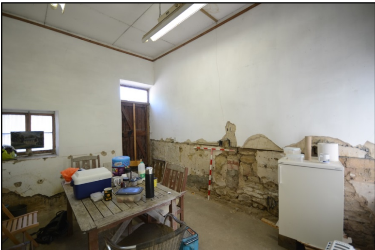
Room 2, looking north-east Fig 172
