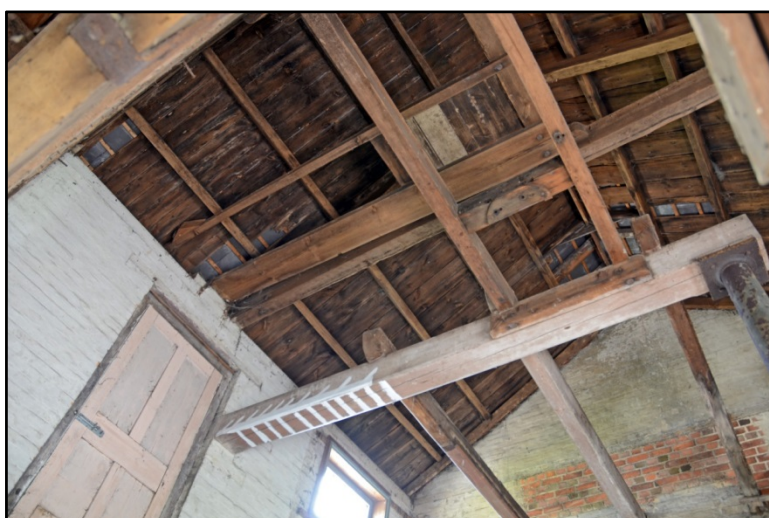
Remnant supporting timbers for overhead brewing equipment and walkways Fig 48
