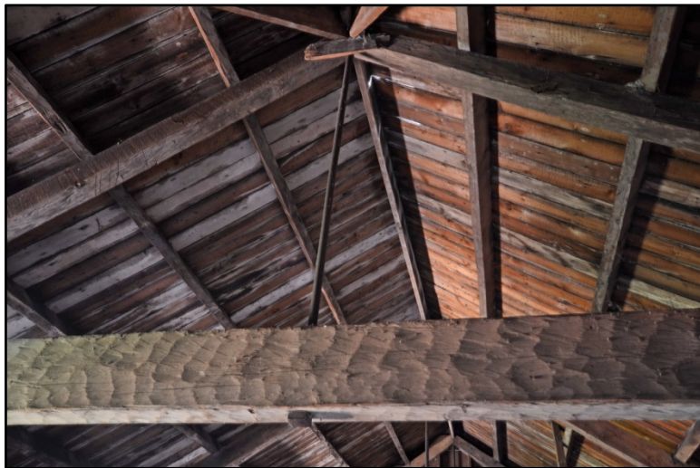
Detail of adze marks on the western tie beam Fig 59
