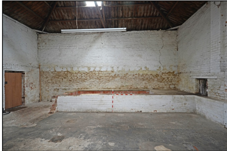
The steep cistern, looking north Fig 126
