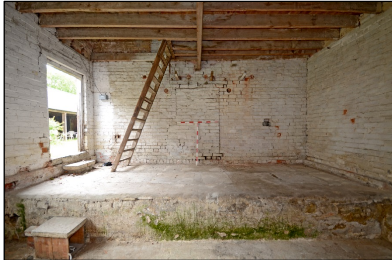
Outhouse 2, looking south, showing blocked door Fig 104
