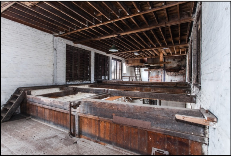
The first floor, looking north-east (©RichardPrimrose2015) Fig 36
