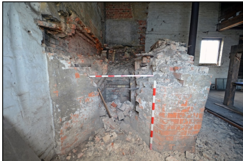
The firebox, looking south Fig 42
