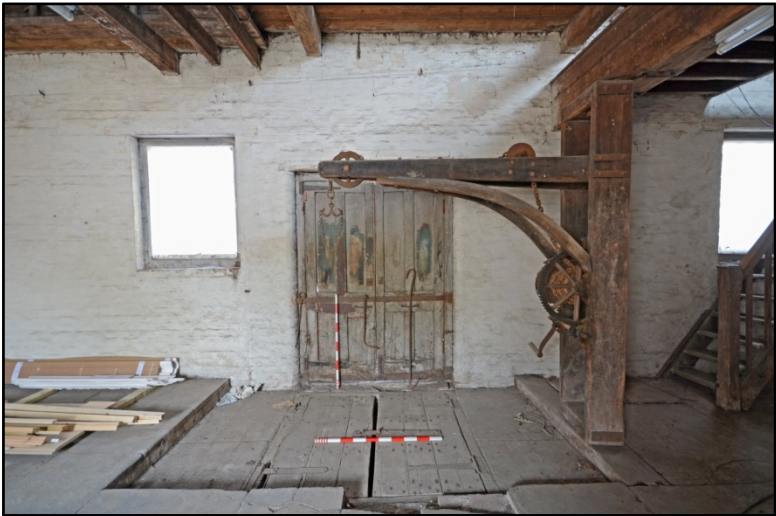
The ground floor loading bay with adjacent hoist Fig 25
