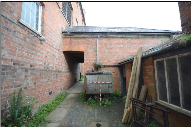
The west elevation of the Brewhouse, looking east Fig 70
