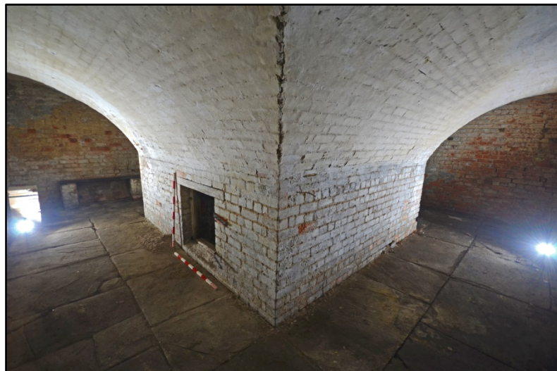
The kiln with hatch to interior, looking north-west Fig 142
