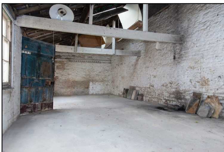
The Tack Room, looking south (©RichardPrimrose2015) Fig 81
