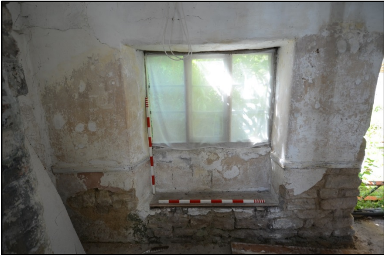
The south facing window of Room 1 Fig 170
