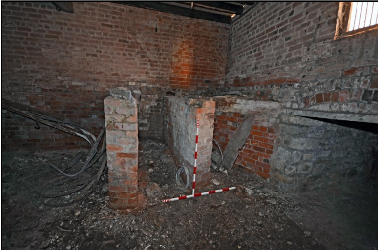
The Brewhouse cellar, looking west Fig 69
