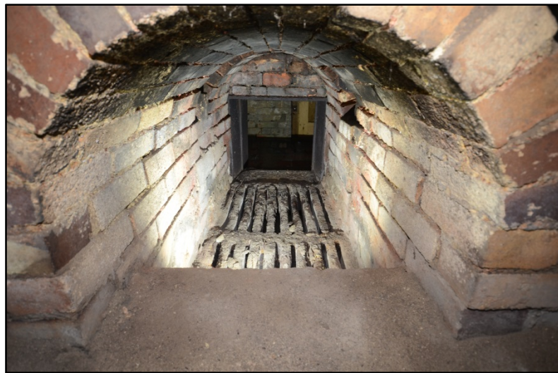
Detail of fire bars within the kiln Fig 144
