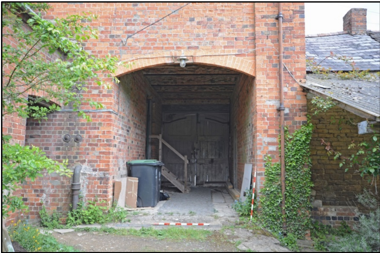
The carriage arch, looking north Fig 19
