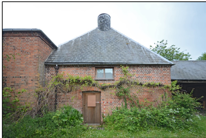
The west elevation of the Oast House Fig 122
