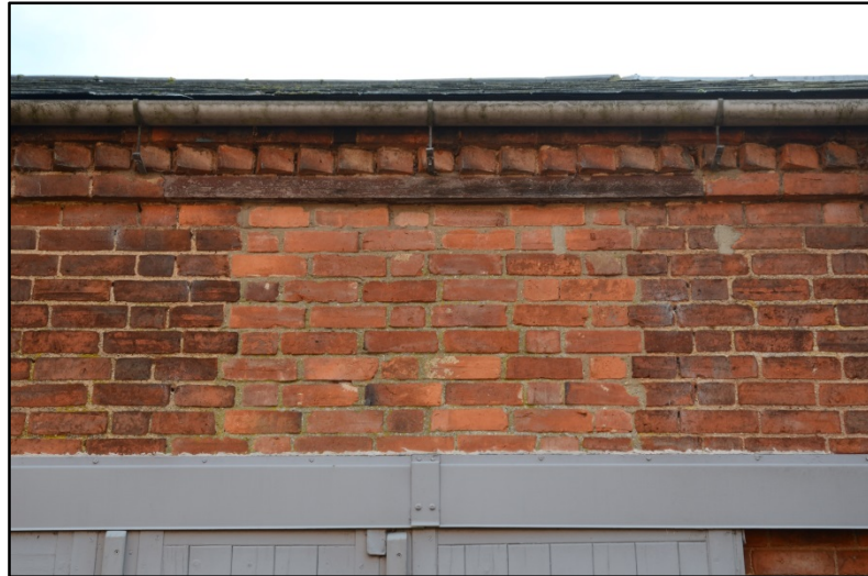
The Maltings, blocking over the double doors Fig 120
