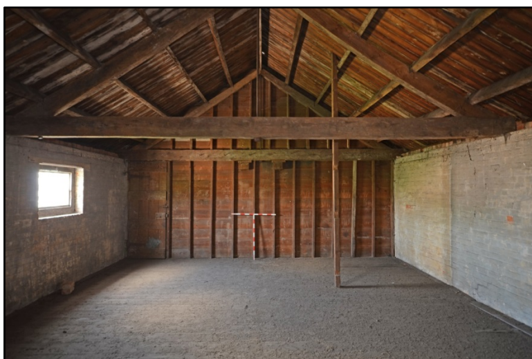
Room S2, looking east Fig 56
