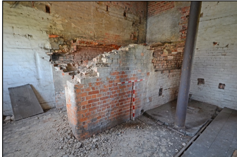
The firebox, looking south-east Fig 41
