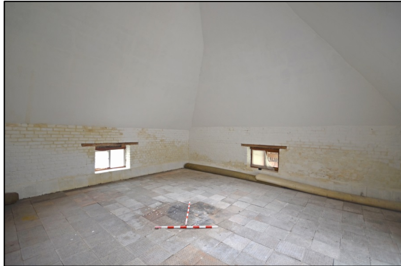
The kiln tile drying floor, looking south-east Fig 137
