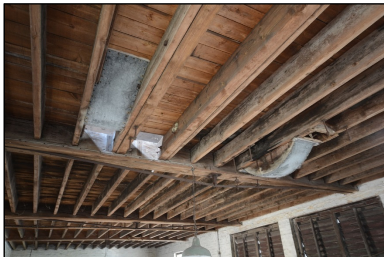
Wheel guards below Room S1, looking north-west Fig 53
