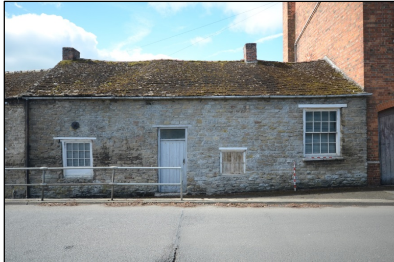
The north elevation of the Cottage Fig 161
