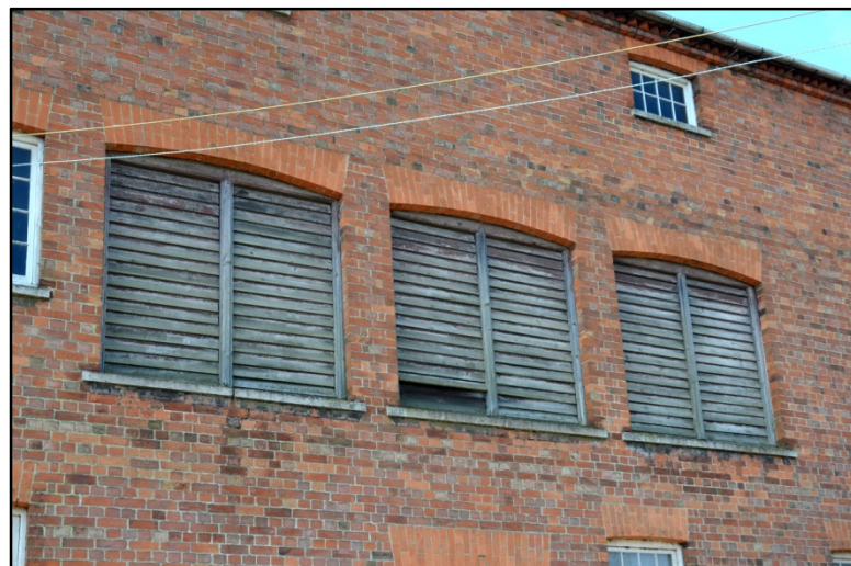
The first floor louvered windows Fig 13
