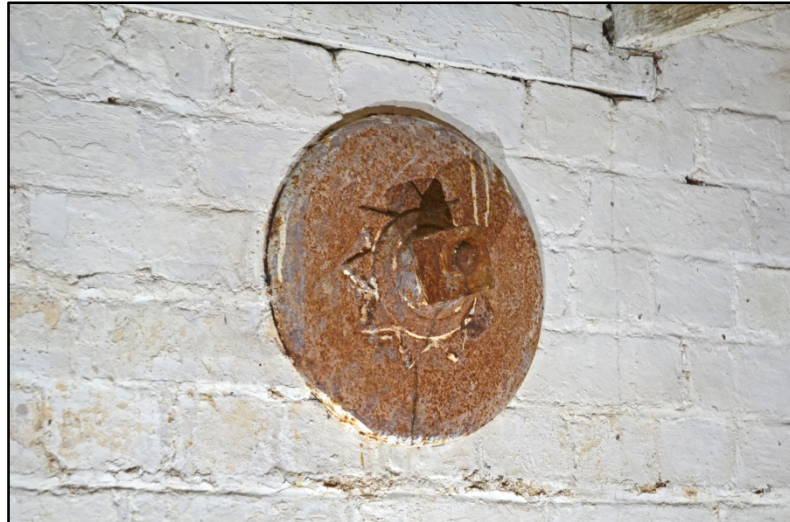
Detail of tie plate Fig 132
