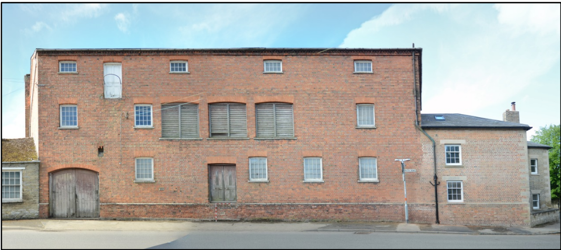
North elevation of the Brewery (photo-composite) Fig 10
