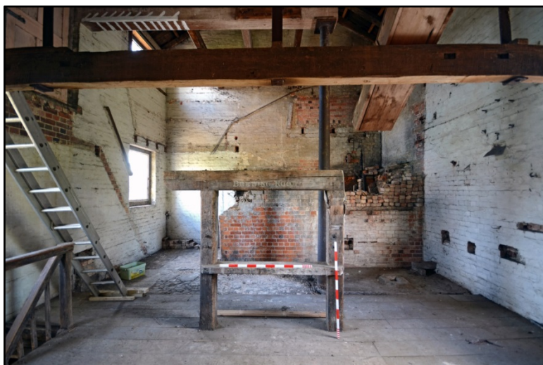
The first floor, looking east Fig 39
