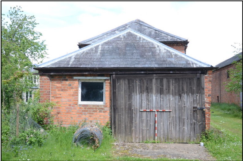
Stable 4, looking north Fig 89
