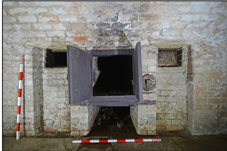
The west elevation of the kiln, with doors to furnace Fig 140
