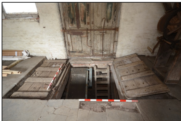
The cellar access Fig 28
