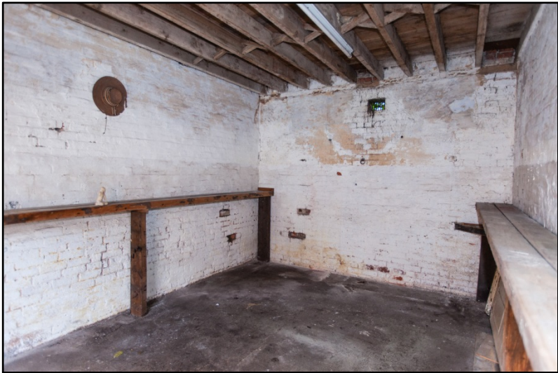
Stable 1, looking west Fig 97
