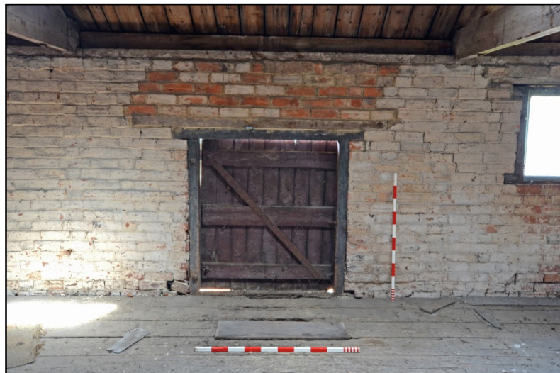
Access hatch with modified brickwork over Fig 111
