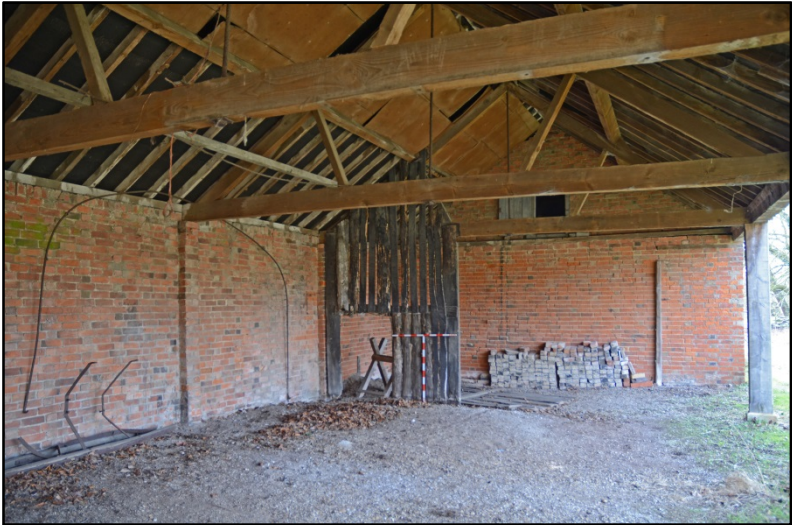
The Cart Shed, looking south-east Fig 151
