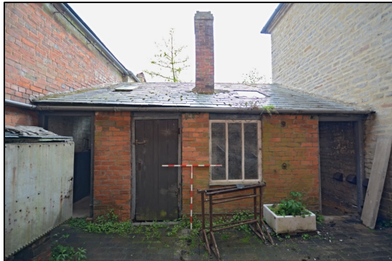
The north elevation of the Outbuilding Fig 72
