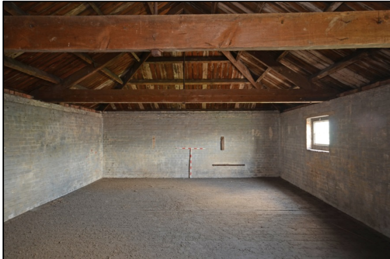
Room S2, looking west Fig 58
