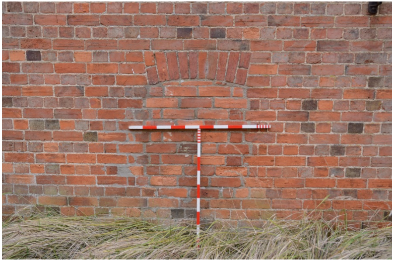
The Maltings, blocked window Fig 118
