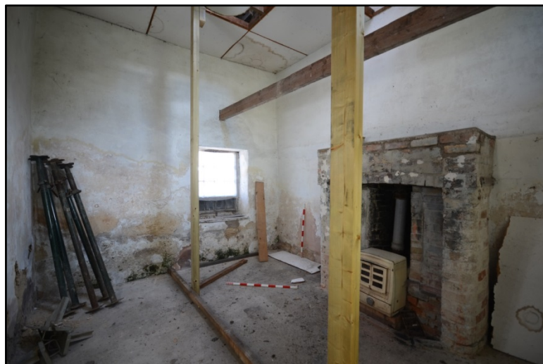
Room 1, looking north-east Fig 168
