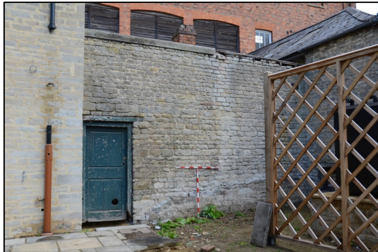
The south elevation of the Outbuilding Fig 78
