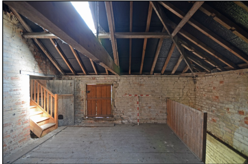
Outhouse 2 loft, looking east Fig 107
