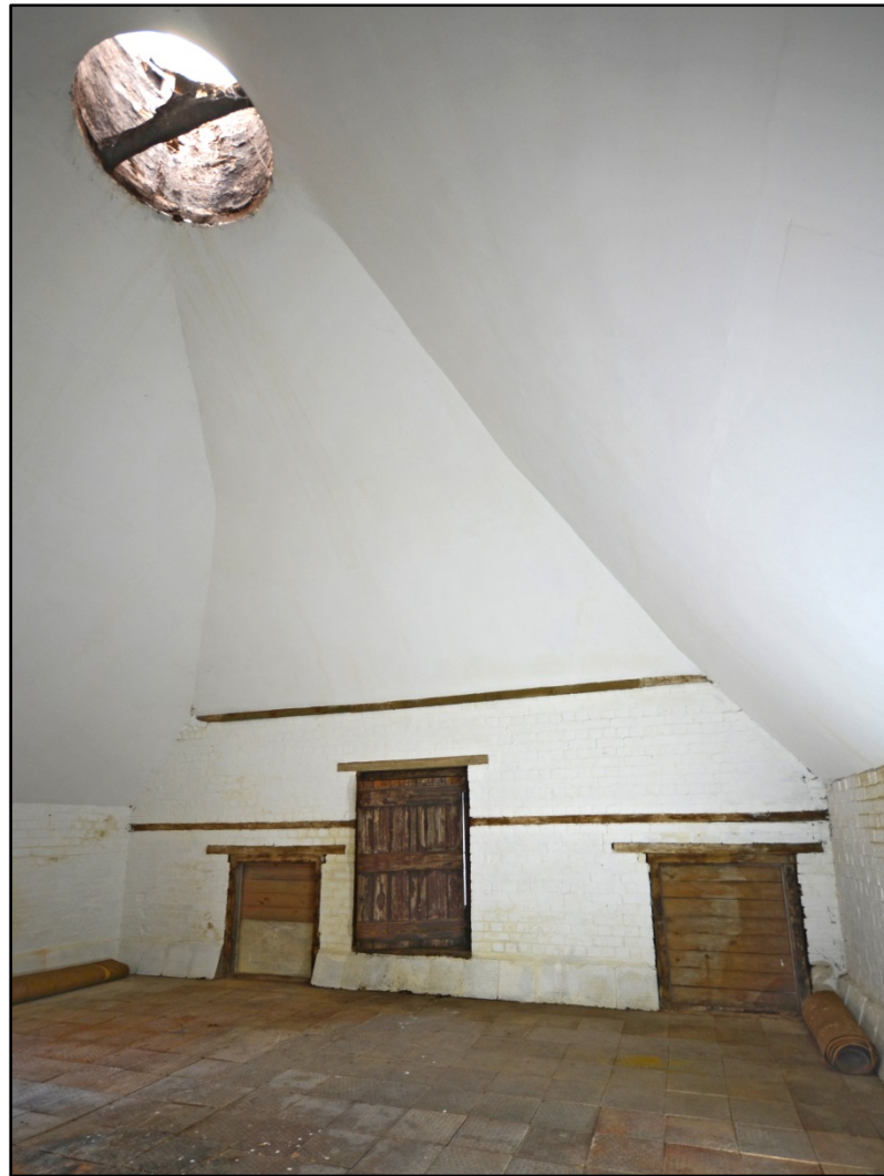
The oast house drying floor, looking north-west Fig 135
