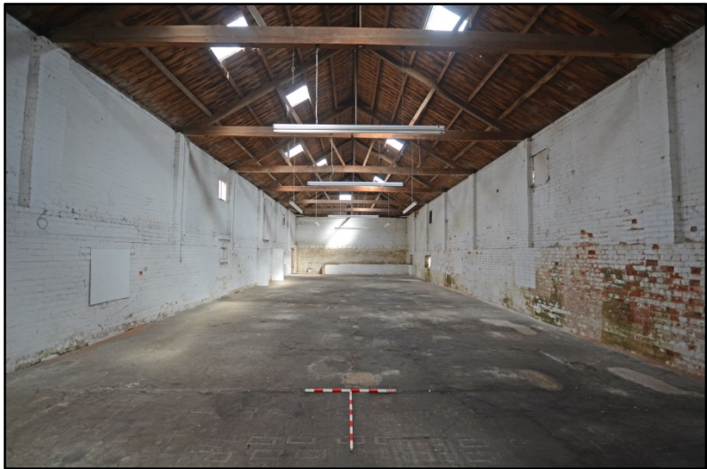
Interior of the Maltings, looking north Fig 125
