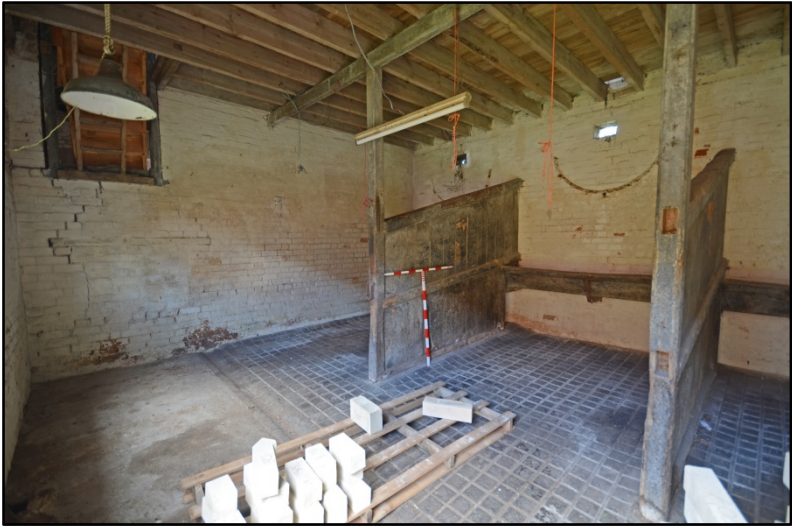
Stable 3, looking south-west Fig 100
