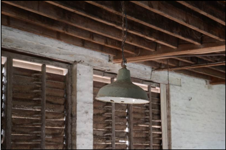
Example of c1930s vitreous enamelled steel factory shades Fig 49
