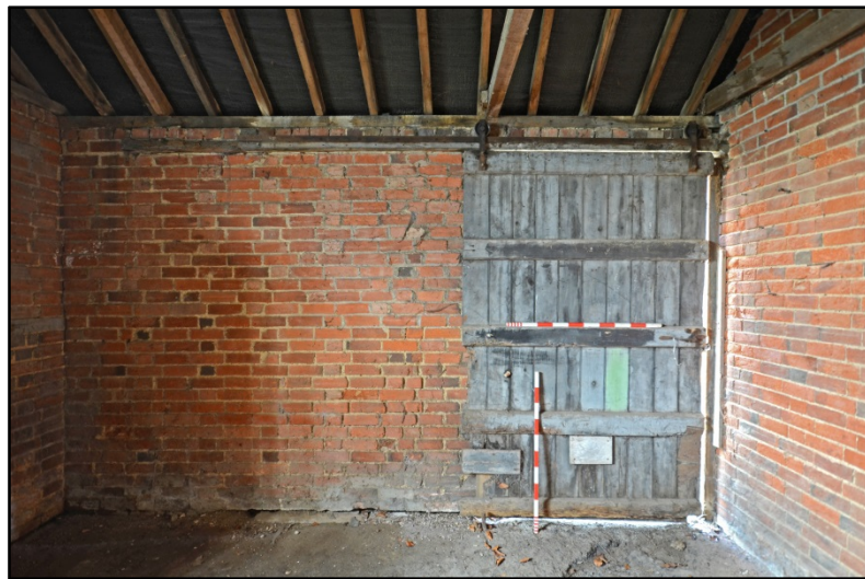
The sliding door of the Blacksmith's Workshop Fig 156
