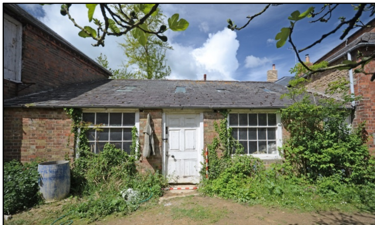
The Tack Room, looking west Fig 79
