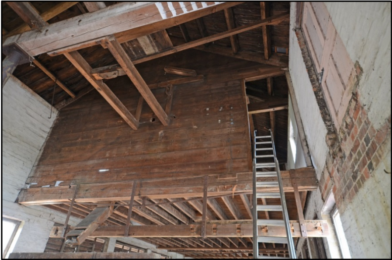
The second floor rooms, looking west Fig 50
