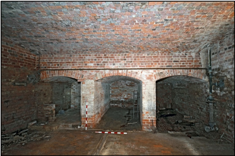
The cellar, looking east Fig 31
