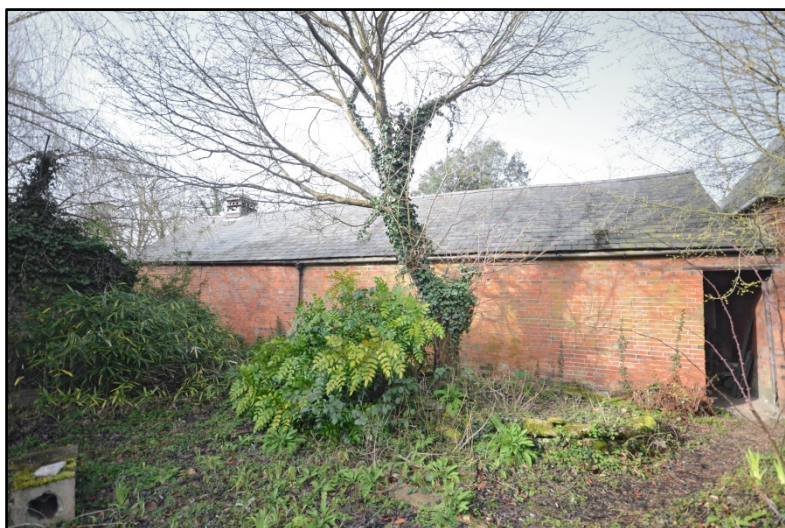
The east elevation of the Cart Shed, looking west Fig 154
