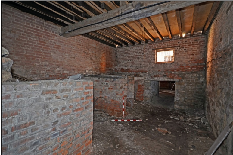
The Brewhouse cellar, looking north-west Fig 68
