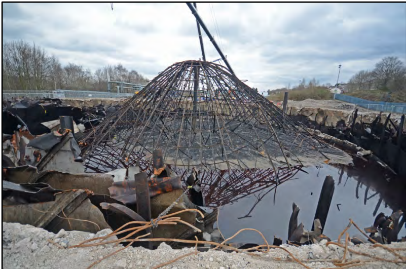
The crown-frame following disconnection from the inner lift Fig 83
