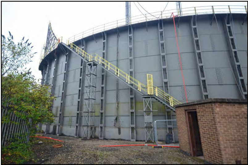
The base-tank stair, looking north Fig 26
