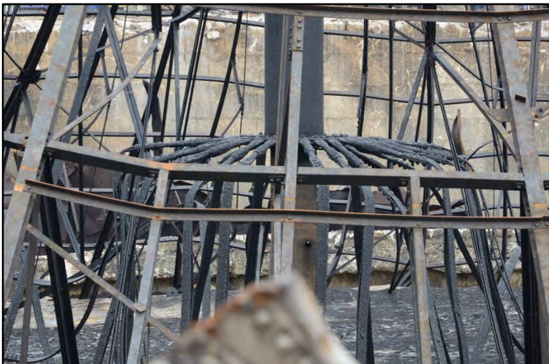
The lower portion of the crown-frame post, with radial straps Fig 85
