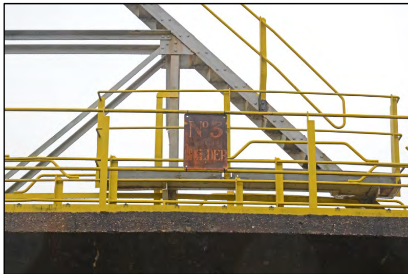
Gasholder designation sign on handrail adjacent to base-tank stair Fig 66
