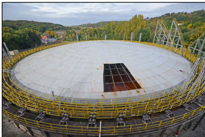
View of the gasholder crown, looking north Fig 67
