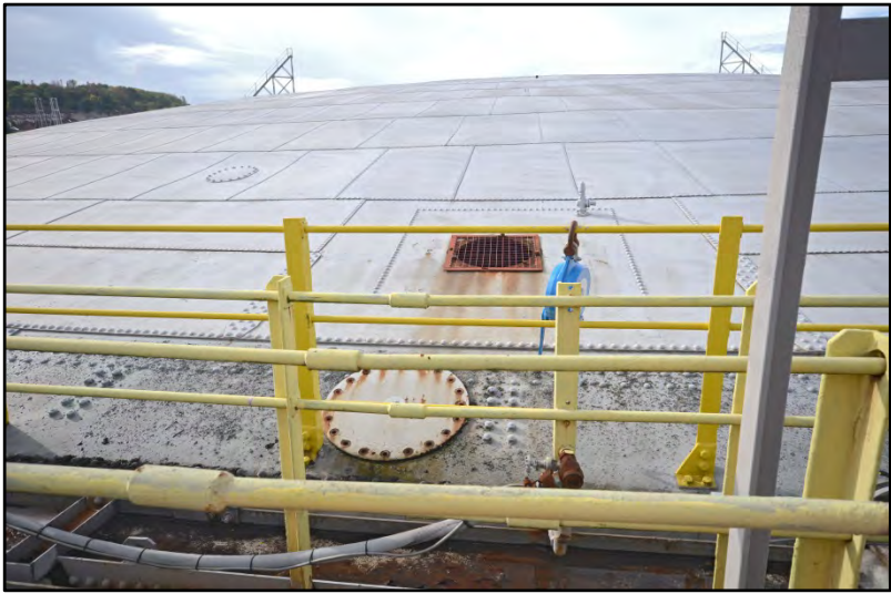
The crown, showing manhole access points Fig 40
