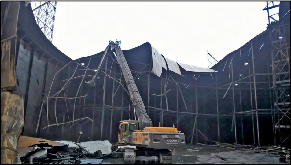
Dismantling of the crown-rest and crown Fig 48
