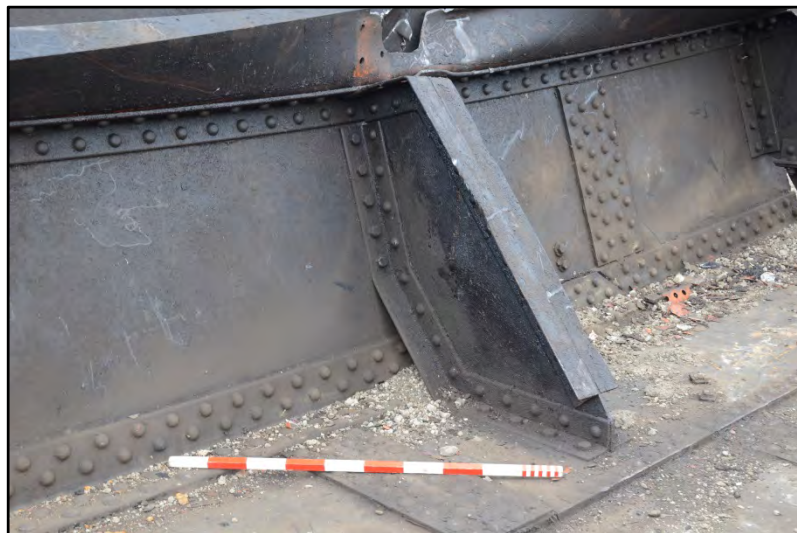
Secondary bracing of the top-curb Fig 90
