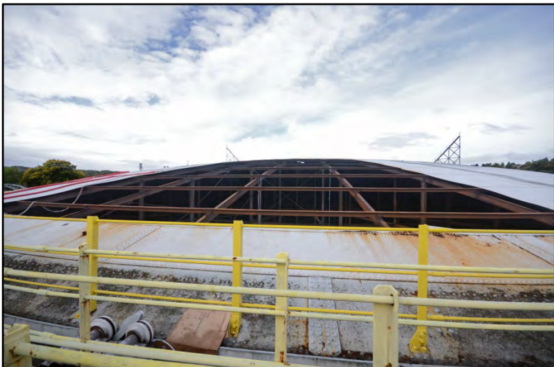
The removal of crown sheets to expose the underlying crown-rest Fig 43
