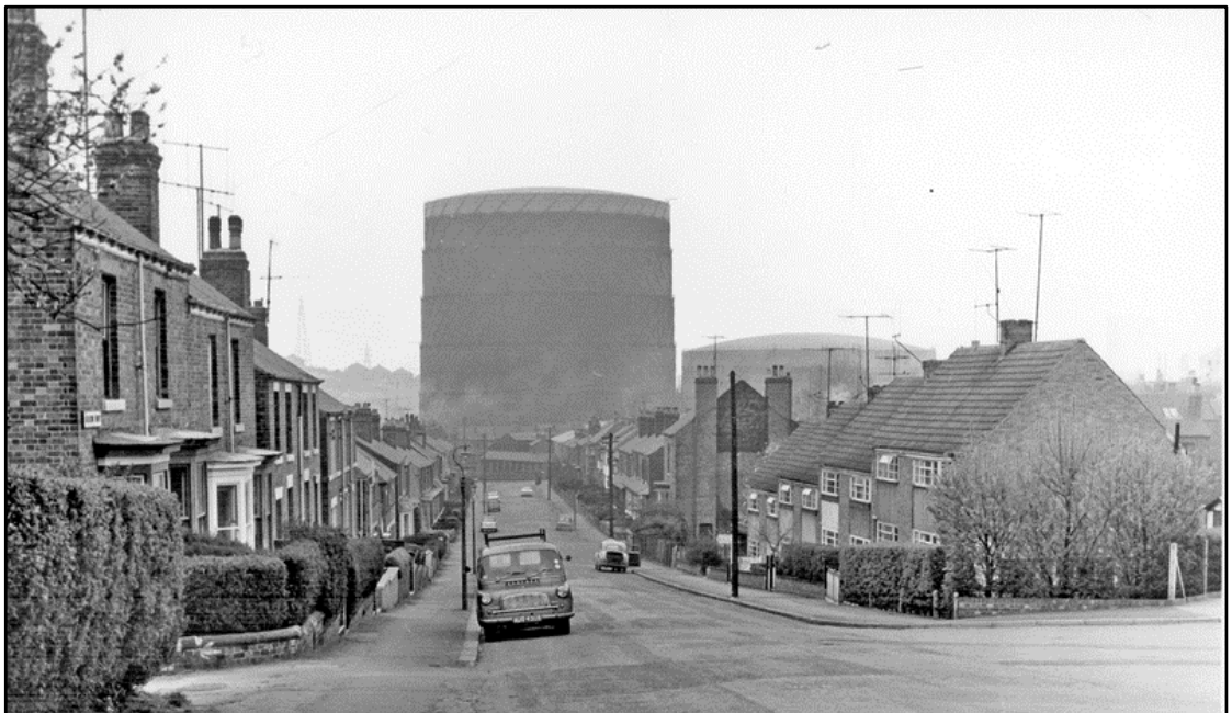
View of the gasholders from the west, showing the scale of the structures in the local skyline (s19682) Fig 10
