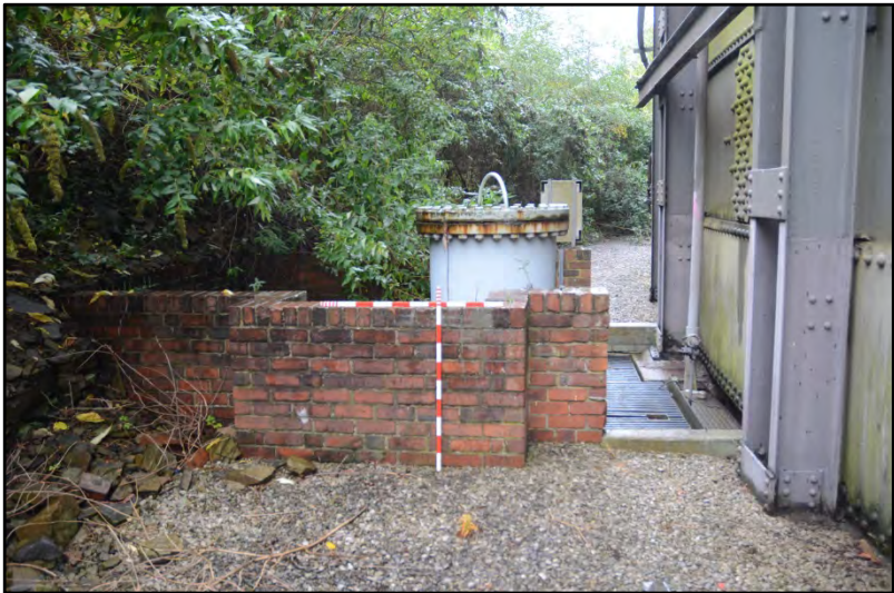
Sump, looking north Fig 24
