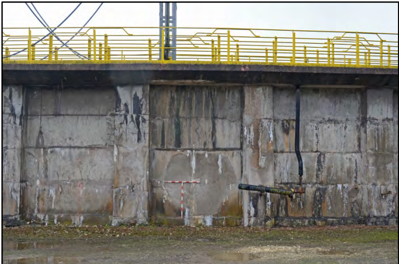
Detail of large repair on north side of the tank Fig 62
