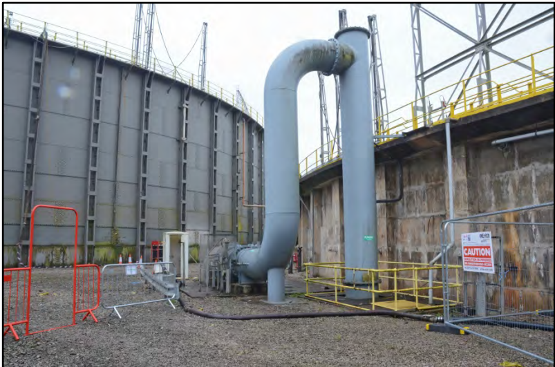
The inlet / outlet pipes and pipe pit, looking south-west Fig 55
