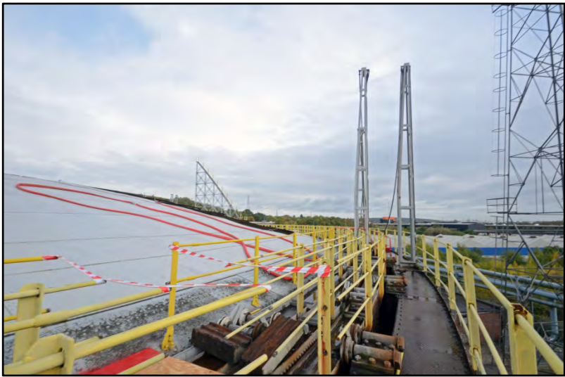
The walkways, hand rails, and anti-freeze pipe supports, looking east Fig 34
