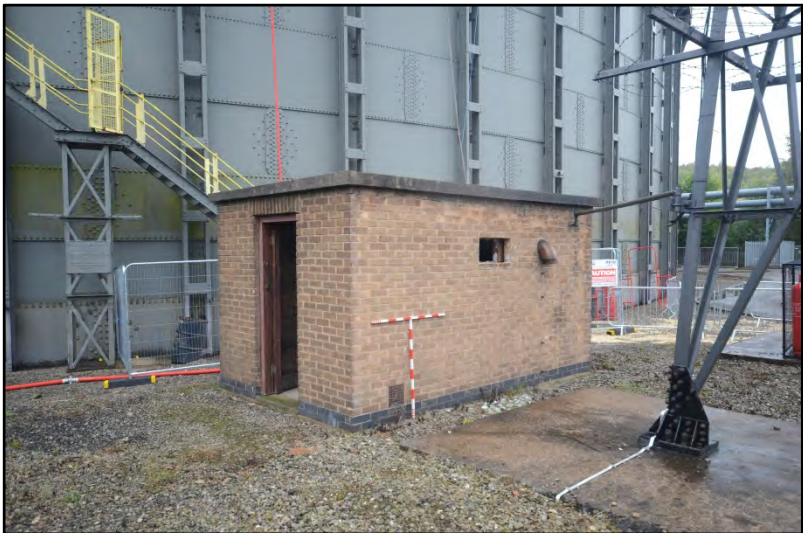
Defunct brick structure adjacent to former transmitter mast Fig 25
