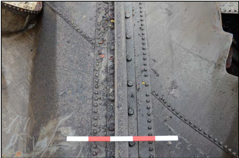
Detail of the lift-tank guide rails Fig 92
