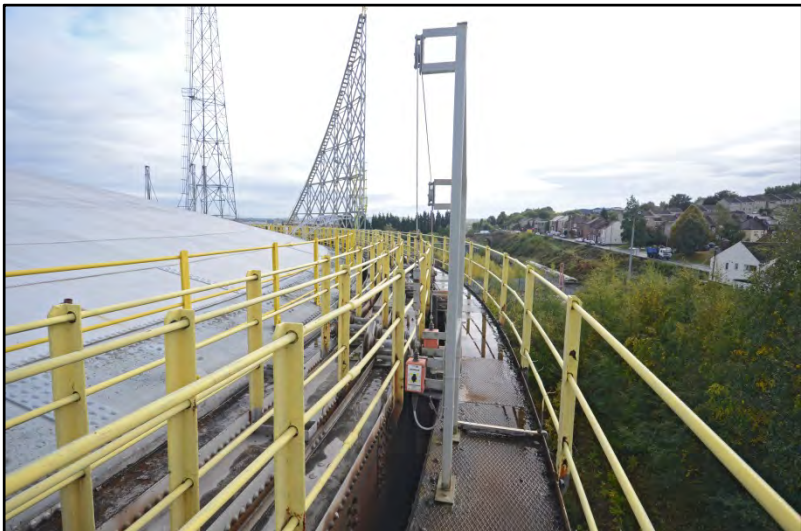
Operational equipment Fig 42
