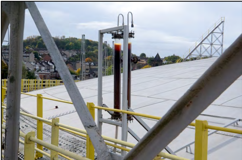
Inspection equipment Fig 41
