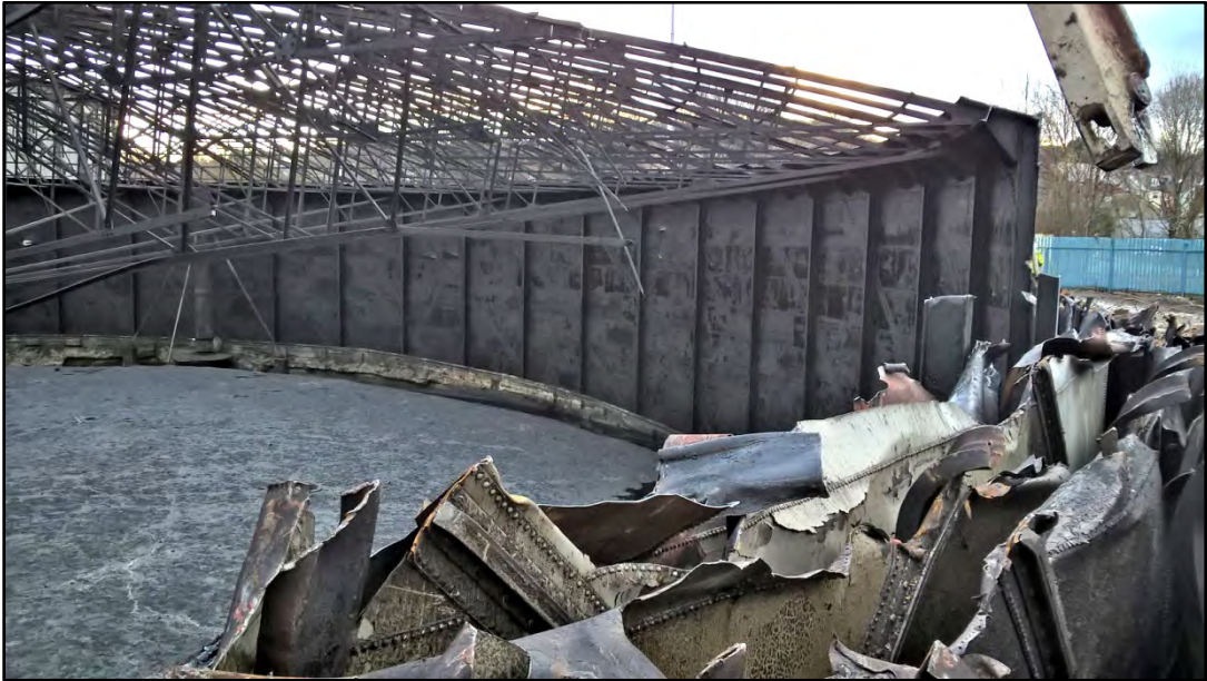
Dismantling of the lift-tanks and revealing the crown-frame Fig 80
