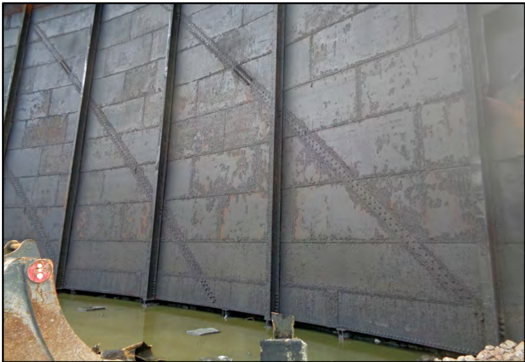
The inner face of the lift-tanks, showing vertical stiffeners Fig 49
