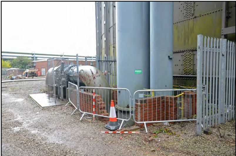
Pipe pit with inlet / outlet pipes Fig 18
