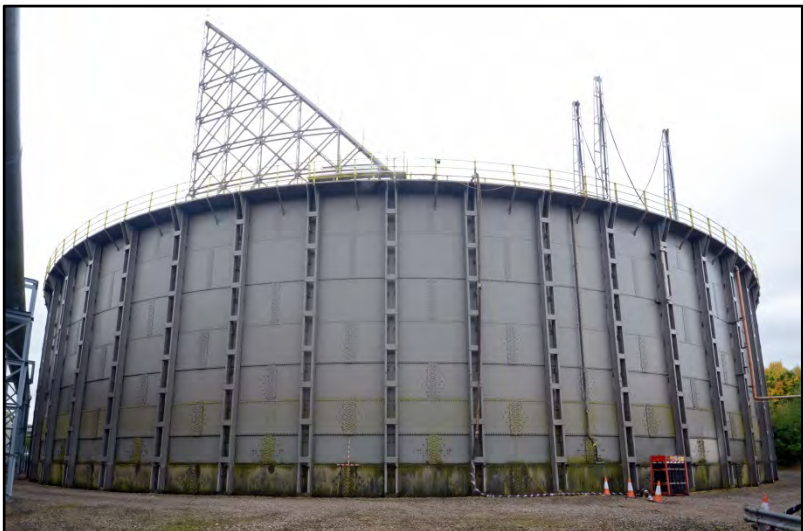
Gas holder 1, looking south-west Fig 20
