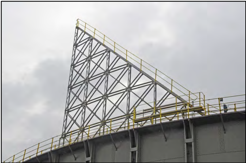
Detail of lift-tank access stair Fig 38
