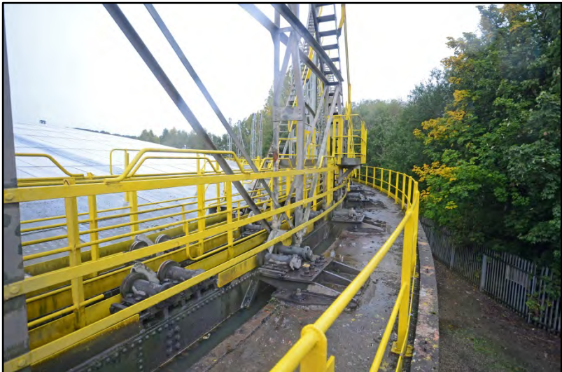
The gasholder walkway and handrails, looking north Fig 68
