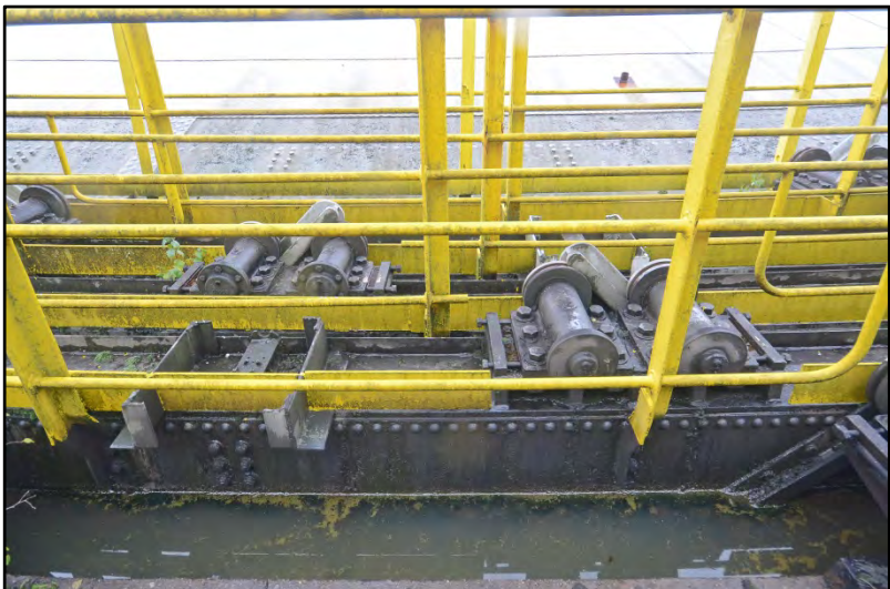
Detail of inner roller carriages Fig 70
