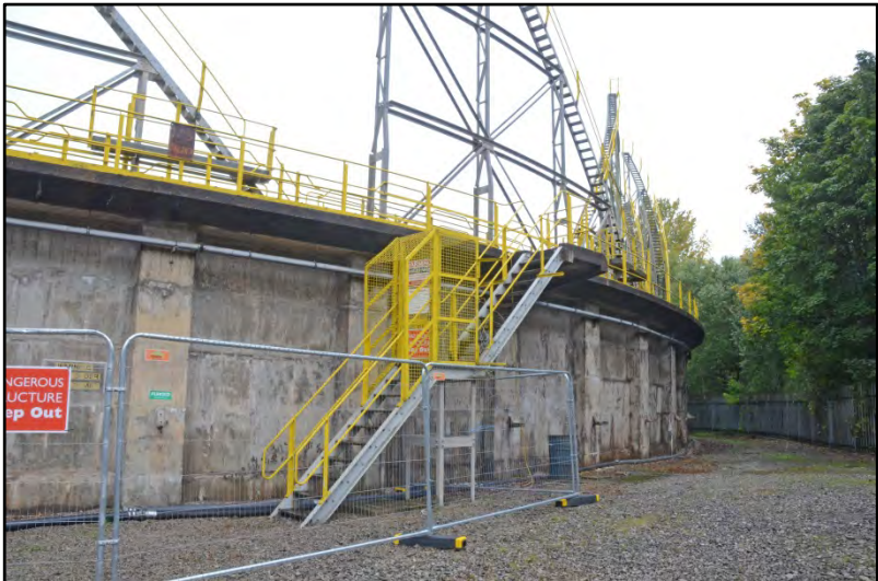
The base-tank steps Fig 64
