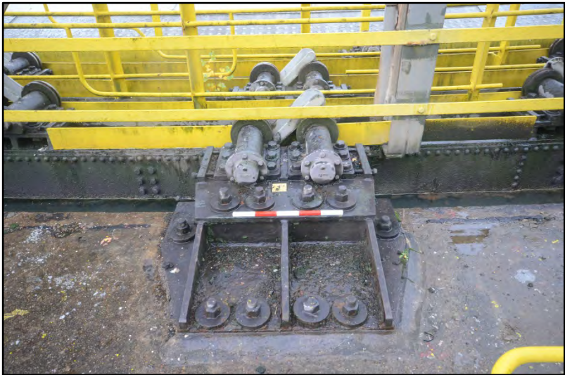
Detail of outer roller carriage Fig 71
