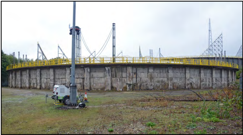
Gasholder 3, looking south-east Fig 58
