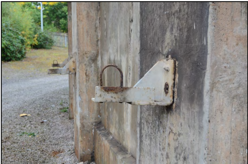
Brackets for former pipes Fig 60
