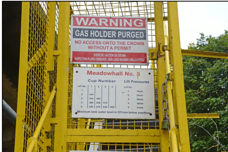
Signage on the base-tank stair Fig 65
