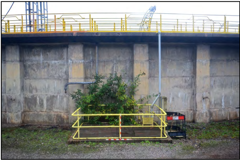
Sump at the south-east side of the gasholder Fig 57
