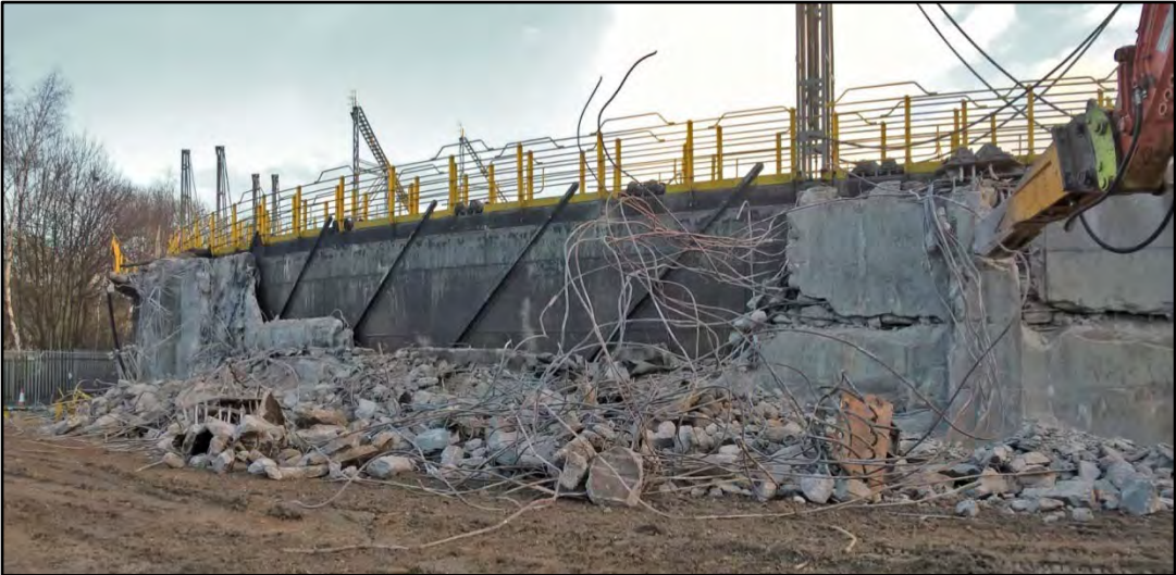
Demolition of the concrete tank, showing reinforcing bars Fig 78
