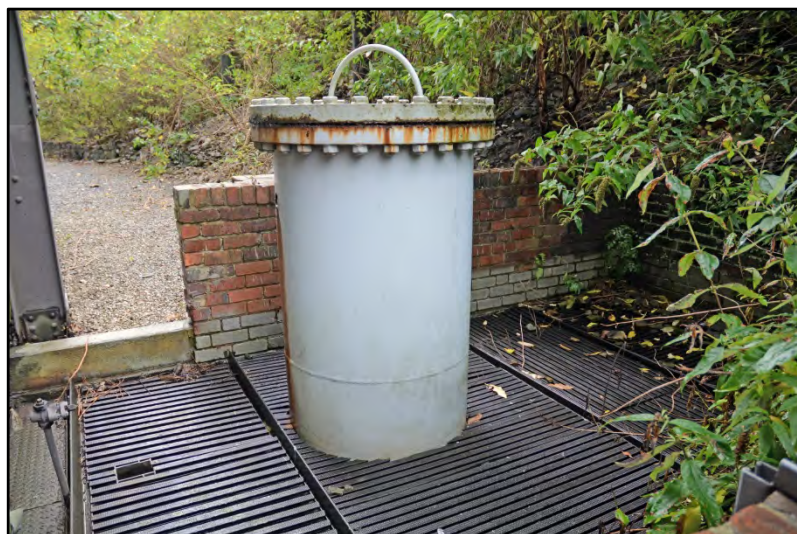
Sealed pipe from the sump Fig 23
