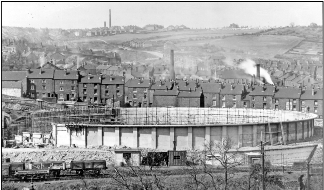
Undated view of Gasholder 3 under construction (u04893) Fig 6
