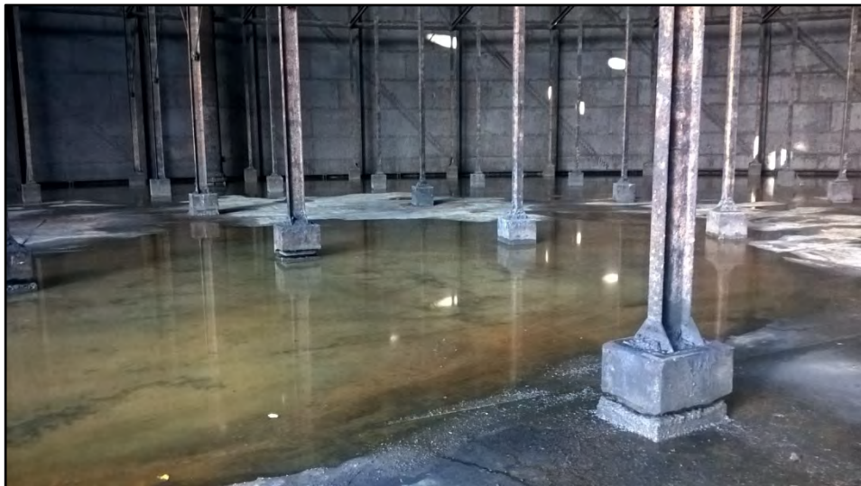
The crown-rest supports Fig 45
