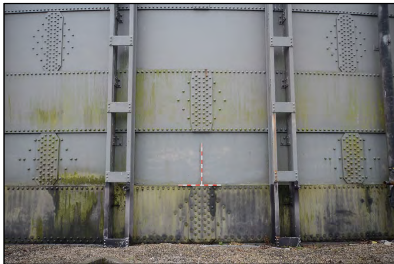
Detail of the outer tank fabrication Fig 13
