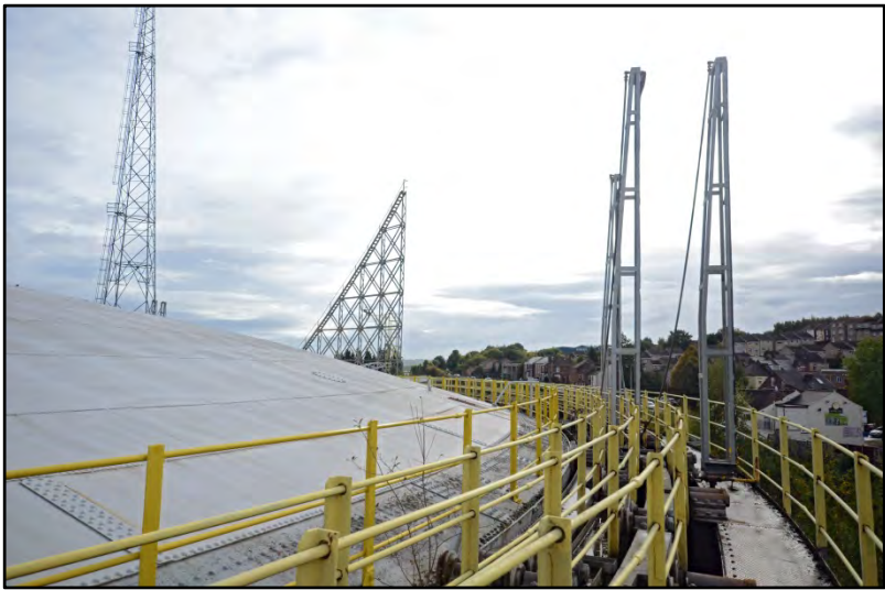
General view of the gasholder, looking south Fig 39
