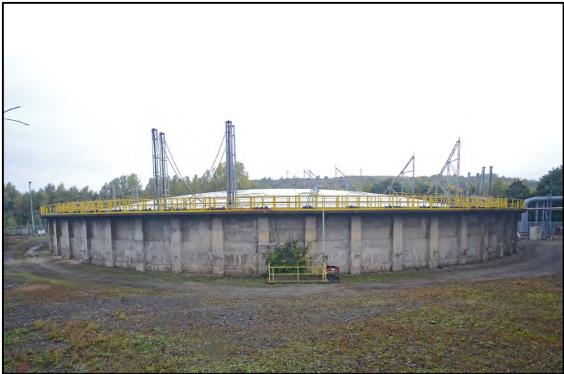
Gasholder 3, looking north-east Fig 56
