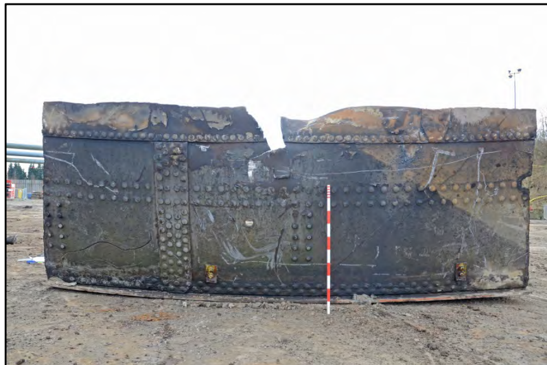
Detail of the top-curb fabrication Fig 88
