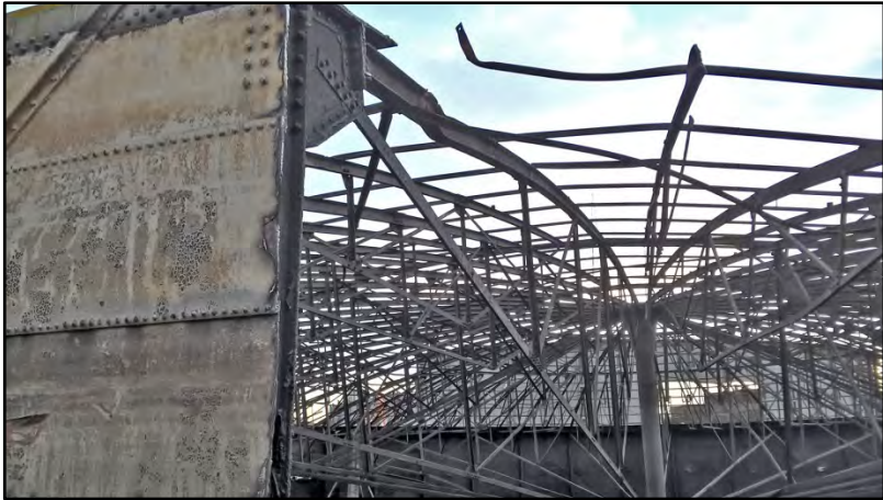
The top-curb and outer extent of the crown-rest Fig 82
