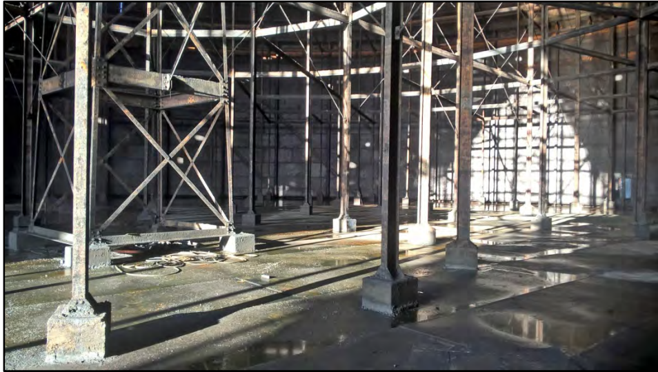
Interior of Gasholder 1, showing the crown-rest supports Fig 44
