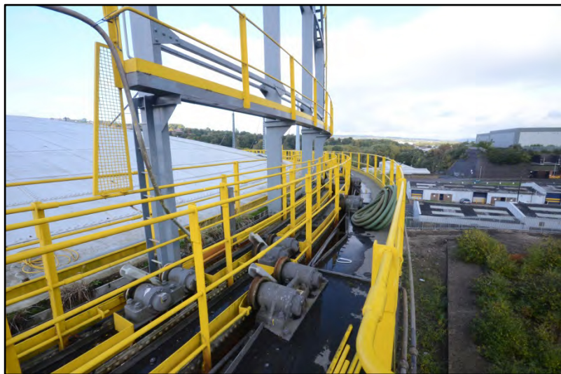
The base-tank walkway and handrails, looking west Fig 32
