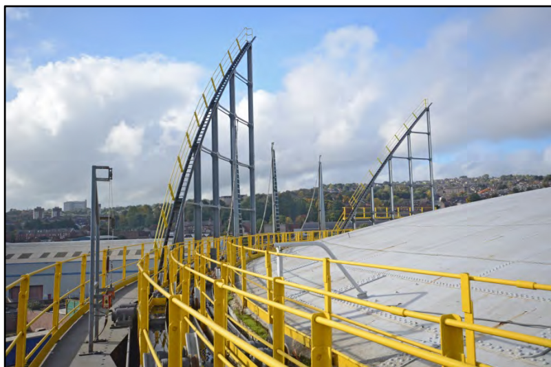
The lift-tank stairs, looking south Fig 33
