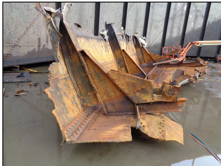
The underside of the top-curb, showing brackets and truss supports Fig 49
