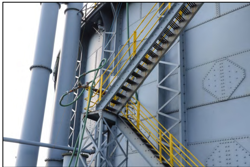
The mid-height stair landing Fig 29
