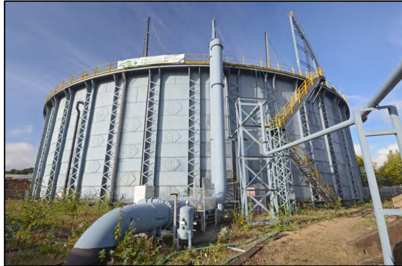
The gasholder, looking south-west, showing inlet / outlet pipes Fig 22
