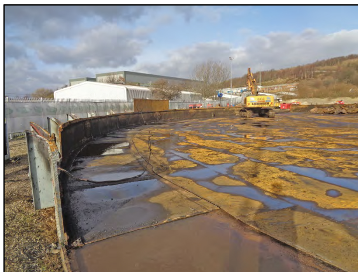
The gasholder base, looking north-west Fig 58
