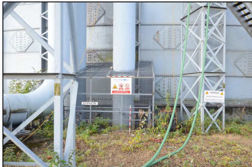
The pipe pit / dry well Fig 24
