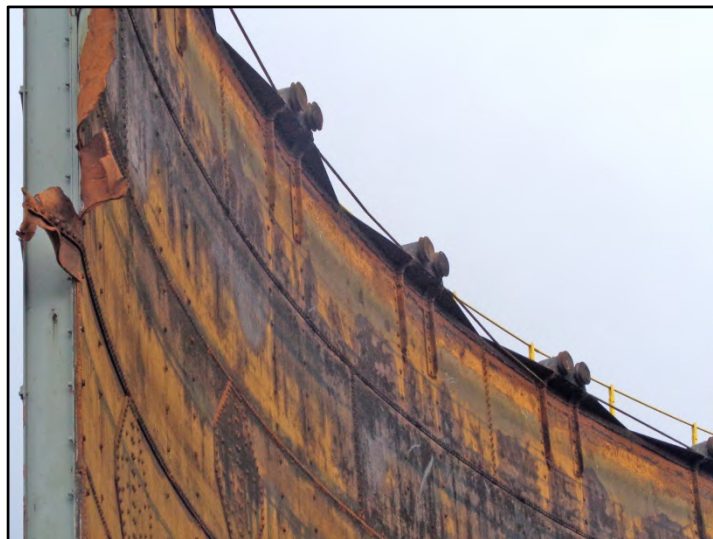
The inner face of the base-tank Fig 52
