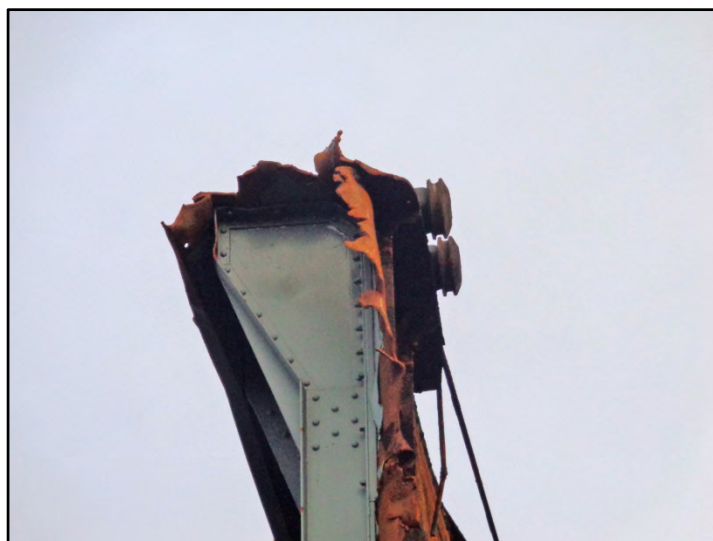
Detail of the base-tank columns' upper brackets Fig 53
