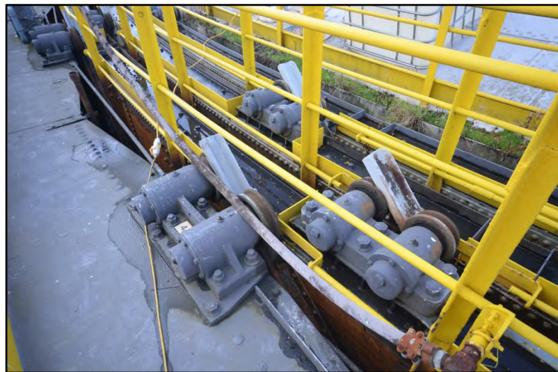
The arrangement of the roller carriages Fig 35
