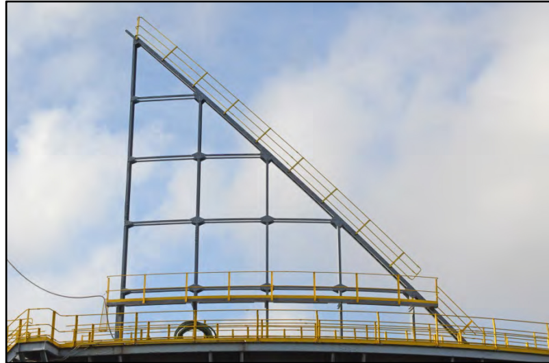
Detail of lift-tank stair Fig 34
