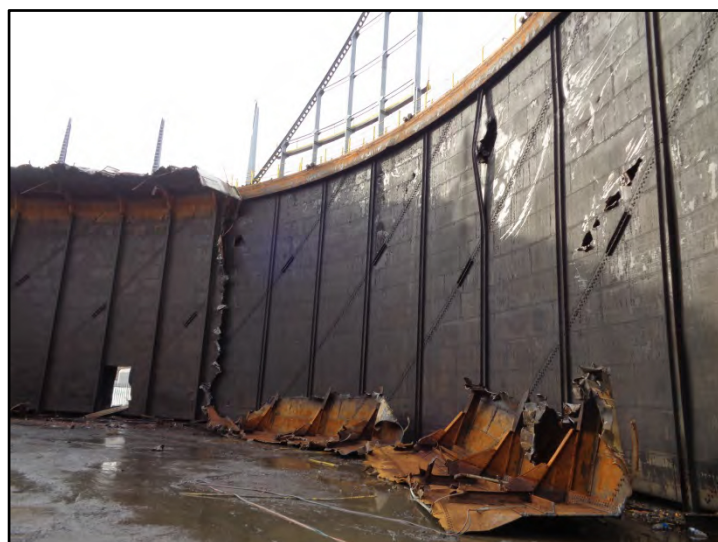
The inner face of the lift-tanks Fig 50
