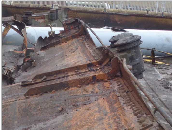
Roller carriage and supporting brackets Fig 51
