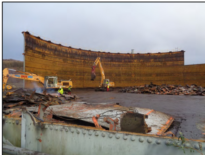
Dismantling of the base-tank Fig 57
