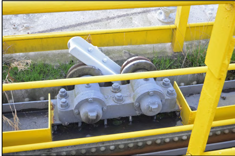
Detail of a lift-tank roller carriage Fig 37
