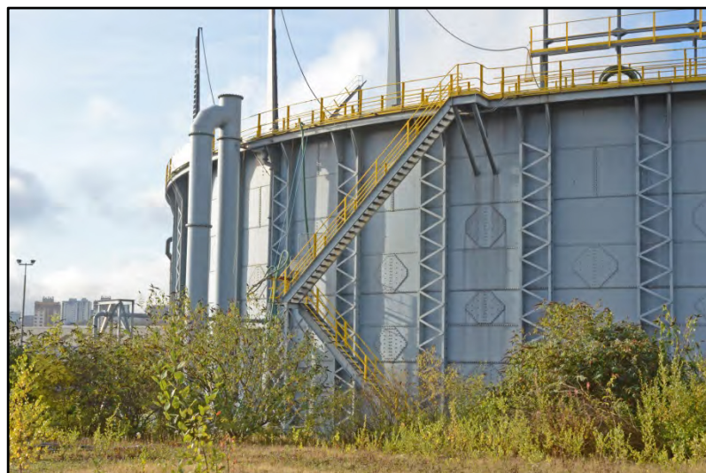
The base-tank stair, looking south Fig 27
