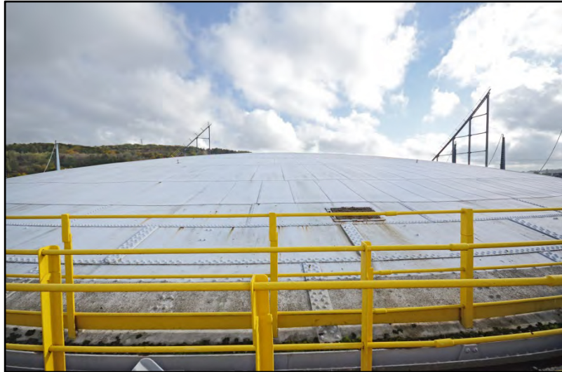
The gasholder crown, looking east Fig 31
