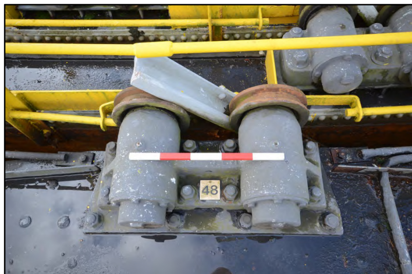
Detail of a base-tank roller carriage Fig 36
