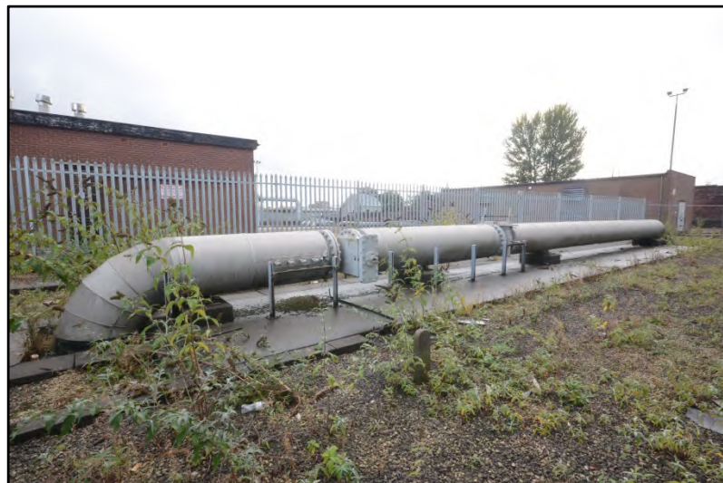
Outlet pipe adjacent to gasholder, looking south-east Fig 26
