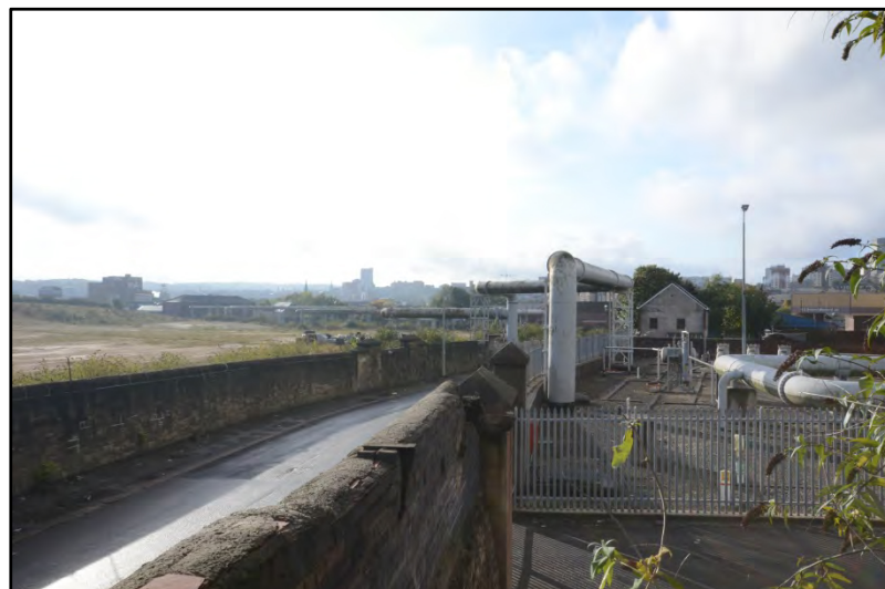
Gas pipes leaving the National Grid compound, looking south Fig 11
