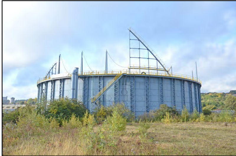
The gasholder, looking south-west Fig 16
