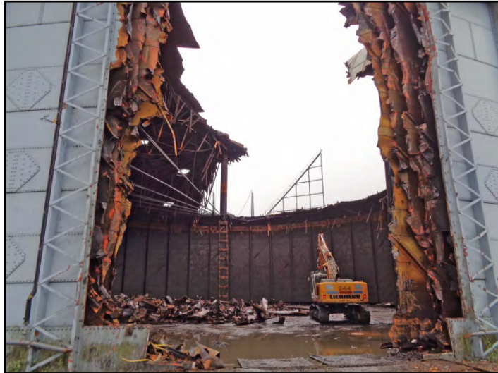
Dismantling of the gasholder Fig 45
