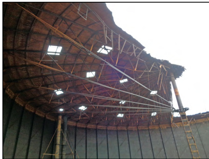
The gasholder crown-frame Fig 47
