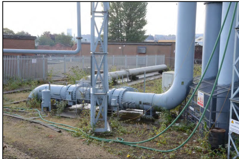
The inlet / outlet pipes, looking south Fig 23
