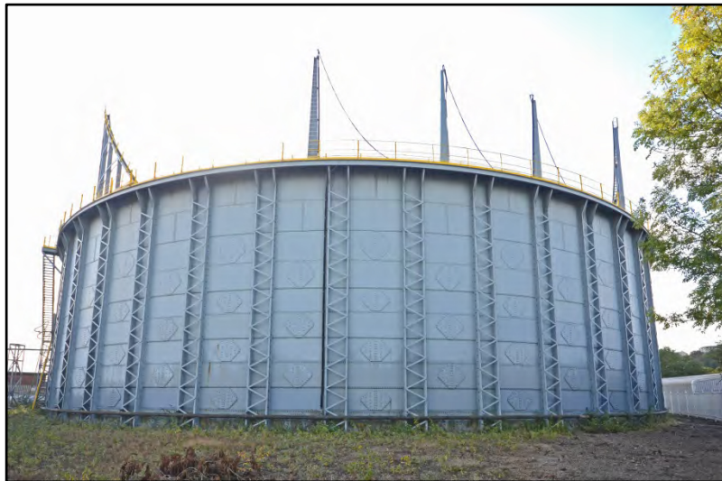
The gasholder, looking south-east Fig 17
