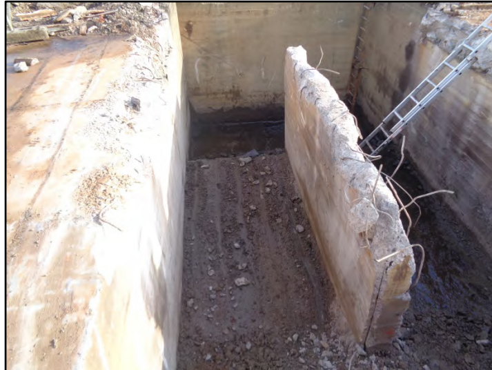
The pipe pit Fig 56
