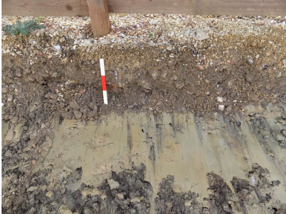
Section in existing gravel layer
