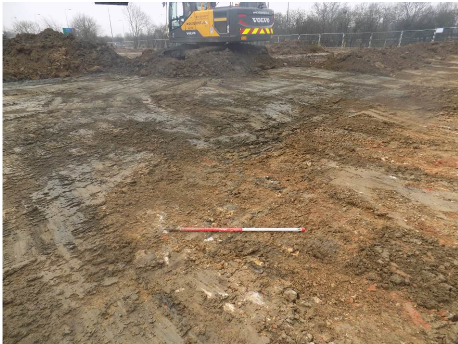
General view showing stripped area, looking south-west Fig 4
