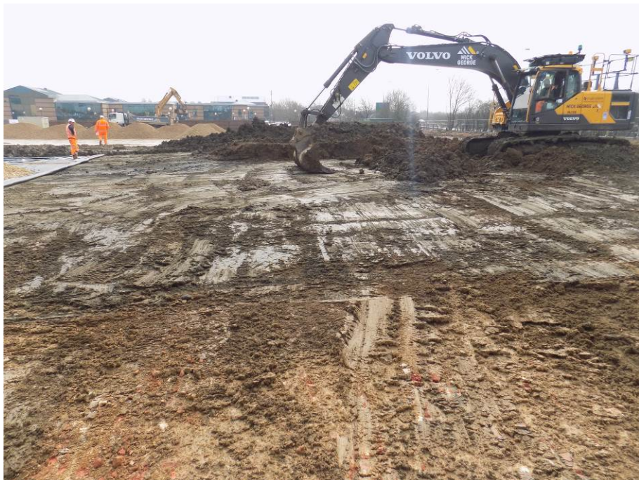
General shot showing stripped area, looking south
