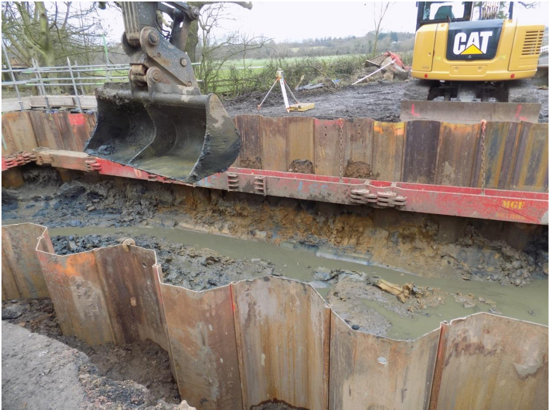
Southern culvert (Culvert 3), possible agger in section, looking north-west Fig 7
