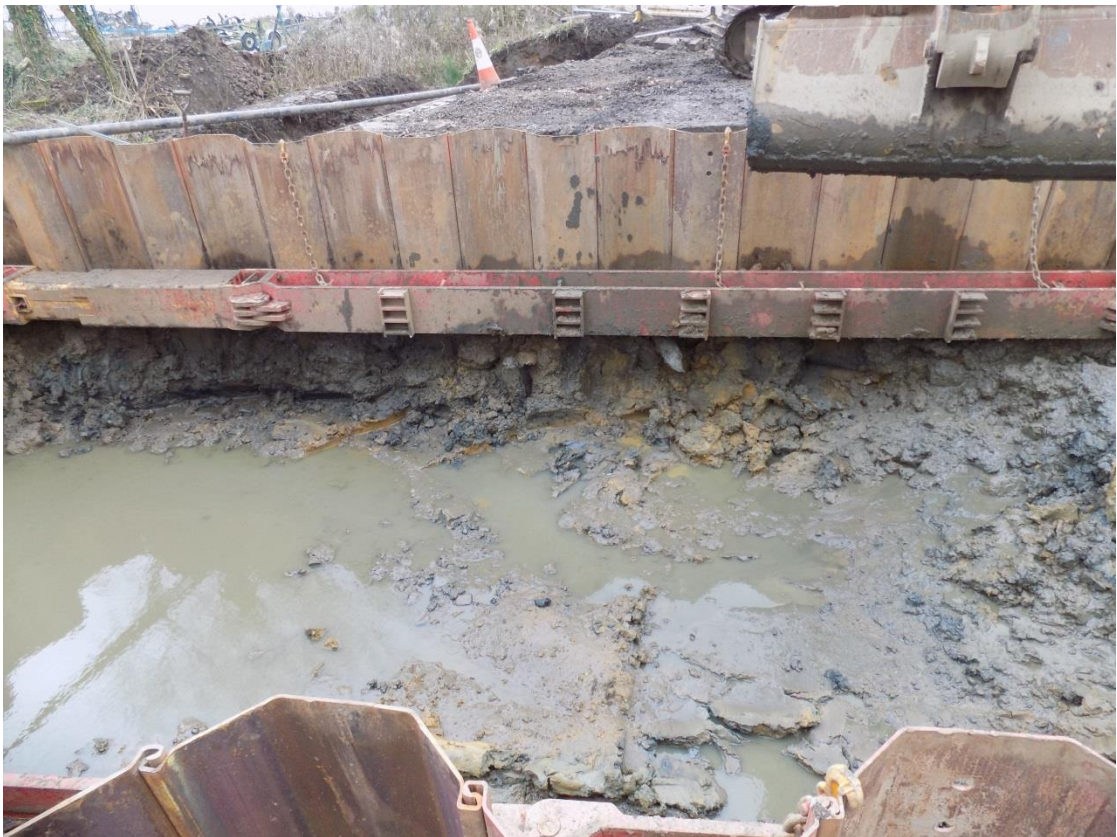
Southern culvert (Culvert 3), timber posts in section, looking south Fig 8
