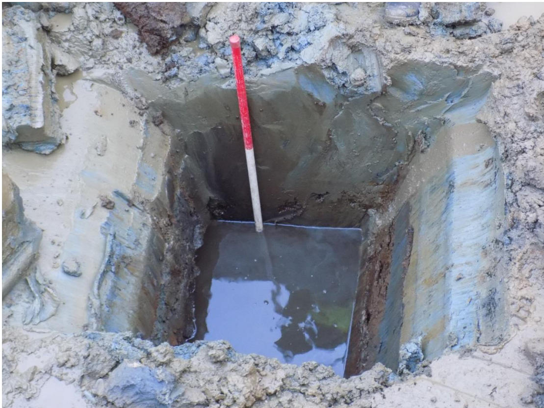
Northern culvert (Culvert 2a), sondage in trench floor, looking north Fig 6
