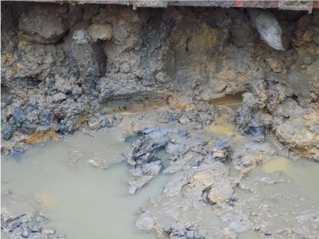
Southern culvert (Culvert 3), timber posts (close up), looking south
