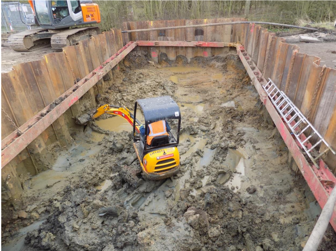
Northern culvert (Culvert 2a), looking east Fig 5
