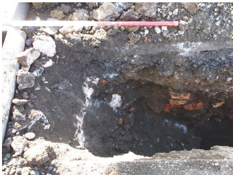
Test Pit 2, section showing modern road build-up (204), looking south Fig 4
