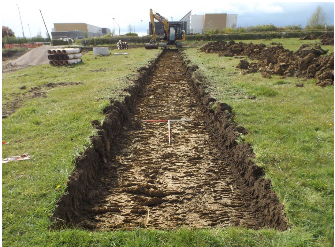
Trench 3, looking west
