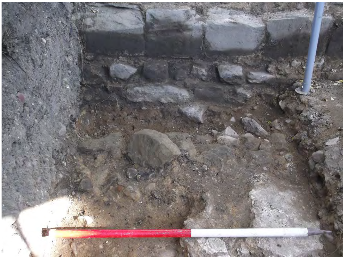
Area B1, foundations for possible earlier cloister wall [1084], with white mortar surface [1085] abutting, looking north Fig 28
