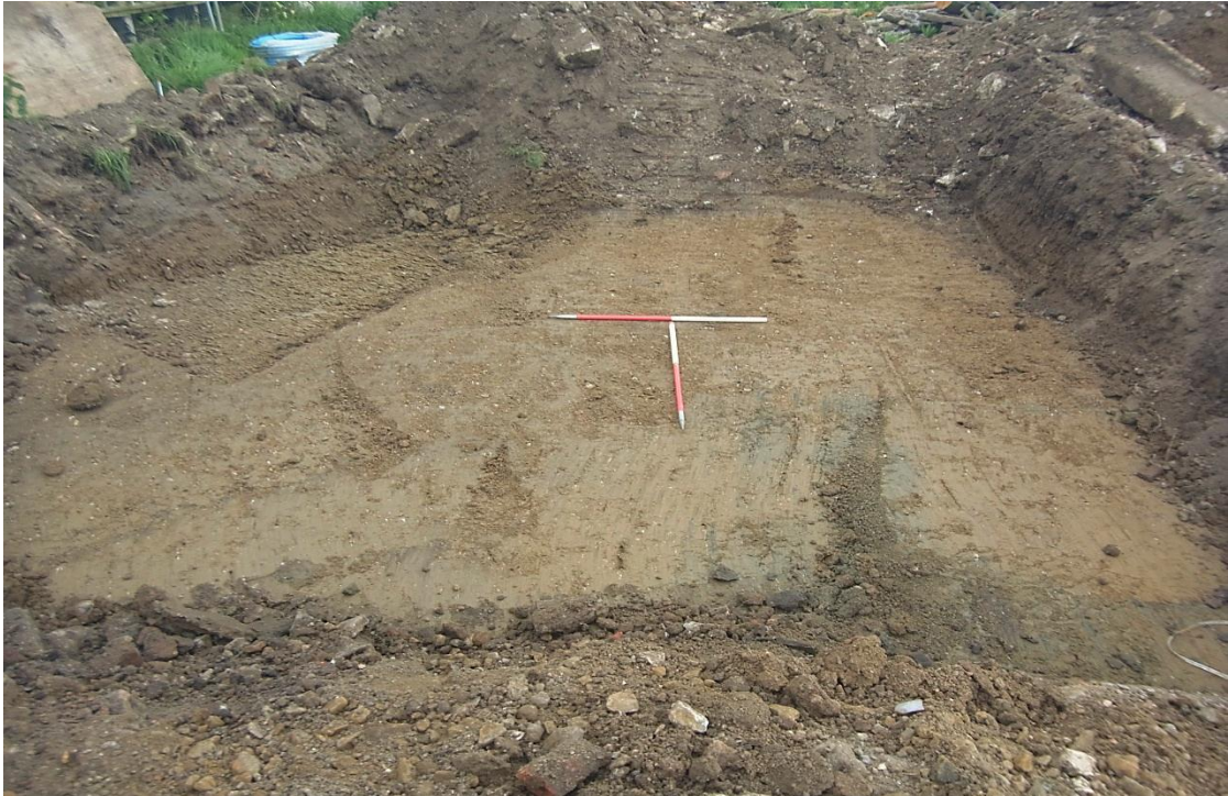
Area 3 general view, looking south Fig 8
