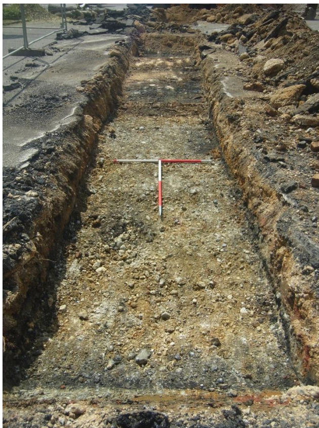
Trench 3, looking south-west Fig 6
