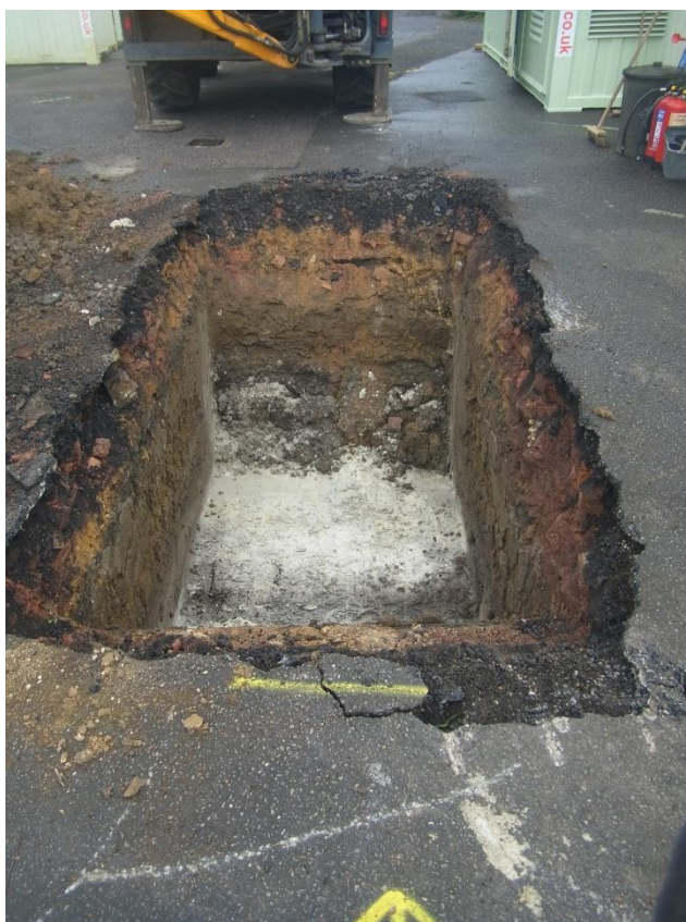
Trench 4, looking north-west Fig 7
