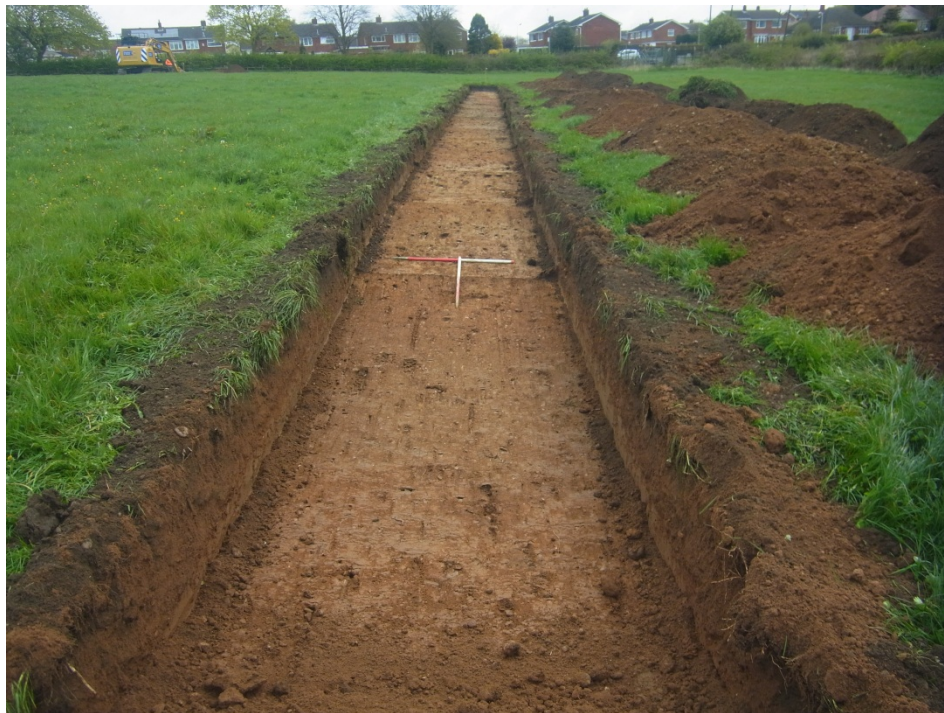
Trench 5 overview, looking east Fig 20
