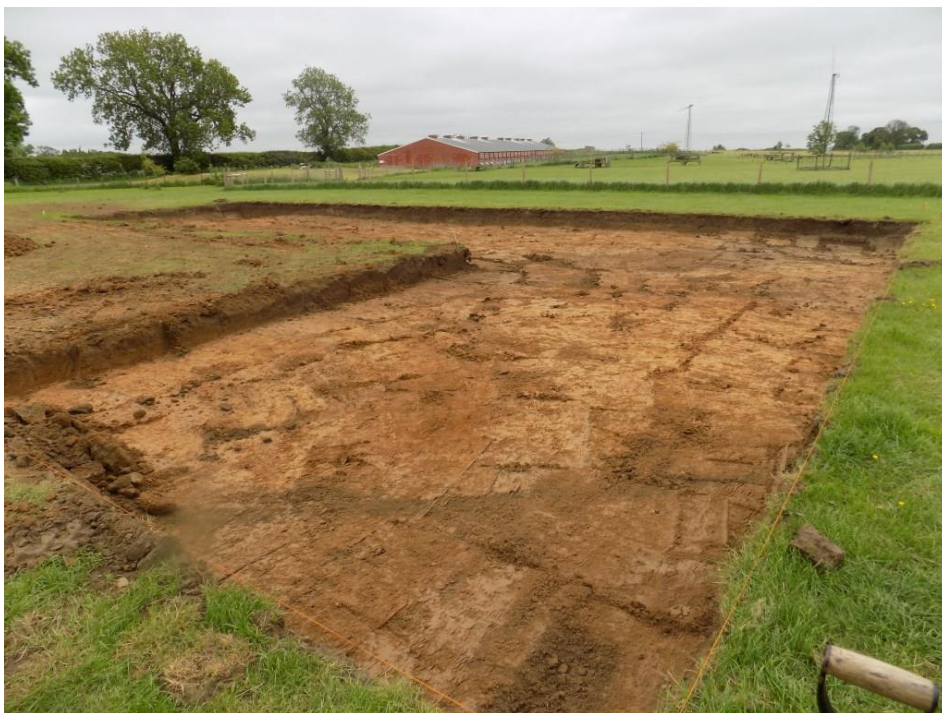
Building plot fully excavated showing furrows, looking south-east Fig 3
