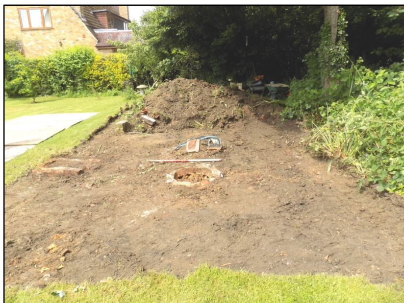
Septic tank [4] and associated structures, looking west Fig 4
