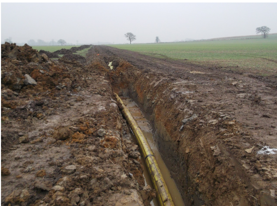
General view; central section, looking east
