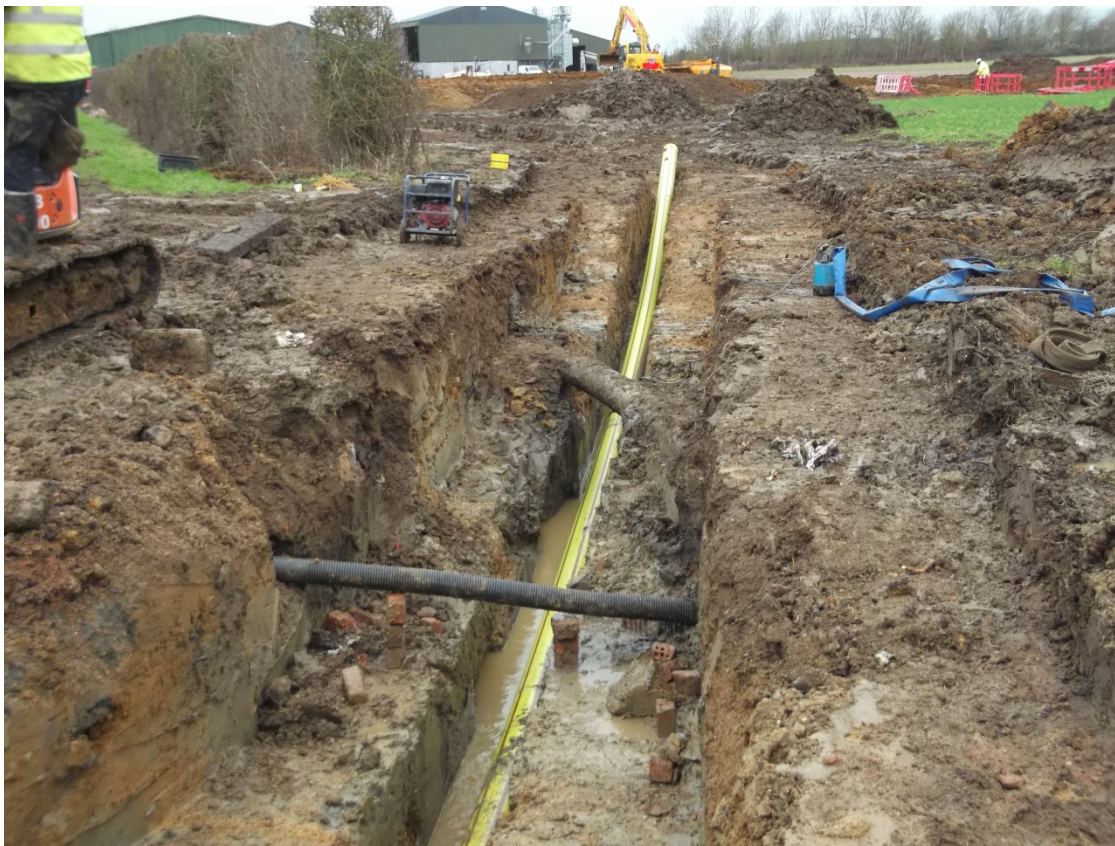
Gas pipeline, south end; looking south-west
