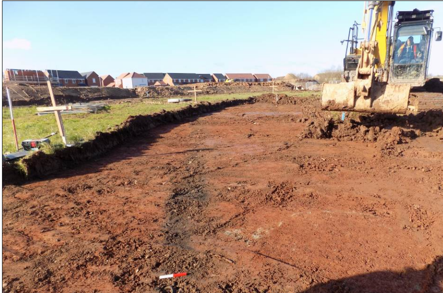
Overview of Area B, looking north-west Fig 12
