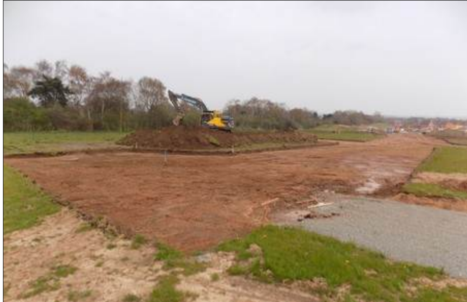
Overview of Area A, north road, looking east Fig 3
