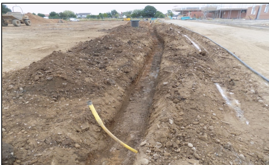
Service trench, looking east Fig 9
