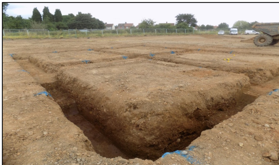
Plots 91-92, showing stepped foundations, looking north-east Fig 7
