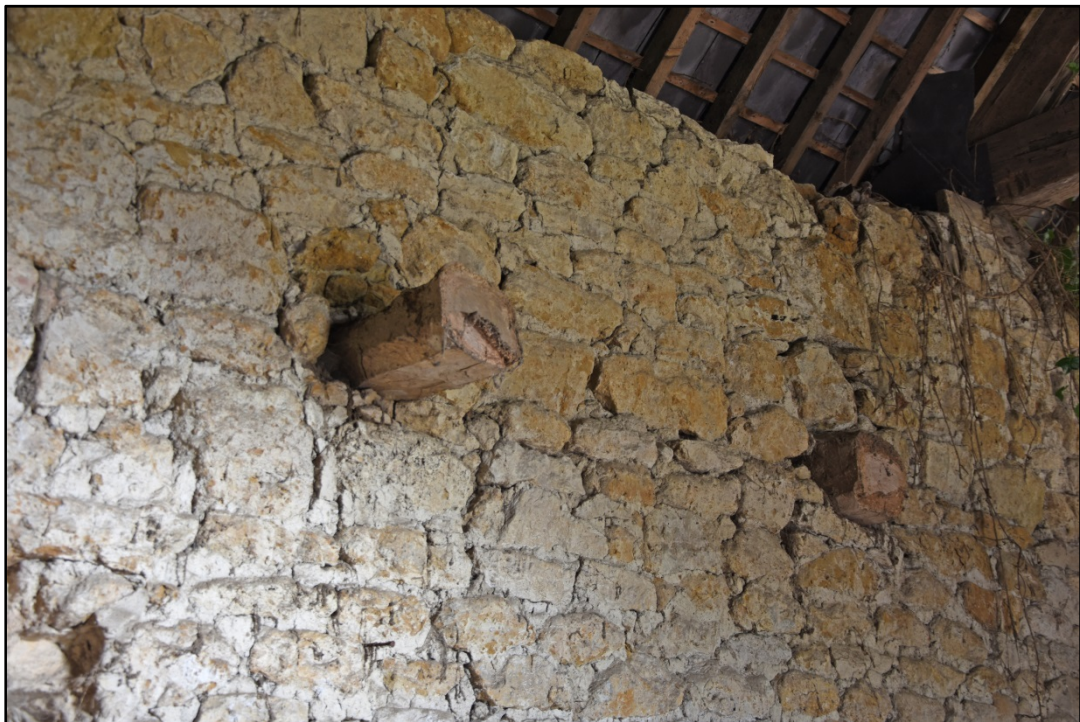
The truncated beams of the north wall Fig 23
