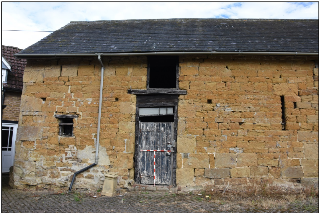
The southern extent of the east elevation Fig 9
