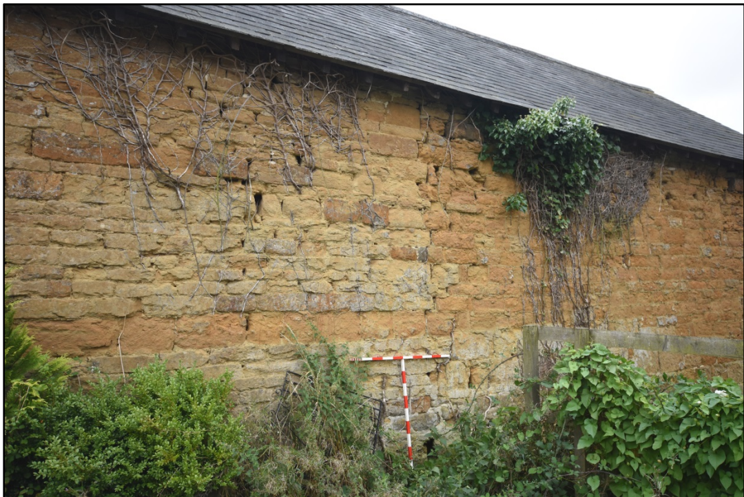
The vertical joint on the west elevation, looking south Fig 15
