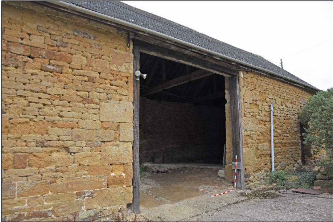
The central doorway Fig 10
