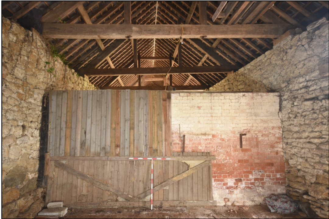
The brick and timber partition, looking north-east Fig 28
