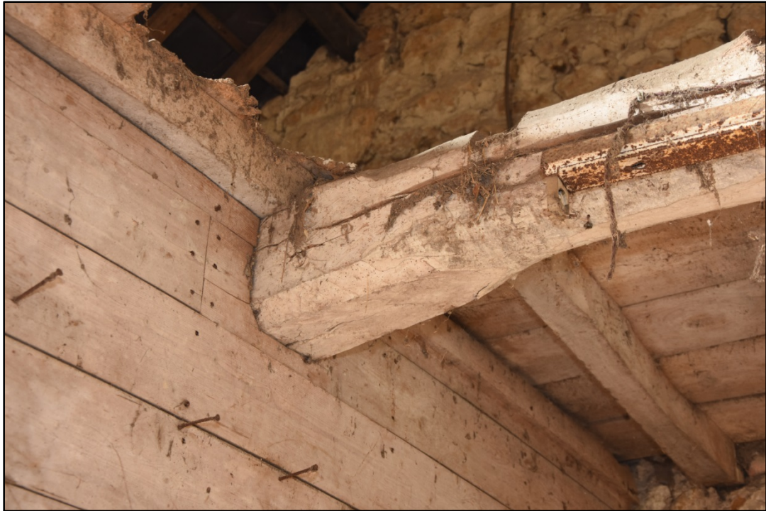
Detail of beam, adjacent to the store room Fig 24
