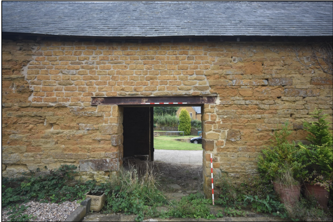
The reduced doorway and area of repair Fig 14
