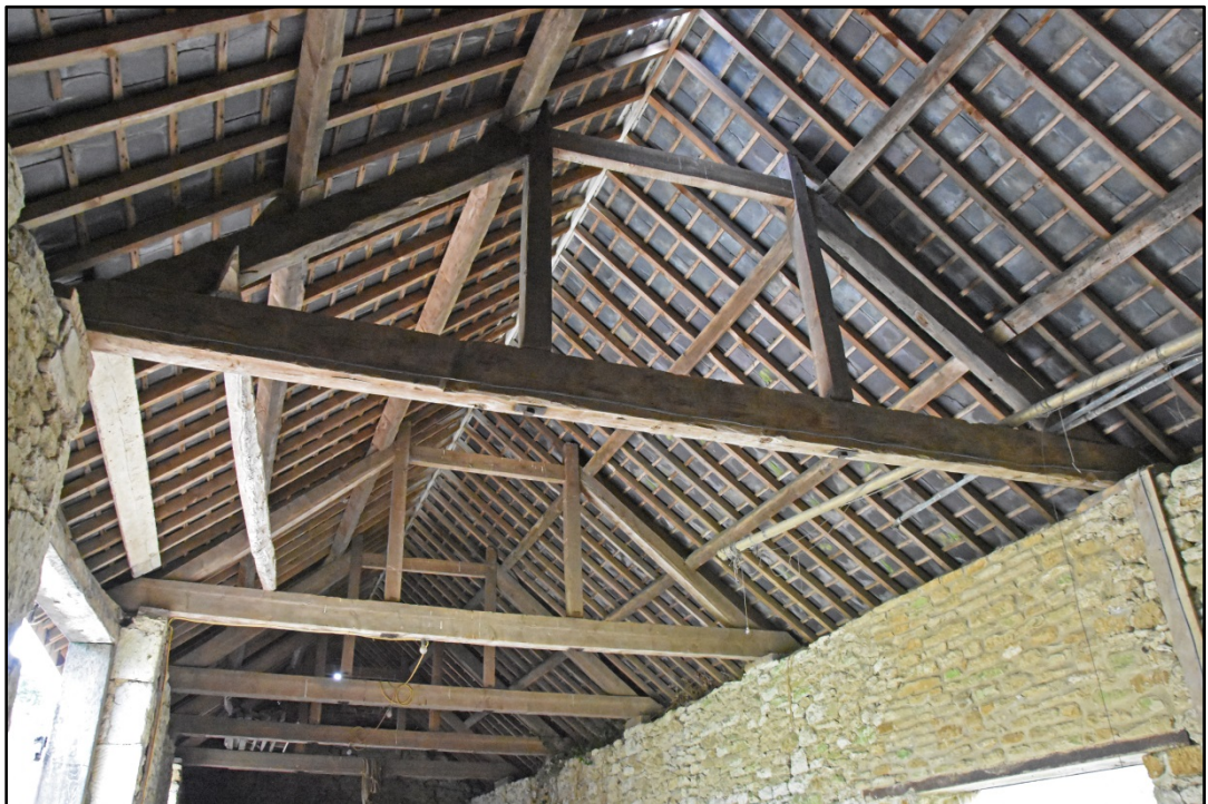
The roof structure, looking south-west Fig 37
