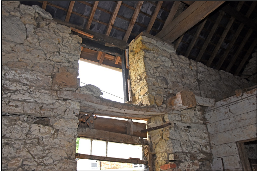
Detail of the timber work around the doorway and overhead window Fig 26
