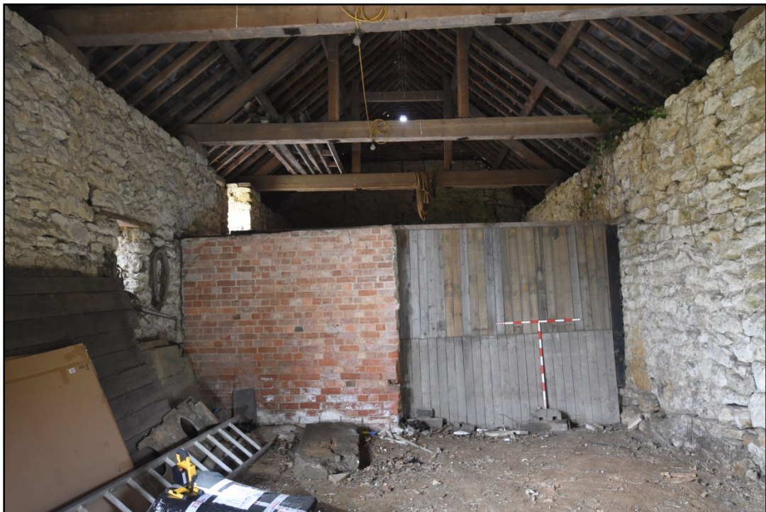
The brick and timber partition, looking south-west Fig 29
