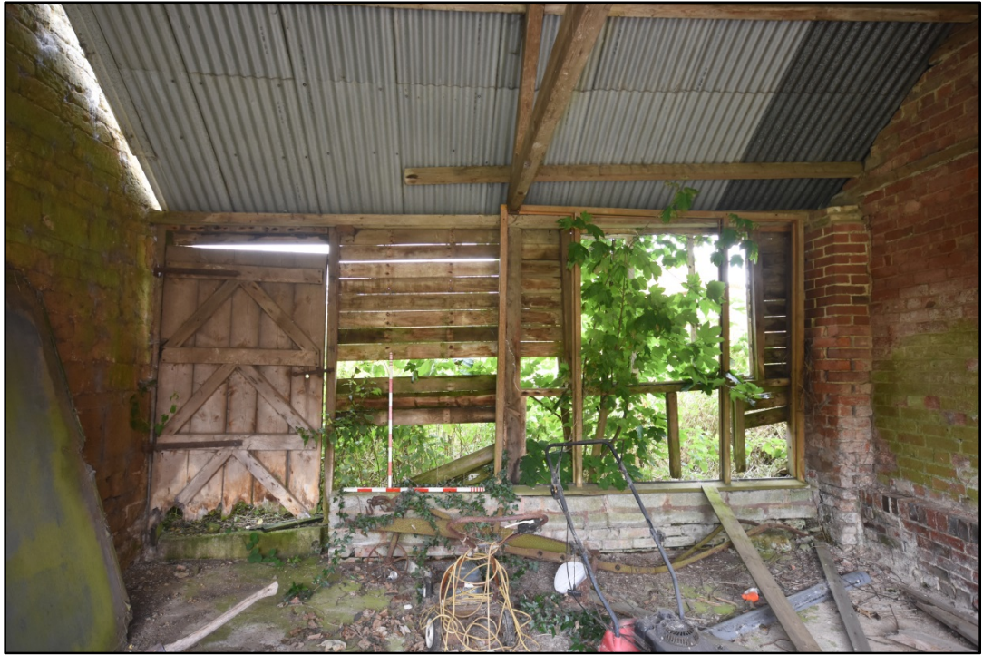
The west wall of the extension Fig 40
