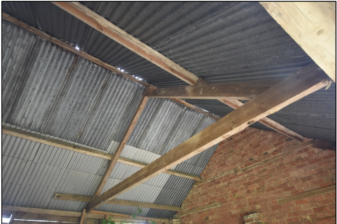
The extension roof support Fig 41
