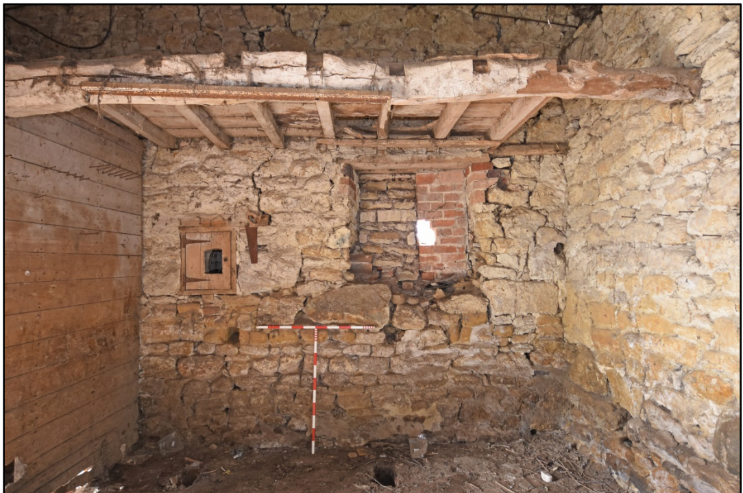
The south wall, showing the remains of the mezzanine floor Fig 21
