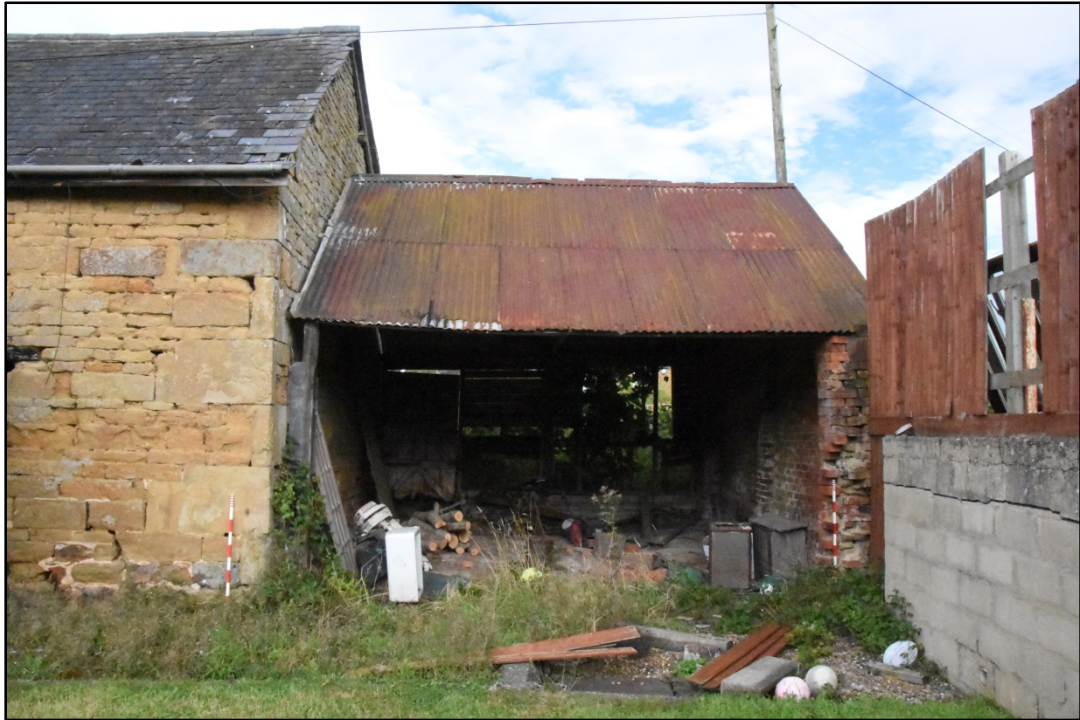
The extension, looking north-west Fig 12
