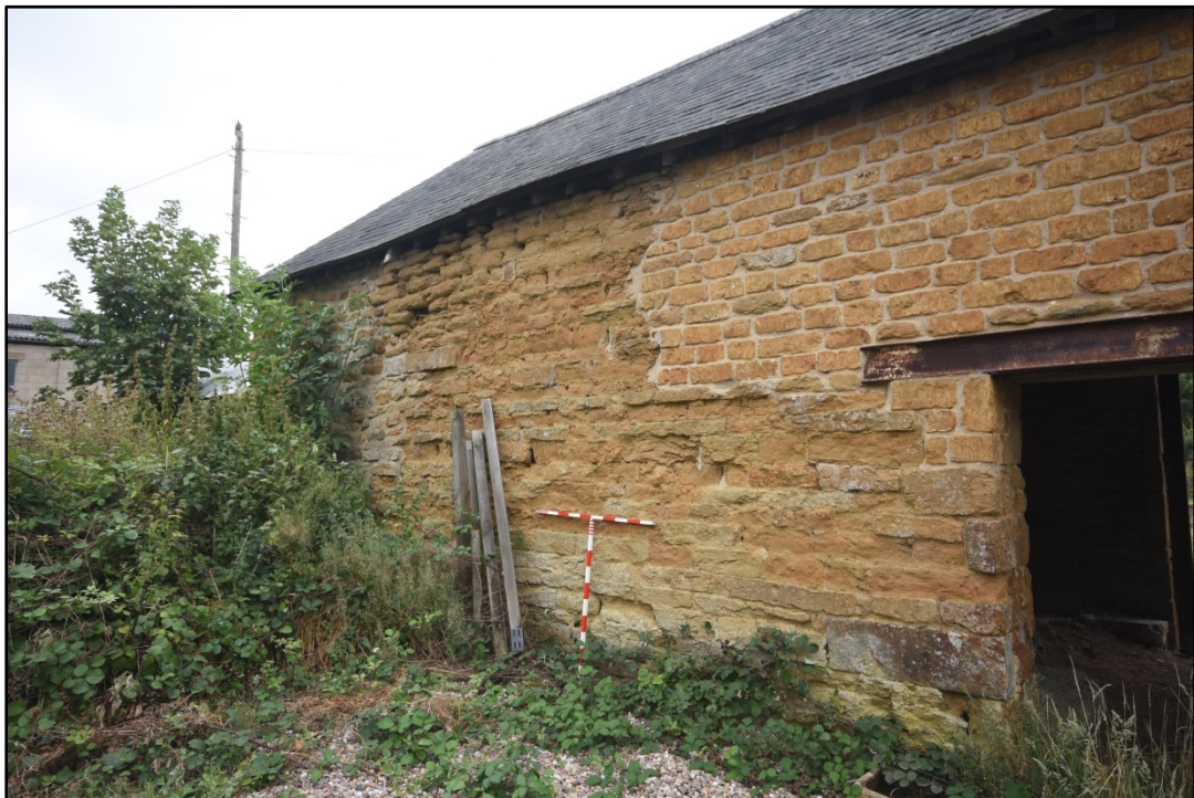
The northern extent of the south elevation Fig 13
