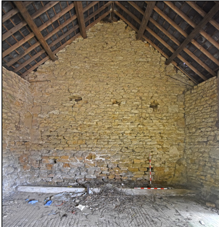
The north wall, showing three beam slots Fig 34
