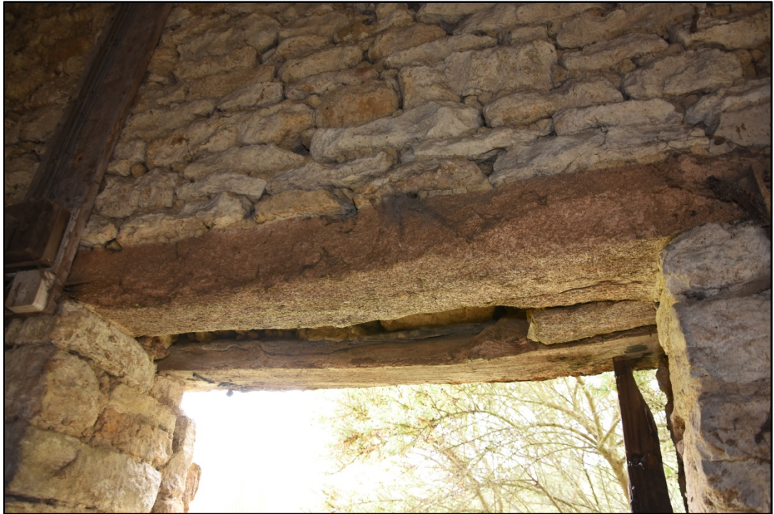
Detail of the lintel over the northern doorway Fig 36
