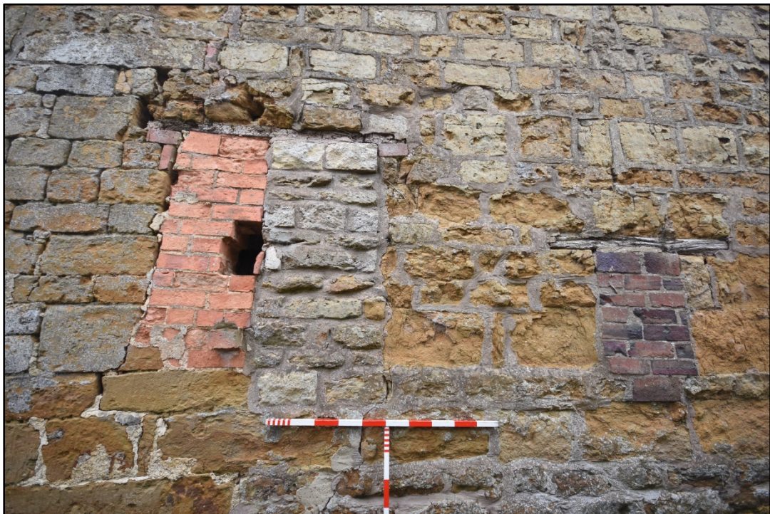
Detail of the blocked windows of the south elevation Fig 19
