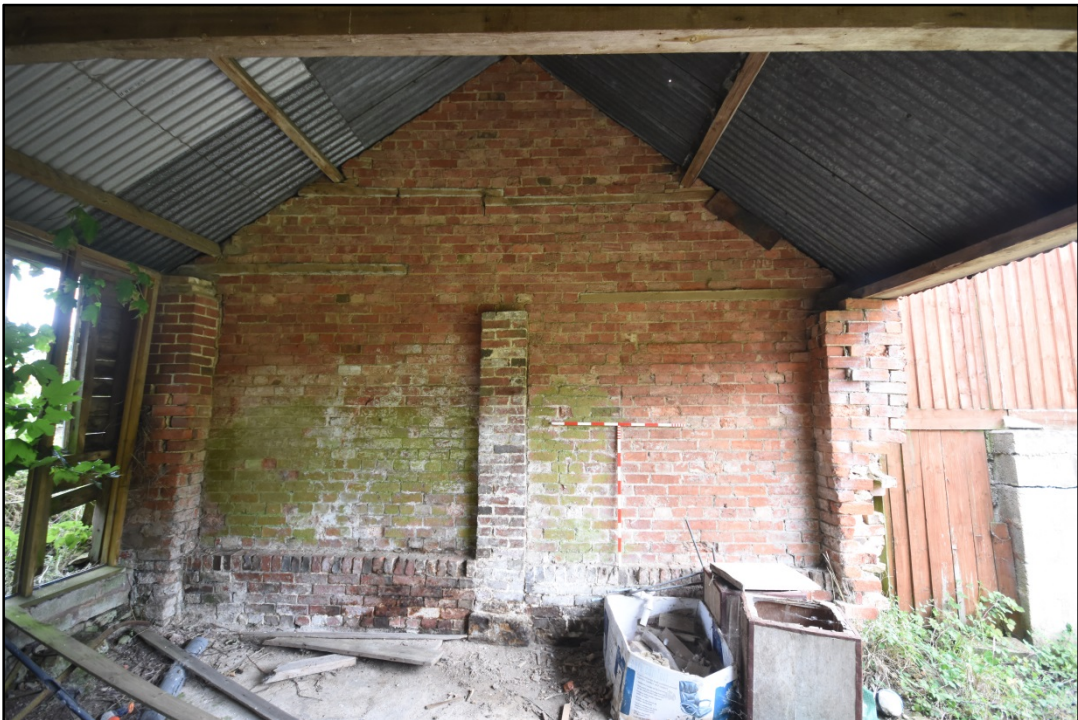
The northern elevation of the extension, looking north-east Fig 39
