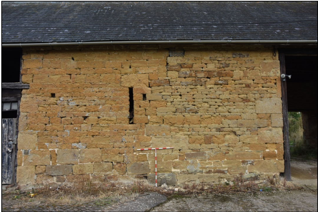
Detail of staggered joint and differing stonework to either side Fig 7
