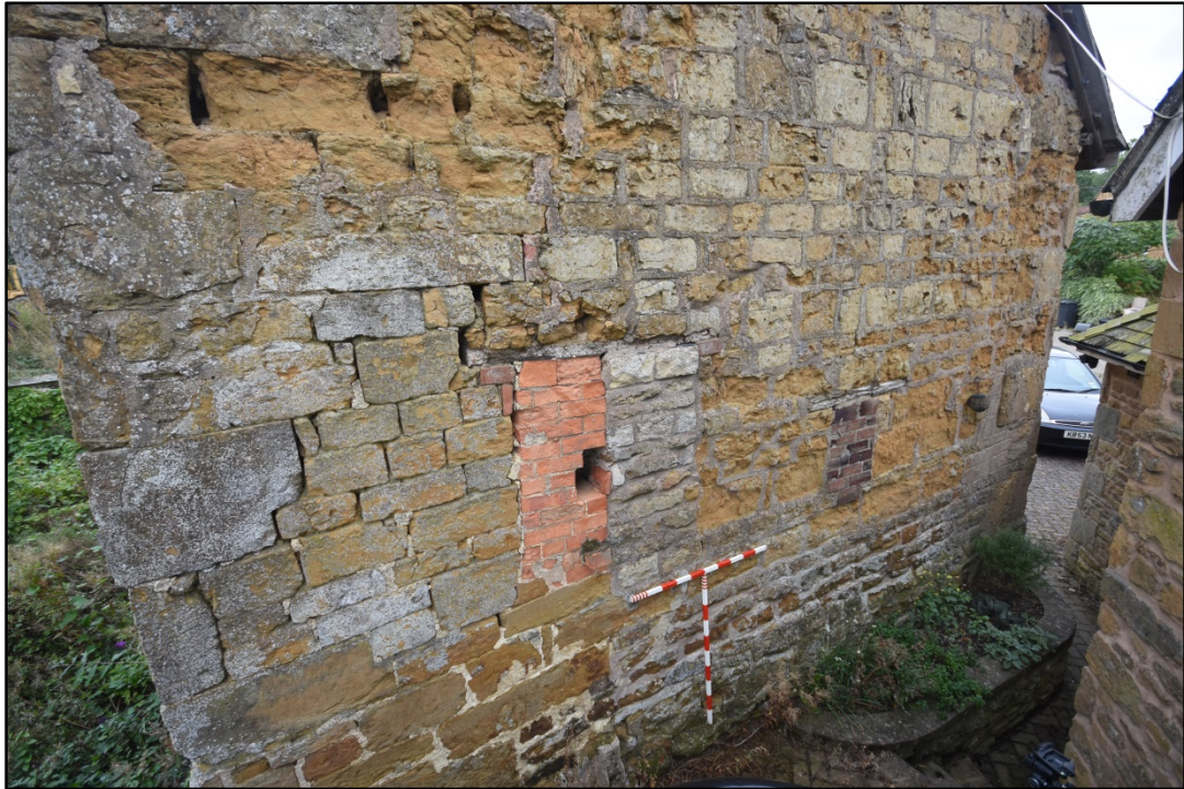
The lower portion of the south elevation Fig 18
