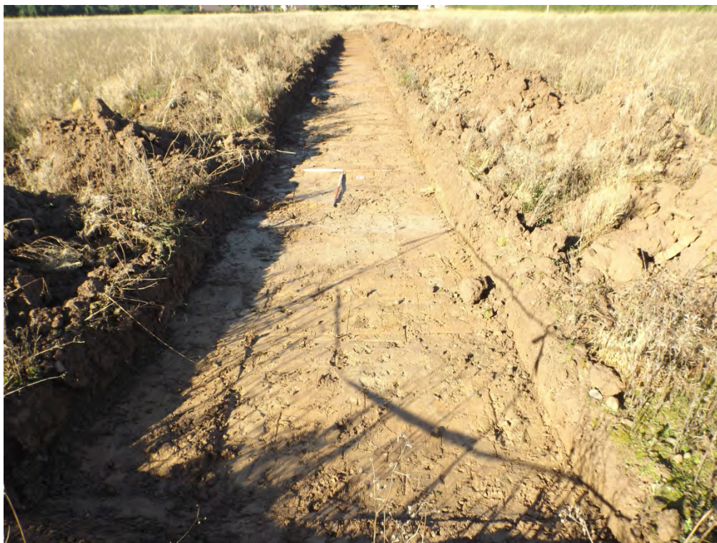
Trench 13 general view looking west
