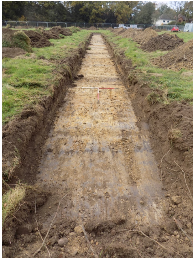
Trench 6 looking West
