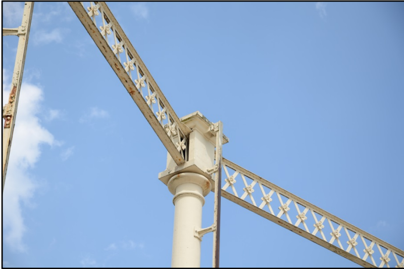
Detail of upper junction box Fig 38
