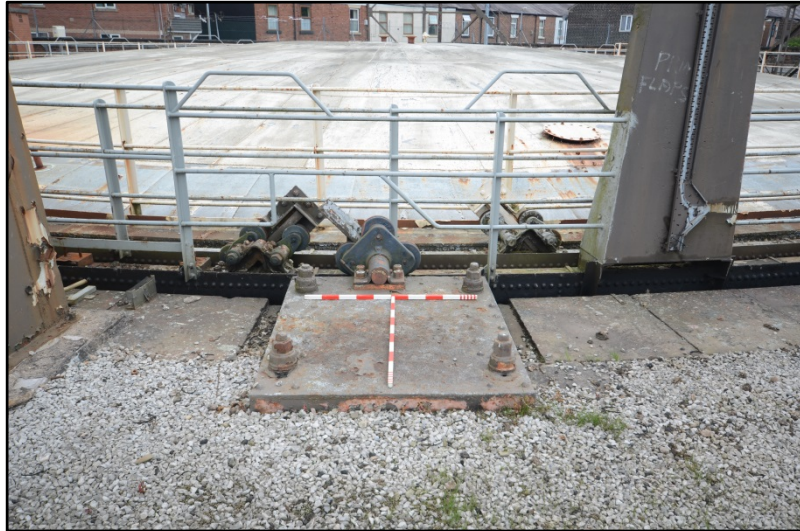
Detail of multiple roller carriage and top curb of the tank Fig 21
