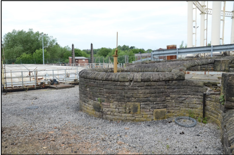
The siphon pit, looking west Fig 55
