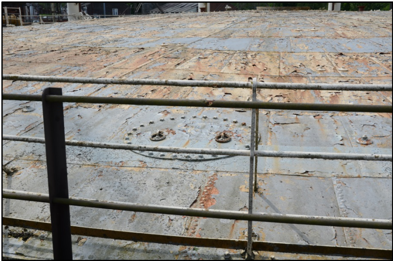
Detail of manhole Fig 44
