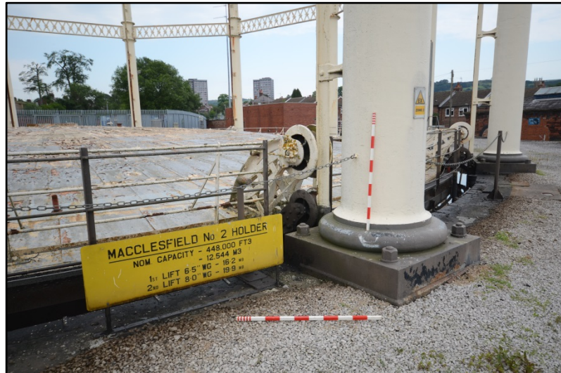
Column base with roller carriages, also showing gasholder signage Fig 33
