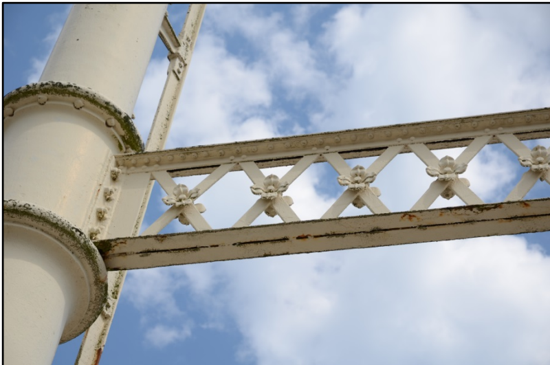
Detail of first tier girder with floret decorations Fig 39
