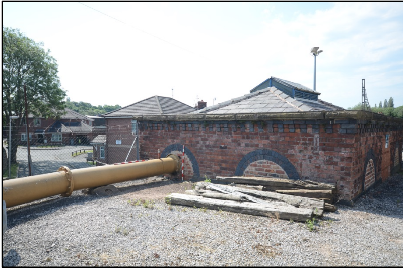
The Valve House, looking south-west Fig 57
