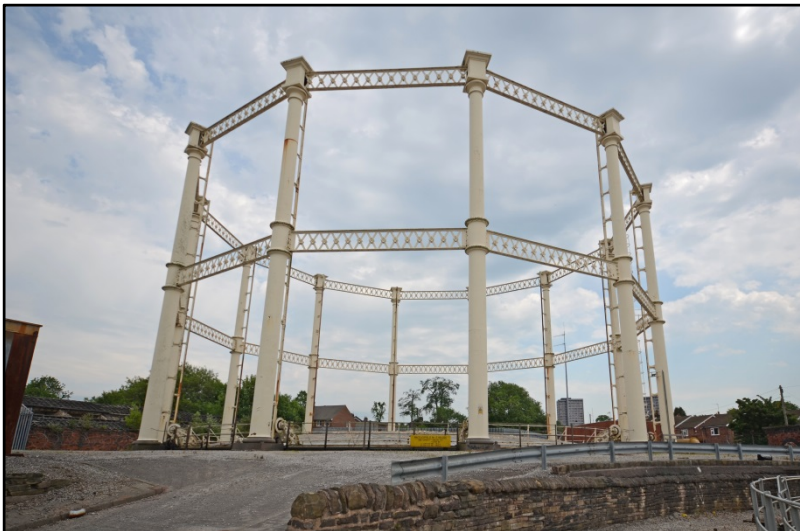
Gasholder 2, looking north-east Fig 31
