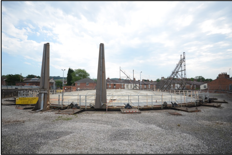
Gasholder 1, looking south-east, showing the anti-freeze supports Fig 19
