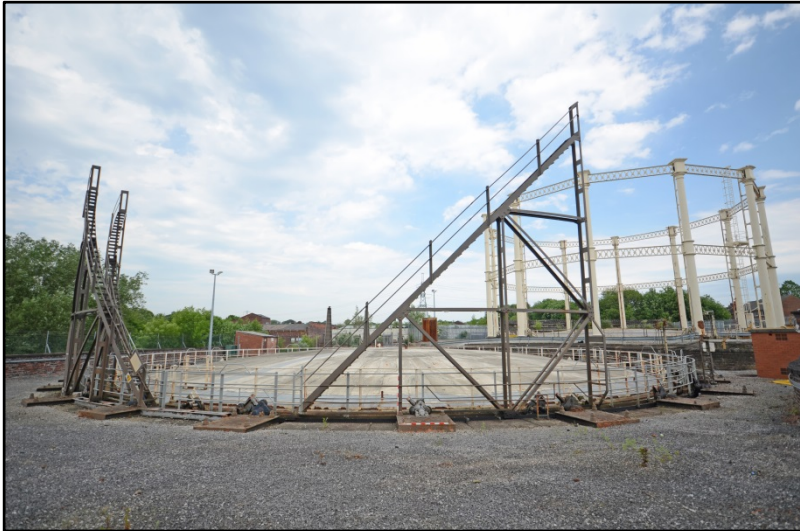
Gasholder 1, looking north, showing the access stairs Fig 18
