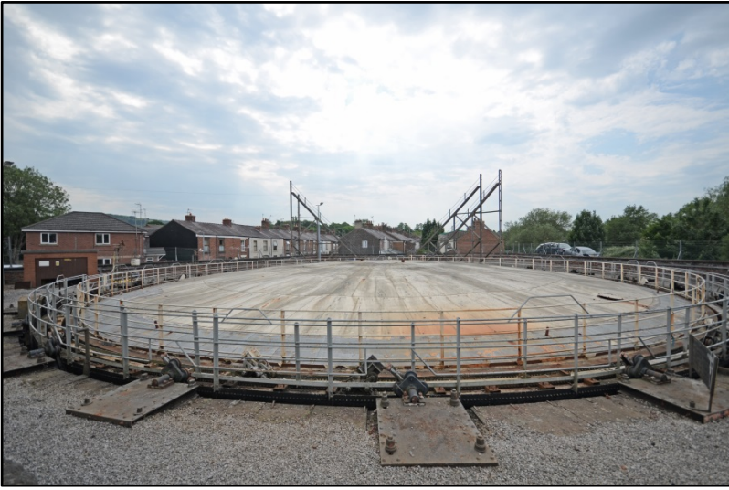
Gasholder 1, looking south Fig 17
