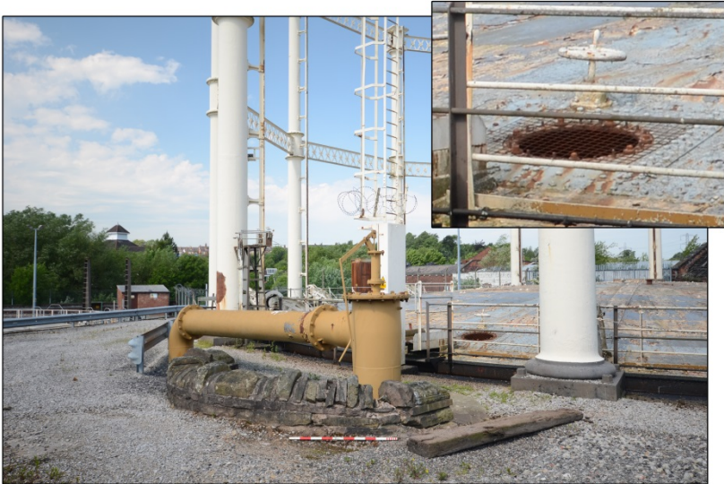
Siphon pit adjacent to the gasholder, with detail of Livesey Lid access Fig 42
