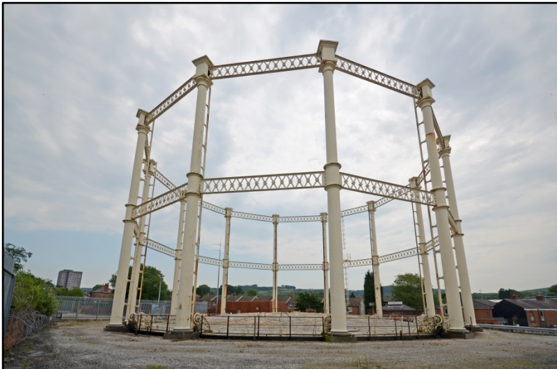
Gasholder 2, looking east Fig 30
