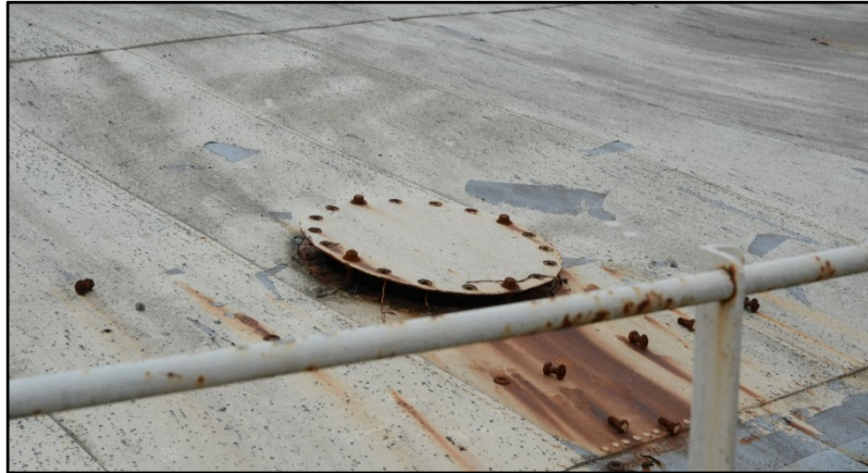
Manhole access through the crown Fig 24
