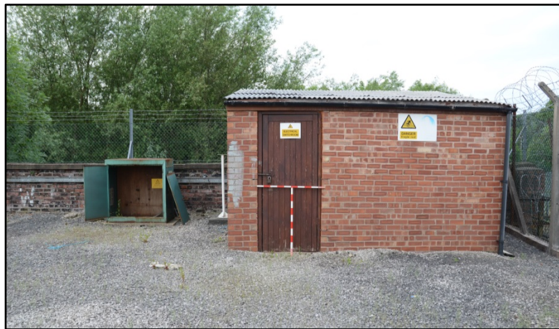
Electrical switch room Fig 29
