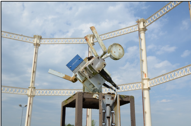
Detail of gasholder fittings Fig 46
