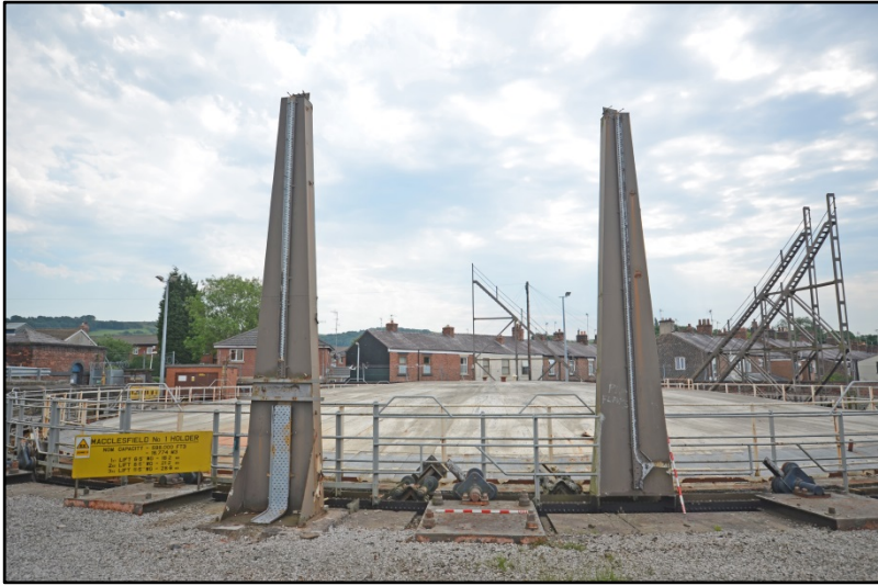
Detail of the anti-freeze supports and adjacent signage Fig 20
