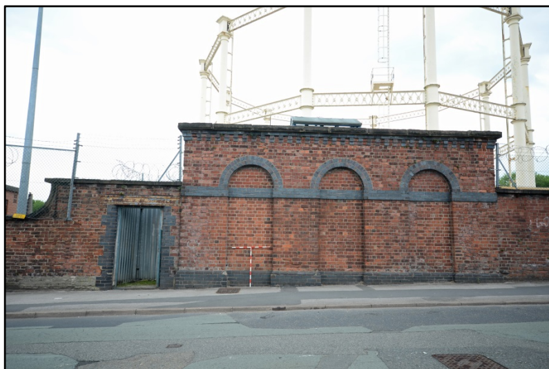
Entrance to the site and eastern elevation of the Valve House Fig 14
