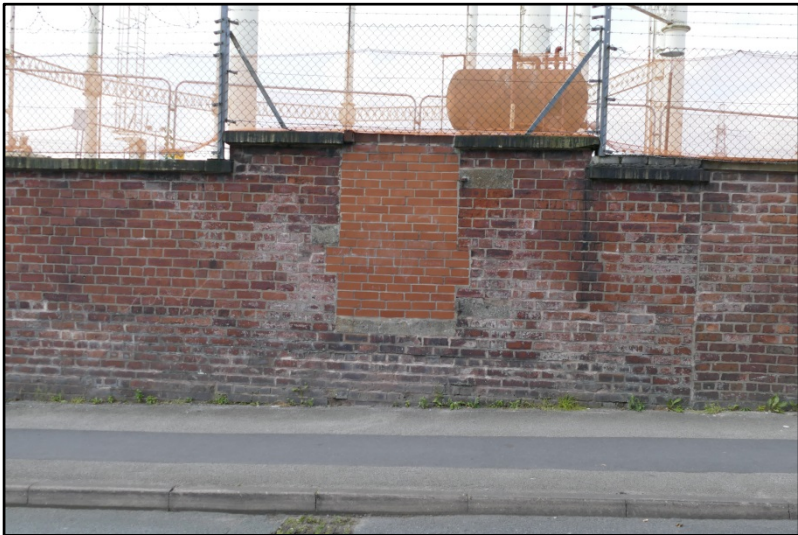
Modern blocking in the boundary wall Fig 15
