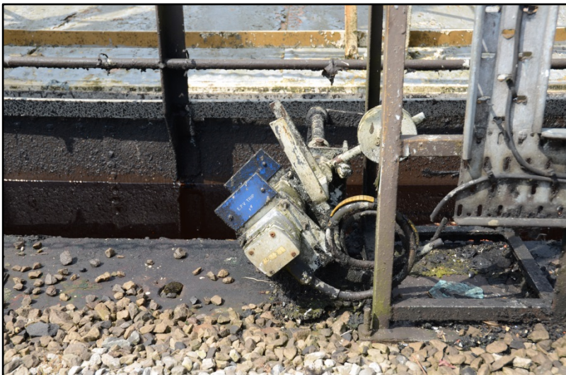
Detail of gasholder fittings Fig 47
