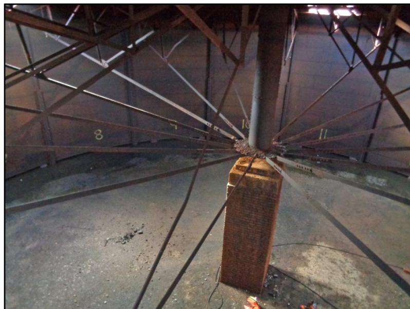
Interior of the gasholder, showing central stanchion and crown frame Fig 25
