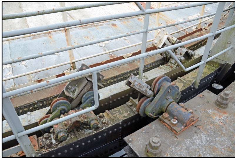
Detail of the lifts, railings and multiple roller carriages Fig 22
