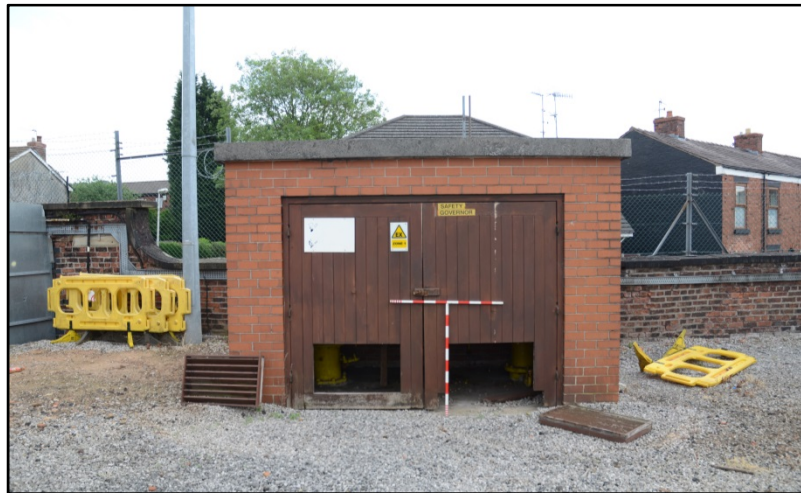
Safety governor room Fig 28
