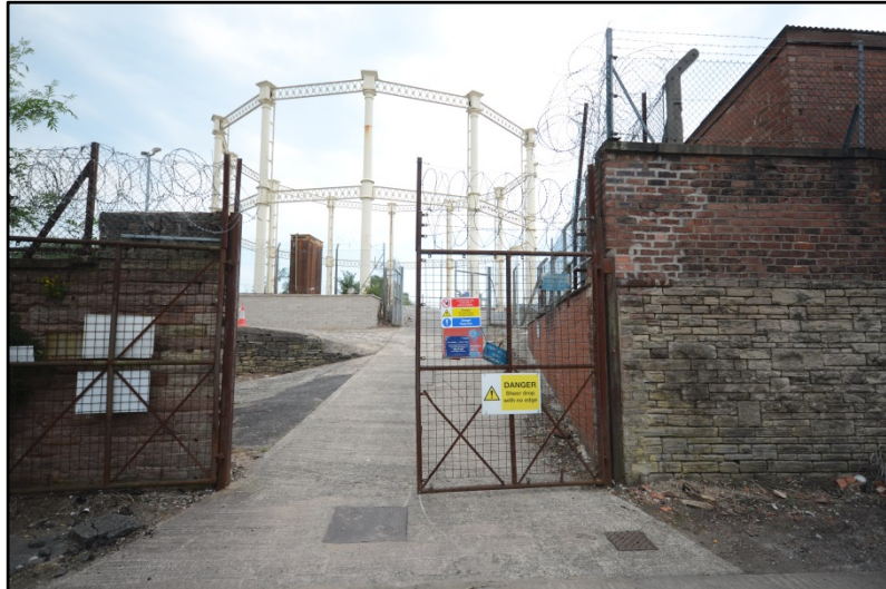
The Black Lane site entrance Fig 12
