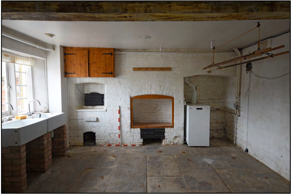
The outbuilding, ground floor, looking west Fig 12
