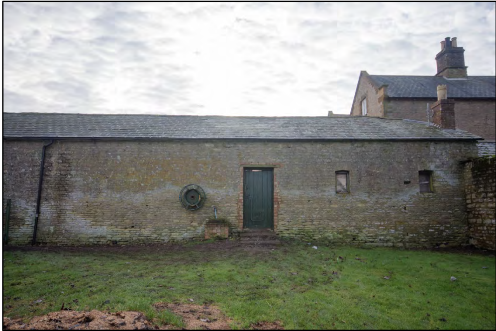
The western end of the north elevation Fig 27
