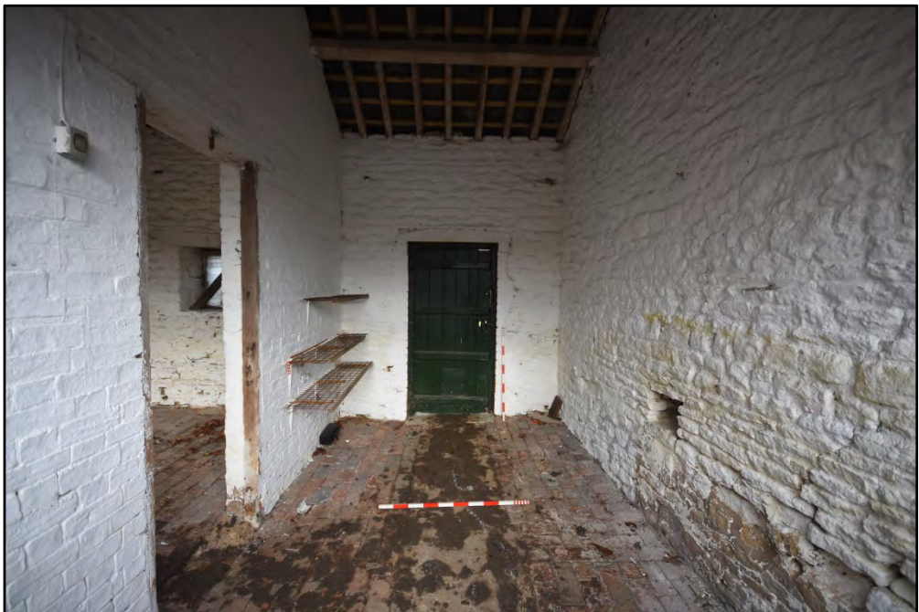
General view of room 3 Fig 32
