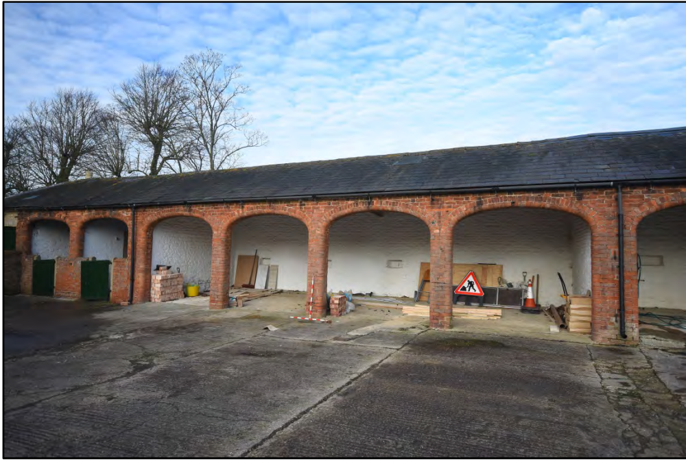
General view of room 4, looking north-west Fig 33
