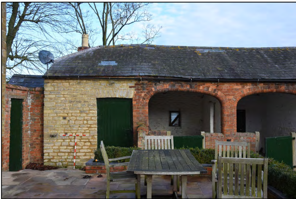
The west end of the Stables, looking north Fig 28
