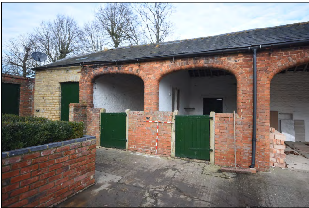
The semi-enclosed rooms at the west of the Stable range Fig 30
