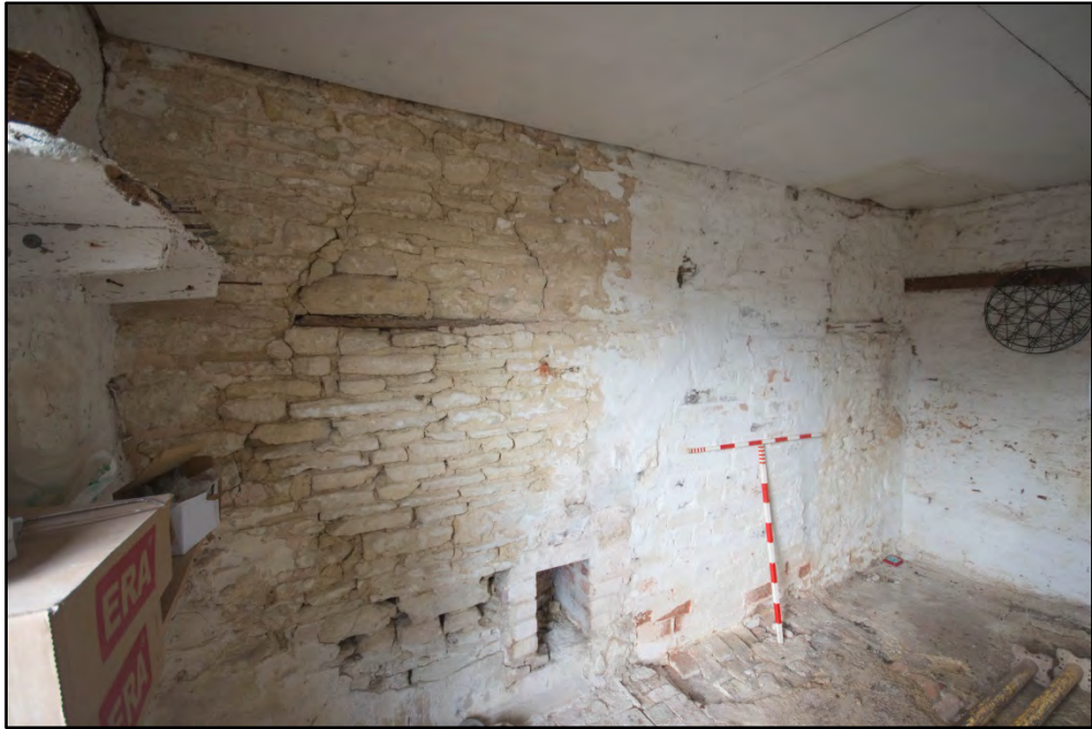
Room 1, showing blocked fireplace and adjacent flue Fig 29
