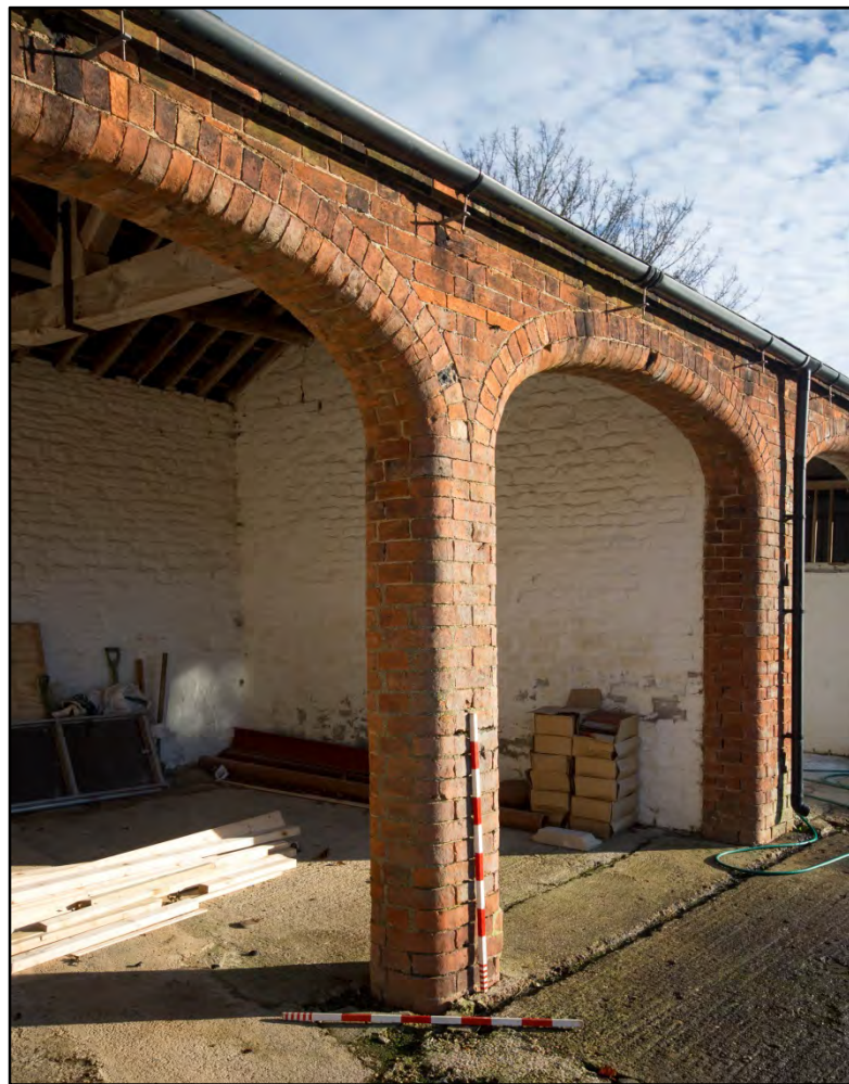
Detail of the brick columns and arched openings Fig 36
