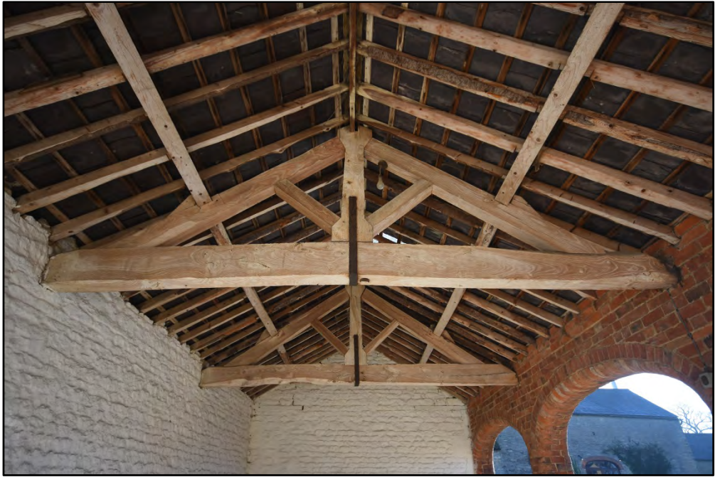
The king post trusses, looking east Fig 37
