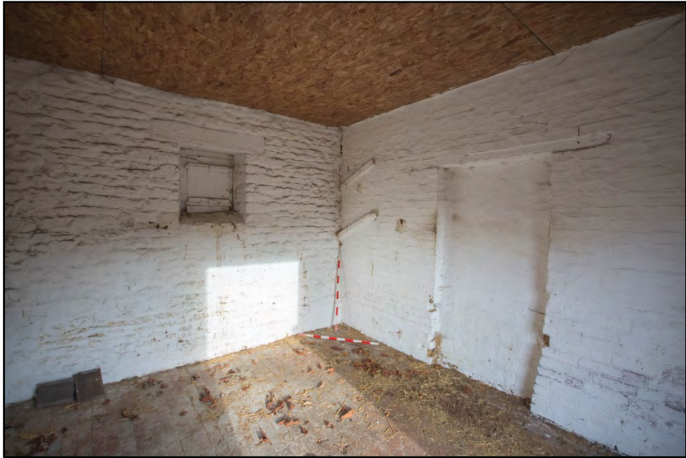
Room 9, showing blocked door to room 10 Fig 41
