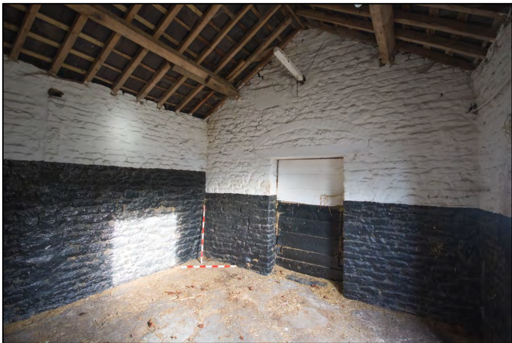
Room 10, showing blocked door to the eastern range Fig 42
