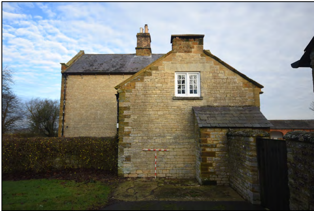
The south elevation of the outbuilding Fig 9
