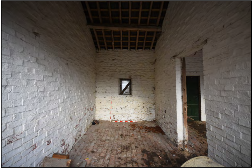
General view of room 2 Fig 31
