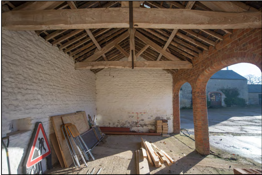
Room 4, looking east Fig 35
