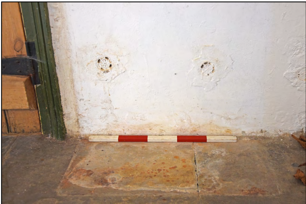
Detail of inserted vents in the north wall Fig 19
