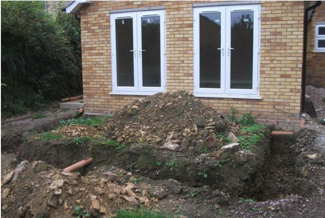
Trenches 1-3 and west elevation of Newhaven, looking north-east Fig 3
