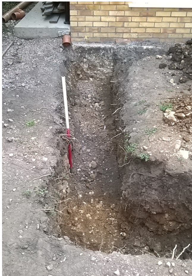
Trench 1, prior to excavation of skeleton, looking east Fig 4
