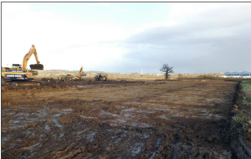
The SMS area during excavation, looking east Fig 10
