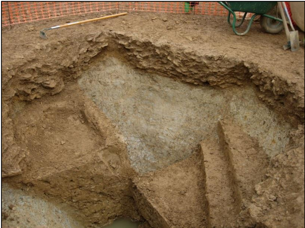
The hard cap rock overlying soft clay Fig 5
