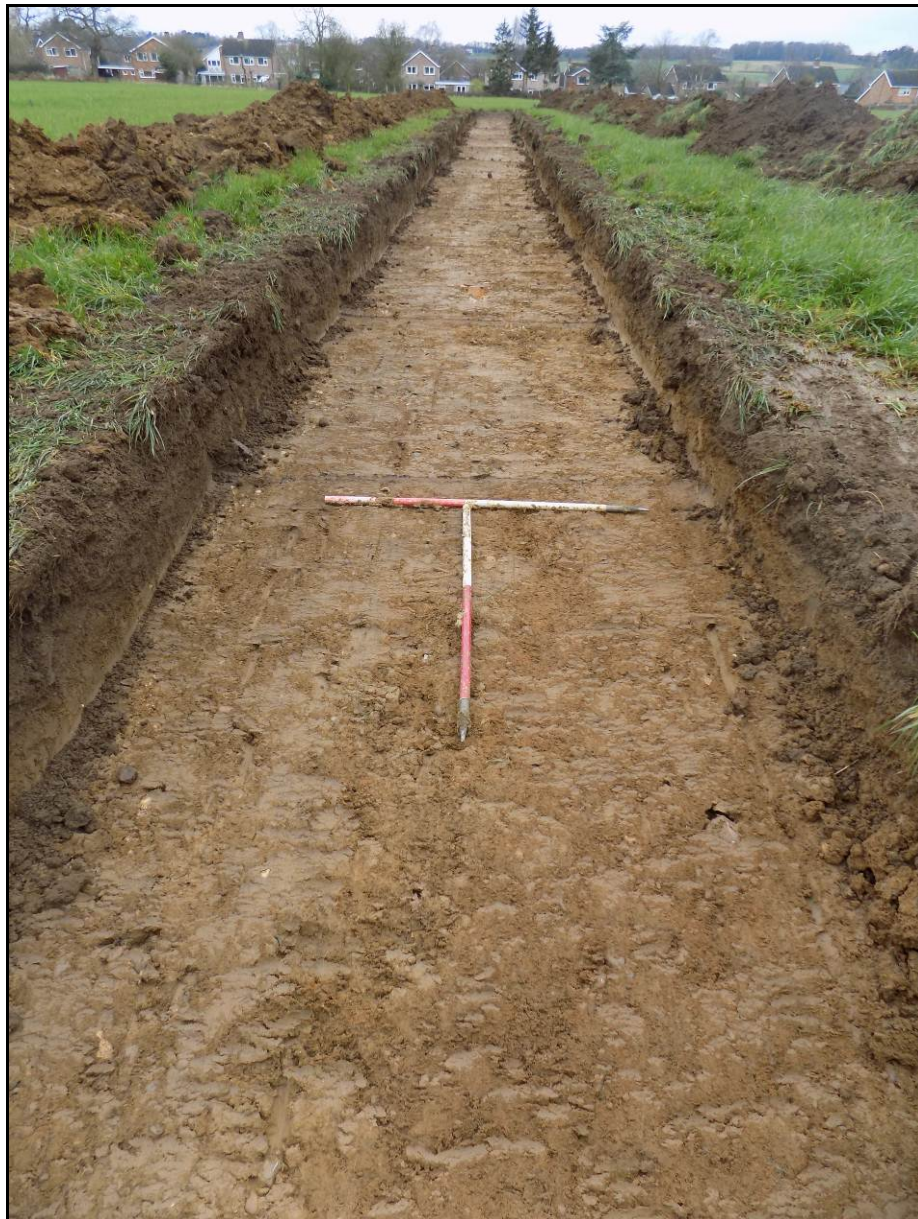
Trench 11 looking north-west (scales 2x 1m) Fig 14
