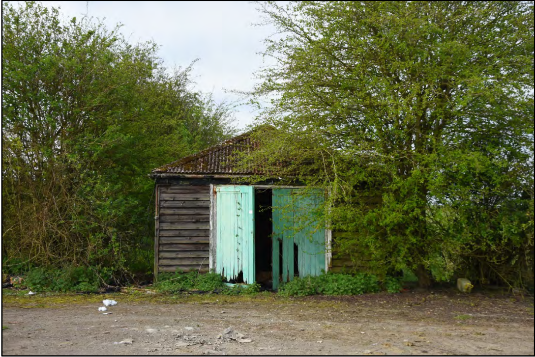
The Shed, looking west Fig 67
