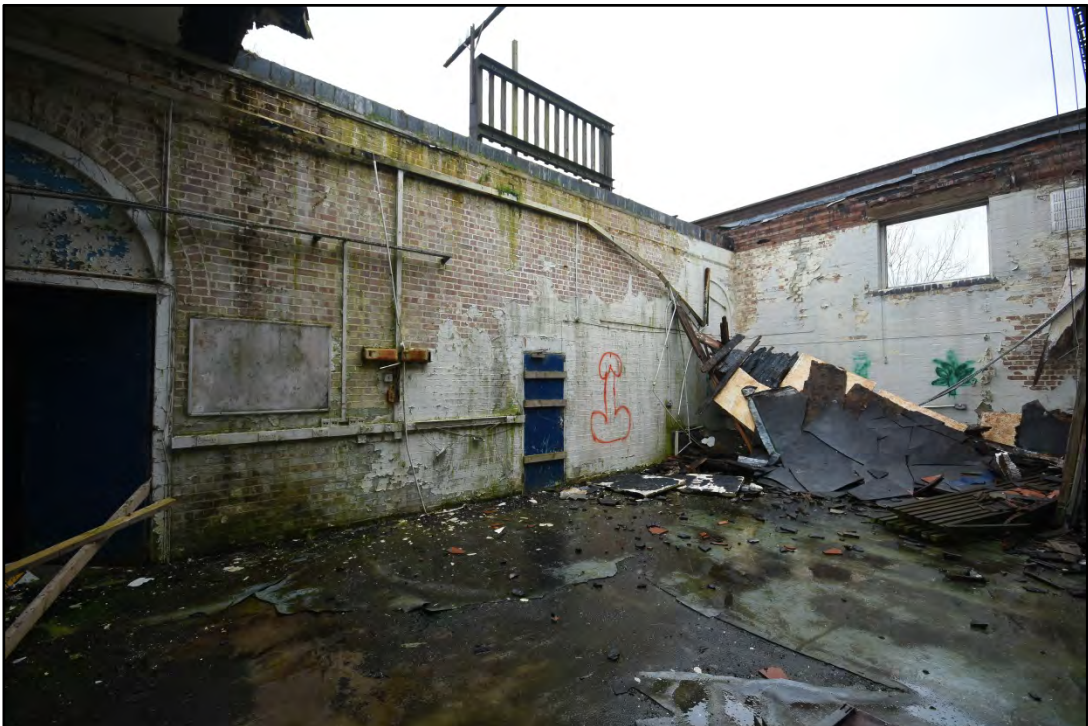
The Apparatus Room, looking north Fig 62
