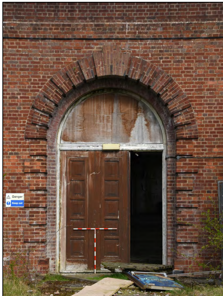
Door to the Machine Room, south elevation Fig 22
