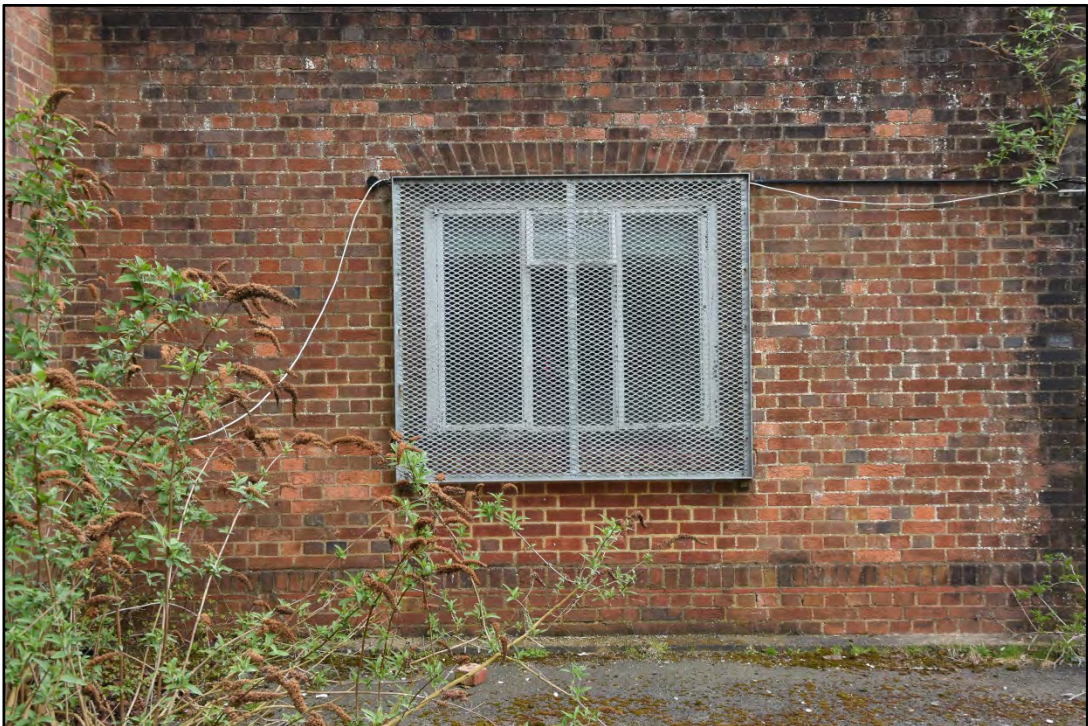
Former transformer room door, converted to a window Fig 30
