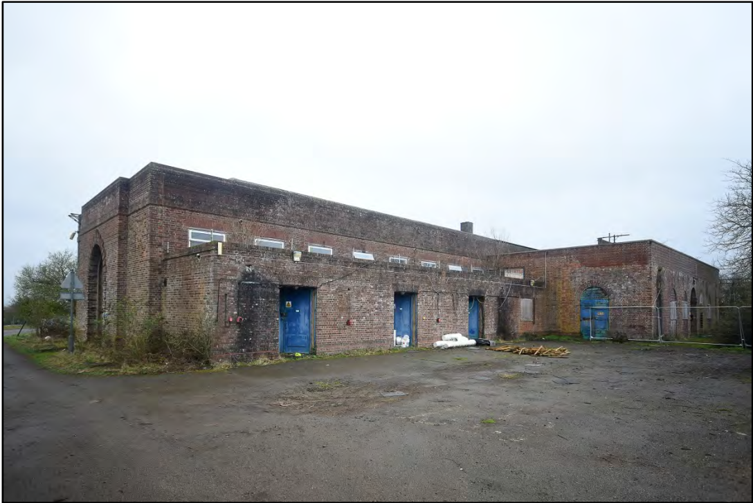
The west range, looking south-east Fig 33
