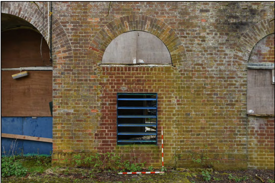
Blocked doorway Fig 32
