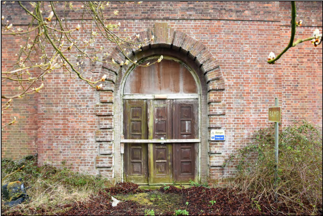
The south door to the Transmitting Room Fig 27
