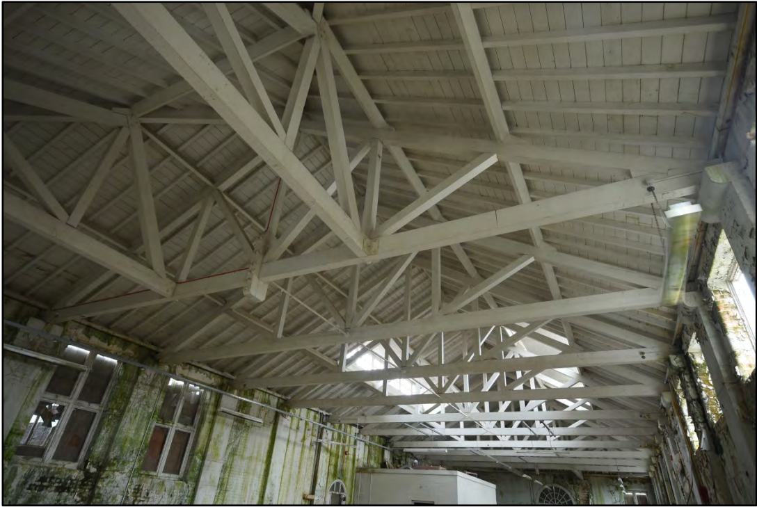
The roof structure Fig 41
