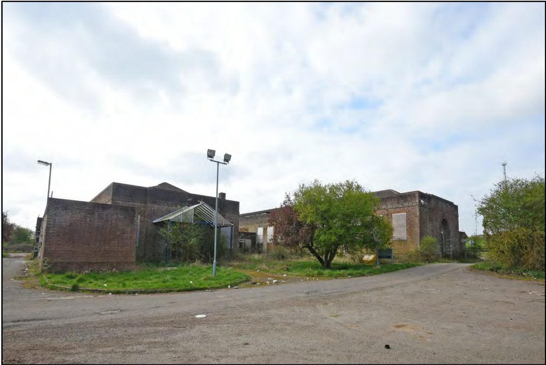
General view of the building, looking south Fig 37
