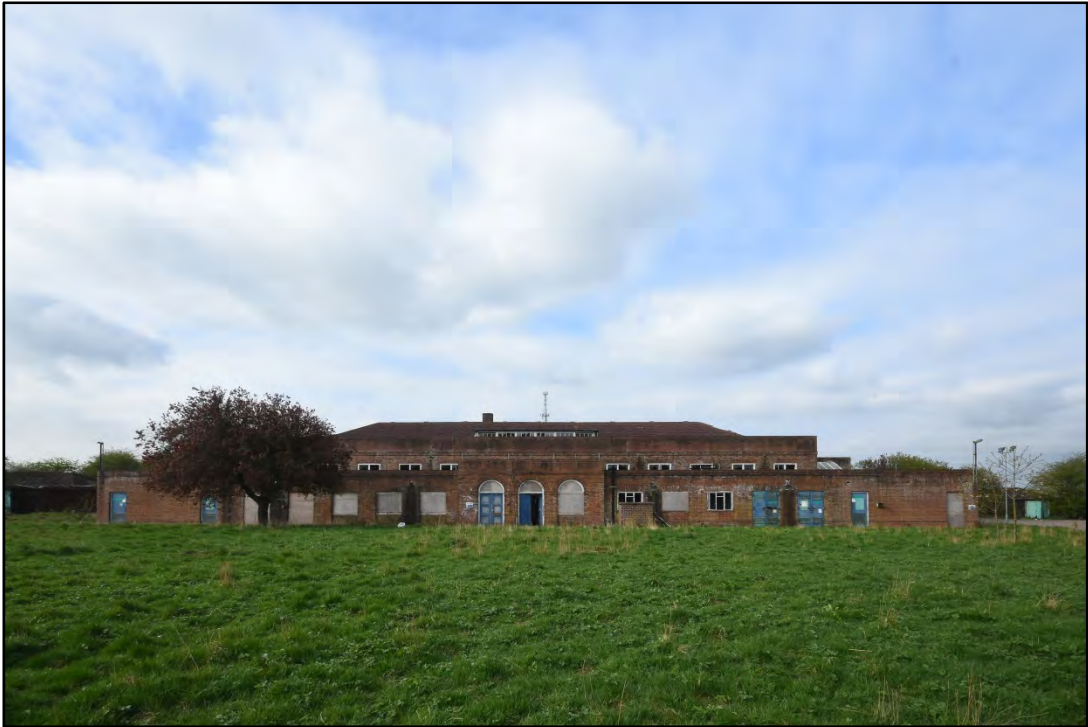
The north-east facing elevation, looking west Fig 15
