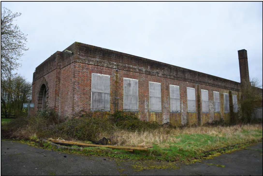
The south side of the western range Fig 26
