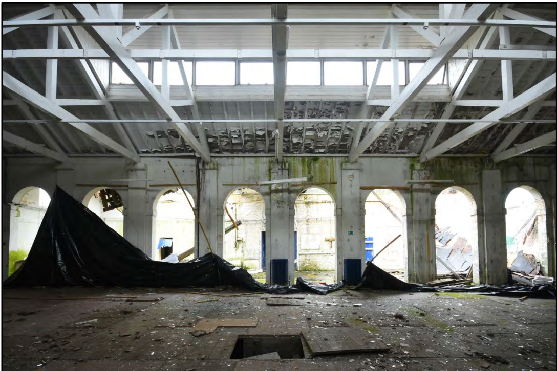
The arched openings to the Apparatus Room Fig 60
