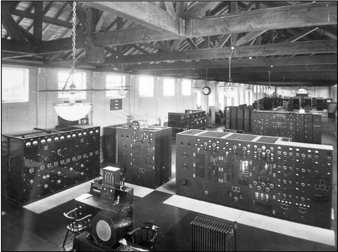
The Transmitting Room, dated 1934 (E8912) Fig 13
