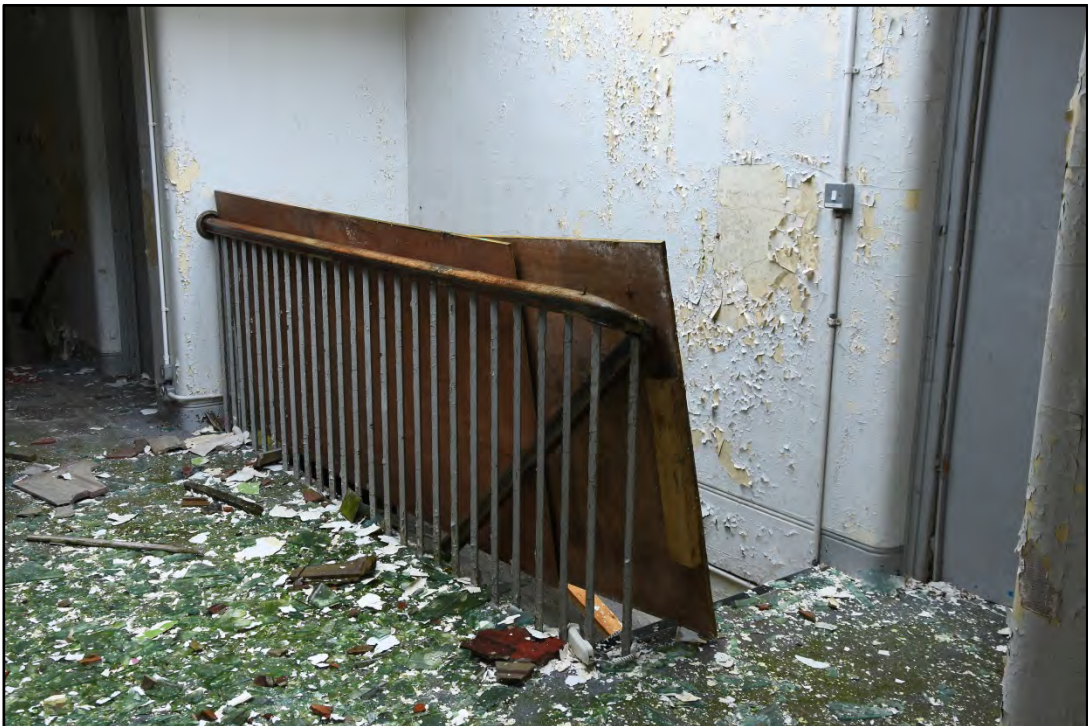
The basement stair Fig 52
