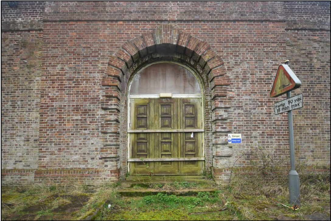
The north door to the Transmitting Room Fig 35
