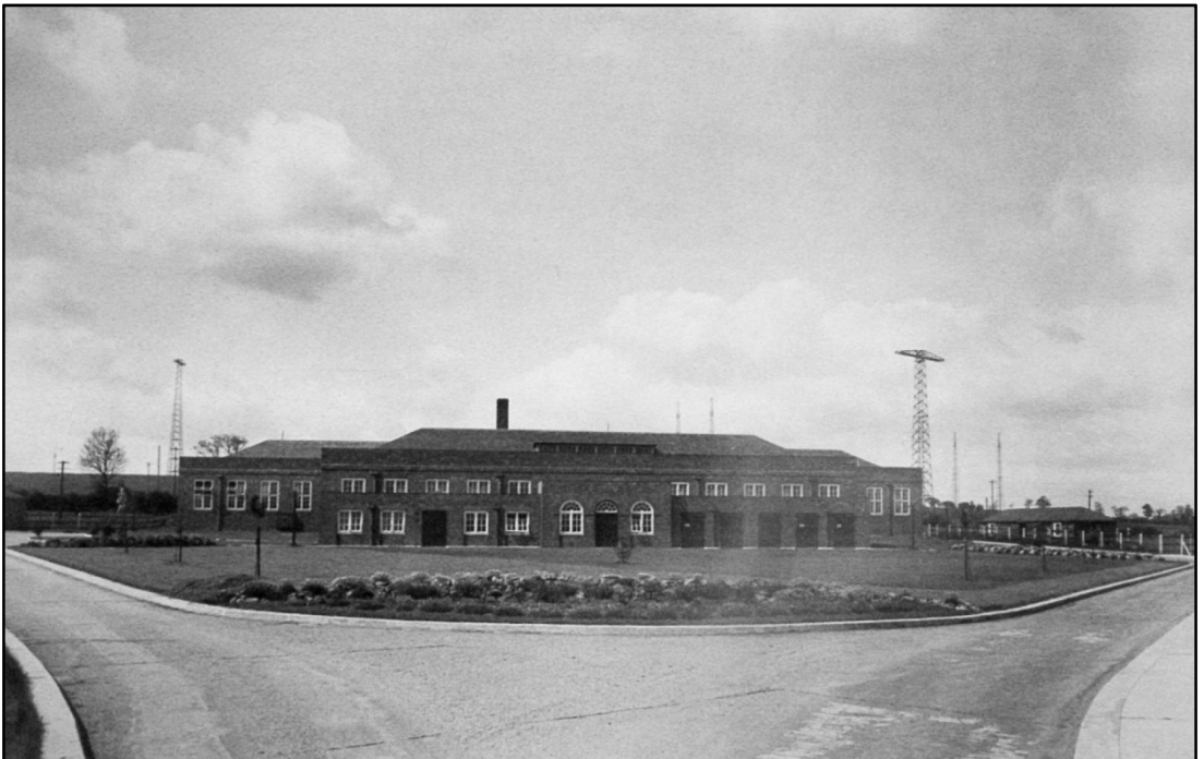
The main (north-east facing) elevation, dated 1934 (E8913) Fig 8
