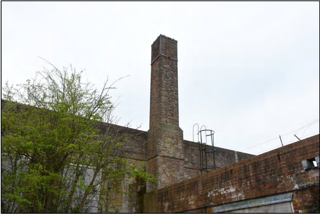
Chimney to the basement boiler room Fig 25
