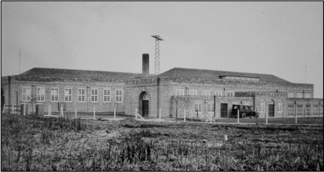
Building A, looking east, dated 1932 (E36) Fig 7
