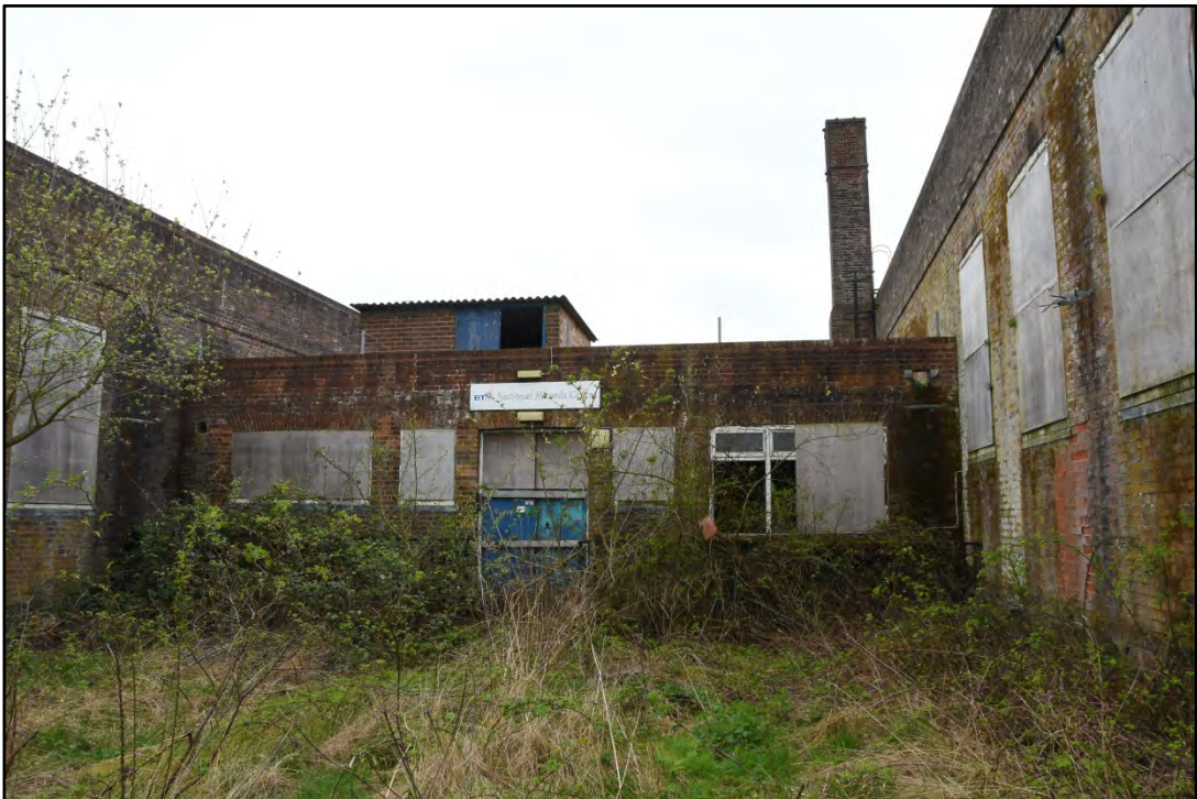
The central connecting block, looking south-east Fig 36
