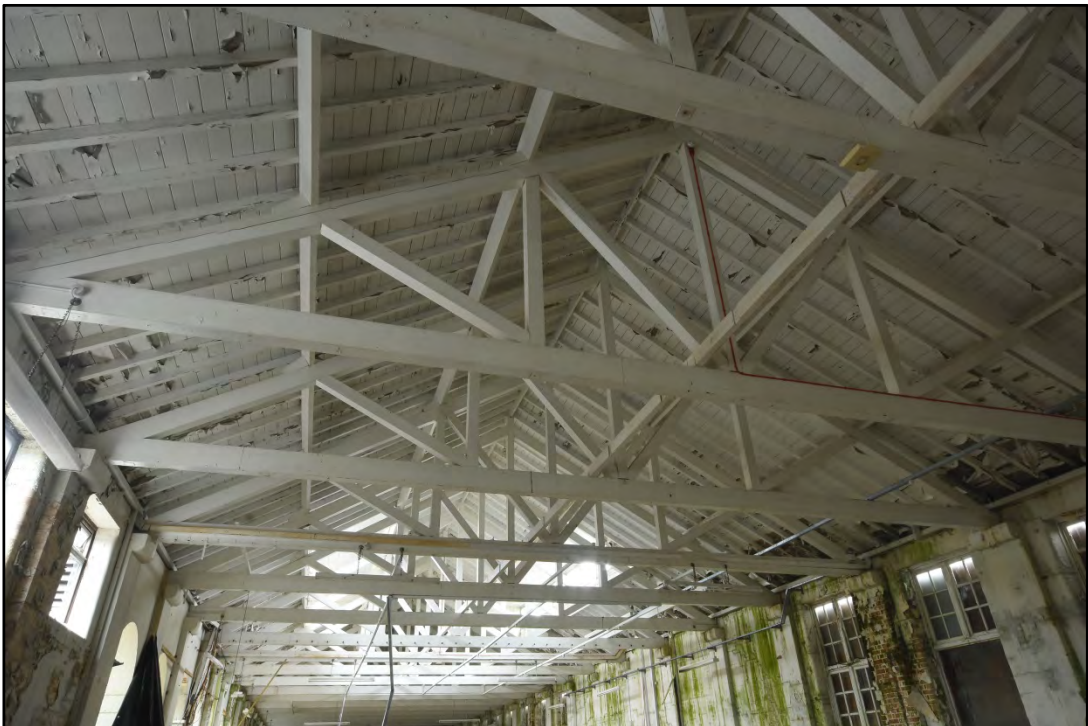
The roof structure Fig 58
