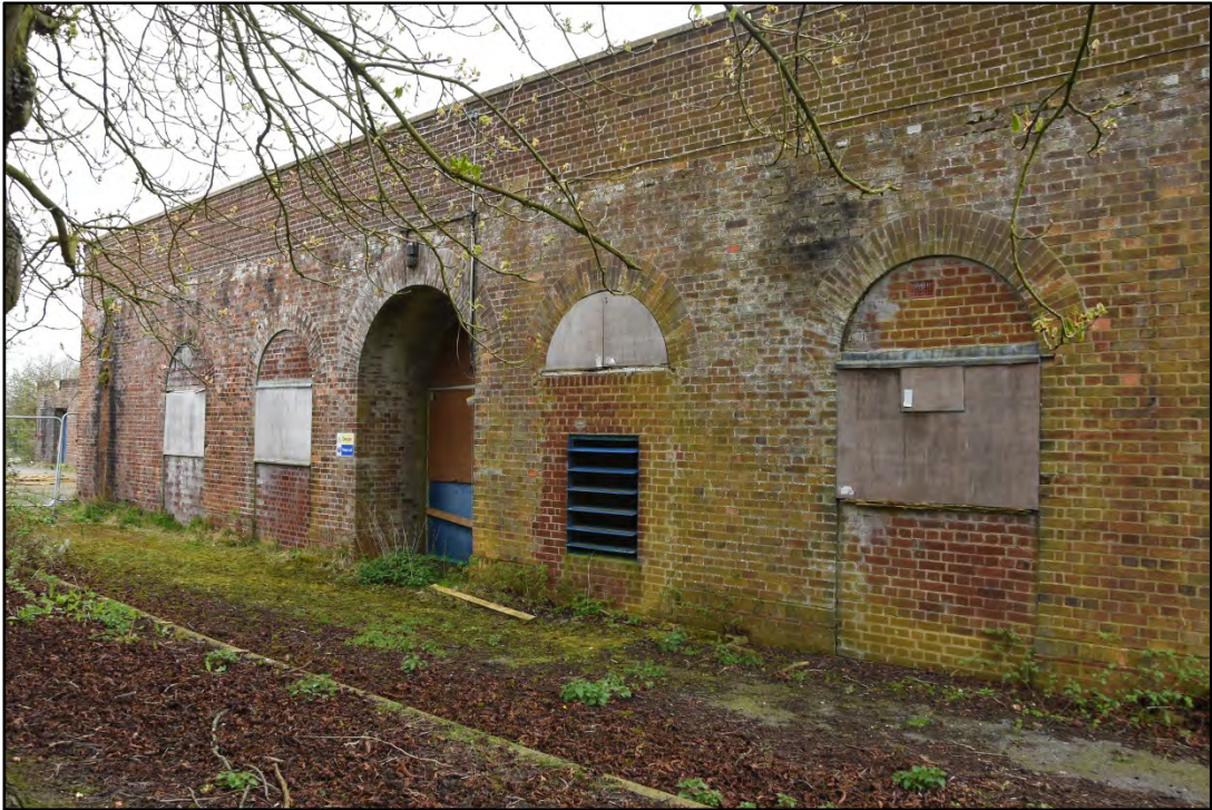
The central block of the west range, looking east Fig 31
