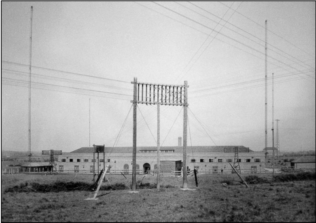
The south-west elevation, dated 1937 (E10106) Fig 9
