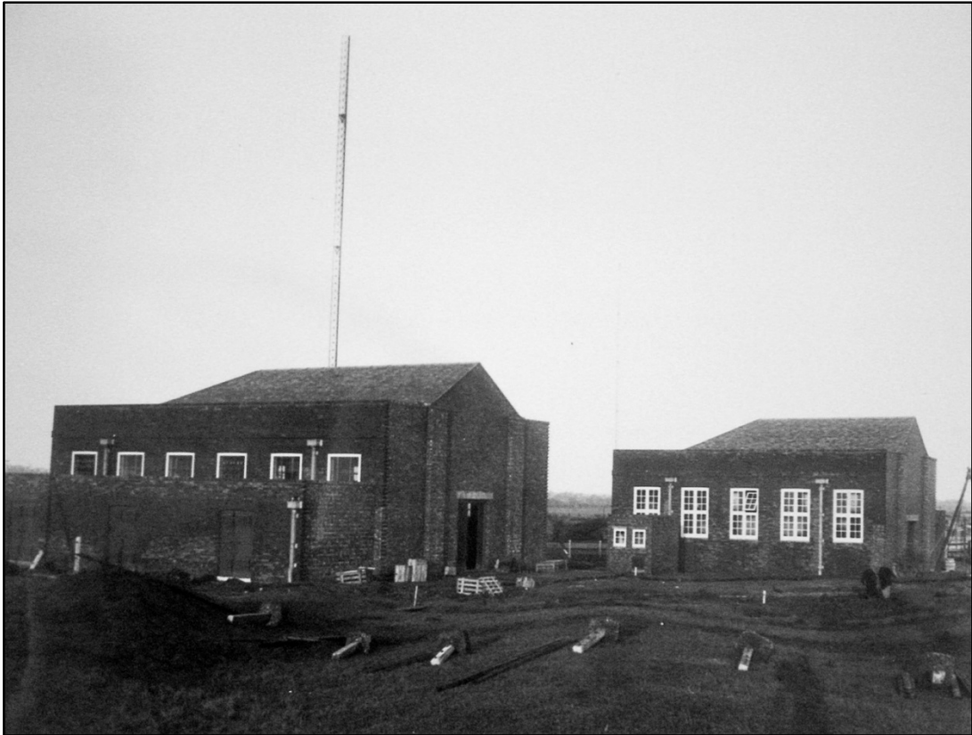
The building during its initial stages of construction, looking north-east, dated January 1930 (E6498) Fig 5
