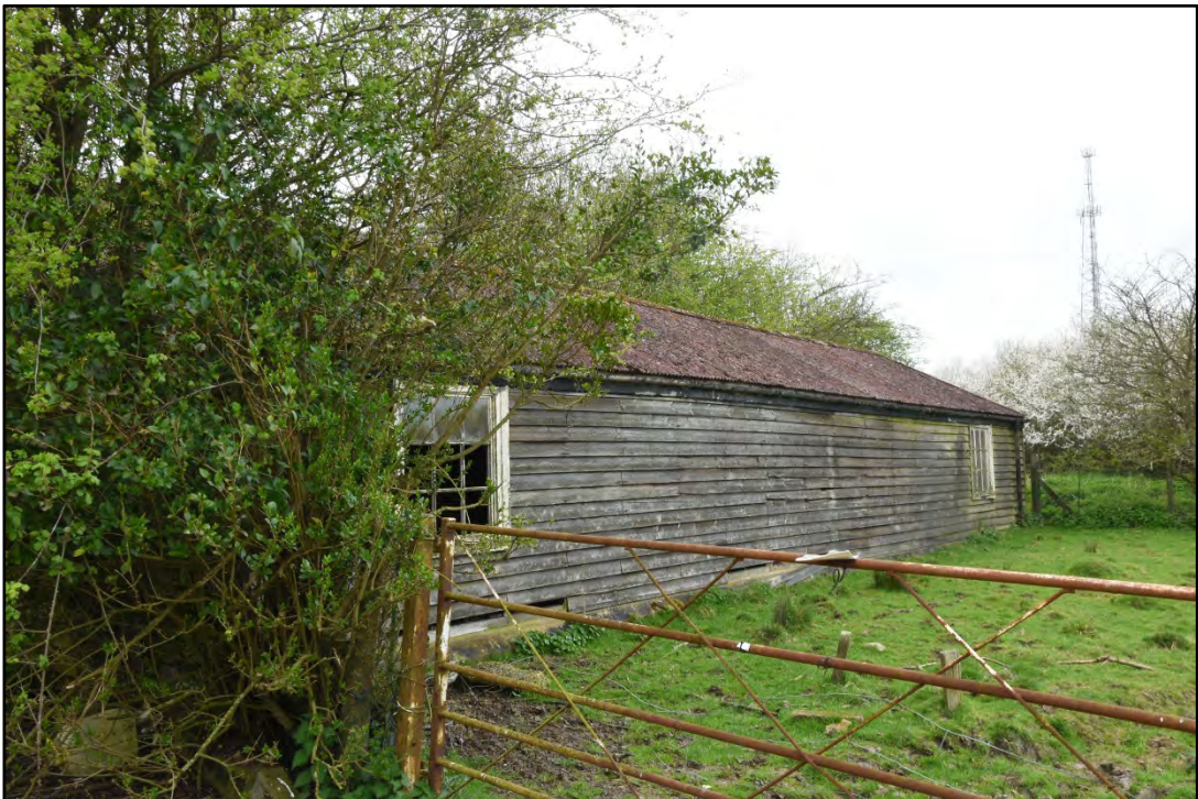
The north elevation of the Shed, looking south-west Fig 68
