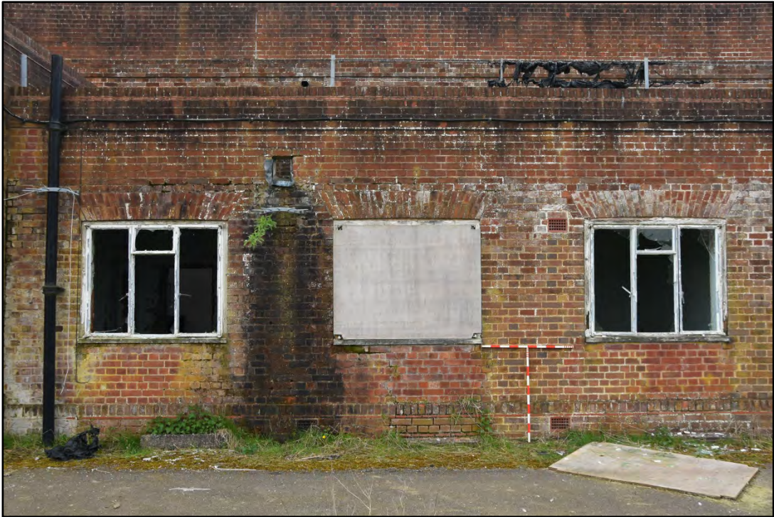
Former doorways converted to windows Fig 17
