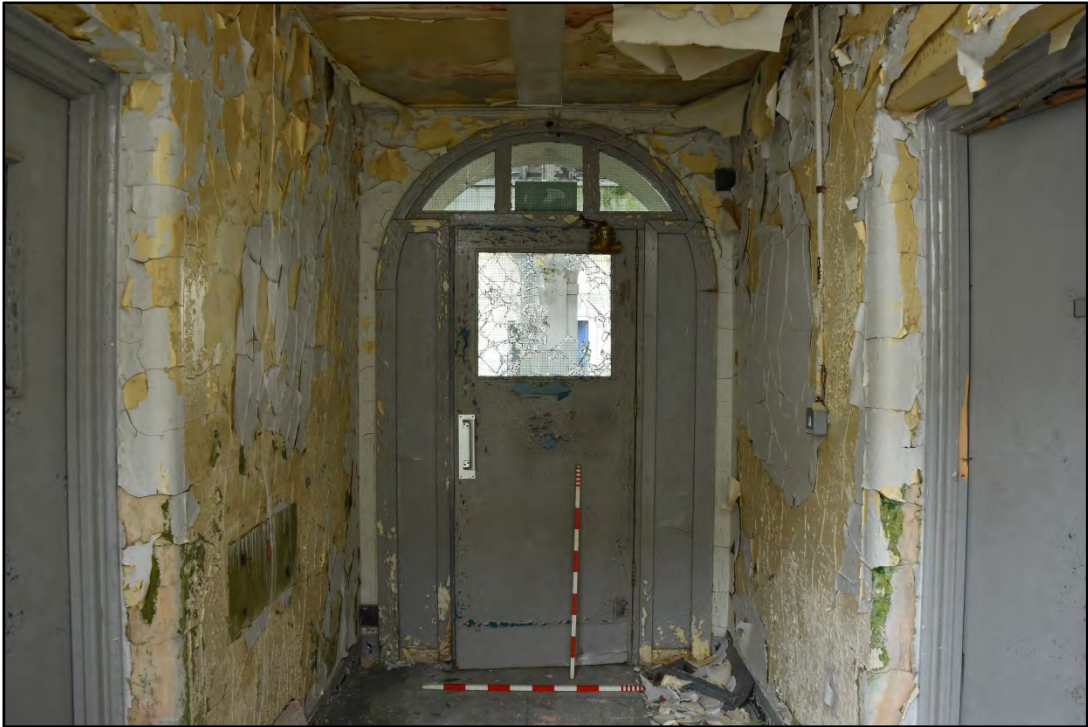
Door between the connecting block and the west range Fig 53
