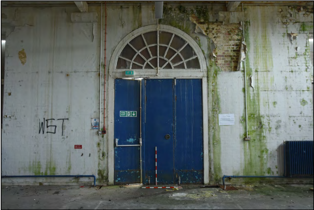
The north door of the east range Fig 43
