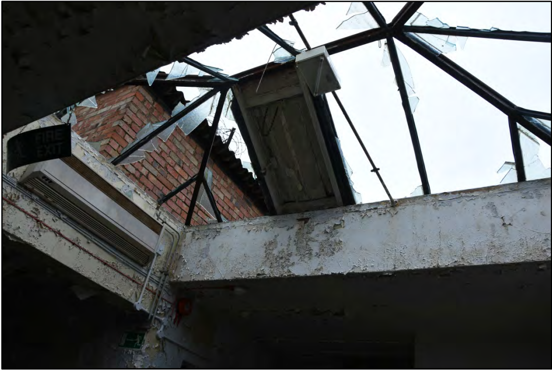
The central block roof-light Fig 51
