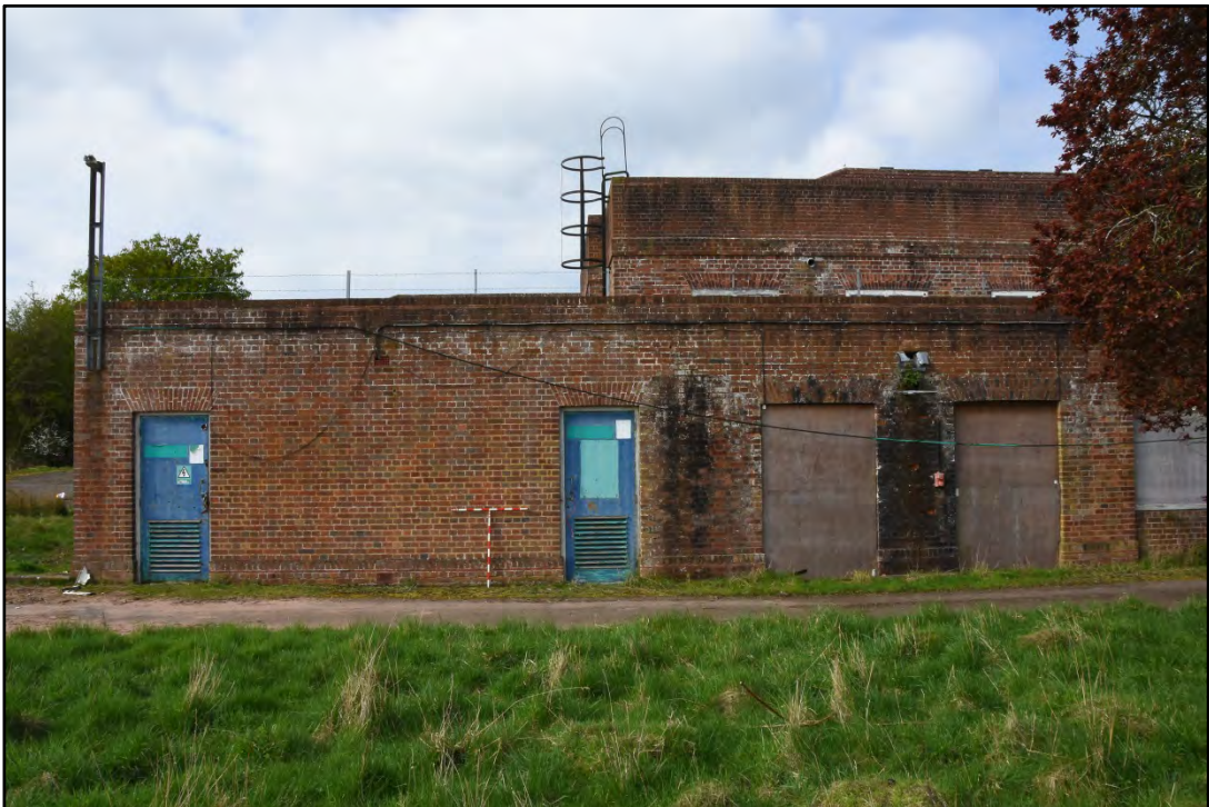
Doorways to transformer and switch rooms Fig 20
