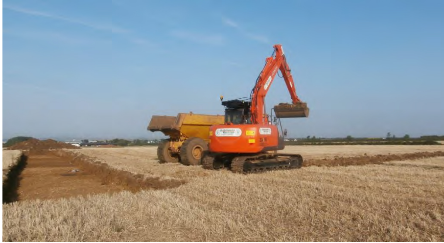
Excavation of Area 1 in progress, September 2014, looking north-west Fig 4
