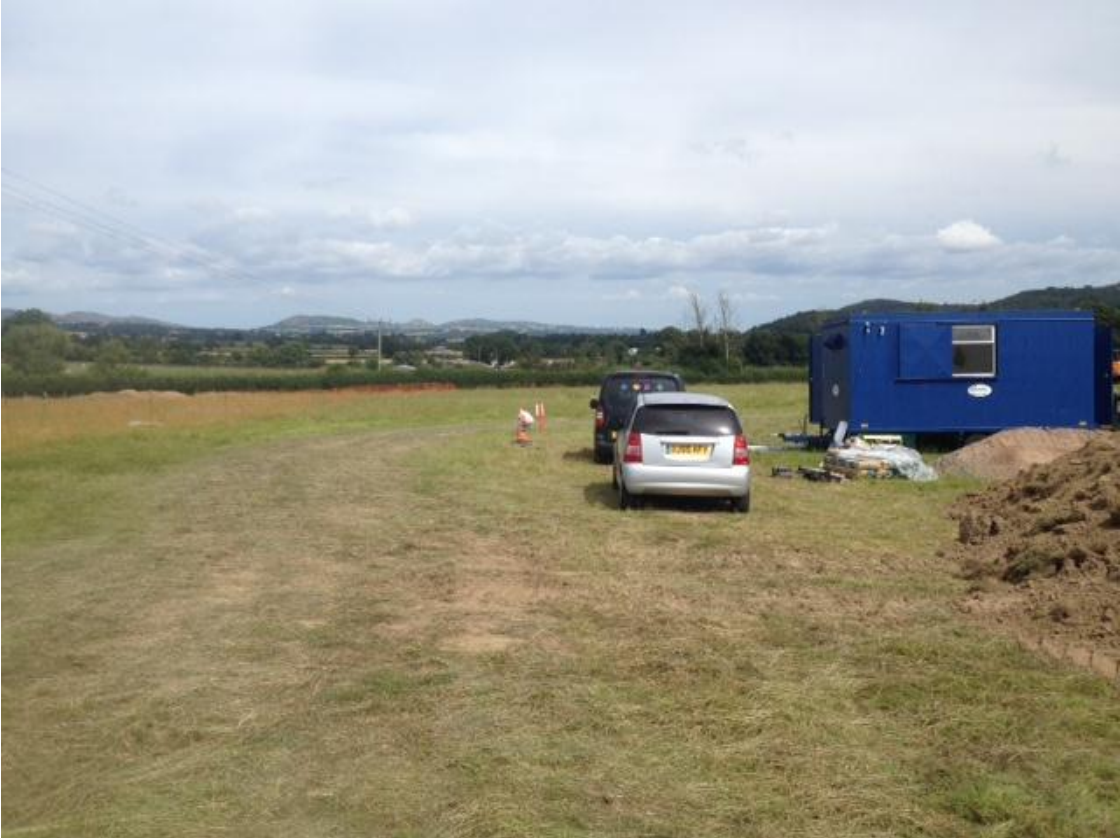
The investigation area prior to the start of groundworks, looking north Fig 3
