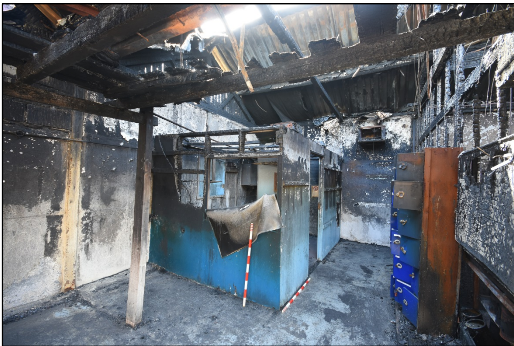
The small office in the south-east corner of the boathouse Fig 22
