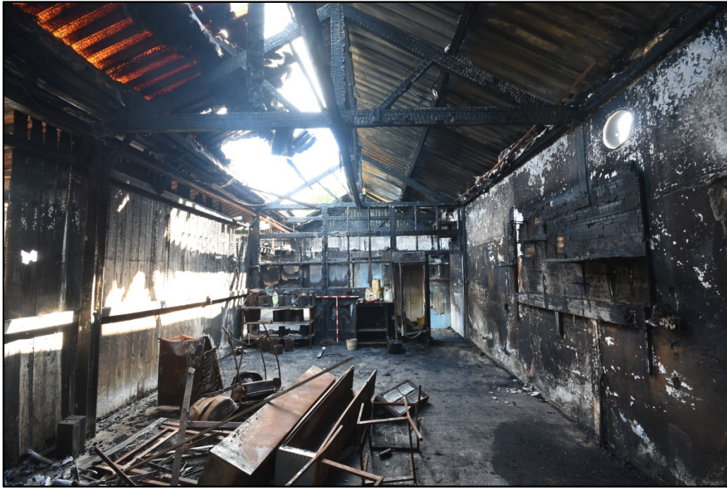
The maintenance room, looking east Fig 21
