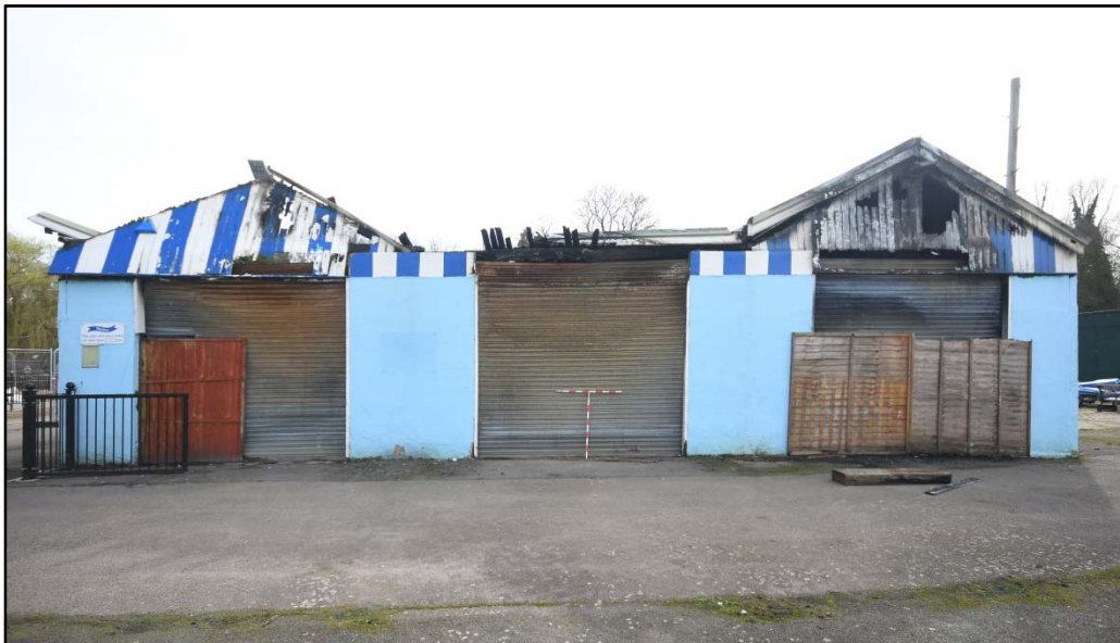
The west elevation Fig 8
