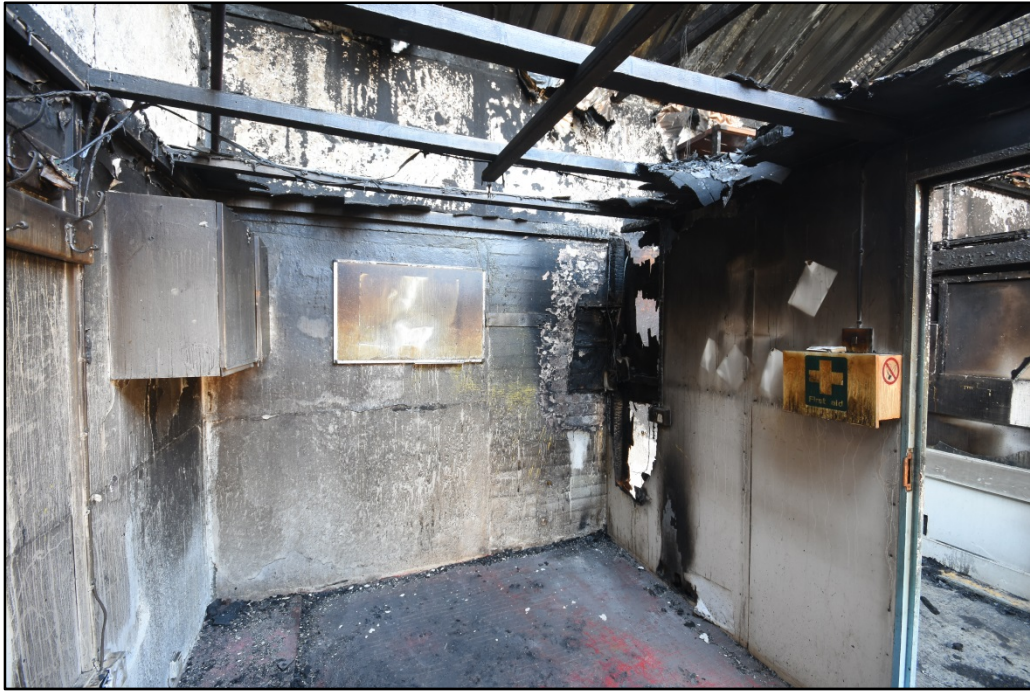
The interior of the small office room Fig 23
