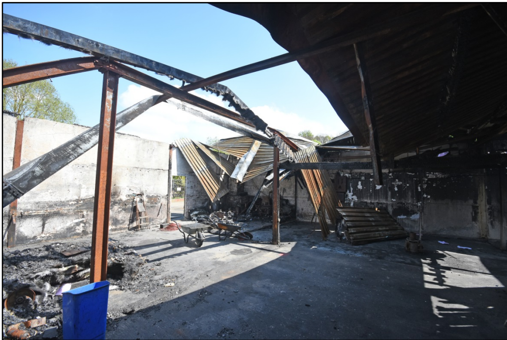
RSJs and beams supporting the roof valleys Fig 26
