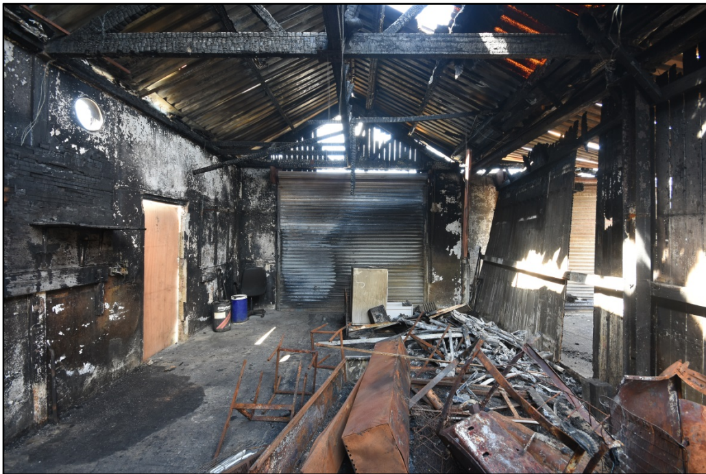
The maintenance room, looking west Fig 20
