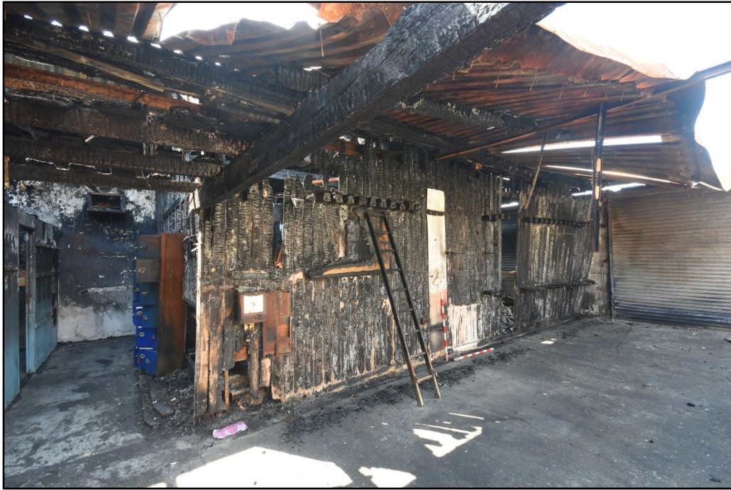
The north wall of the maintenance room, showing projecting supports Fig 19
