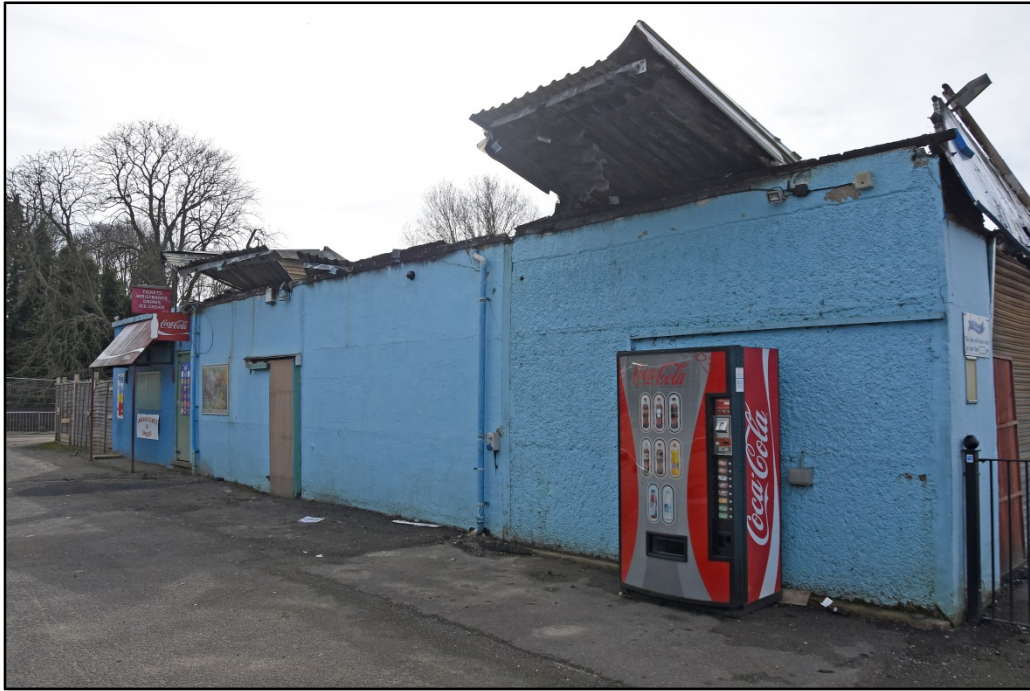
The north elevation, looking south-east Fig 13
