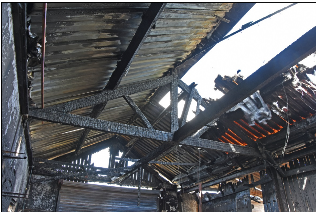
Detail of the roof trusses Fig 24
