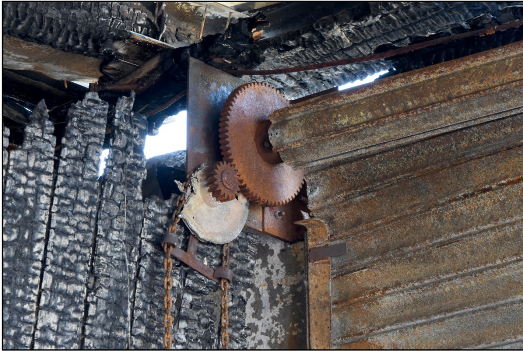
Detail of door roller mechanism Fig 17
