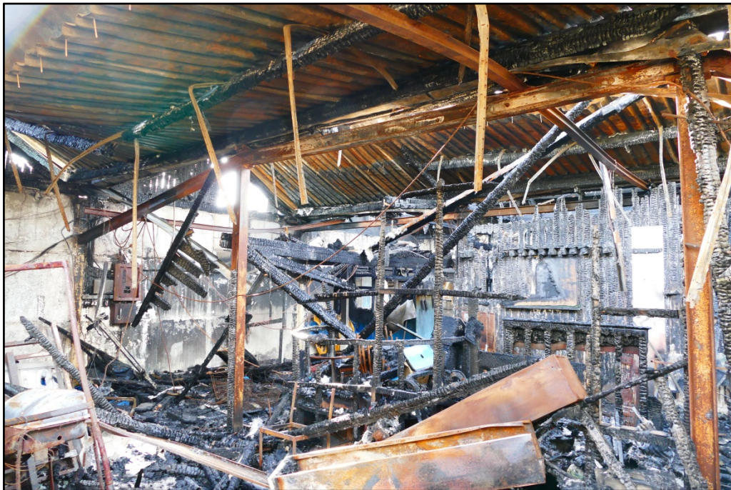
The interior, prior to clearing and making safe Fig 14
