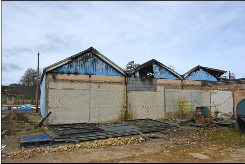
The east elevation, showing scars of former lean-to buildings Fig 11
