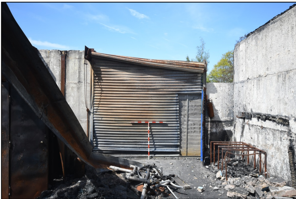
The north roller door Fig 16
