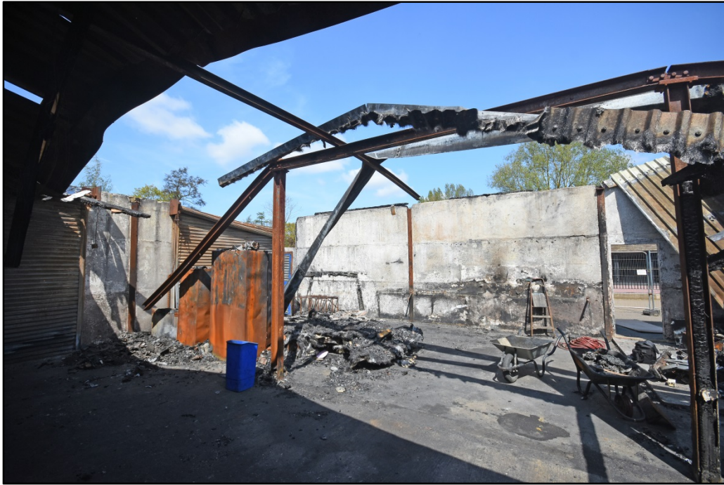
The interior, following clearing, looking north-west Fig 15
