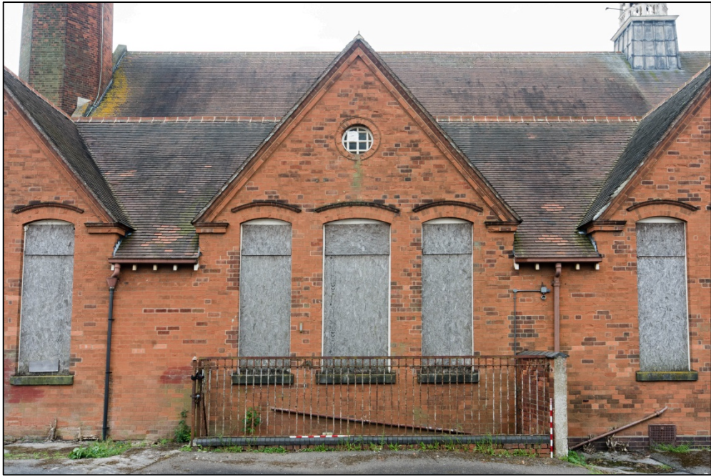
Classroom elevation with stairs to basement Fig 29
