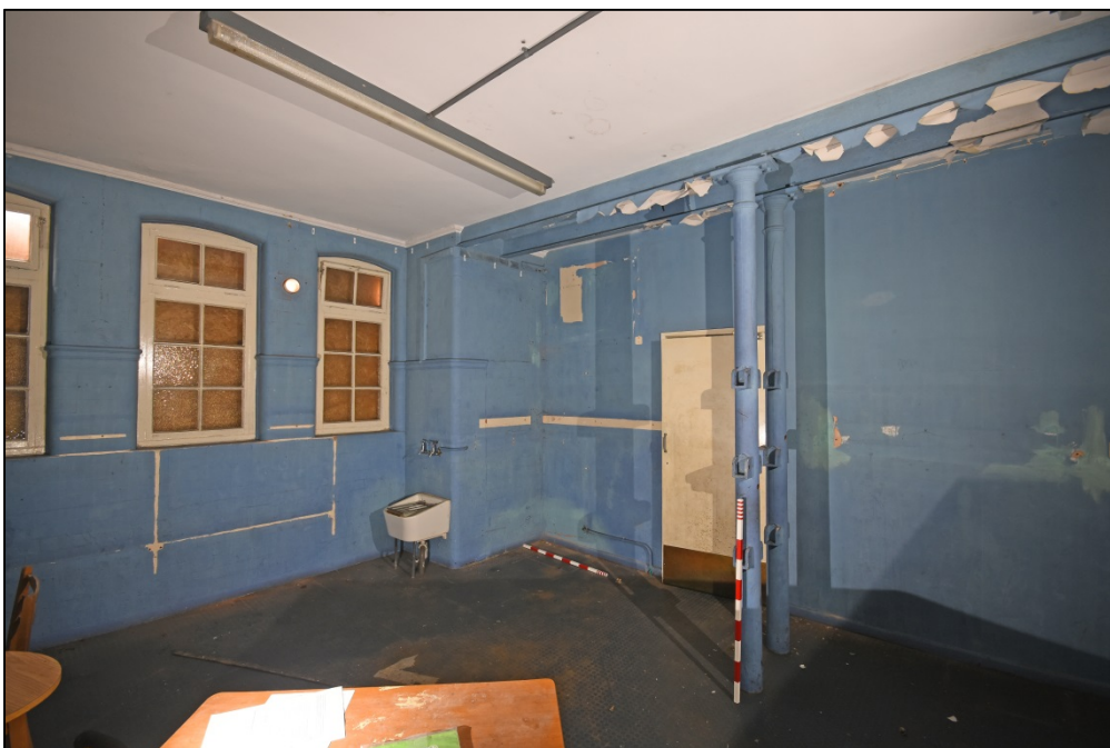
The boys' changing room, note columns supporting RSJs Fig 97
