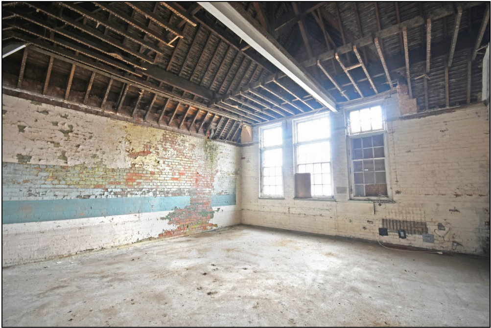
Classroom 7, looking north-west Fig 90
