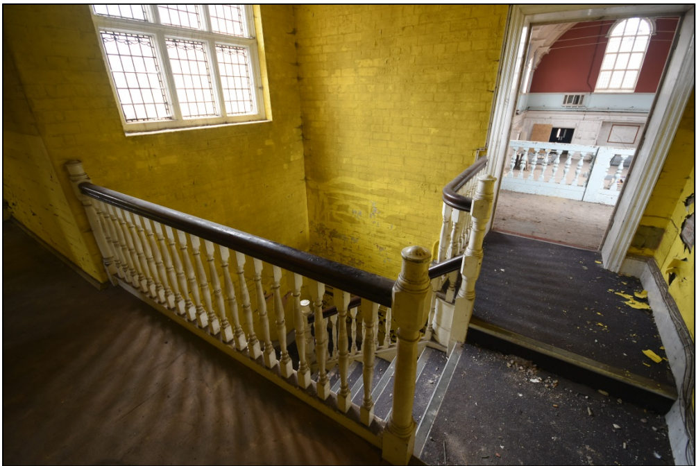
The stair landing, with door to balcony Fig 99
