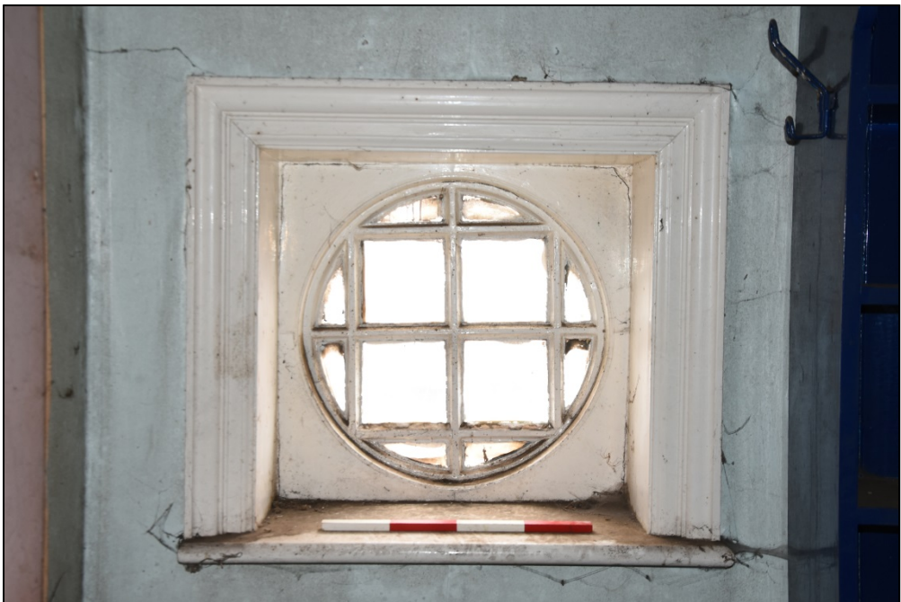
Internal face of round window of first floor office Fig 103
