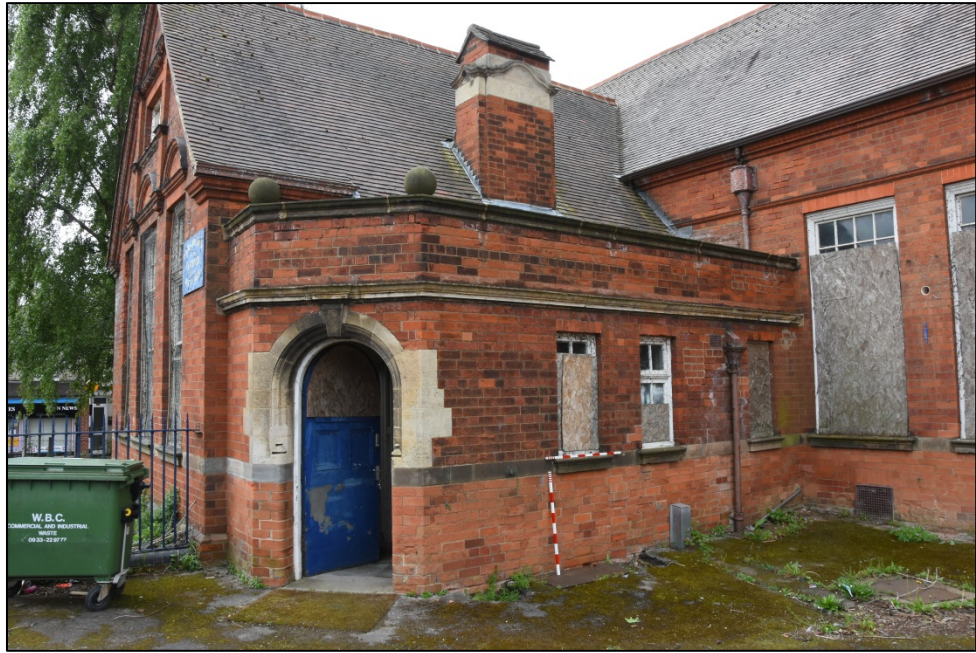
Porch and store adjacent to classroom 1 Fig 13
