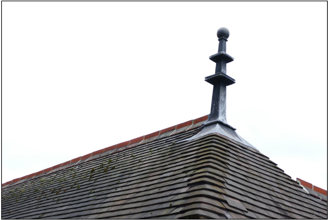
Detail of lead finial Fig 19
