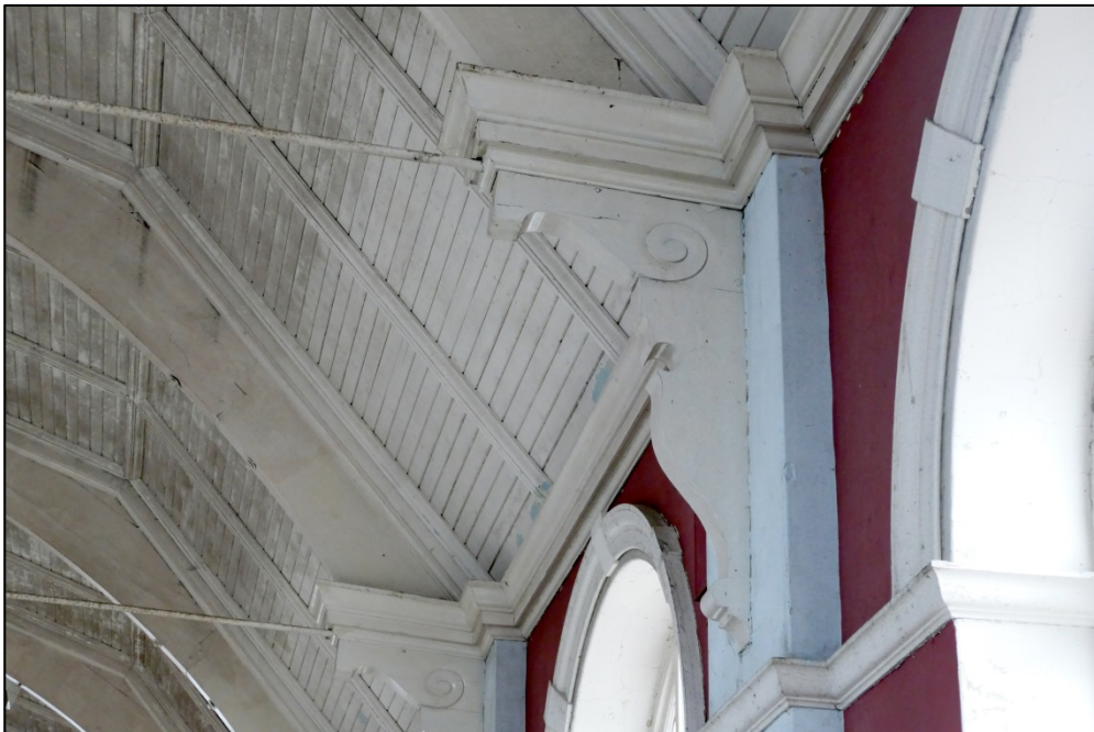
Detail of truss bracket Fig 65
