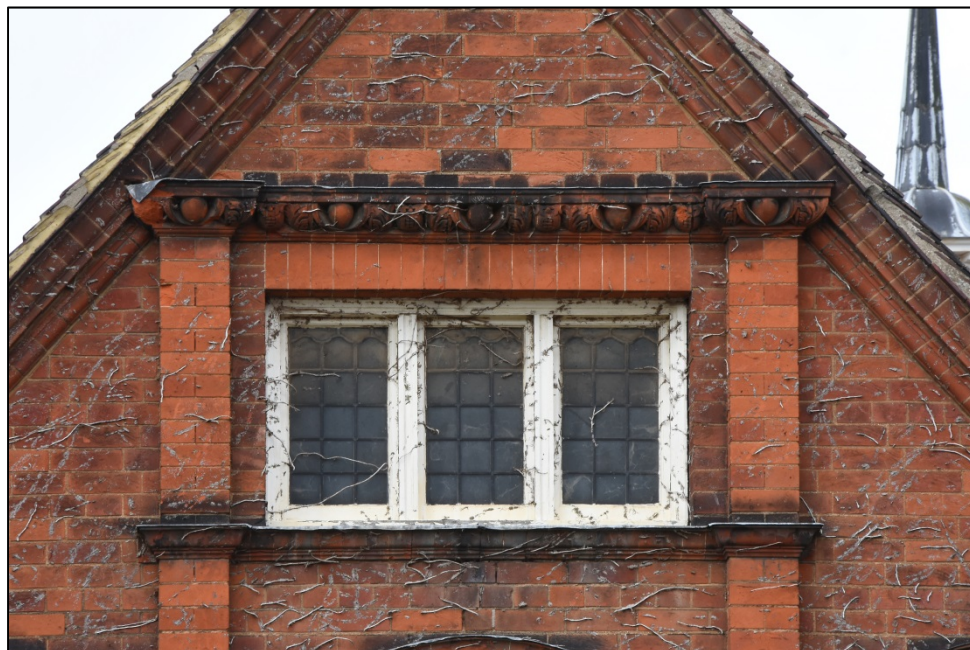
Detail of first floor window with egg and dart moulding Fig 12
