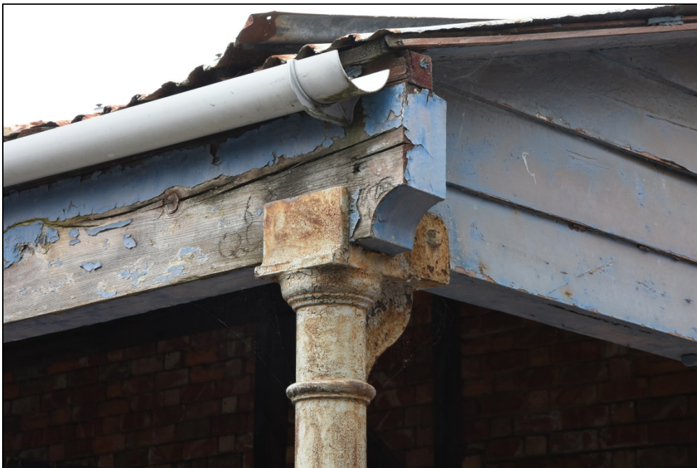
Detail of the column roof supports Fig 109
