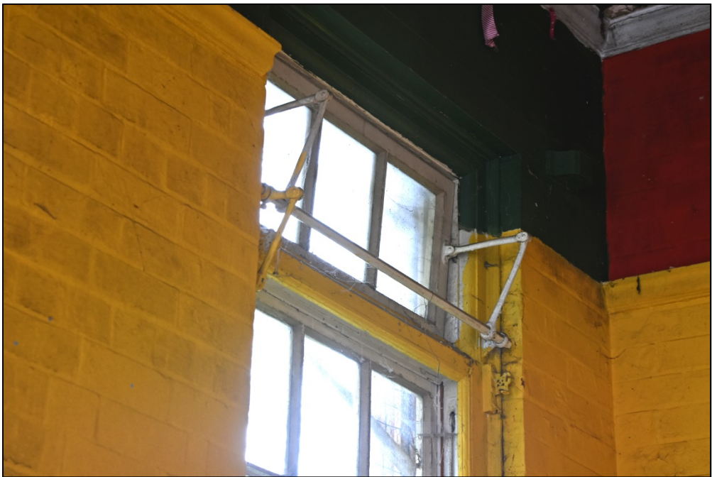
Detail of window pivoting arms Fig 39
