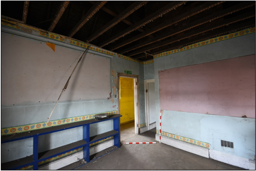
First floor office Fig 102
