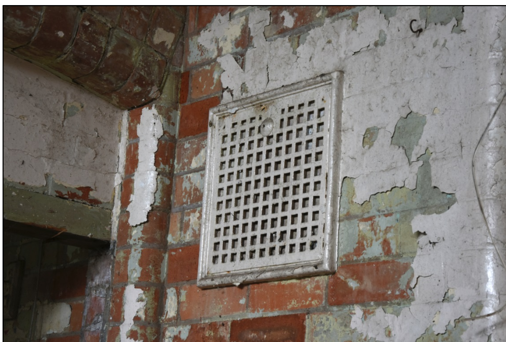
Detail of vent cover adjacent to doorway, classroom 3 Fig 79
