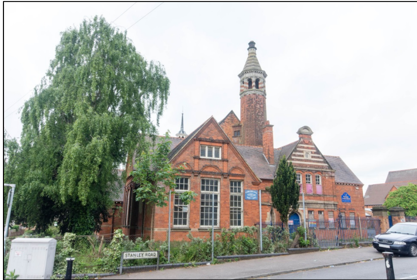
The Stanley Road elevation, looking west Fig 7
