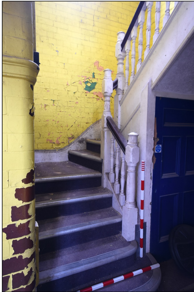
The stairwell Fig 45
