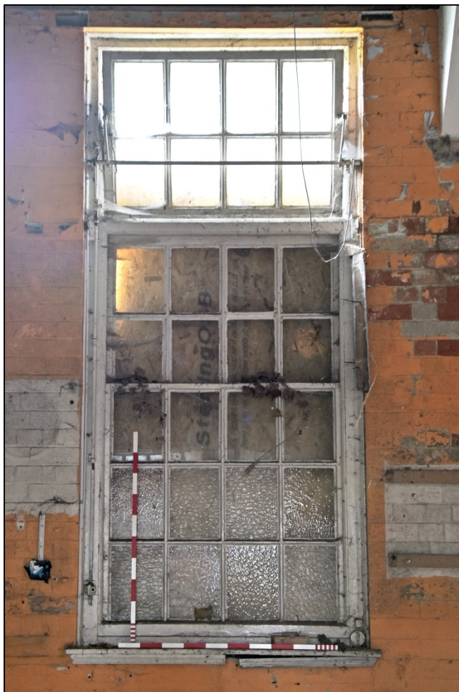
Detail of window, staff room Fig 84
