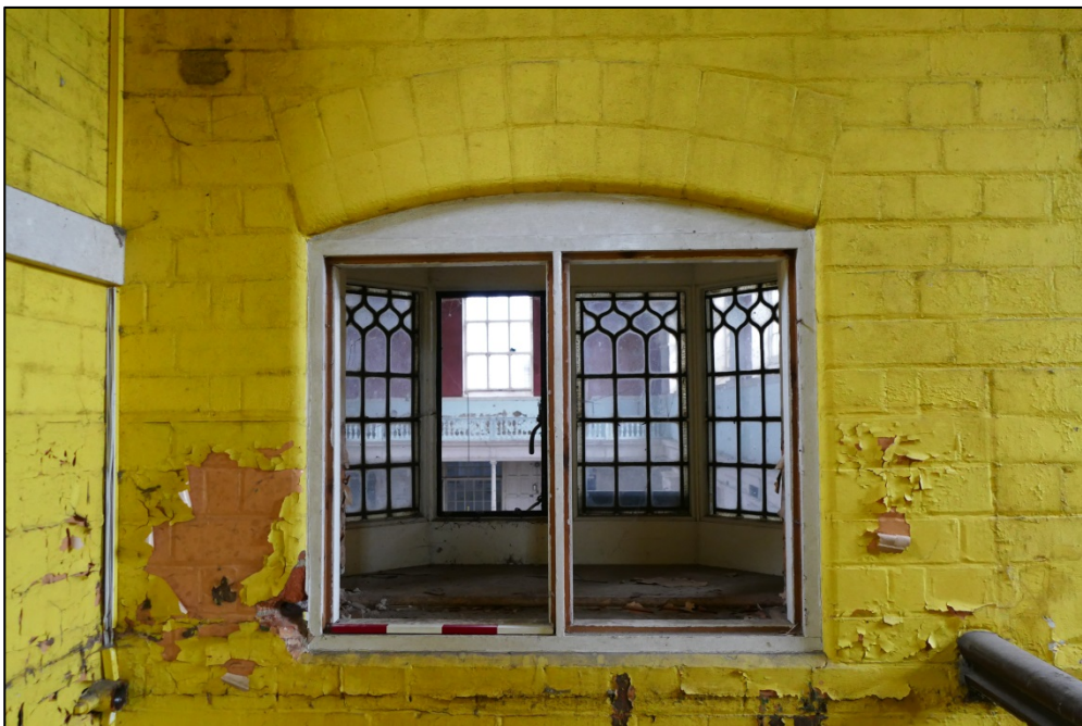
Interior view of oriel window at first floor landing Fig 47
