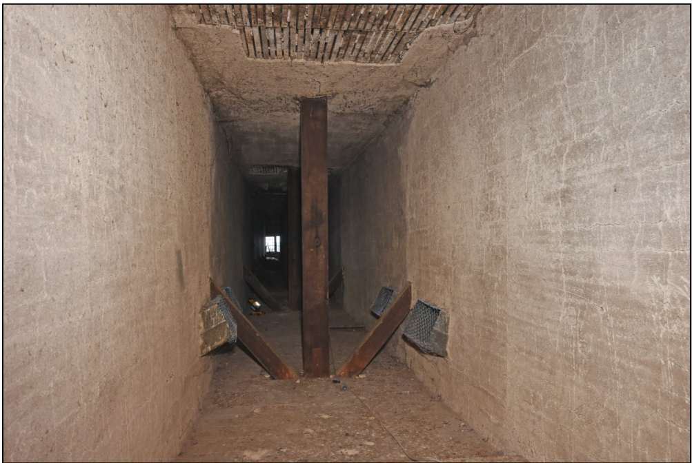
The hall roof walkway, looking east Fig 69
