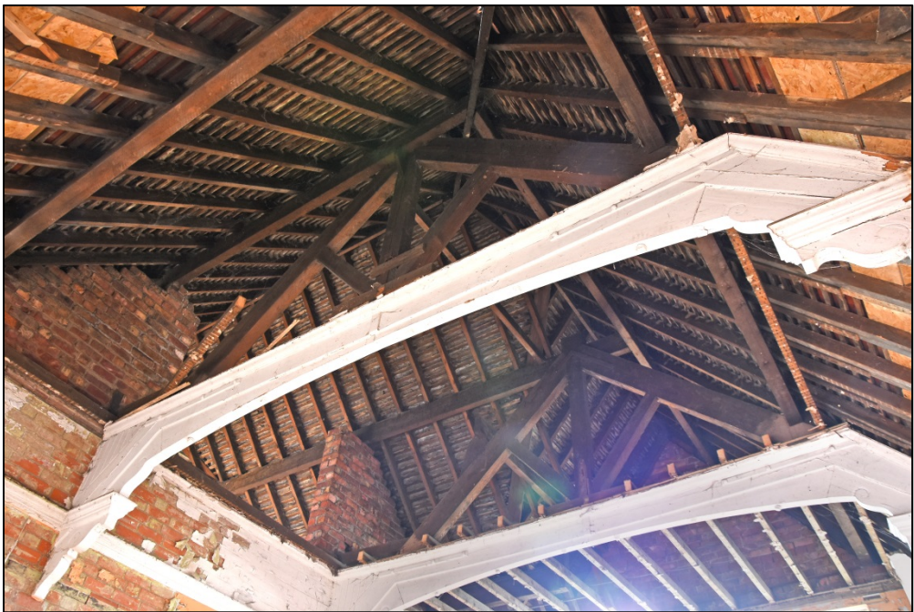
The roof structure over the staff room Fig 83
