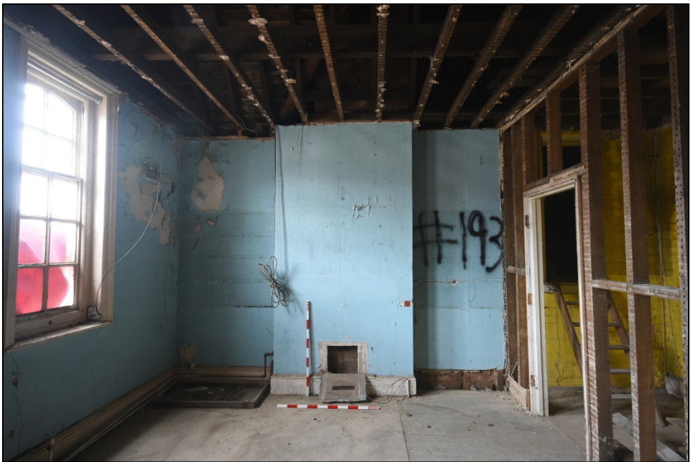
First floor office, looking south Fig 49
