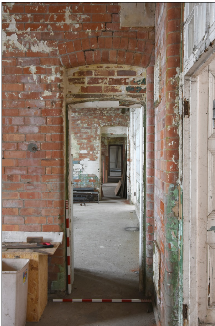
The doorways between the classrooms, looking west Fig 78
