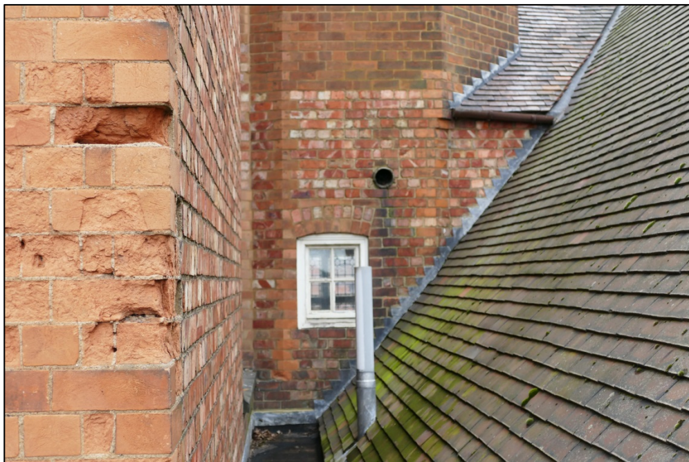
Common bricks utilised on the tower Fig 35
