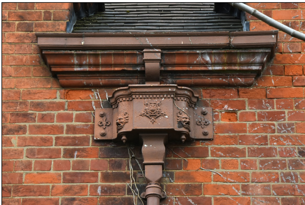
Detail of guttering and decorative hopper Fig 18
