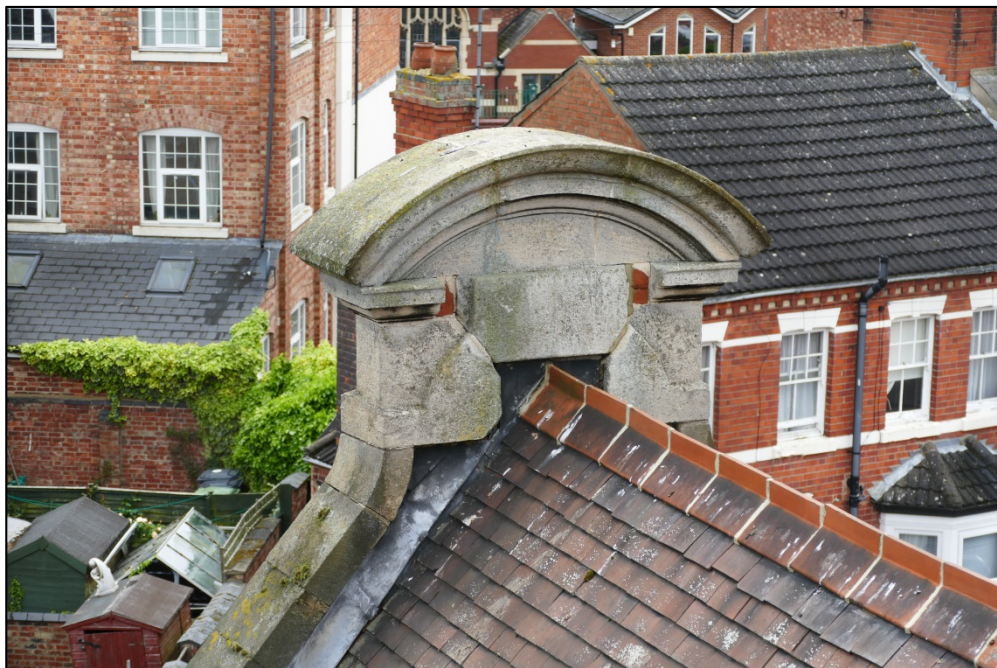
Detail of roof parapet and gable pinnacle Fig 26
