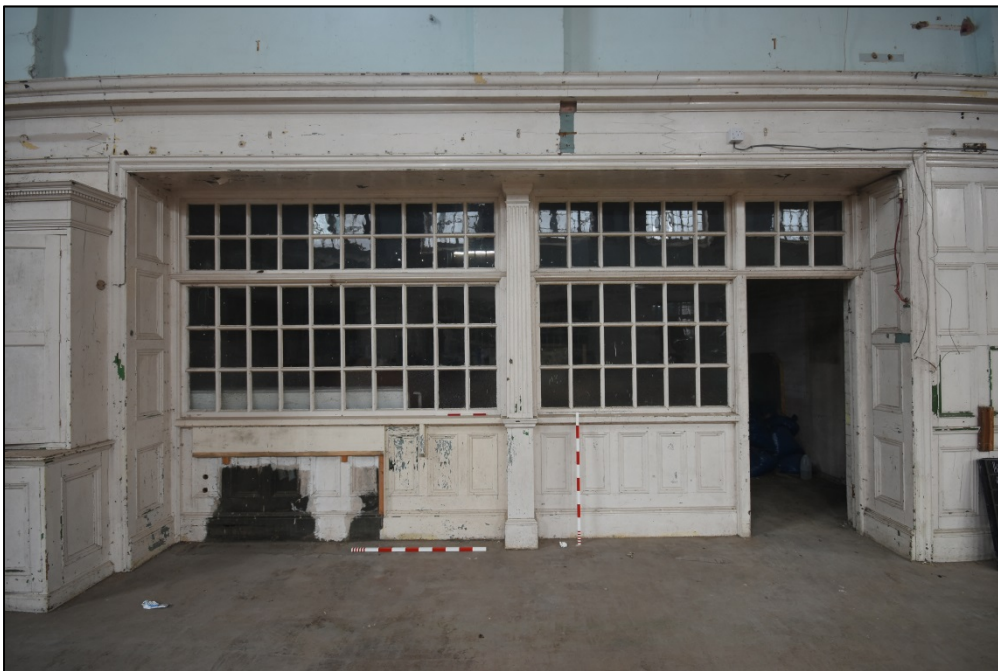
Example of the glazed screens to the classrooms Fig 55
