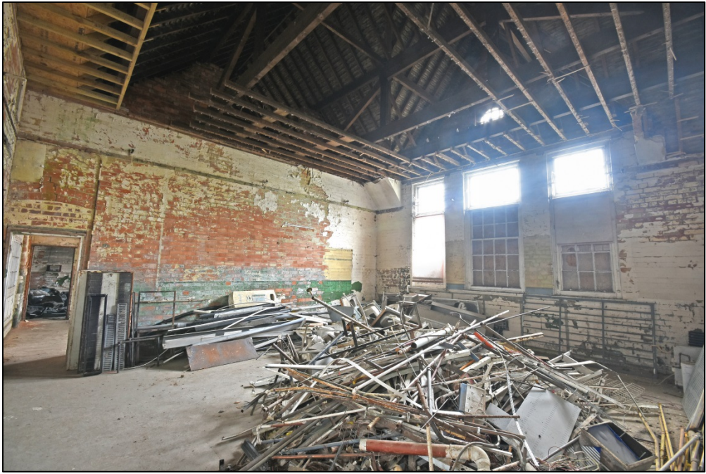
Classroom 4, looking south-east Fig 80
