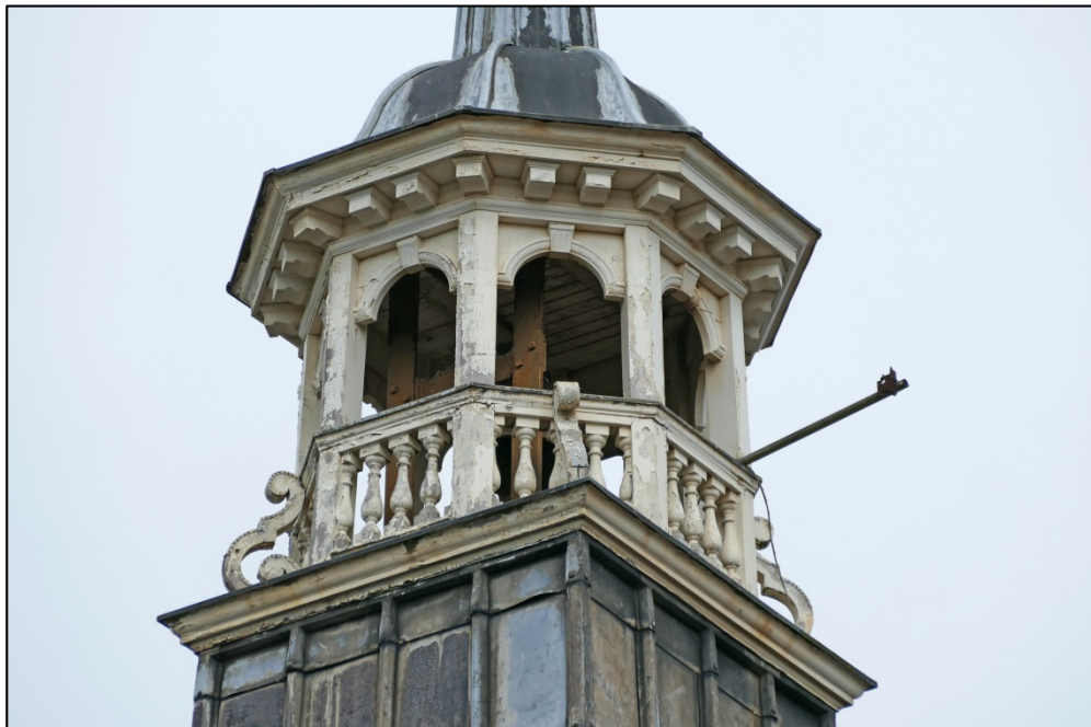
Detail of the bellcote Fig 31
