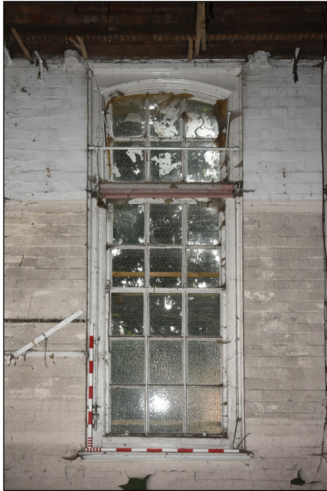
Detail of the classroom window Fig 72
