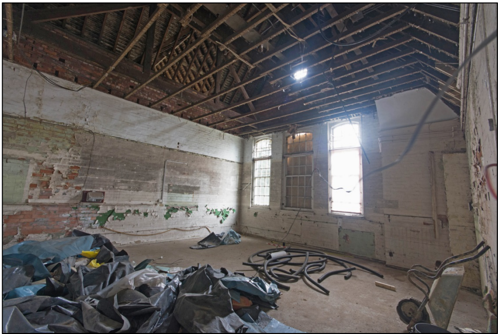
Classroom 2, looking south-east Fig 71
