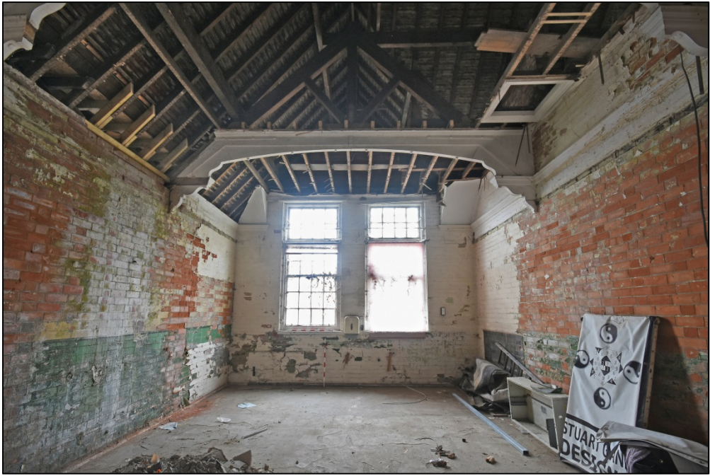
Classroom 3, looking south Fig 76
