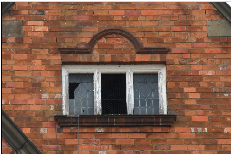
Detail of window to corridor above the central hall Fig 24
