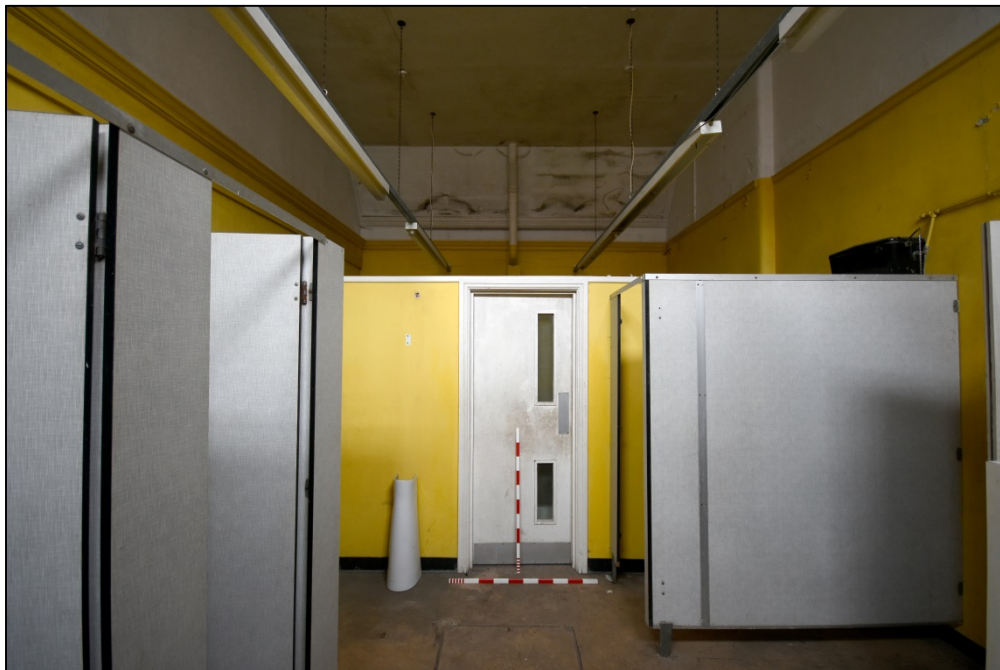
The view towards the changing room Fig 43
