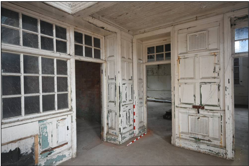
Detail of panelling, doorways, and ventilation Fig 57
