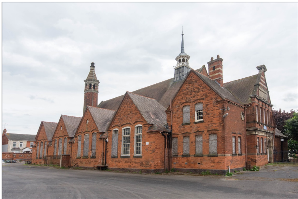
The north elevation, looking south-east Fig 28
