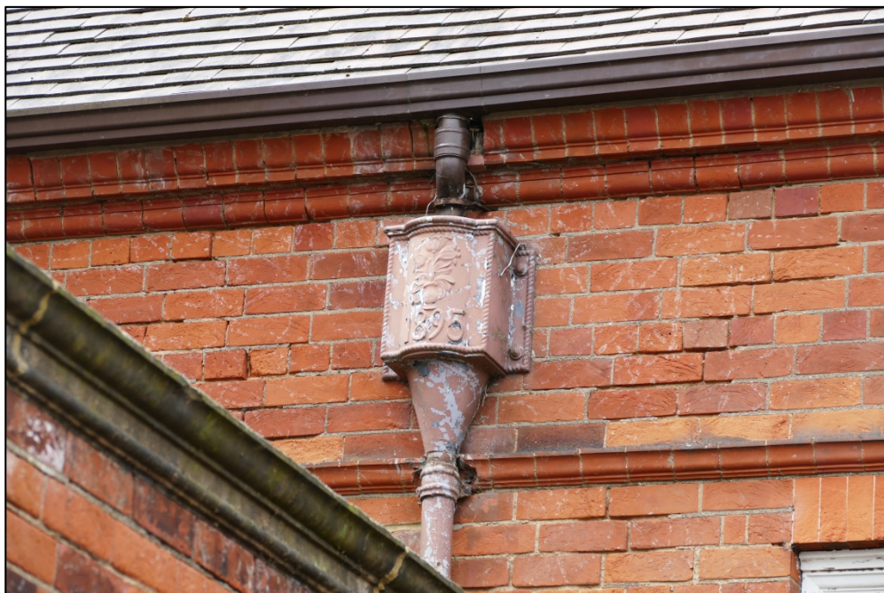
Detail of commemorative cast iron hopper with date of 1895 Fig 14
