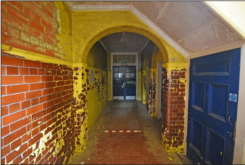
The boys' entrance corridor, looking south-west Fig 96
