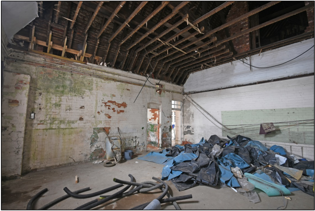
Classroom 2, looking north-west Fig 70
