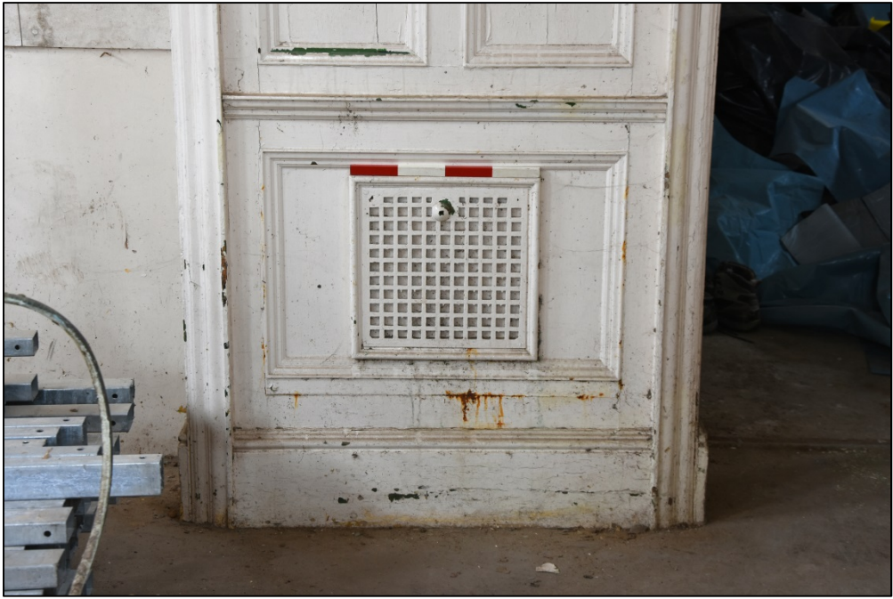
Detail of ventilation panel Fig 58
