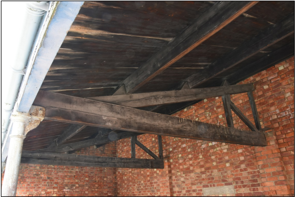
The roof structure Fig 110
