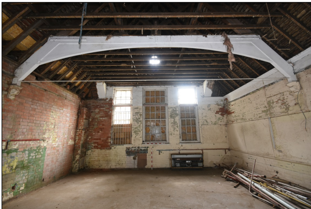
Classroom 6, looking south Fig 85
