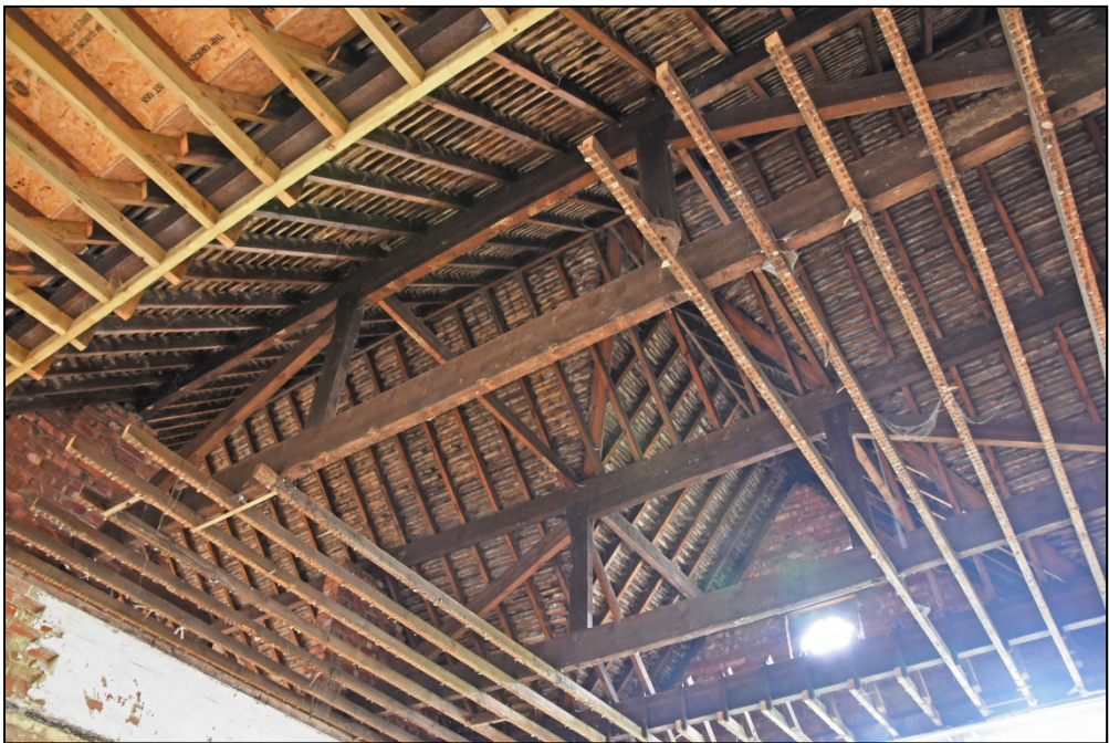
The roof structure over classroom 5 Fig 81
