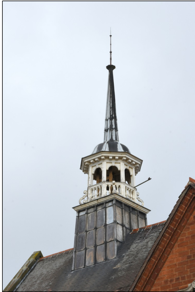
The bellcote, looking north-west Fig 30
