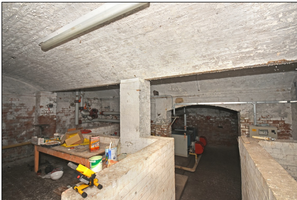
The cellar, below classroom 9, looking south-east Fig 104
