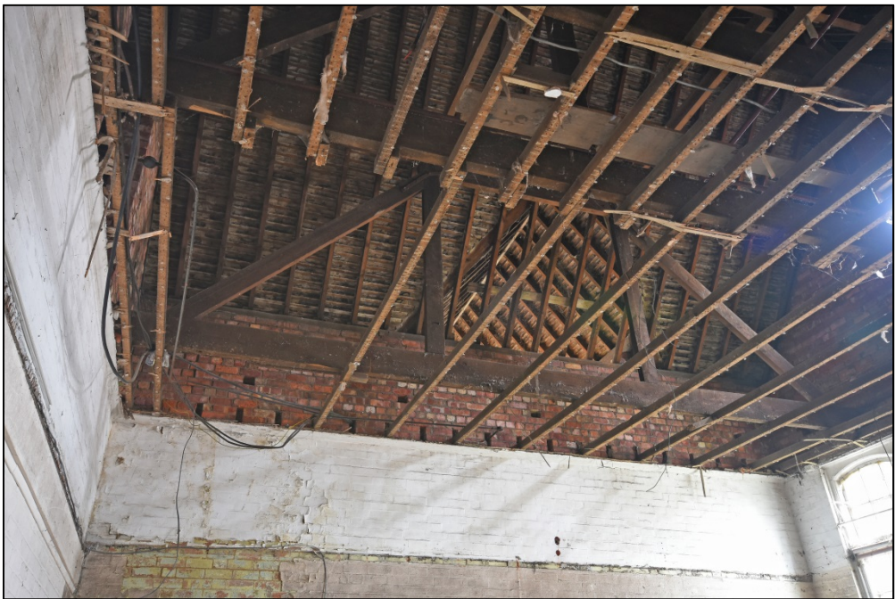
The roof structure over classroom 2 Fig 75
