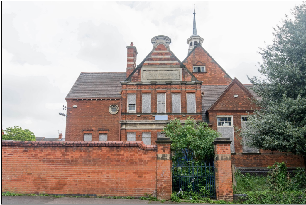
The Gordon Road elevation Fig 21
