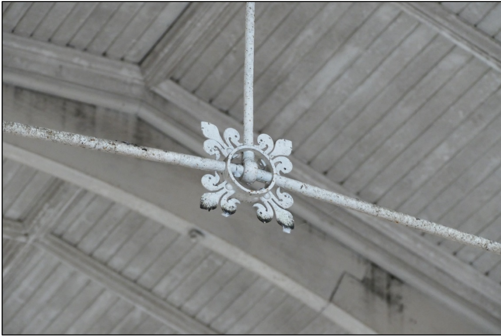
Detail of truss rod connector Fig 66
