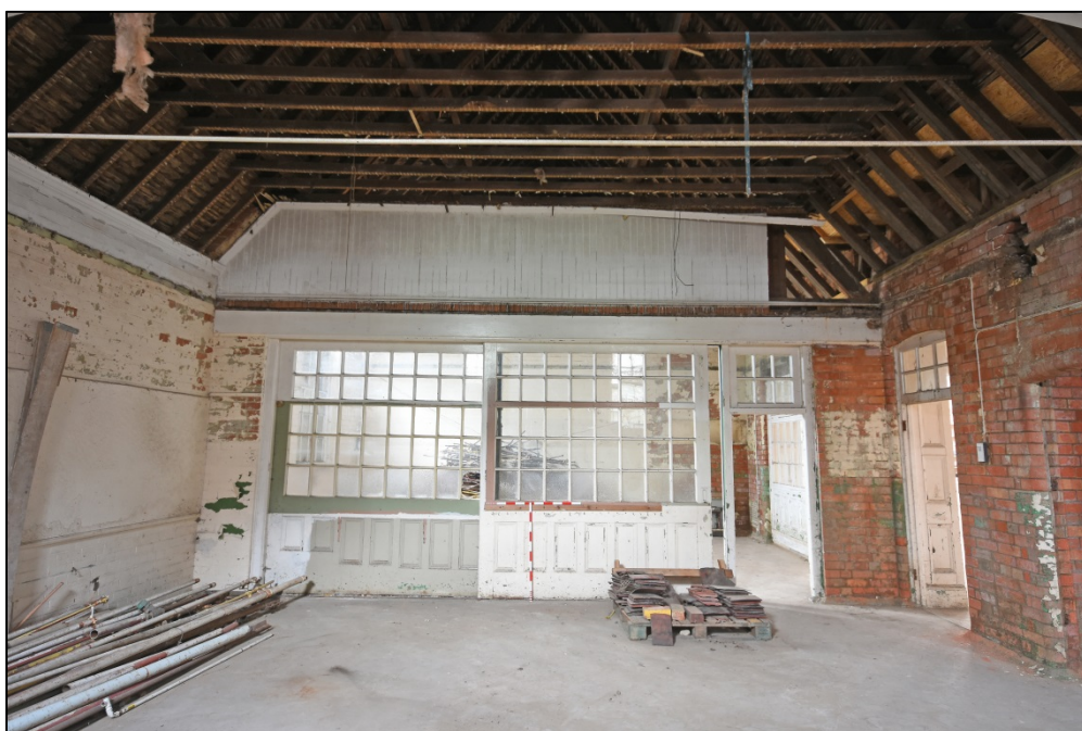
Classroom 6, showing the sliding door to the library Fig 87
