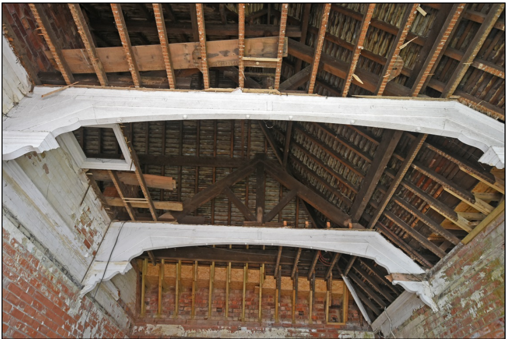
The roof structure over classroom 3 Fig 77
