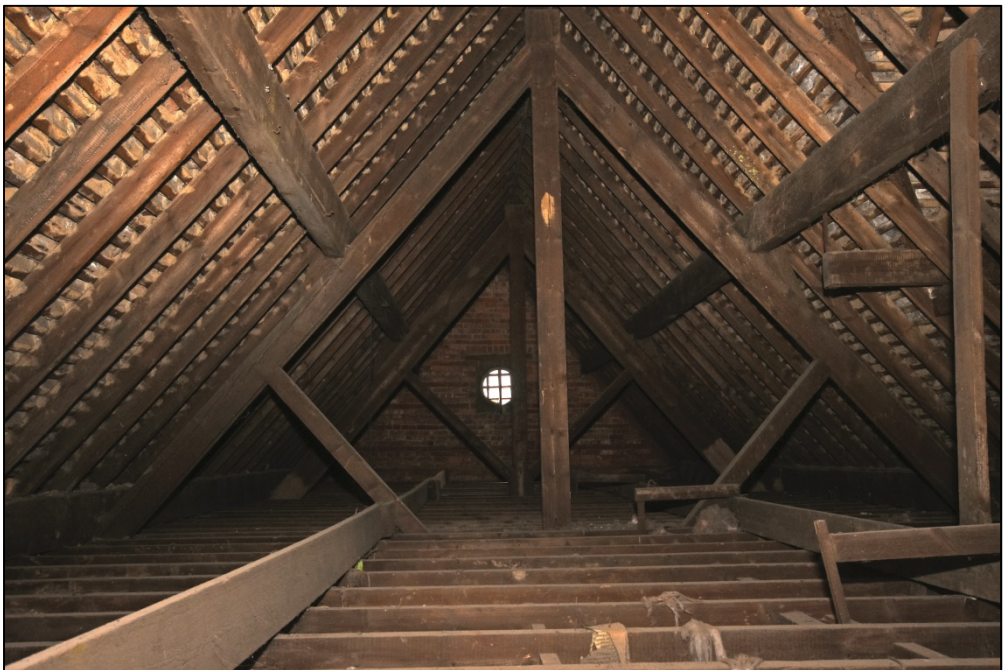
The roof above the library and classroom 6, looking south Fig 89
