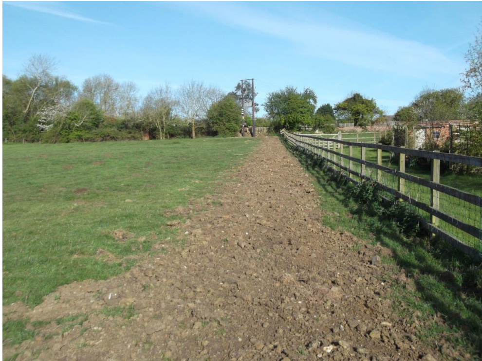
Back-filled cable trench, looking north-west towards location C Fig 6
