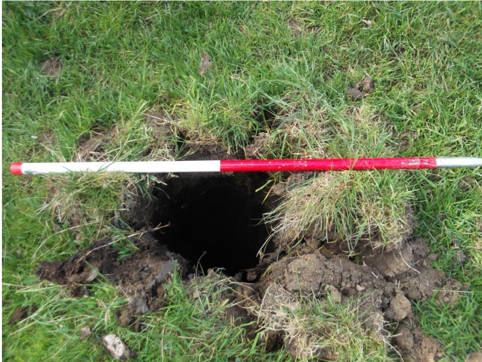
Pylon H, following removal looking south-east Fig 3
