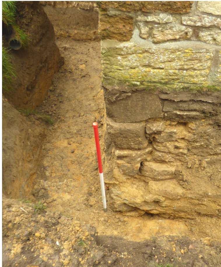
Footings of north-western corner of tower, looking east Fig 5
