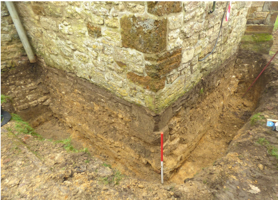
Footings of north-western corner of tower, looking south-east Fig 4
