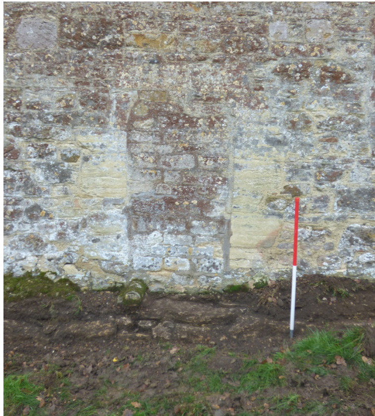
Blocked doorway, north wall of nave, looking south Fig 7
