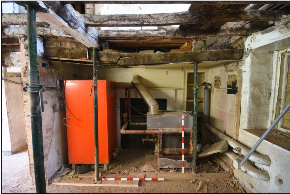
The fireplace of room G3 Fig 26
