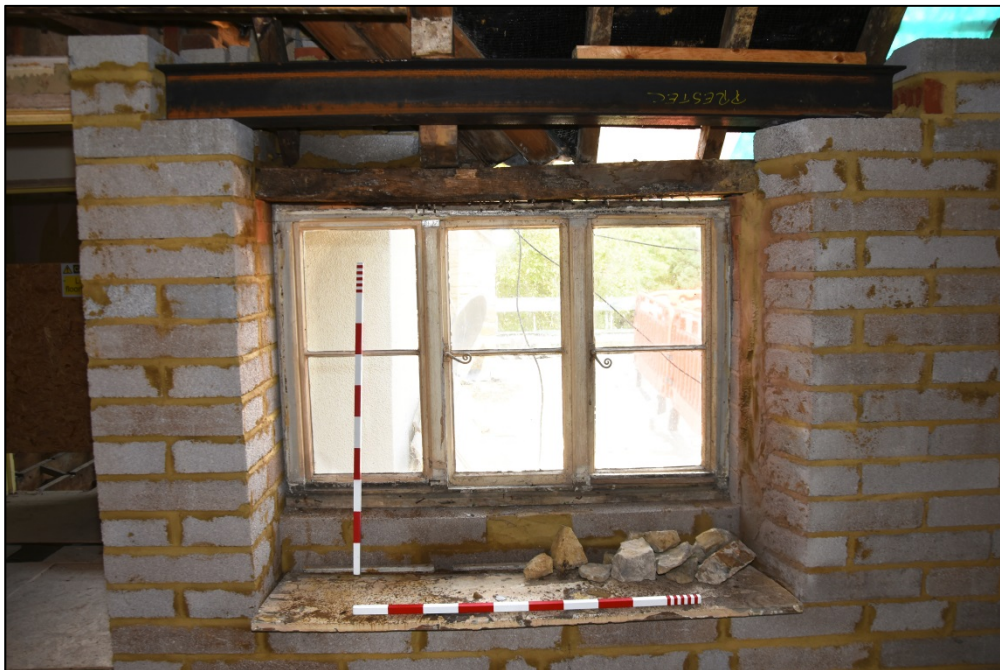
Detail of remediation work around north-facing window of room F5 Fig 55
