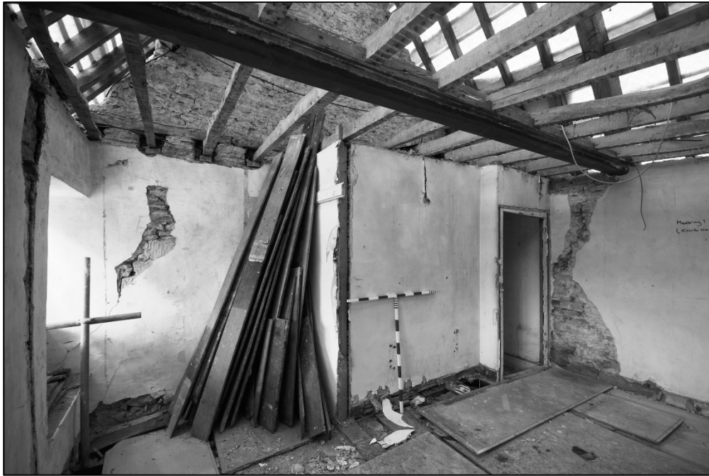
Room F1, looking north-west (image converted to greyscale) Fig 38
