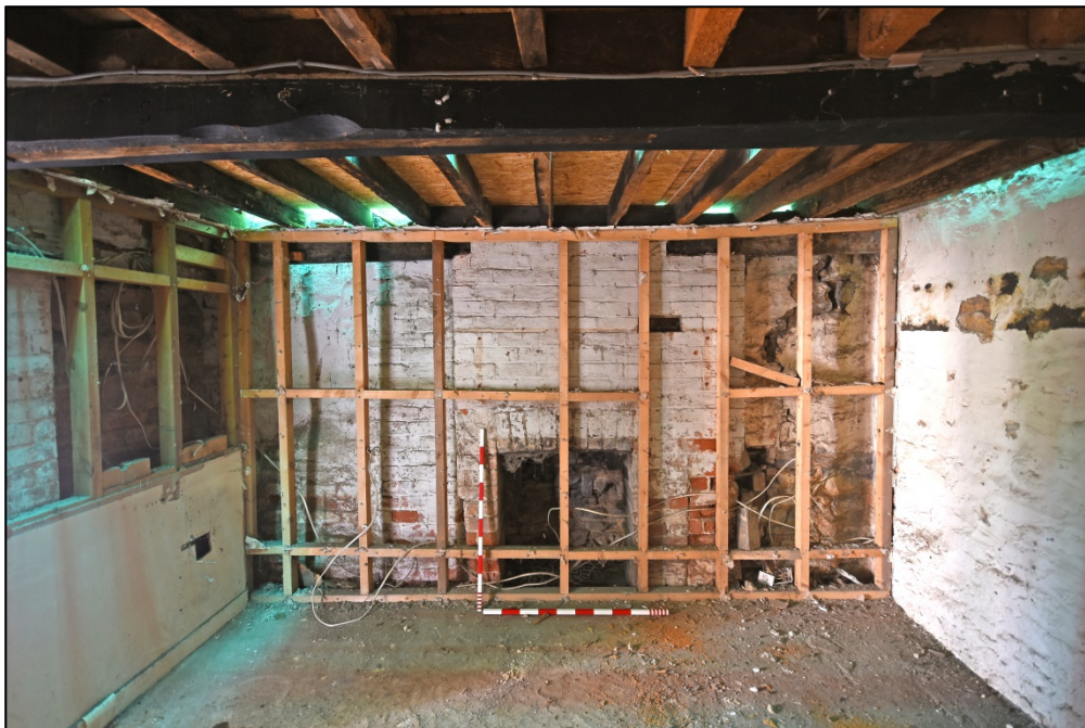
Room G4, looking east Fig 29
