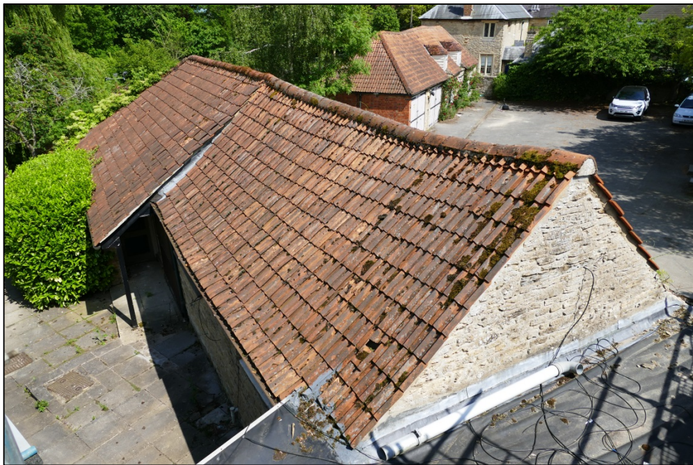
The coach house roof, looking north-east Fig 69
