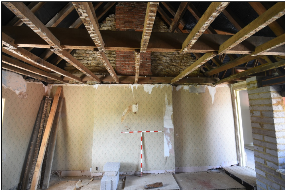
The west wall of room F5 Fig 53
