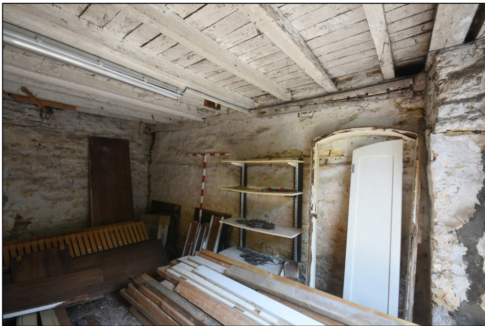
Room S2, looking north-east Fig 77
