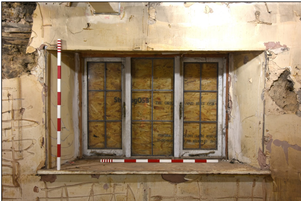
Detail of window, room G5 Fig 35
