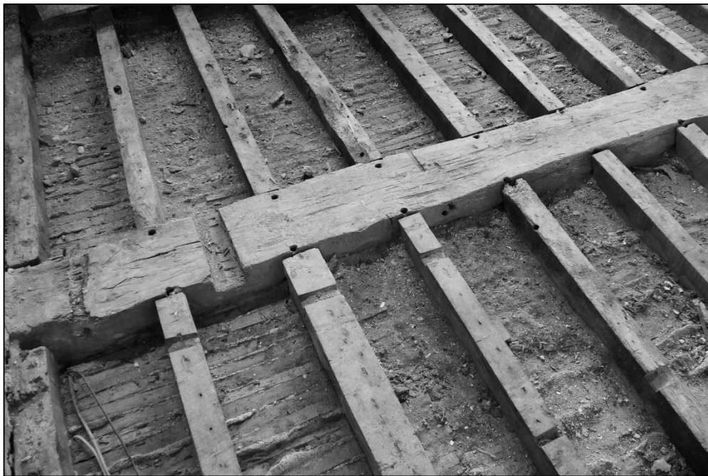
Detail of the spine beam and joists, room F2 (image converted to greyscale) Fig 43
