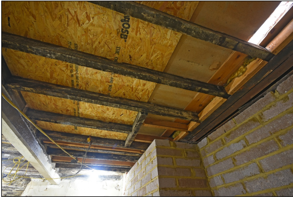
The ceiling of G5, showing trimmer joist Fig 36
