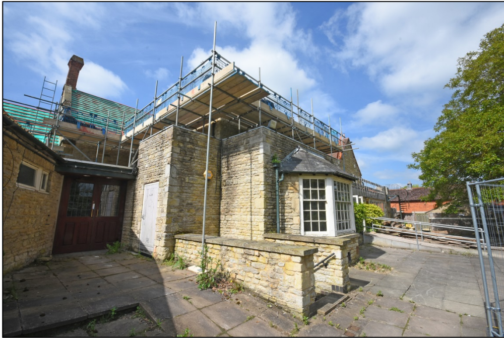
The 19th and 20th-century extensions, looking south-west Fig 56
