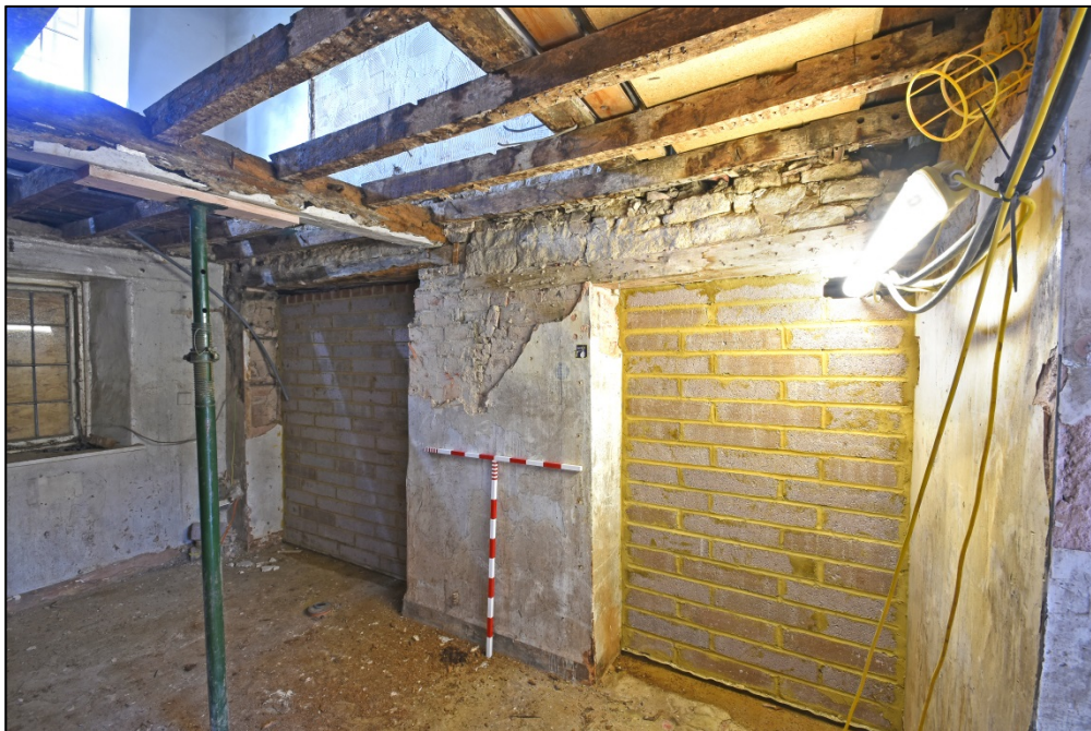
The west wall of room G3 Fig 27
