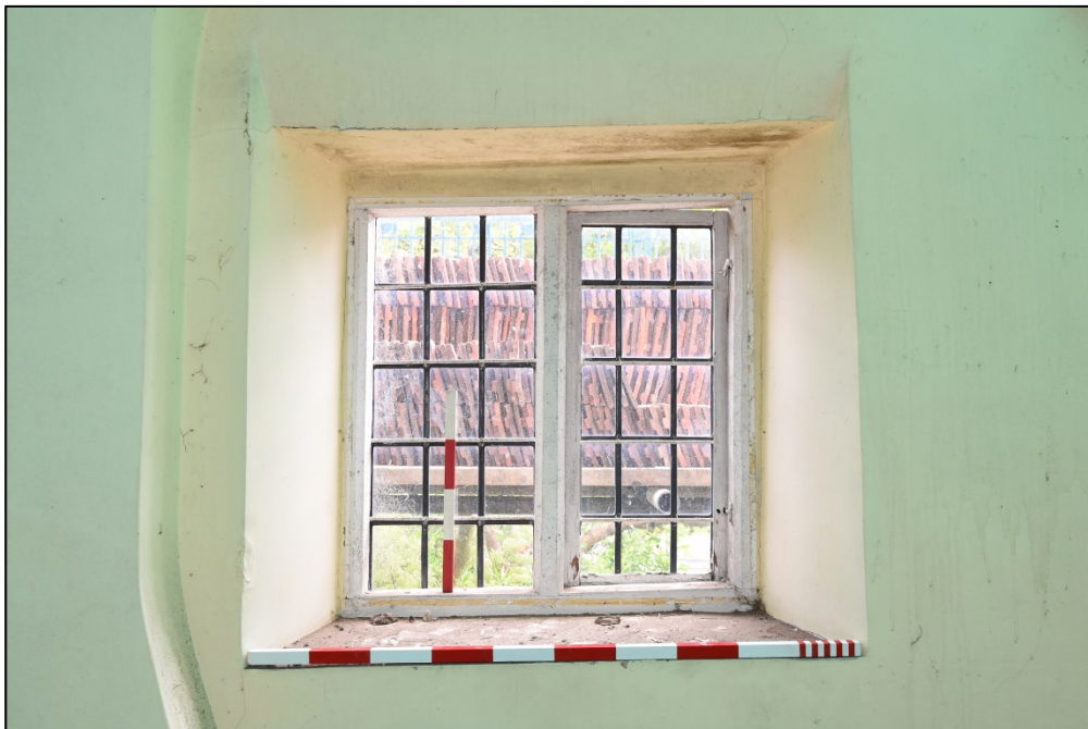
Detail of window, room F4 Fig 47
