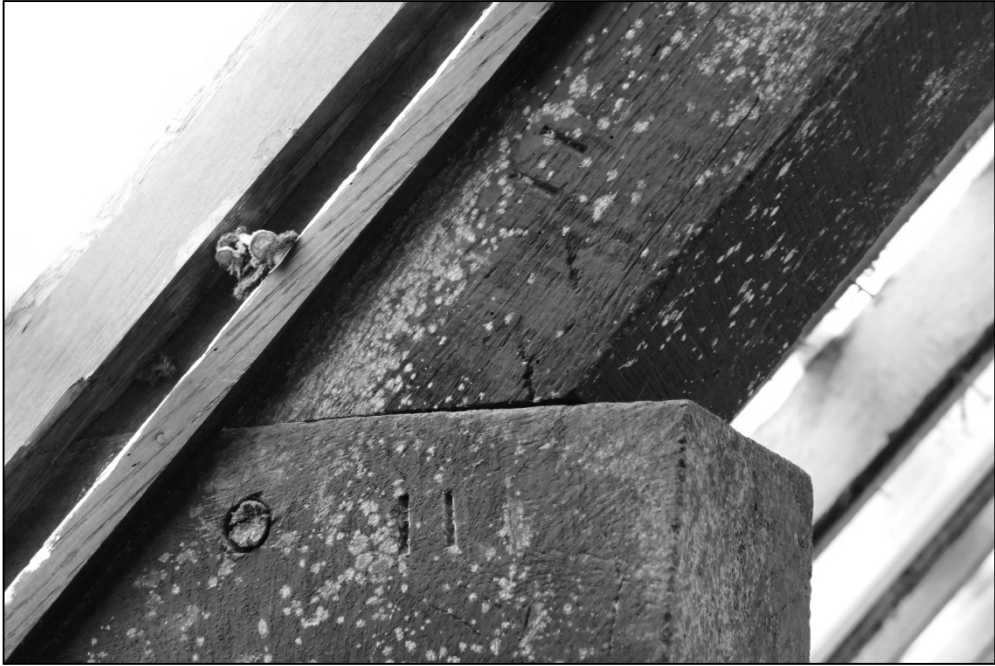
Detail of assembly marks on base of principal rafter Fig 50
