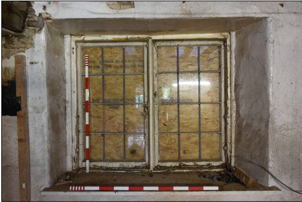
Detail of the window, room G3 Fig 28
