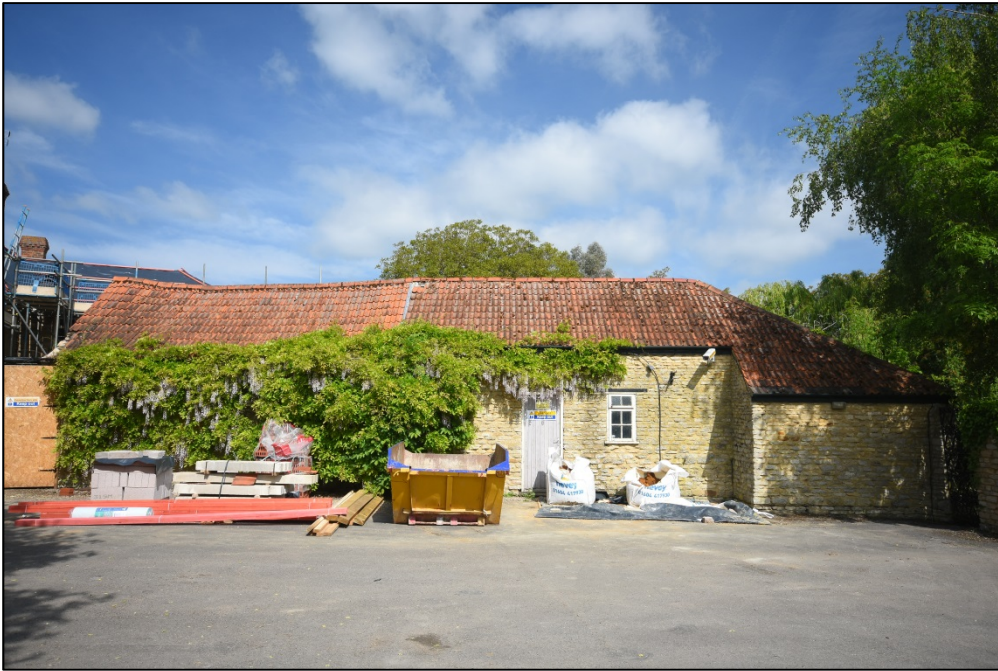
The east elevation of the coach house Fig 68
