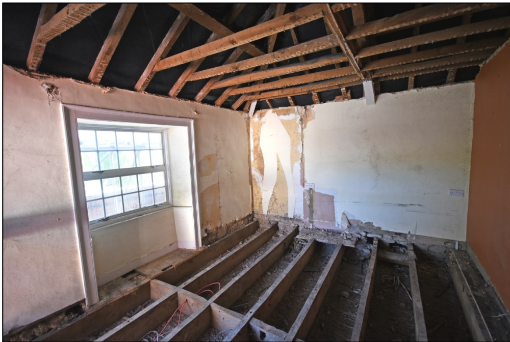
Room F7, looking north-east Fig 67
