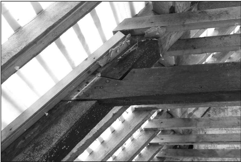
Detail of collar joinery Fig 51
