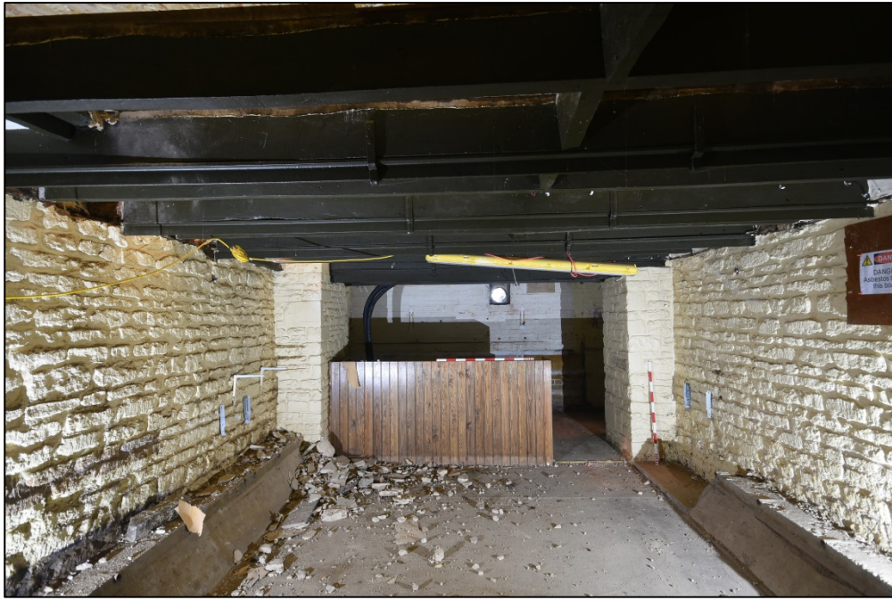
The cellar, looking north Fig 60
