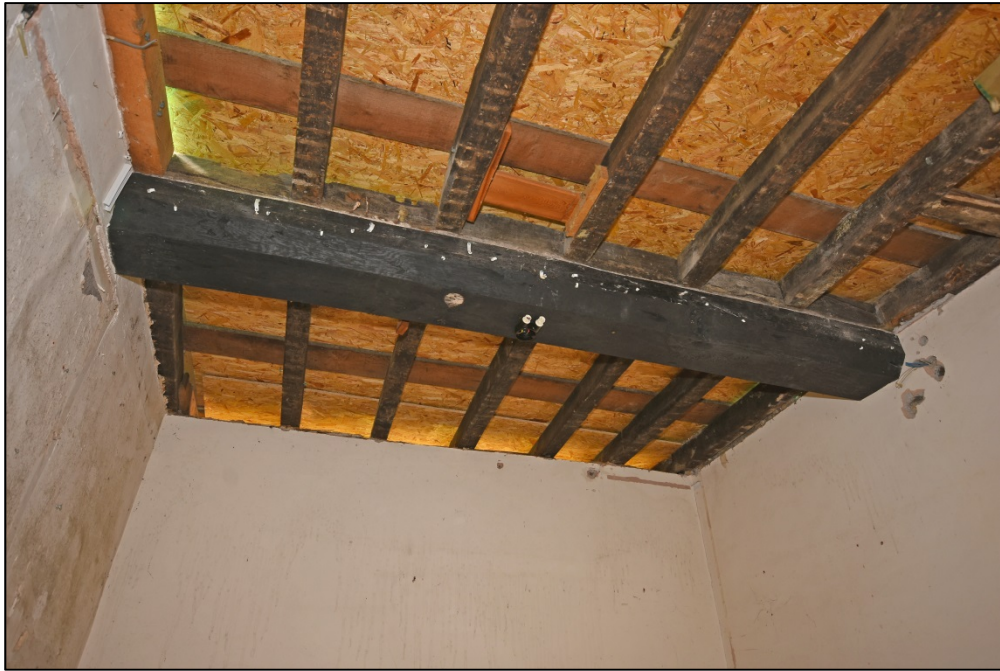
The spine beam and joists, room G2 Fig 22
