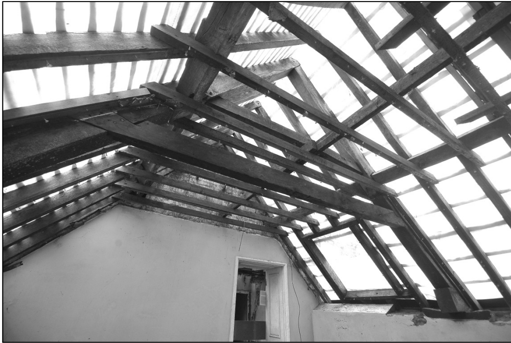
The roof structure of room F4 (image converted to greyscale) Fig 48
