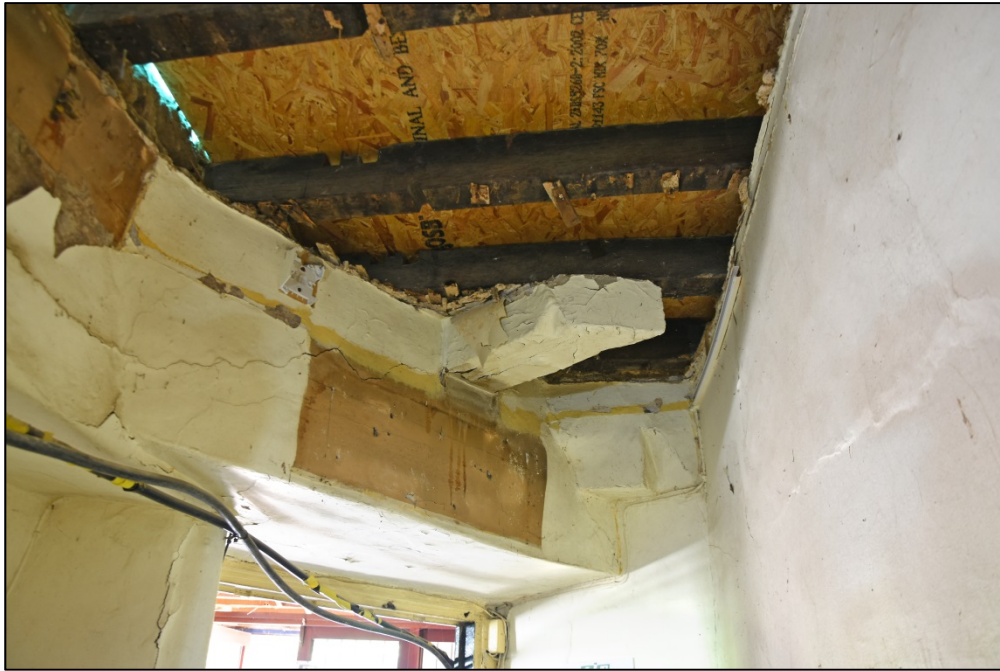
Detail of truncated beam with stops Fig 32
