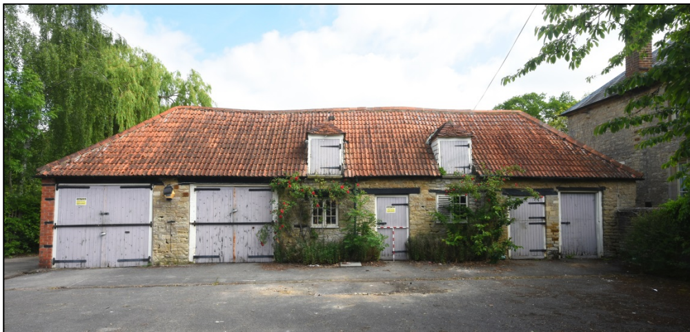
The stables, looking north Fig 71
