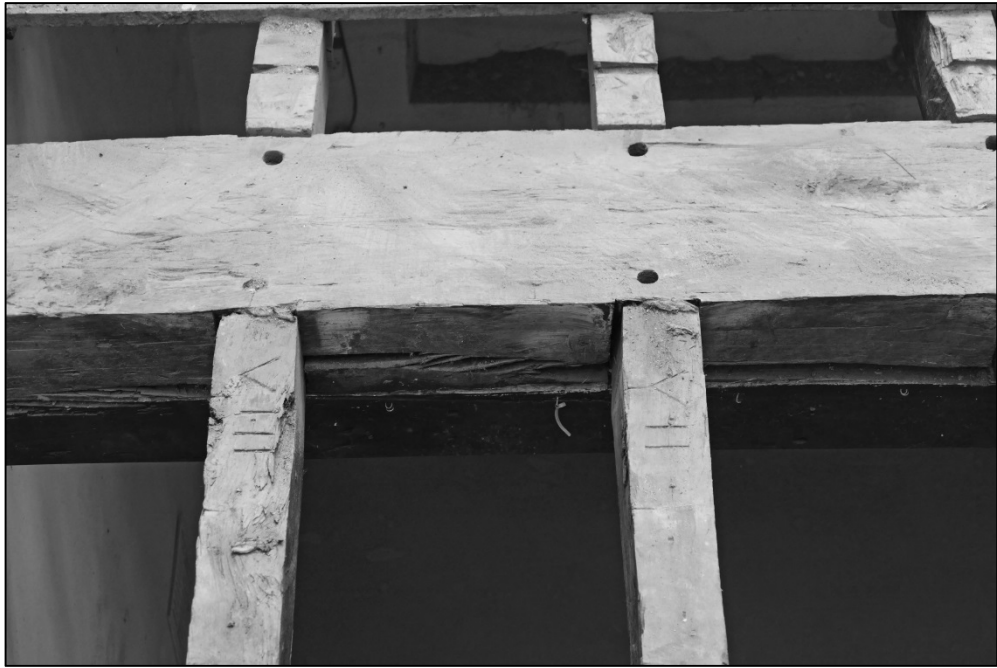
Detail of assembly marks and joinery (image converted to greyscale) Fig 24
