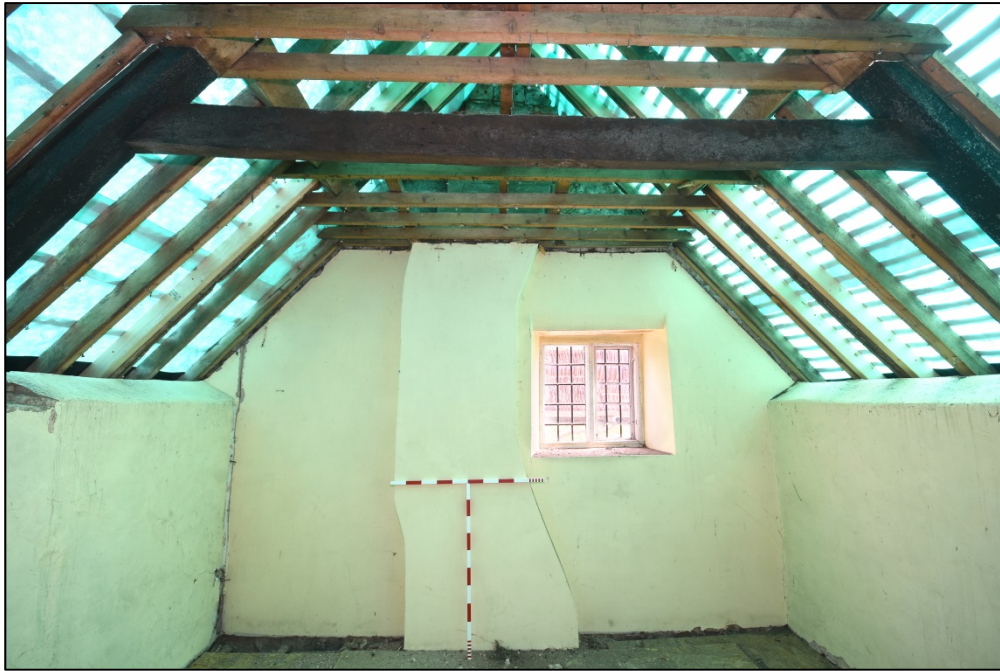
Room F4, looking east Fig 46
