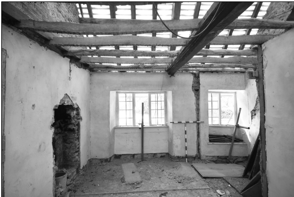
Roof F1, looking south (image converted to greyscale) Fig 41
