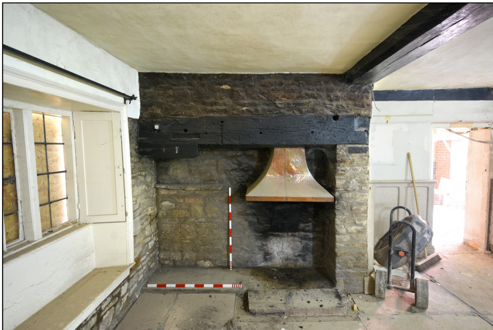
The open fireplace, room G1 Fig 19
