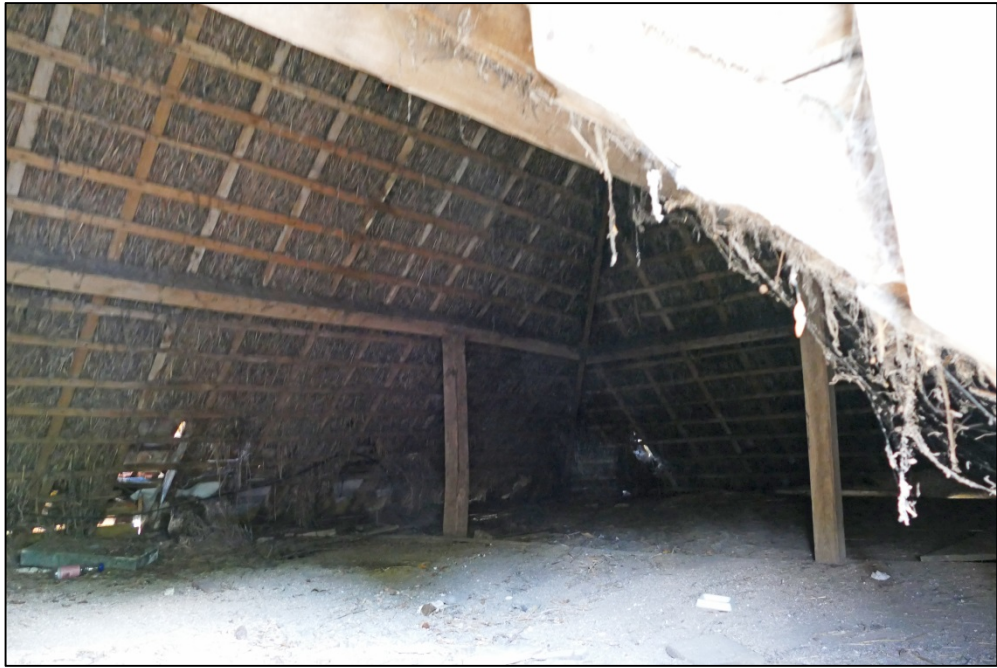
The loft, looking north-east Fig 76
