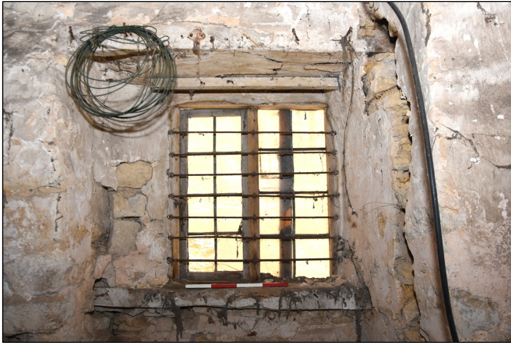
Detail of window, room S5 Fig 80
