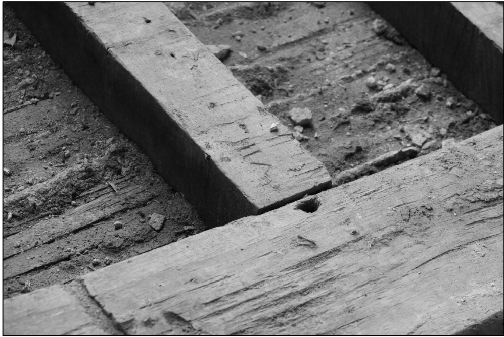
Detail of assembly mark Fig 44
