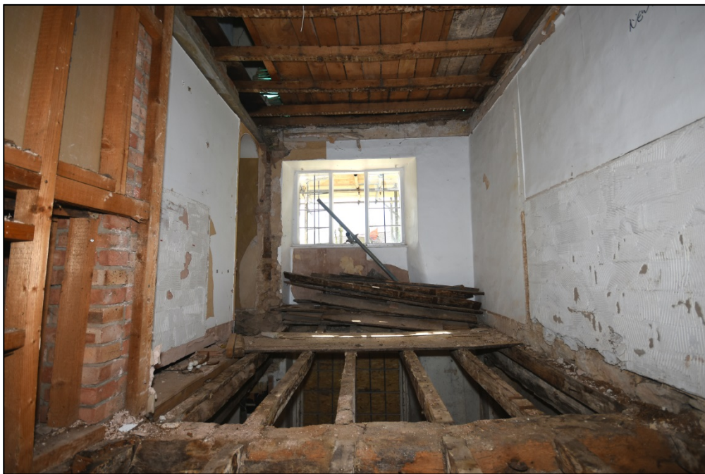
Room F3, looking south Fig 45
