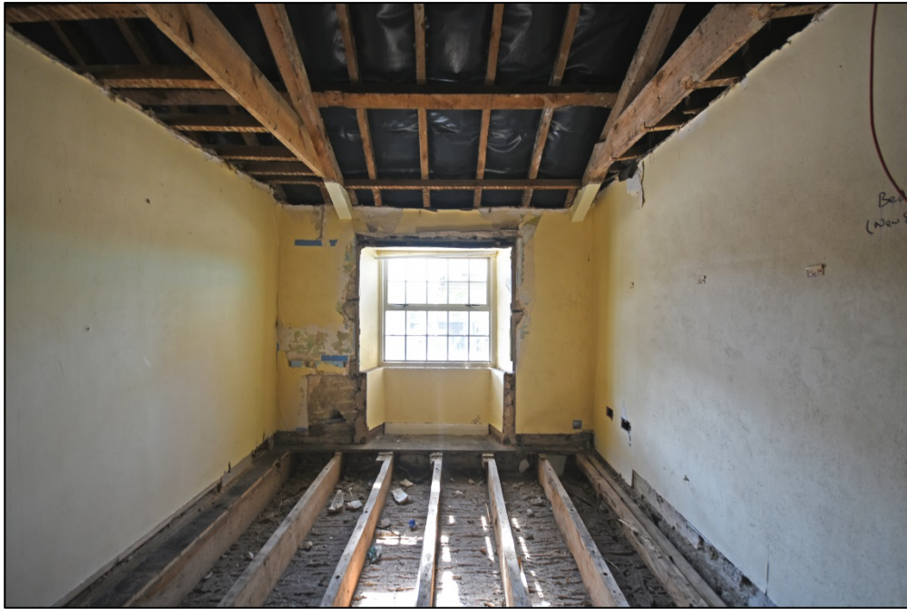
Room F6, looking east Fig 66
