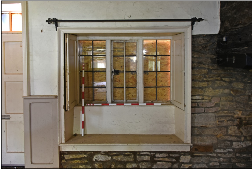
Detail of window, room G1 Fig 20
