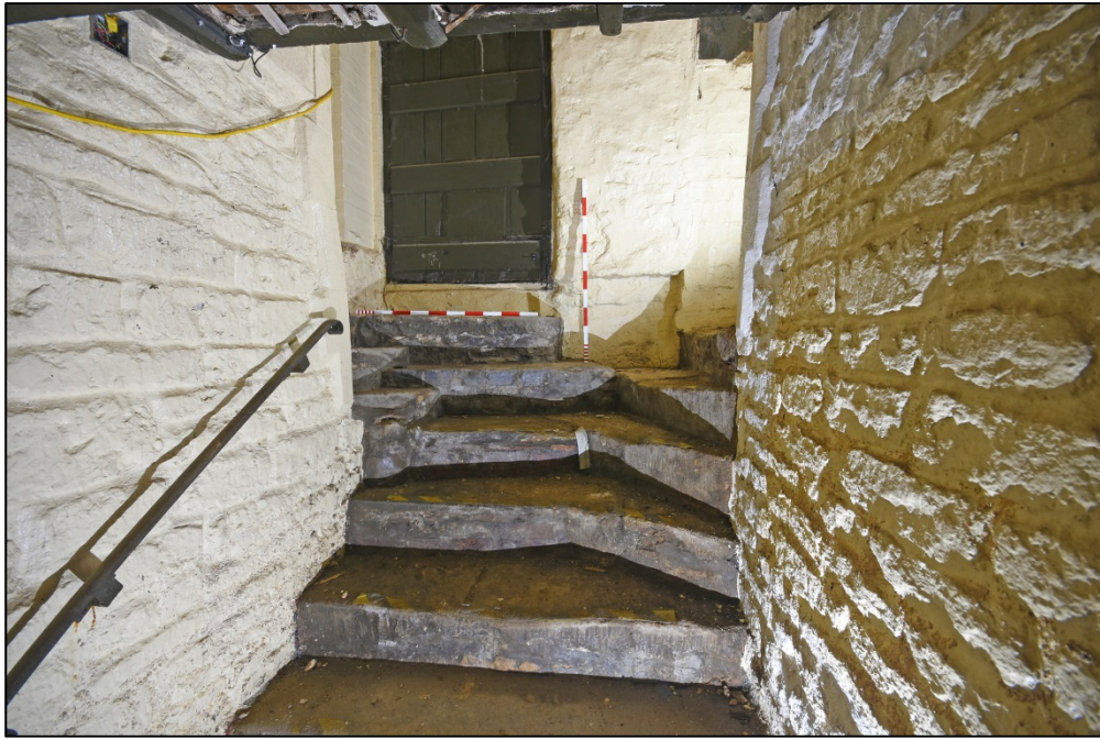
Stairs to the cellar Fig 58
