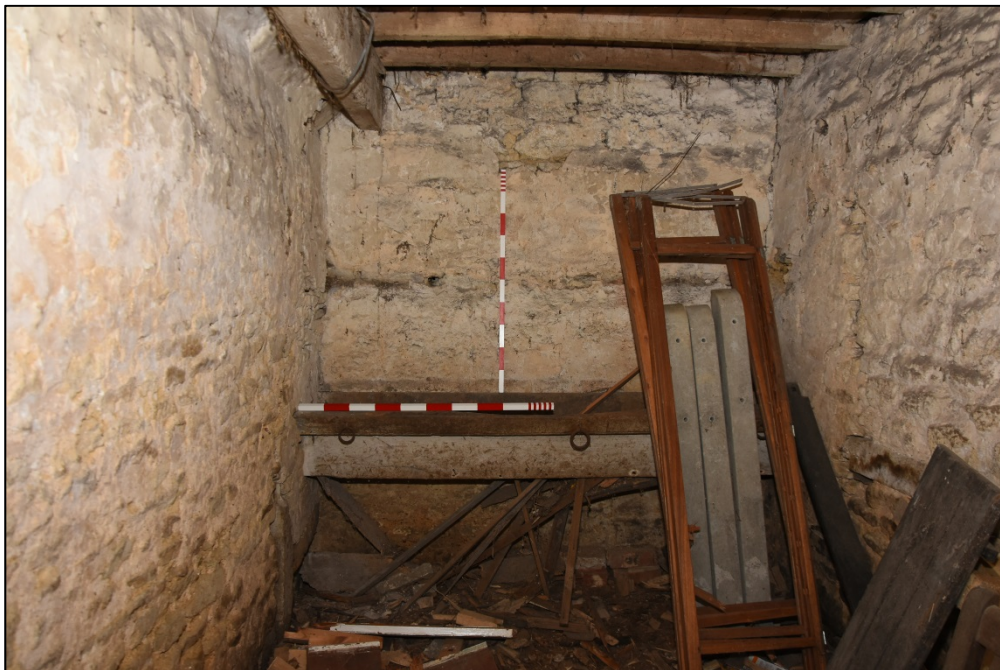
Trough in room S5 Fig 79
