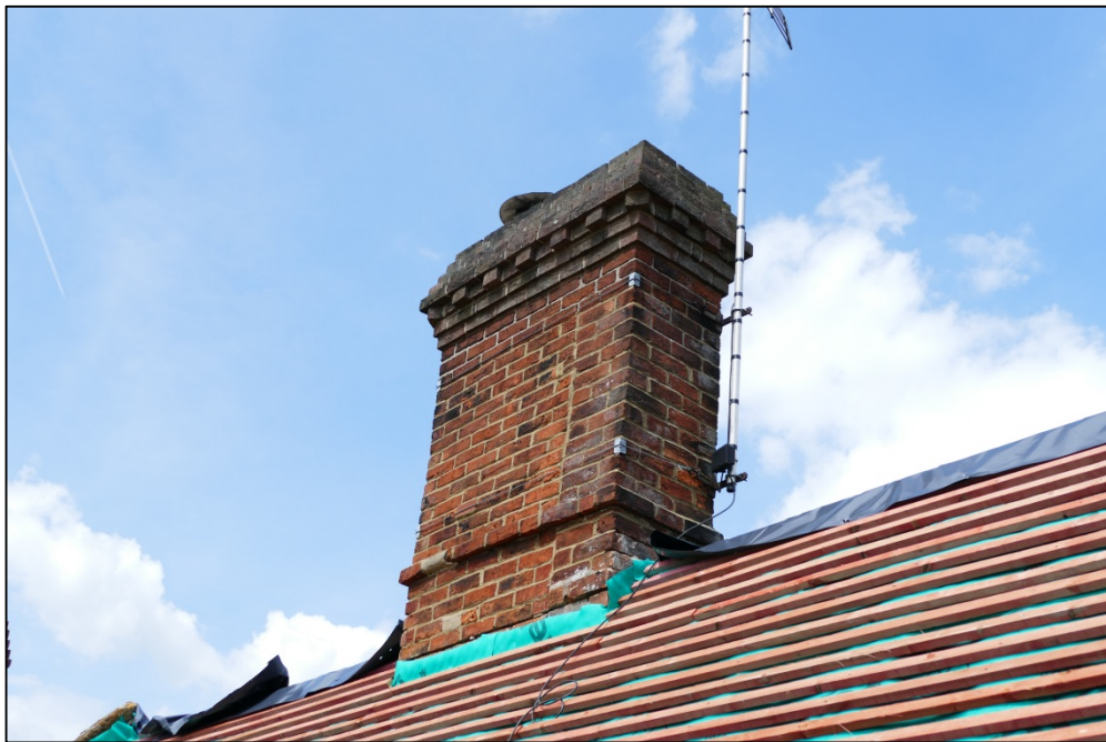
The central chimney, showing the widening of the original flue Fig 17
