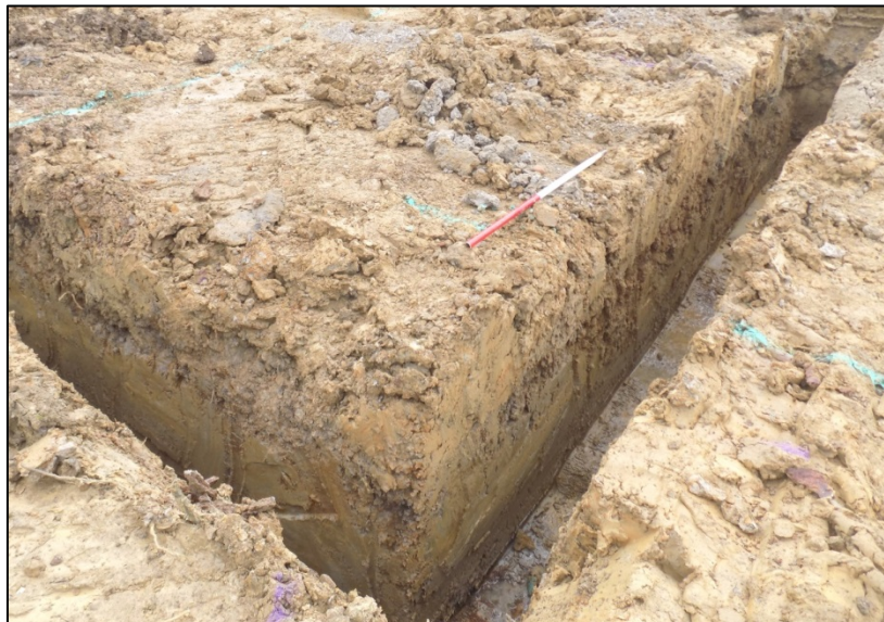
Plot 5 garage, footings trenches, looking north Fig 11
