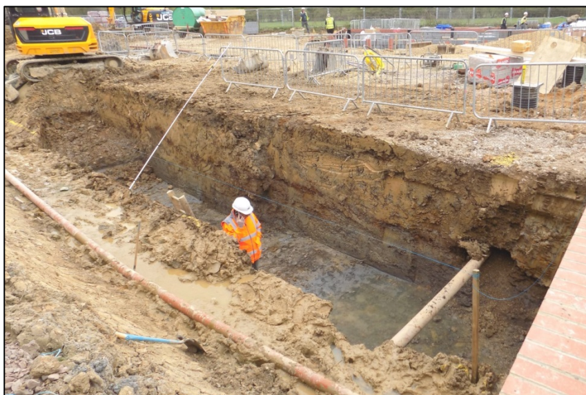
Retaining wall trench looking south-east Fig 13
