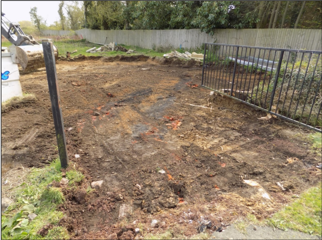
Layer of modern demolition rubble (006) looking south-east Fig 6
