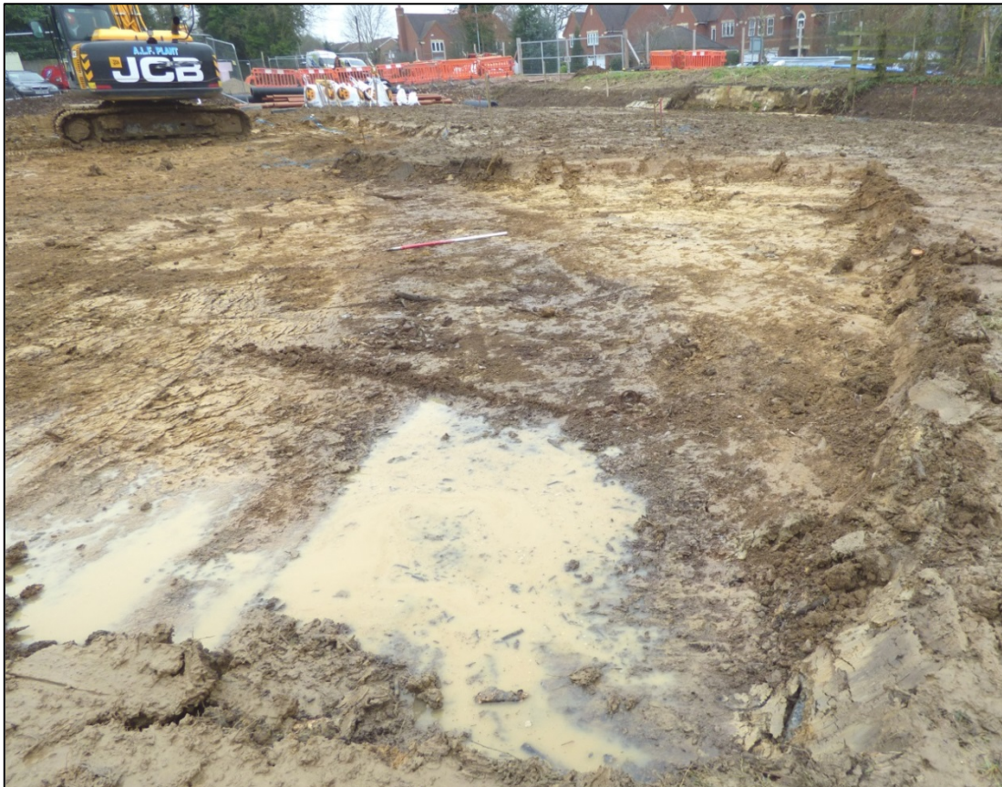
Ditch [005]/[605], looking north-west Fig 3
