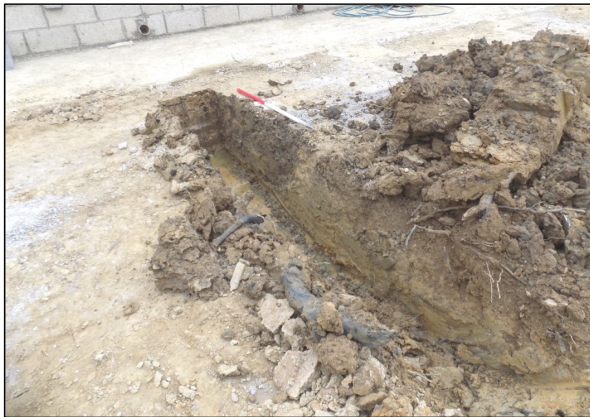
Plot 6, exploratory trench, looking north Fig 12
