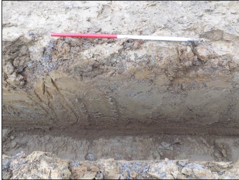
Plot 3, north-western side, footings trench section, looking south east Fig 9
