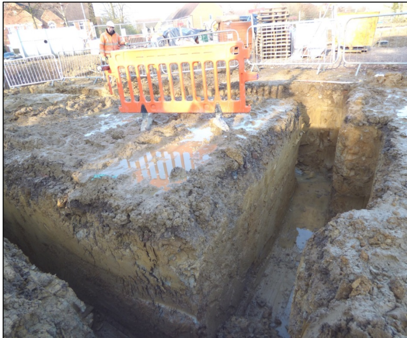
Plot 1, south-eastern corner, footings trenches, looking north-east Fig 7
