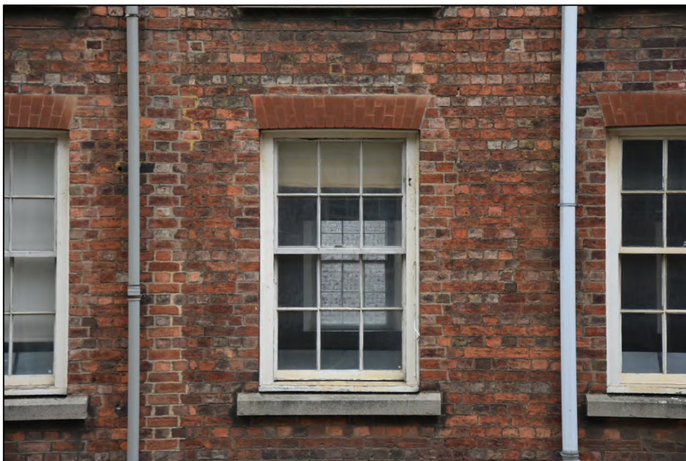
Example of the ground floor windows Fig 55
