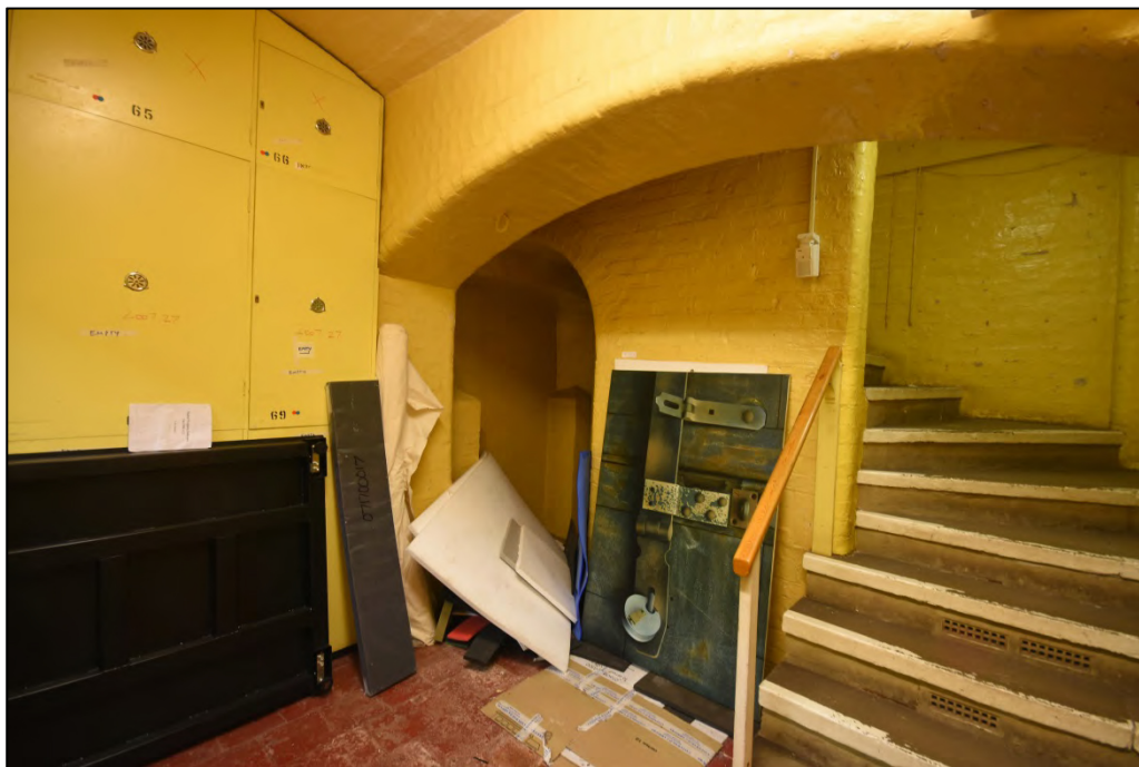
The basement stair, showing the awkward arrangement of this feature Fig 43
