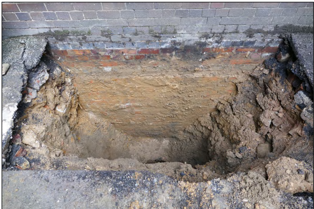
Foundation trench 1, showing the exposed foundations Fig 143
