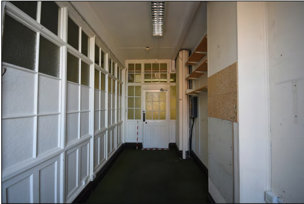
Interior of the panelled offices Fig 106
