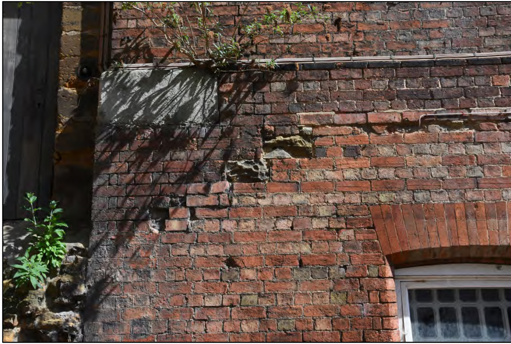
Detail of former steps to the hanging shed and platform Fig 62
