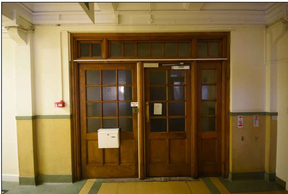
The main entrance at ground floor level Fig 131
