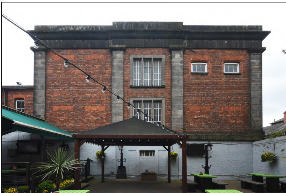
The north elevation of the west wing Fig 67
