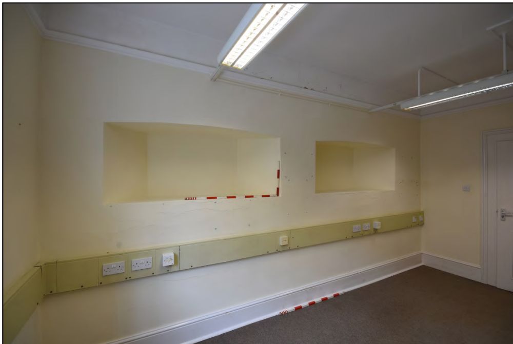
Blocked windows of the north elevation Fig 97
