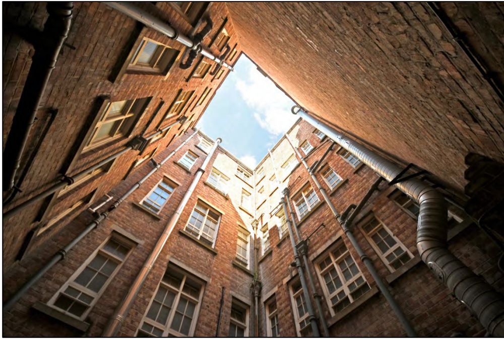
The west wing lavatory block atrium Fig 70
