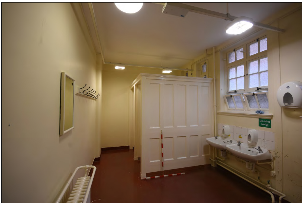
The men's lavatory Fig 93
