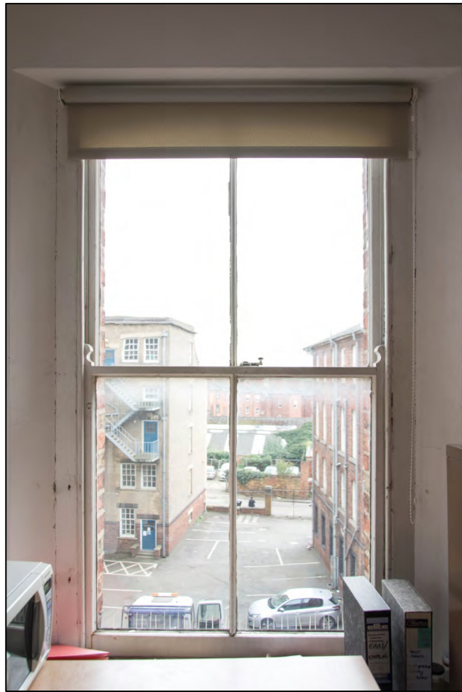
Internal view of the south-facing upper floor sash windows Fig 34
