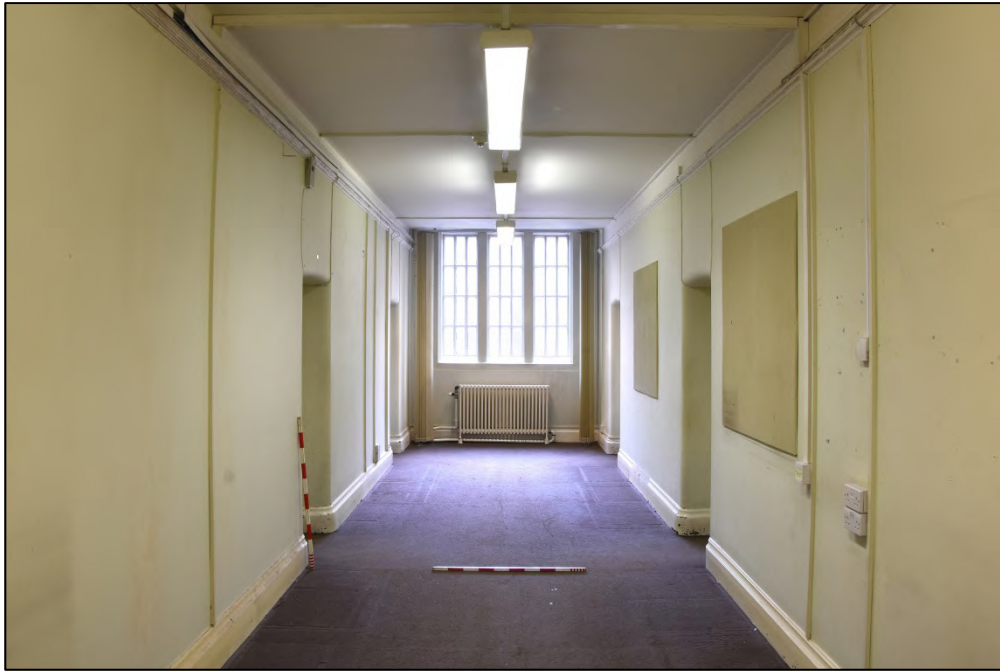
The north corridor Fig 108
