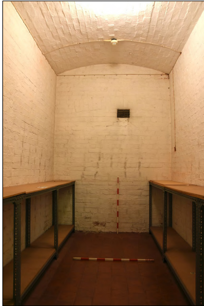
Former cell, now a strong room. Note blocked window at the rear wall Fig 74
