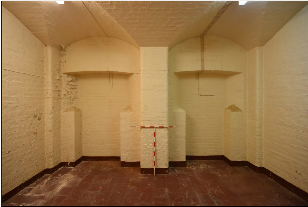
The north-western room of the museum basement, showing blockings Fig 40
