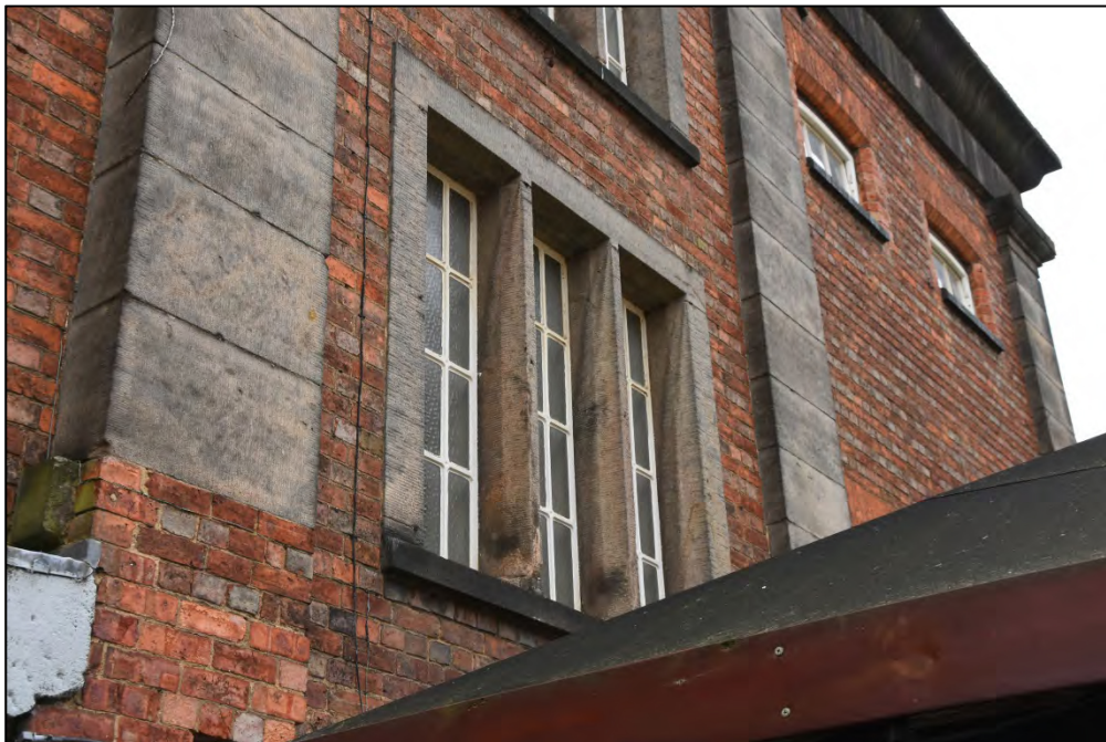
Detail of the first floor window Fig 69
