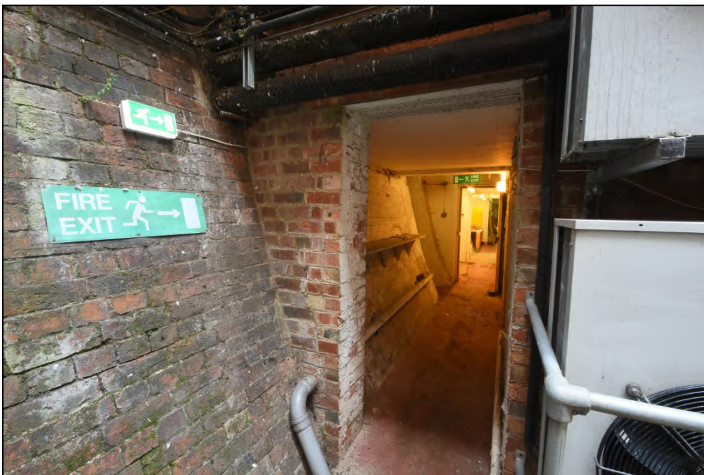
The battered retaining wall at the north of the museum Fig 37
