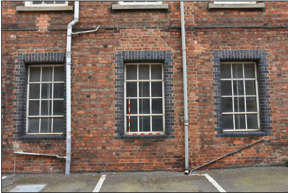
Detail of lower ground floor level windows Fig 54
