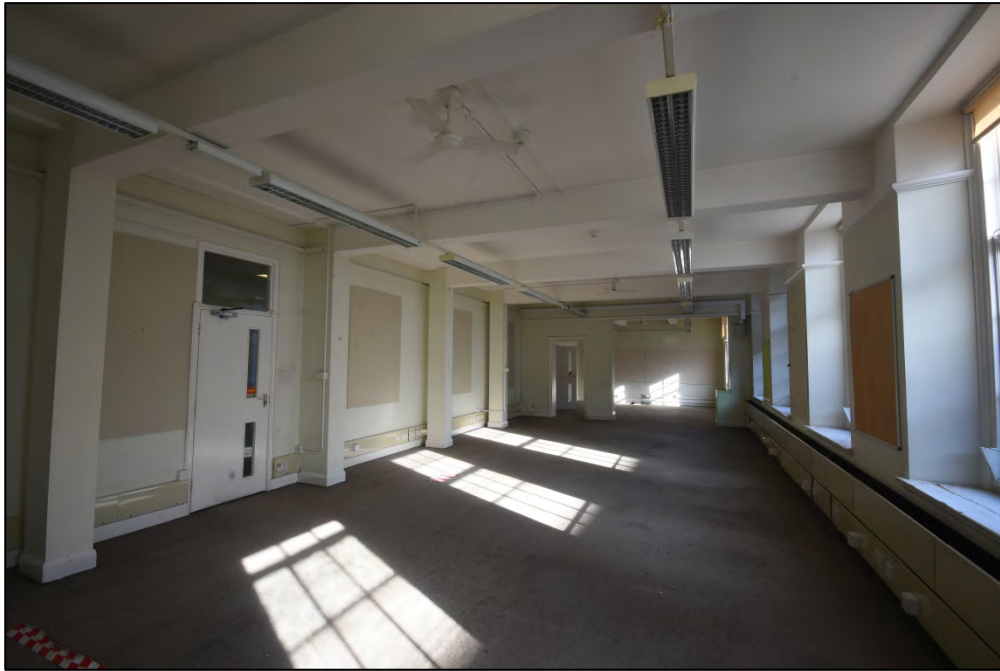
Open plan office at the eastern side of the first floor Fig 102
