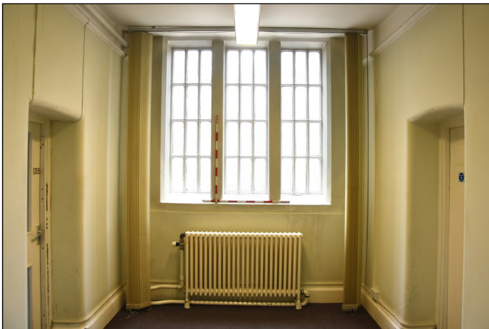
Detail of the corridor window Fig 109
