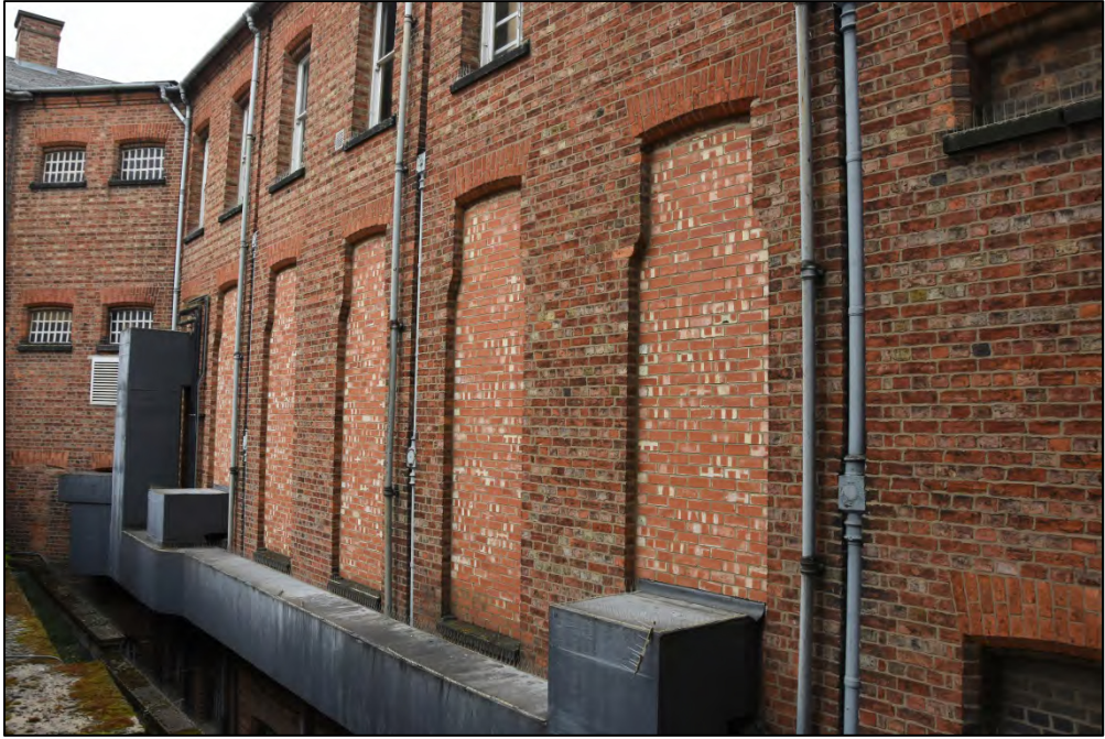
Detail of the enlarged and blocked windows on the south elevation of the museum / east gaol wing Fig 32
