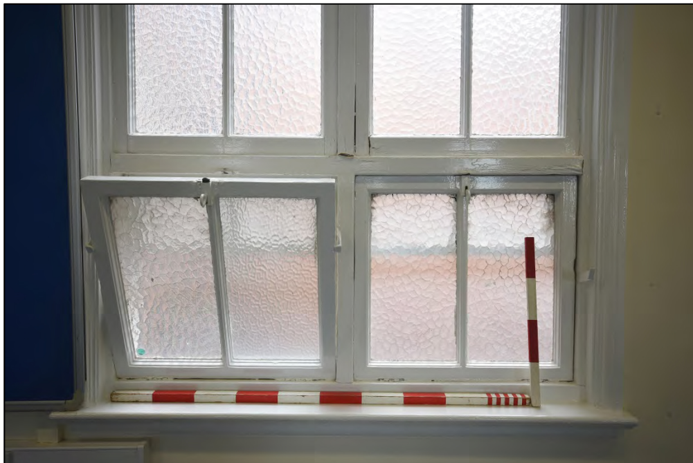
Detail of the atrium windows Fig 117
