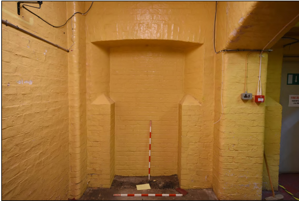
Example of the blocked doorways, showing the shouldered jambs Fig 42
