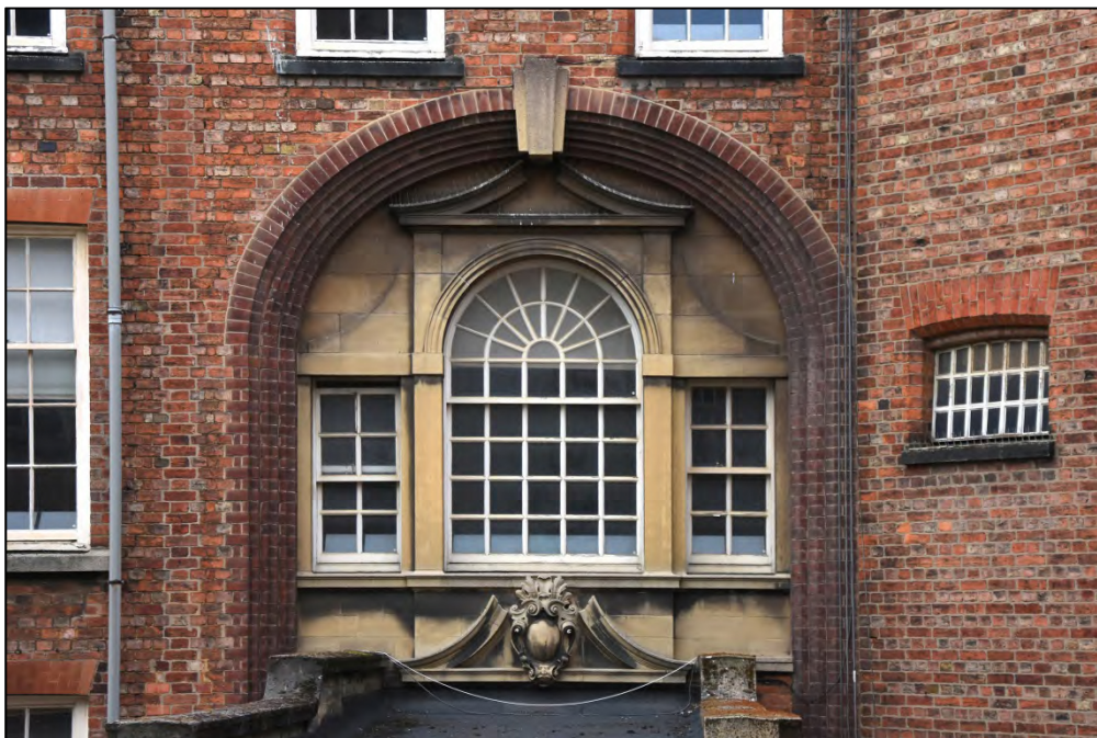
The 1930s elevated access porch and windows Fig 53
