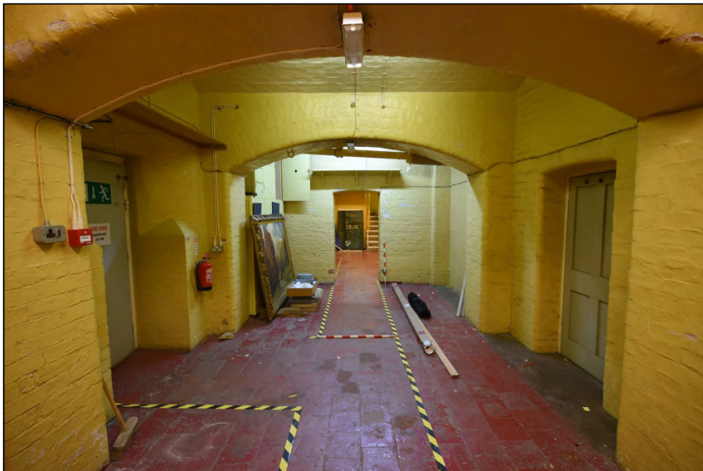
View across the former northern basement rooms, looking east Fig 41
