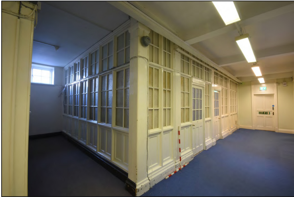
The panelled offices at the north of the first floor Fig 104
