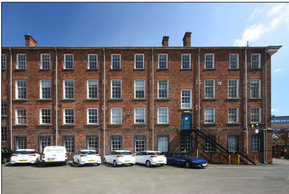
The southern end of the west elevation Fig 59
