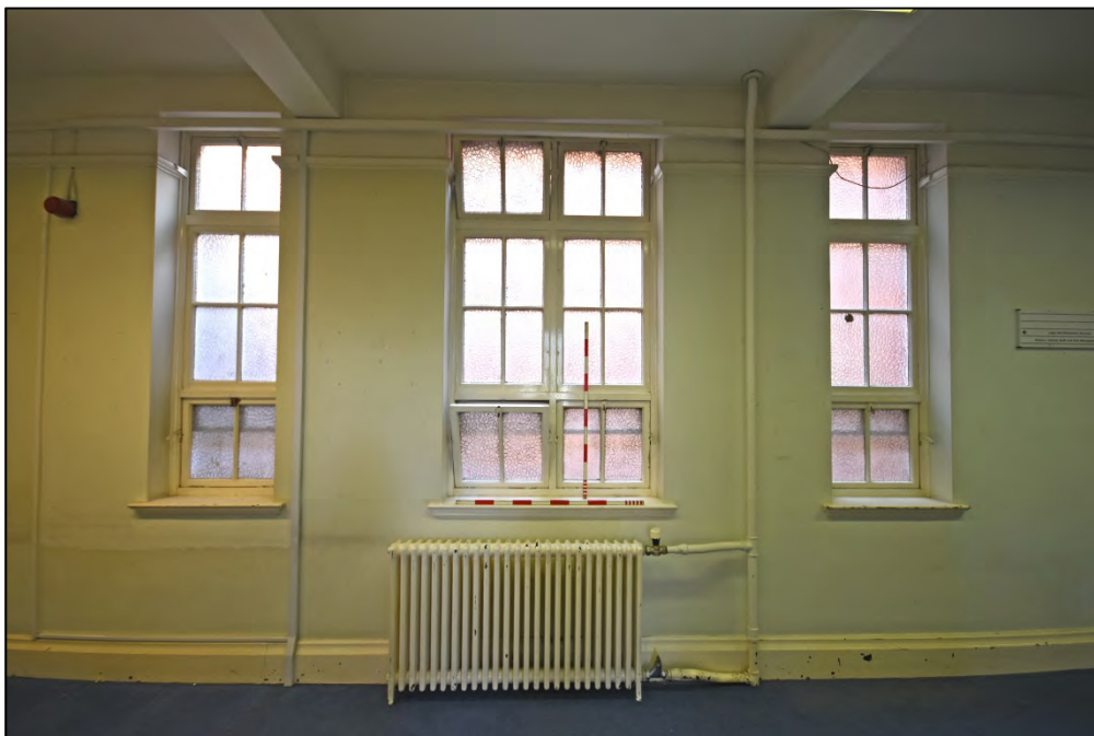
Detail of the atrium windows Fig 107
