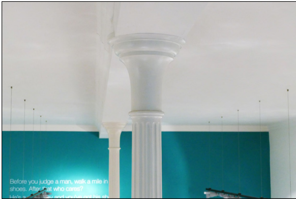
Detail of column crowns Fig 46
