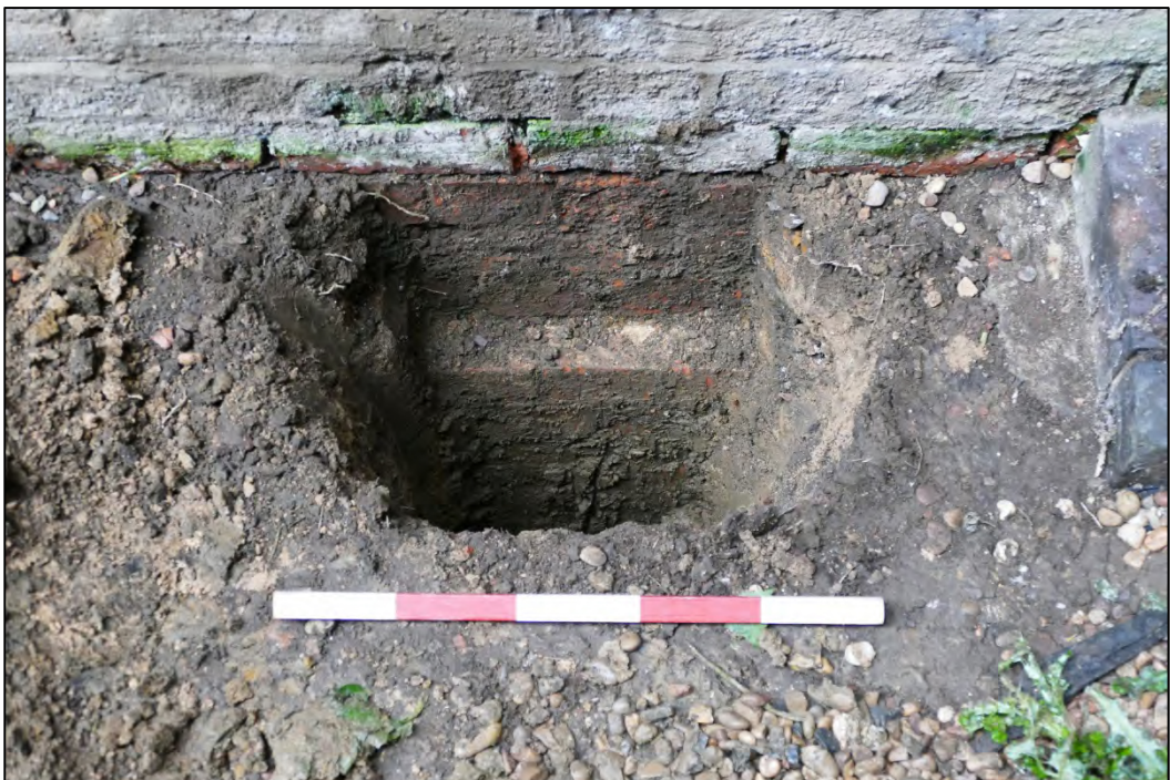
Foundation trench 4 Fig 149
