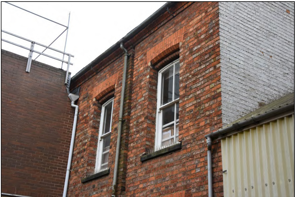
Detail of the north-facing upper floor sash windows Fig 33
