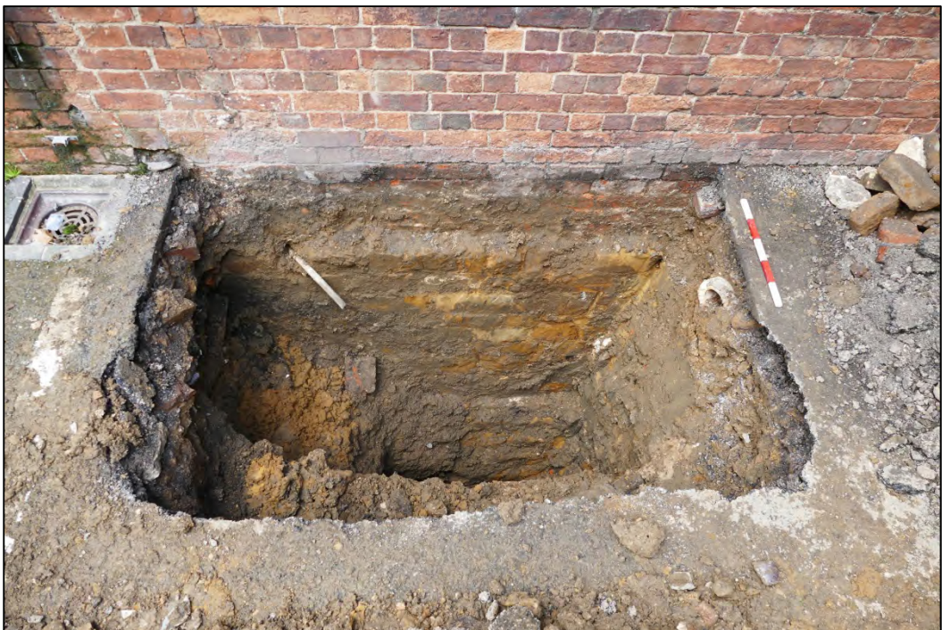
Foundation trench 2, showing the stone-built foundations Fig 145
