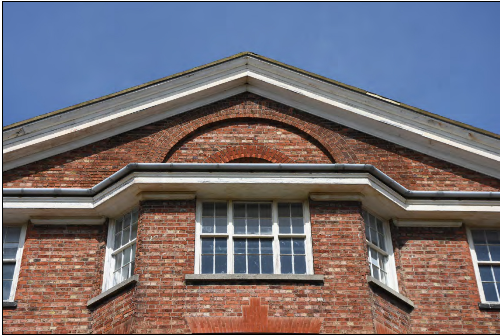
The second floor windows and gable window Fig 58
