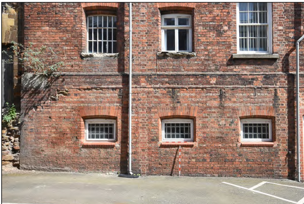
Three lower ground floor gaol windows with scar of former hanging shed platform above, with scar of former steps to the left. Note the blocked drain chase Fig 61
