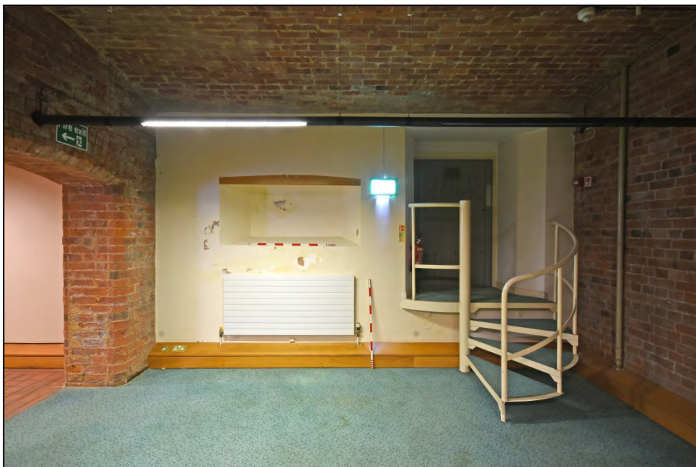
Blocked window to the north and adjacent doorway to enclosed passage Fig 87
