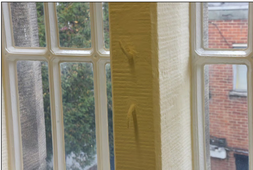
Detail of the bars, mullion, and small iron hooks embedded in the mullion Fig 121
