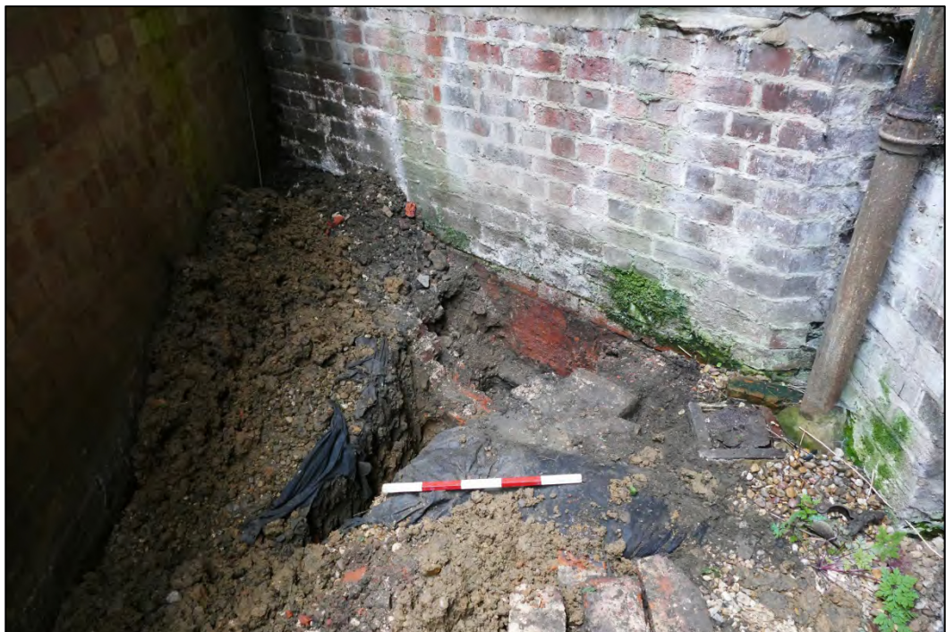
Foundation trench 3 Fig 147
