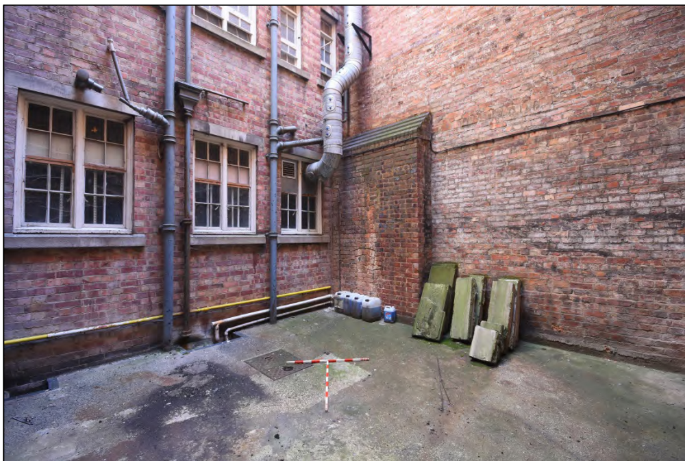
The atrium, looking north-east Fig 71
