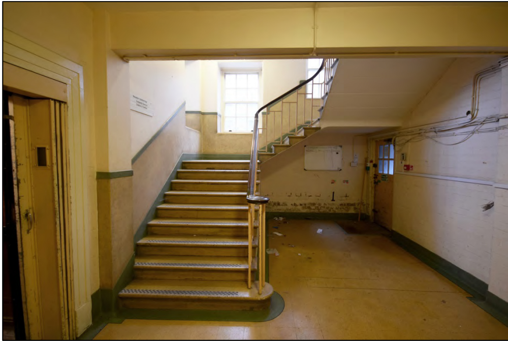
The main stair at basement level Fig 124
