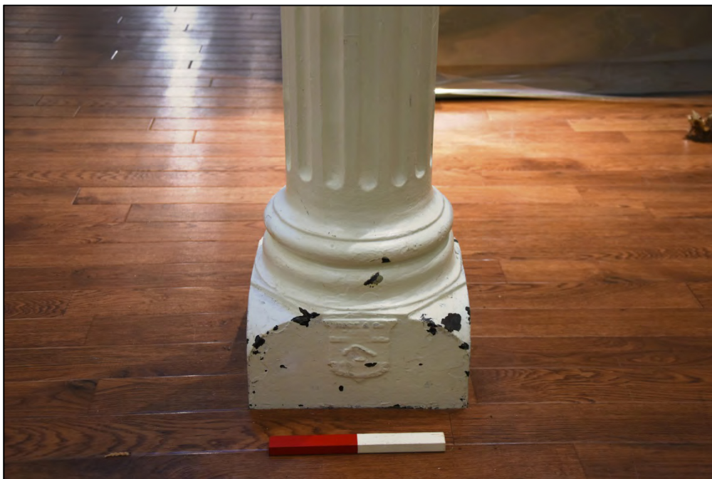
Detail of column base, showing the mark of the Eagle Foundry Fig 45
