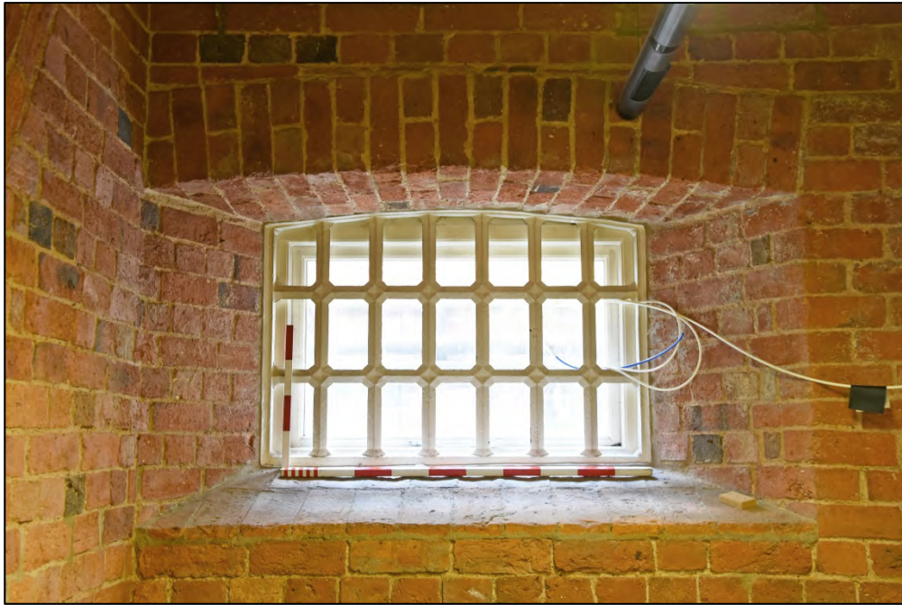
Detail of gaol window with iron bars Fig 86
