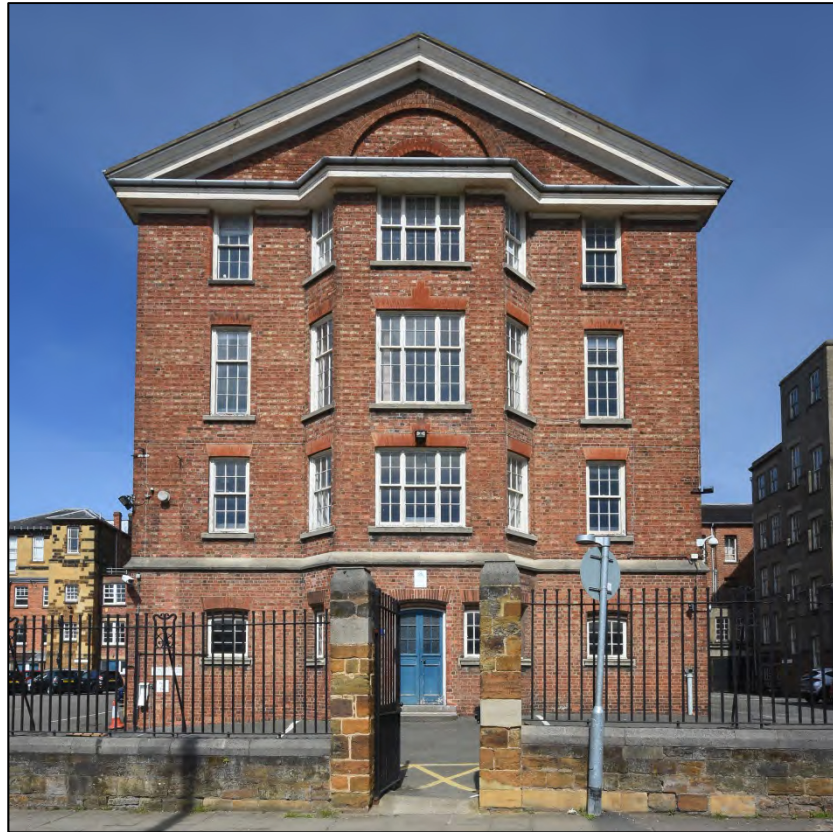
The south elevation of the west wing Fig 56
