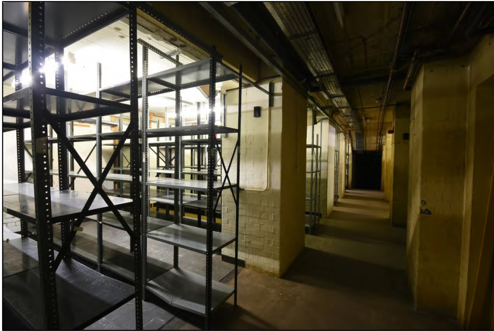
Basement storage area Fig 128
