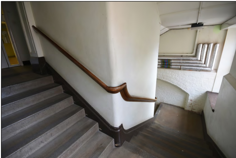
View of staircase between basement and ground floor Fig 89
