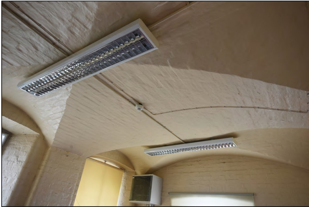
Detail of ceiling vaulting Fig 82
