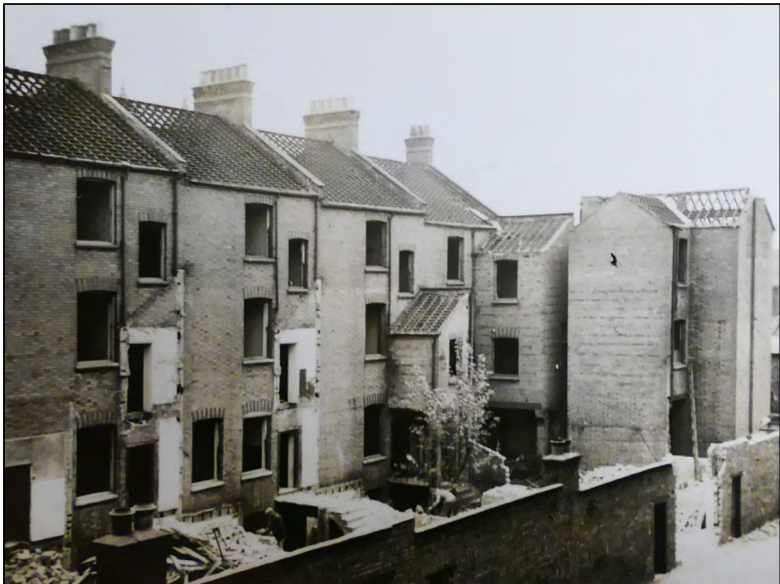
The Guildhall Road row of terraced houses during demolition, c1935 (Local Studies Library PH/198/T/119) Fig 23
