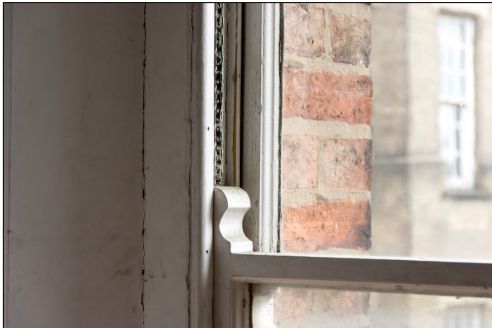
Detail of sash horn and sash chain Fig 35
