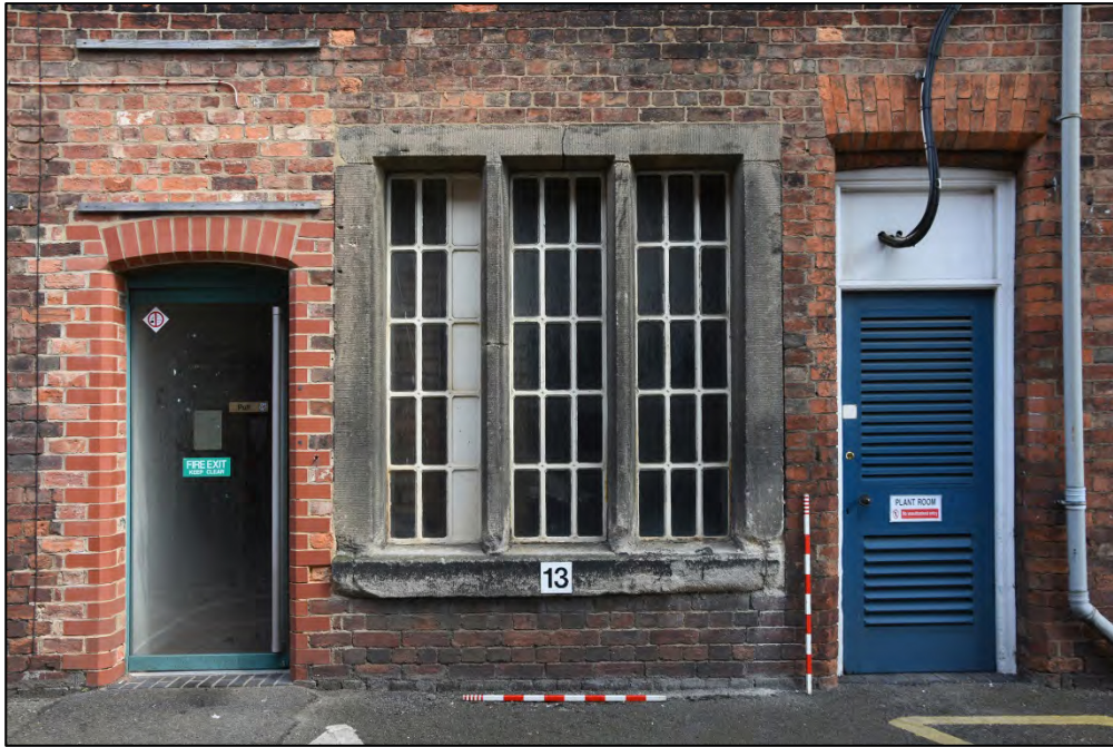
Chamfer-moulded cast-stone mullioned window Fig 66
