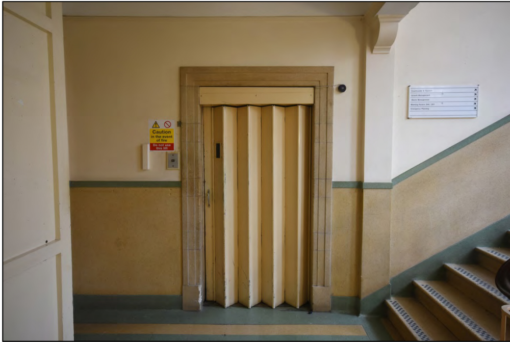
Tiled surround to the first floor lift access Fig 126
