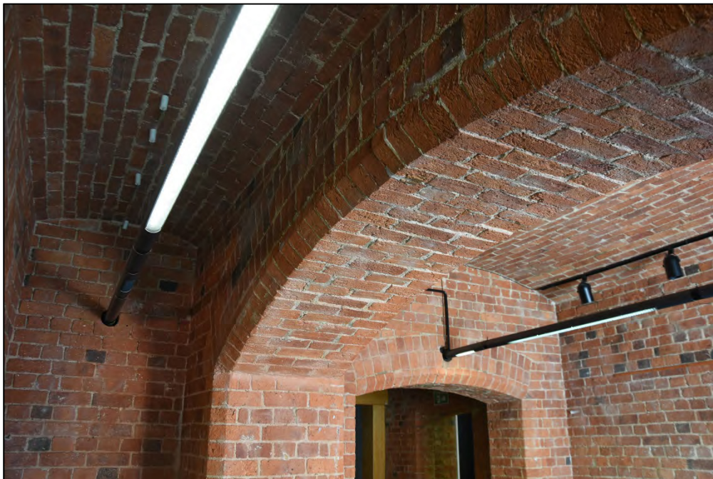
The jack vaulted ceiling Fig 85
