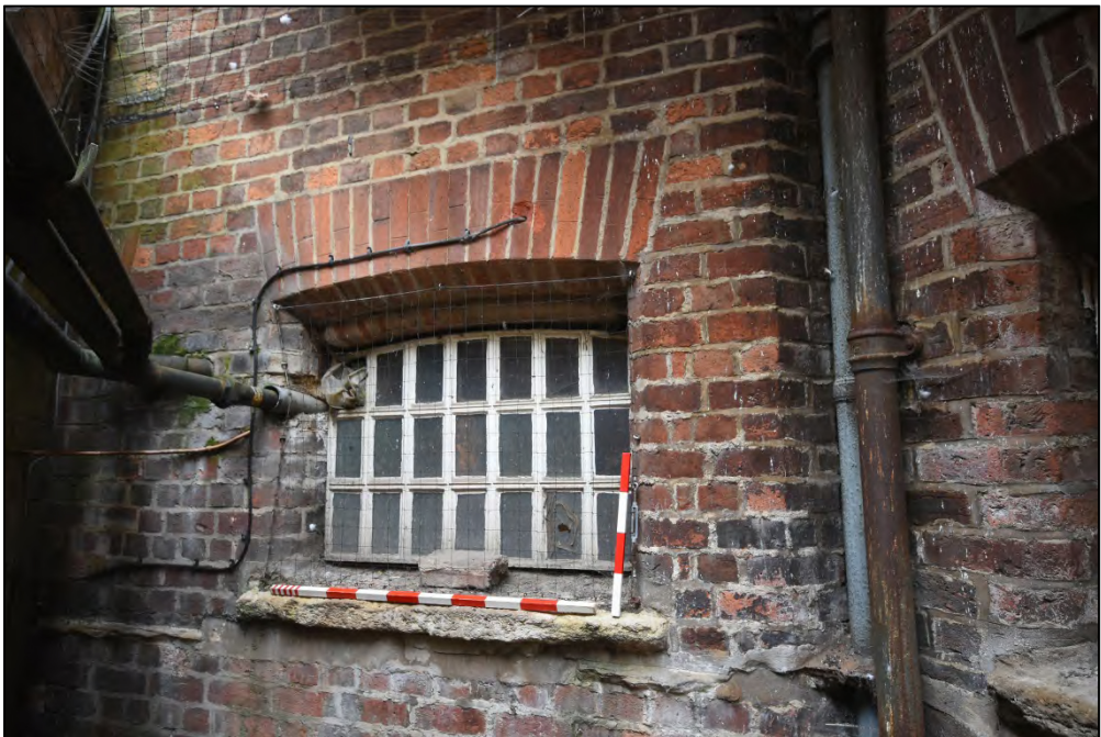
Example of the pivoting gaol windows Fig 29
