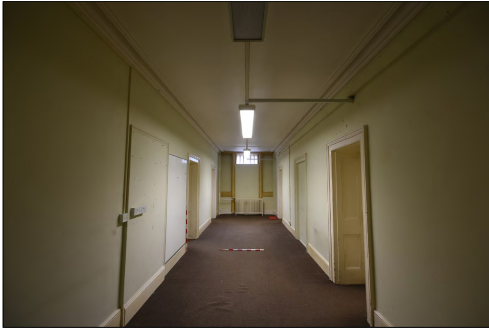
The north corridor with rooms to each side, looking north Fig 94
