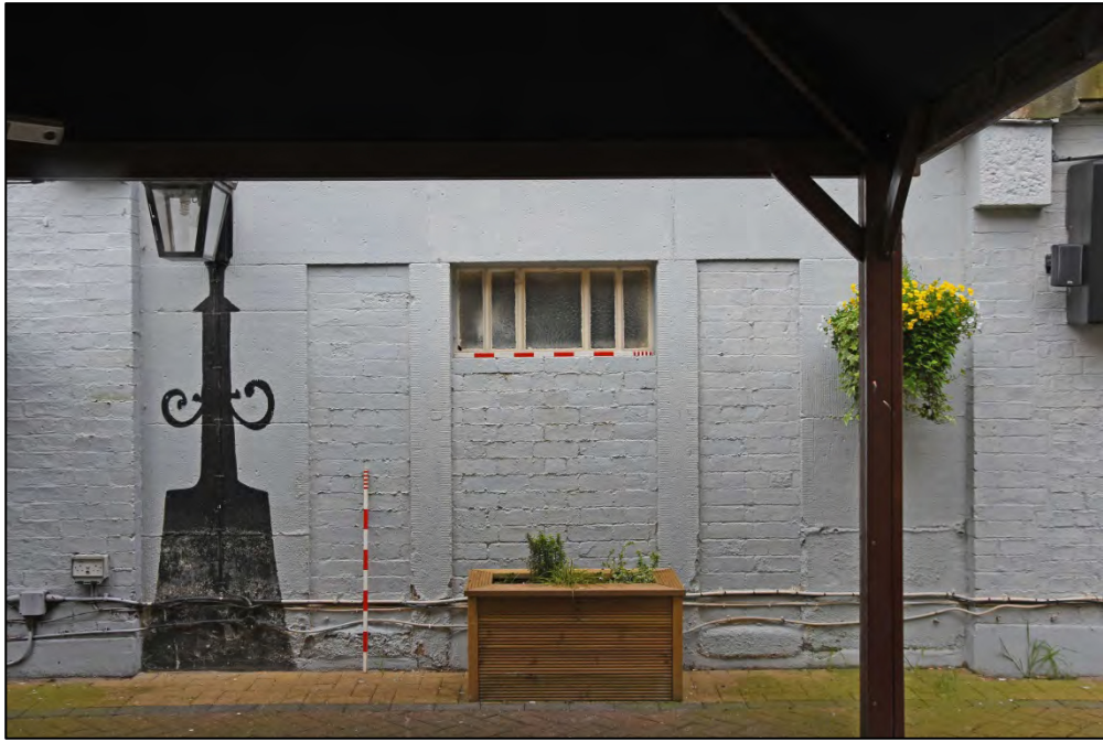
Former ground floor entrance, now blocked Fig 68
