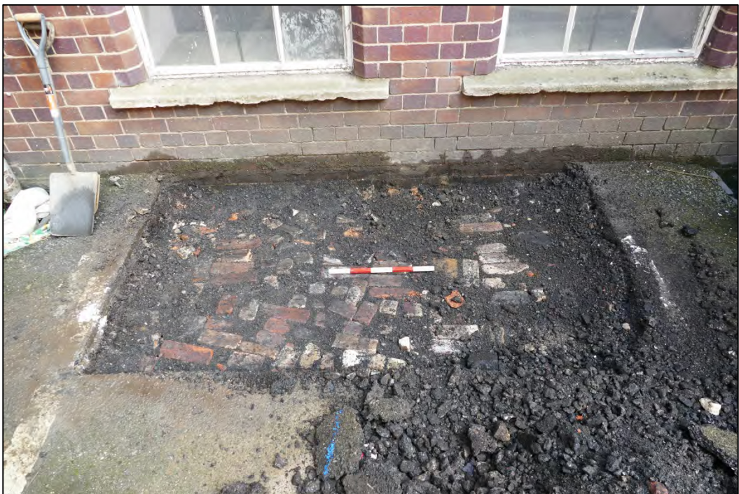
Foundation trench 1, the brick levelling layer Fig 141
