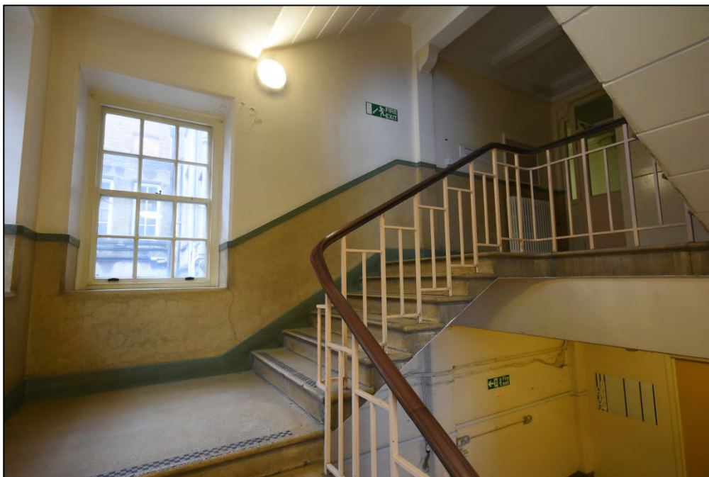
The main stair Fig 125
