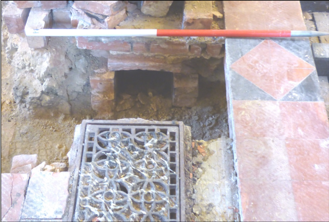
Victorian heating duct [010], looking east Fig 8
