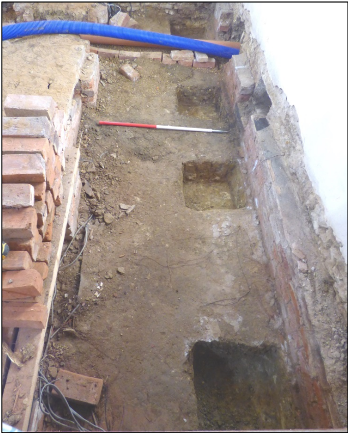
Stanchion trenches and [011], looking west Fig 9
