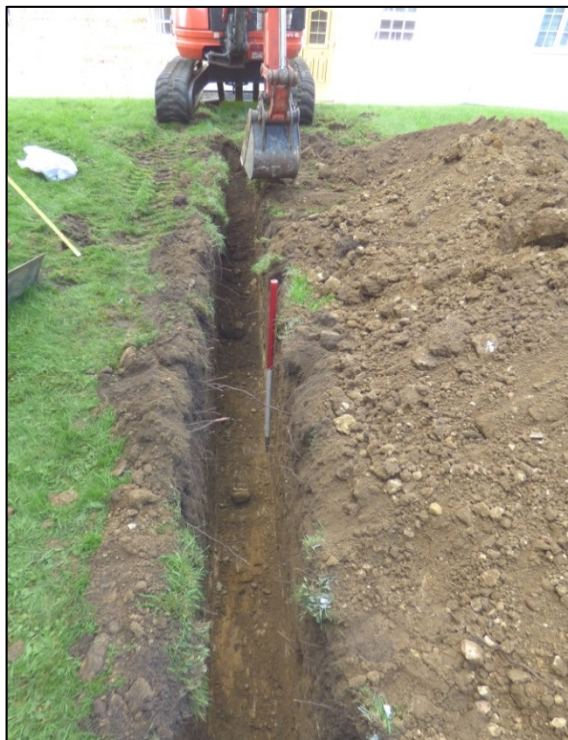
Service trench looking west Fig 3
