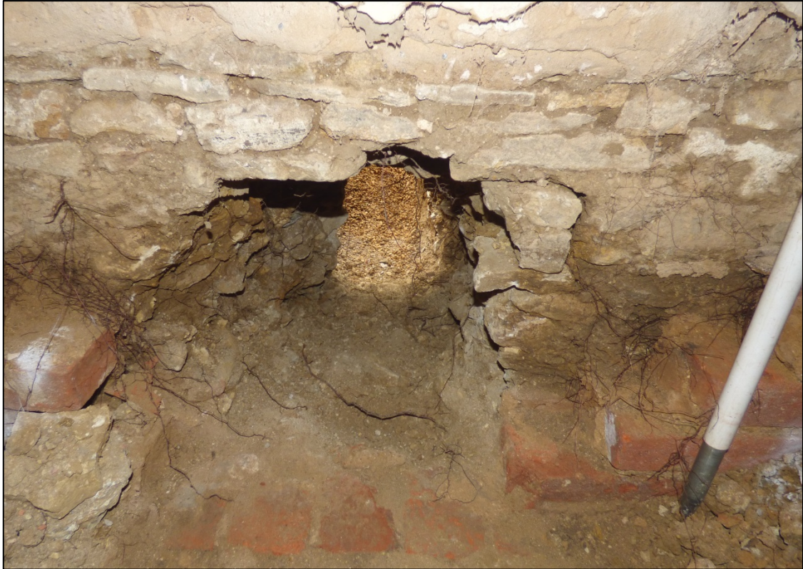
Access hole cut through north wall footings, looking north Fig 6
