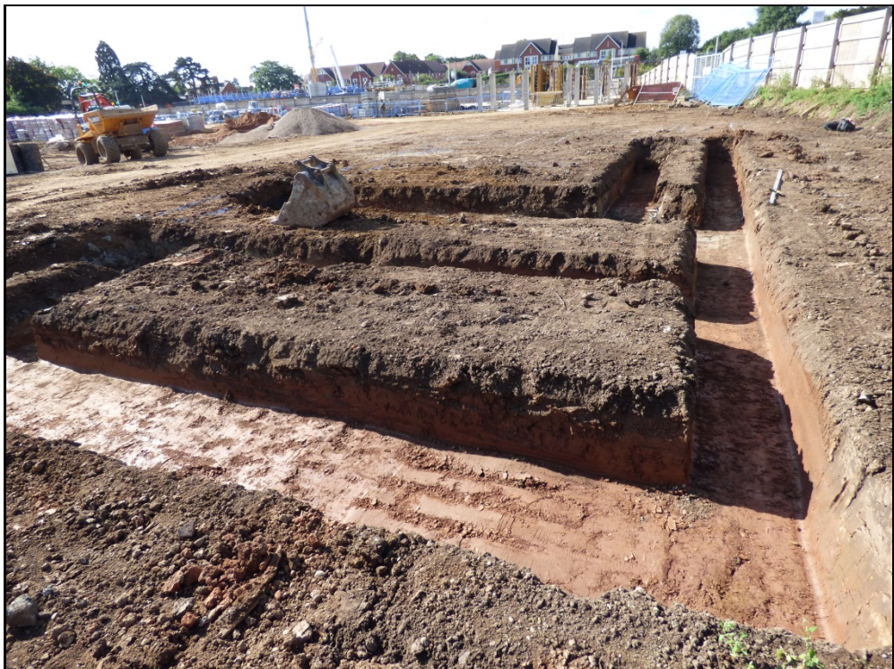
General shot of foundation trenches, looking south Fig 7
