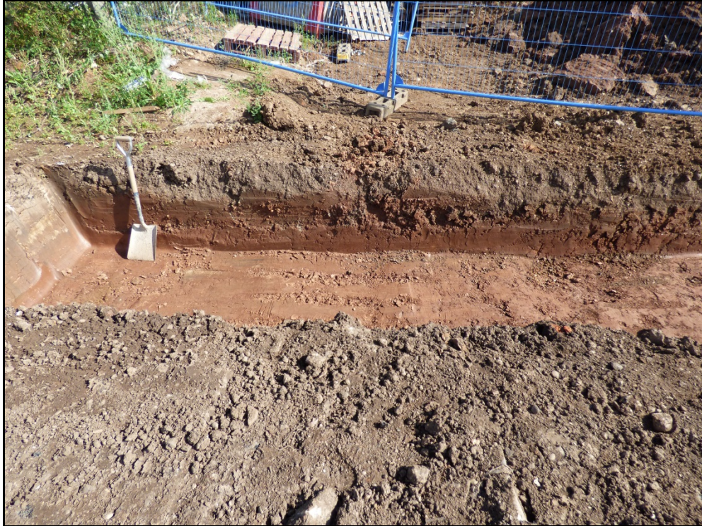
The stratigraphy within the foundation trench, looking north Fig 8
