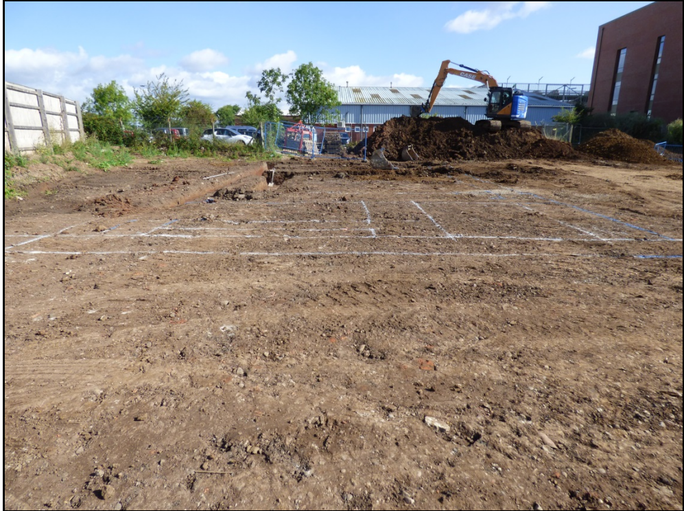
General shot of foundation trenches, looking north Fig 6
