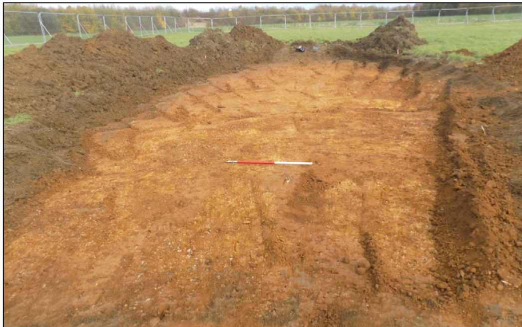
Trench 2 (eastern pond) showing excavated base, looking east Fig 4
